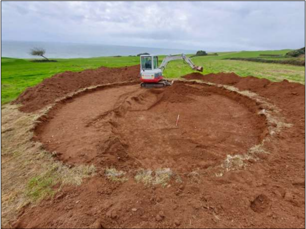
FIGURE 2: WORKS IN PROGRESS, VIEWED FROM THE EAST (1M SCALE).
