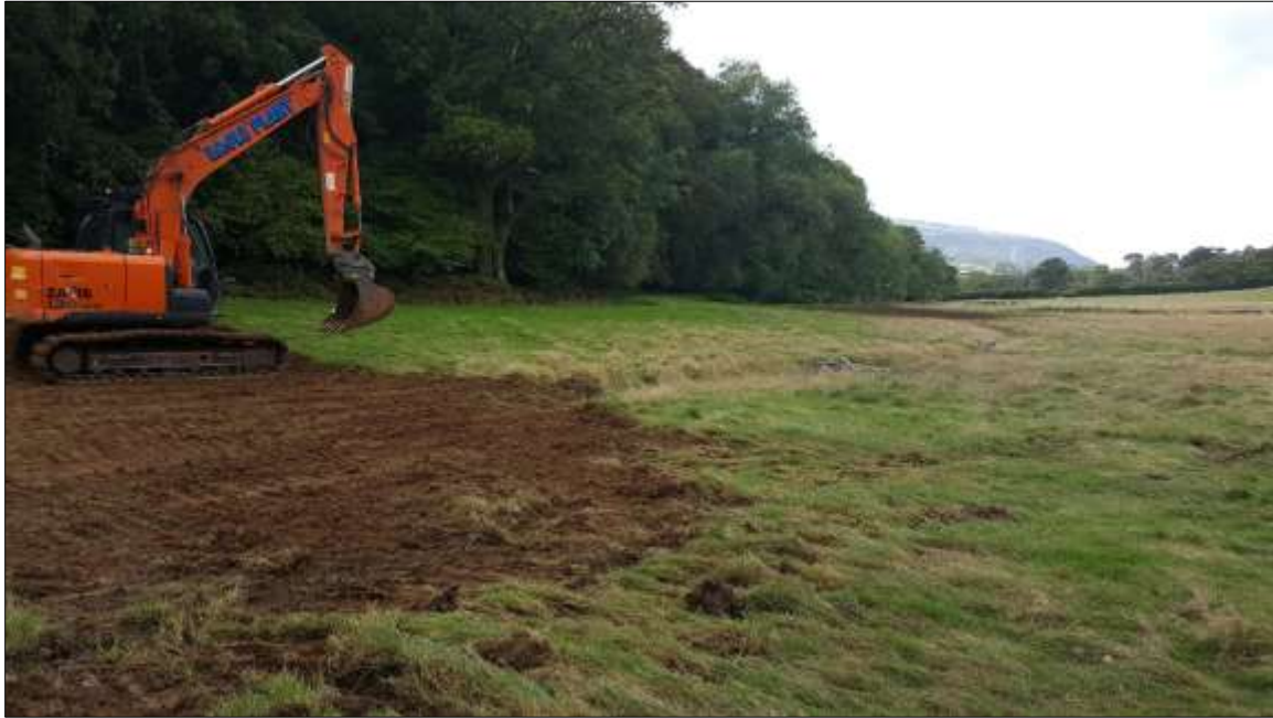
FIGURE 4: BACKFILLING PROGRESS; VIEWED FROM THE NORTH-EAST (NO SCALE).
