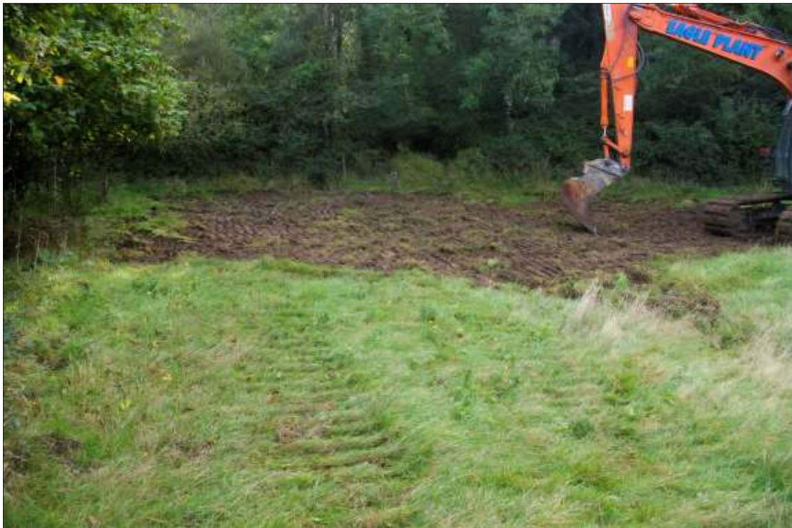
FIGURE 3: START OF BACKFILLING; VIEWED FROM THE NORTH-WEST (NO SCALE).
