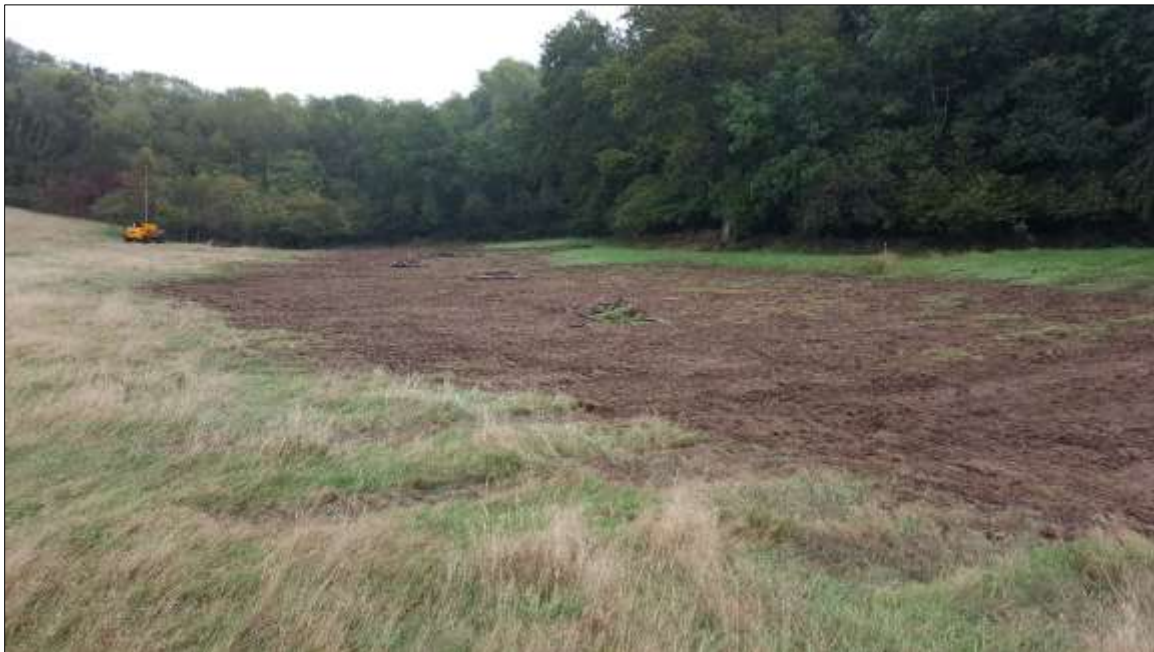
FIGURE 9: AREA SHOT, POST-BACKFILL; VIEWED FROM THE WEST (NO SCALE).
