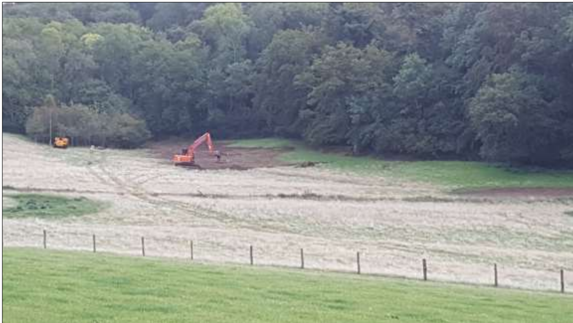
FIGURE 7: AS ABOVE; VIEWED FROM THE NORTH-WEST (NO SCALE).
