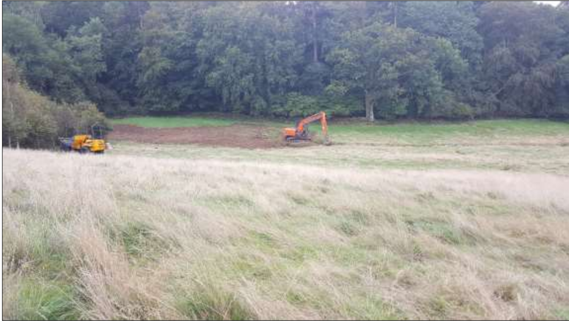
FIGURE 6: BACKFILLING PROGRESS AND AREA SHOT; VIEWED FROM THE NORTH (NO SCALE).
