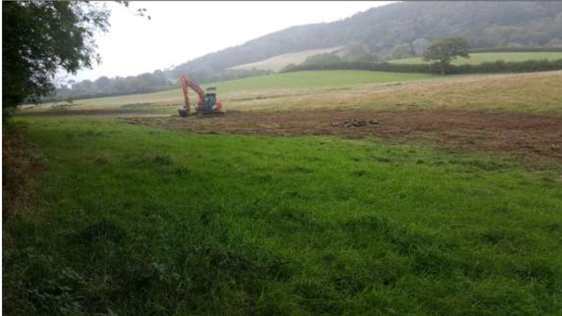
FIGURE 8: BACKFILLING PROGRESS; VIEWED FROM THE SOUTH (NO SCALE).
