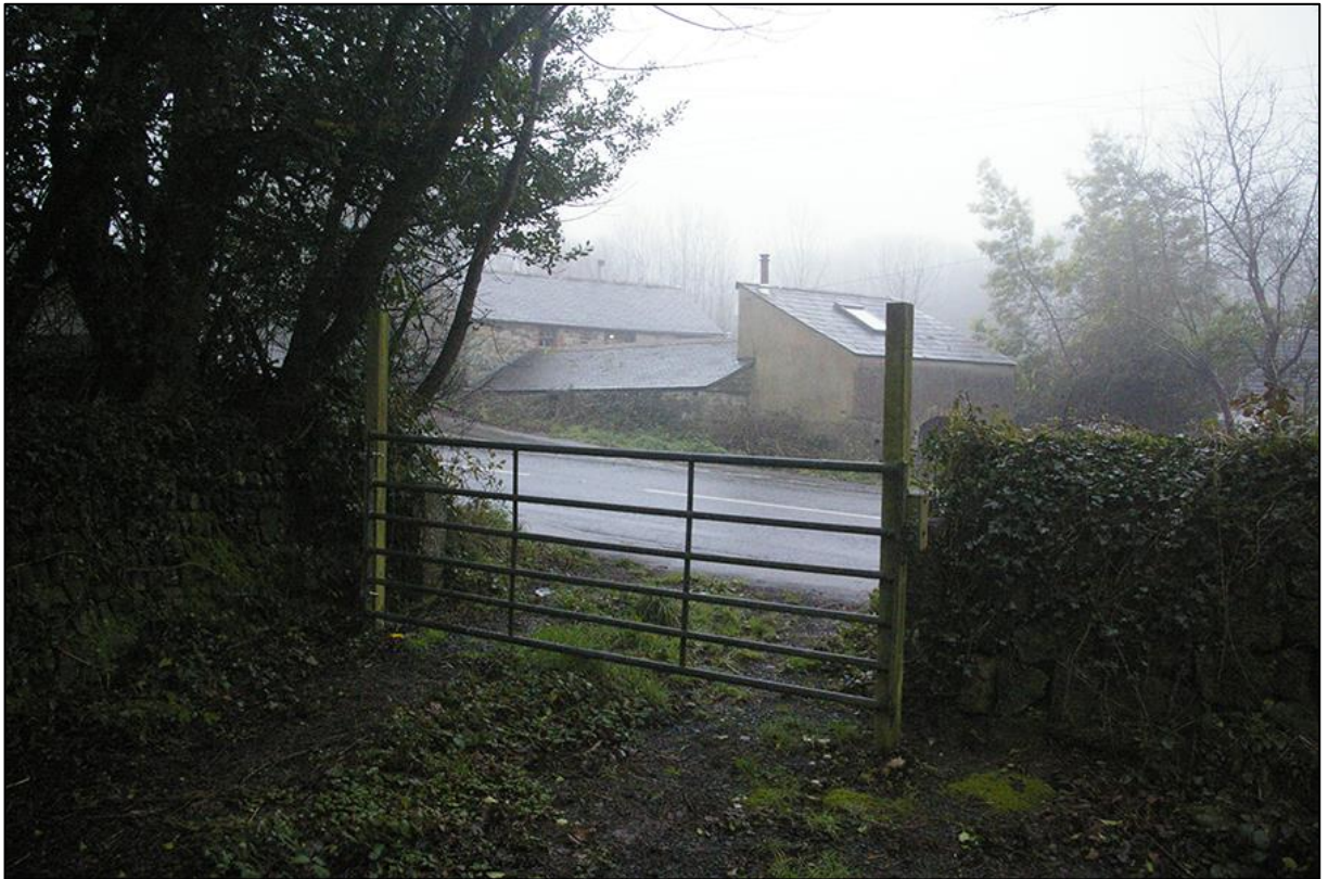
1. SITE ENTRANCE FROM OFF THE B3280, LOOKING TOWARDS NANTURRAS BARNS; VIEWED FROM THE NORTH-WEST (NO SCALE).
