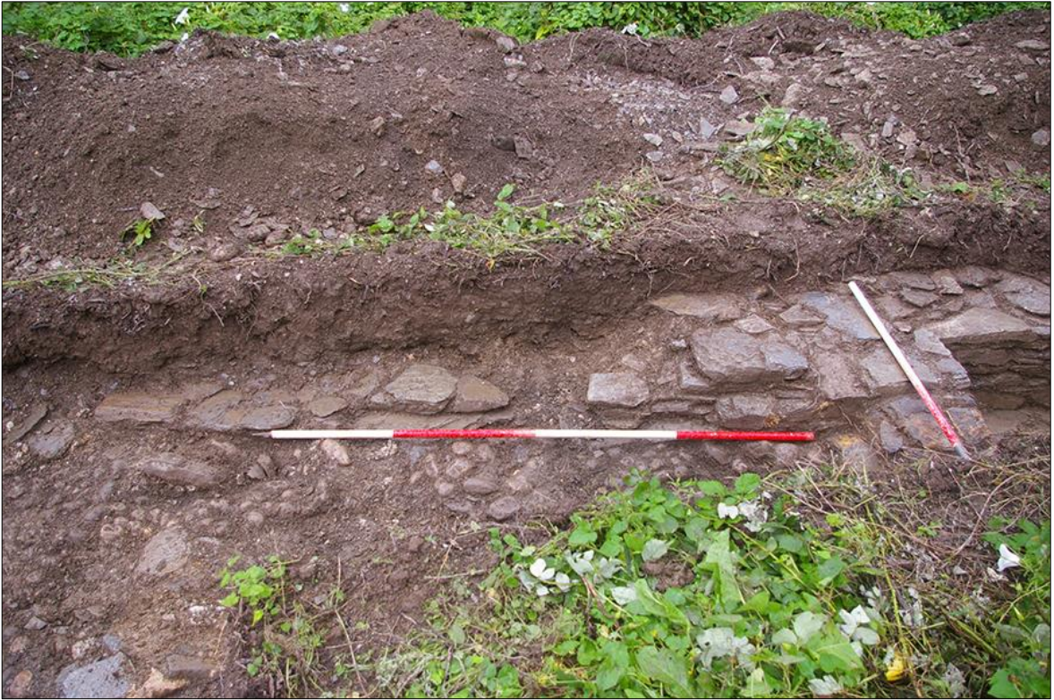
17. STRUCTURE <S2> SHOWING WALLS {120} AND {121} ABUTTING STRUCTURE <S1>; VIEWED FROM THE WEST-SOUTH-WEST (1M & 2M SCALES).
