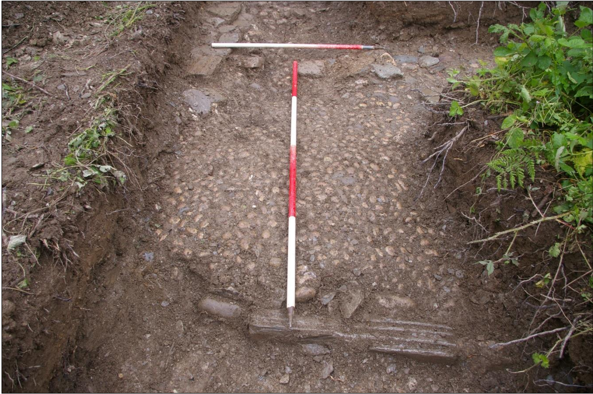
FIGURE 5: THE NORTHERN END OF STRUCTURE <S2>; VIEWED FROM THE NORTH (1M & 2M SCALES).
