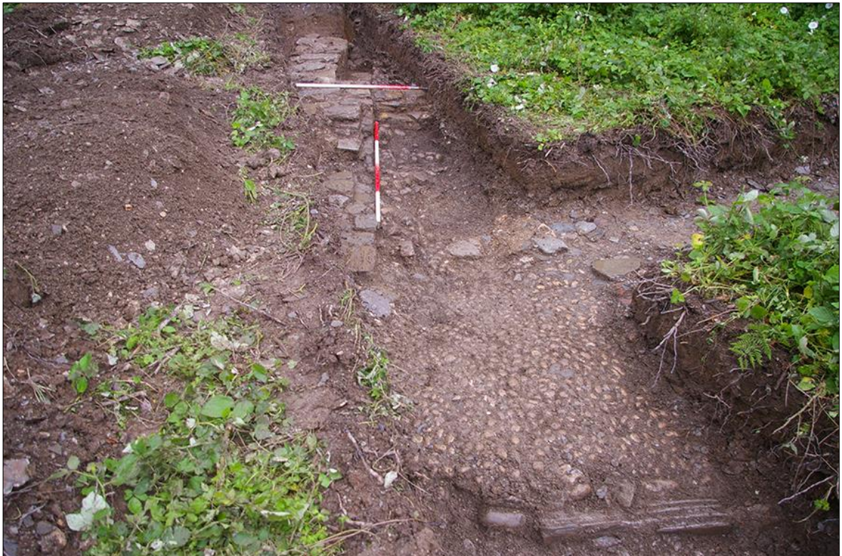
16. STRUCTURE <S2> SHOWING COBBLE FLOOR (122)/(124) AND WALLS {120}, {121} AND {123} ABUTTING STRUCTURE <S1>; VIEWED FROM THE NORTH (2M SCALE).
