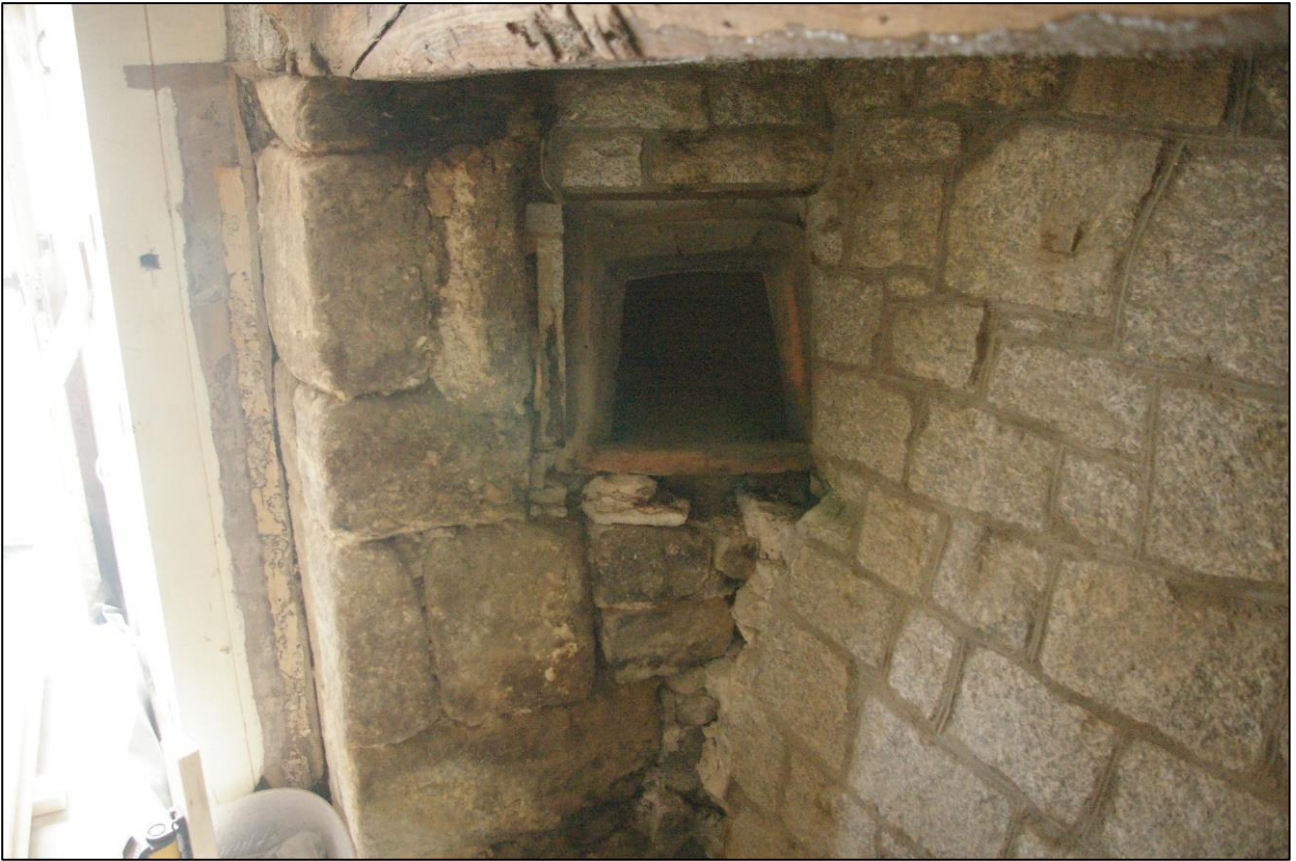
25. R2, DETAIL OF THE OVEN IN THE FIREPLACE TO THE EAST GABLE WALL; VIEWED FROM THE SOUTH-WEST.
