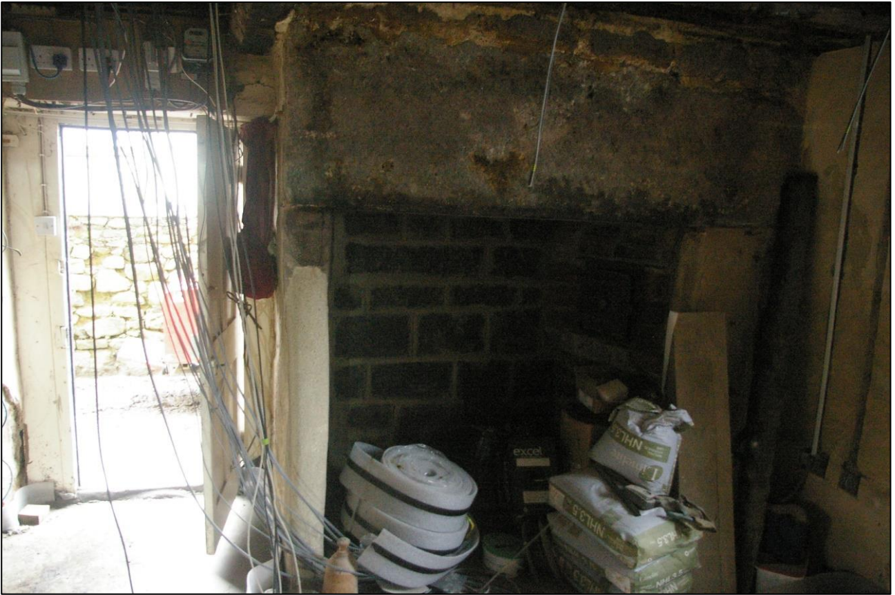
11. R1, DETAIL OF THE FIREPLACE IN THE WEST GABLE WALL WITH GRANITE LINTEL AND SHAPED CORBELS; VIEWED FROM THE SOUTH-EAST.
