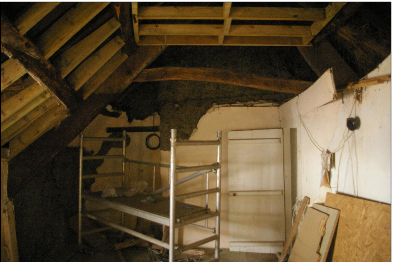
36. R4, DETAIL OF THE EAST GABLE; VIEWED FROM THE WEST.
