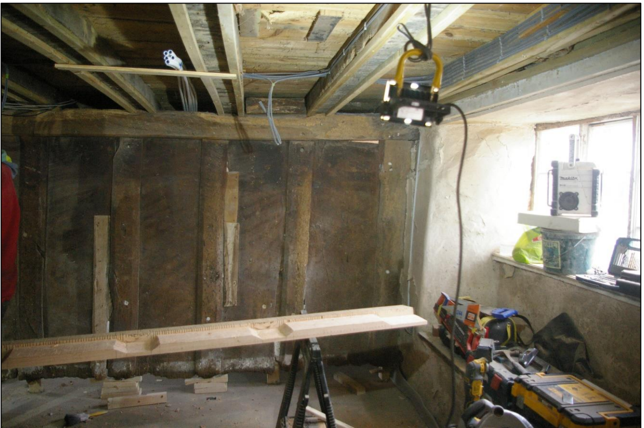
18. R2, THE PLANK AND MUNTIN SCREEN PARTITION BETWEEN R1 AND R2; VIEWED FROM THE EAST.
