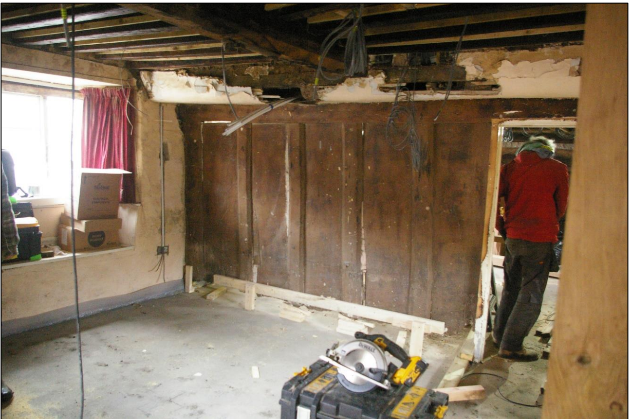
16. R1 DURING REMEDIAL WORKS; VIEWED FROM THE SOUTH-WEST.
