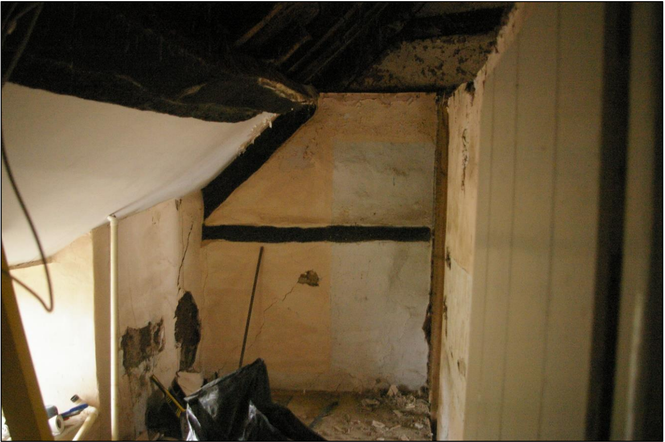
39. R5, DURING REMEDIAL WORKS; VIEWED FROM THE EAST.
