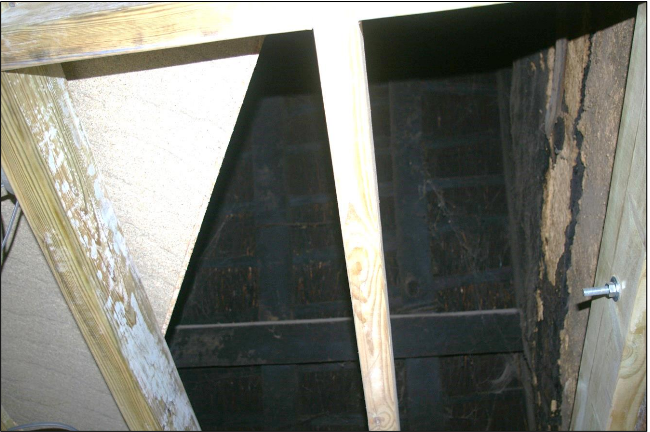
31. R3, DETAIL OF THE HEAVILY SMOKE-BLACKENED THATCH ABOVE THE ROOM; VIEWED FROM THE SOUTH-EAST.
