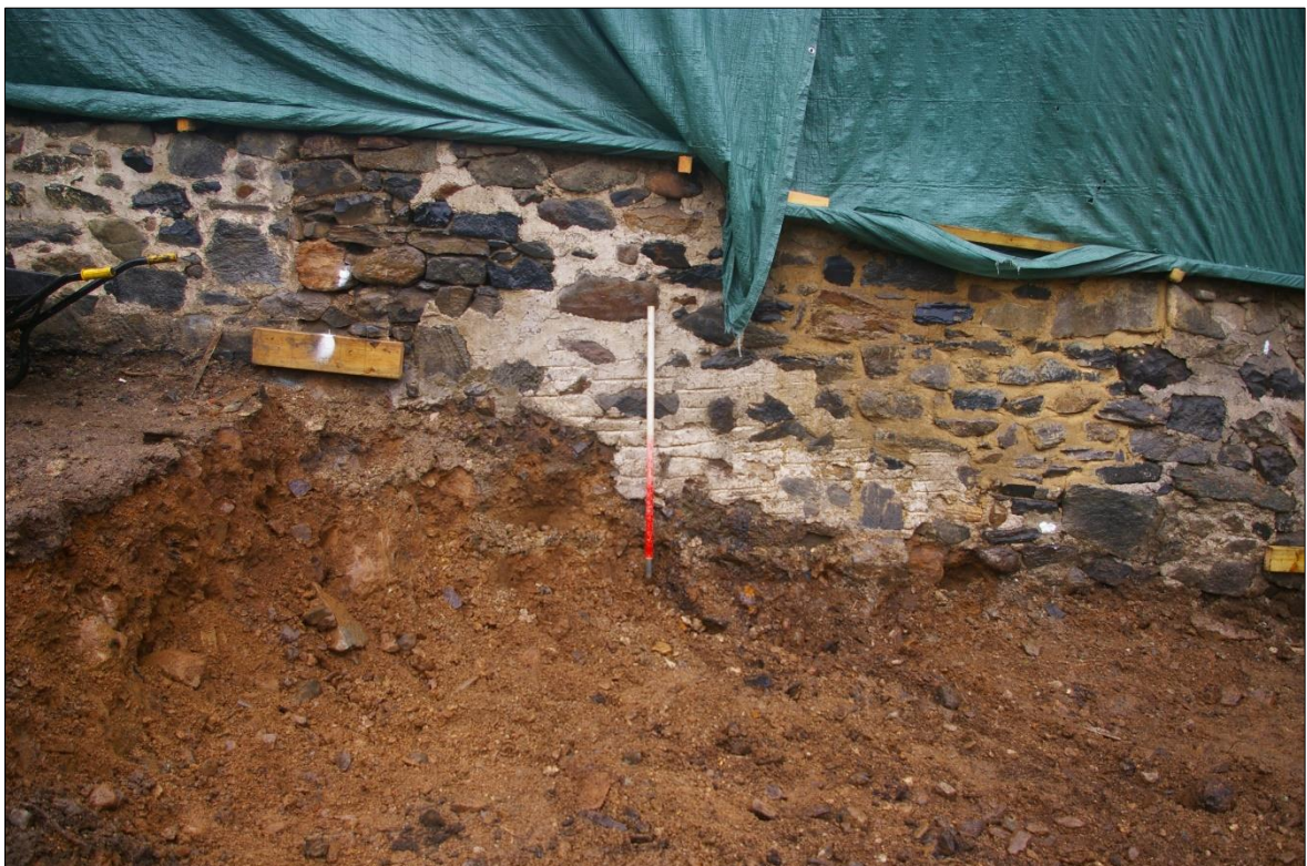
FIGURE 3: AREA 01, WEST FACING SECTION SHOWING EXISTING EAST PROPERTY BOUNDARY WALL CONSTRUCTED DIRECTLY OVER THE NATURAL, AND EXTENT OF TERRACING FOR THE 20 TH CENTURY OUTBUILDINGS; VIEWED FROM THE WEST (1M SCALE).
