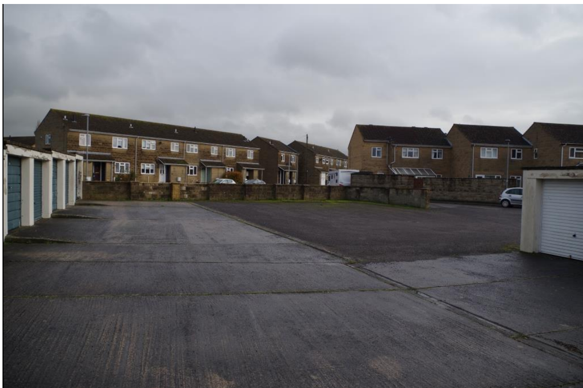
FIGURE 9: CONCRETE SURFACES, DRAINS AND GARAGES OCCUPYING THE SITE CURRENTLY, VIEWED FROM THE SOUTH-WEST.
