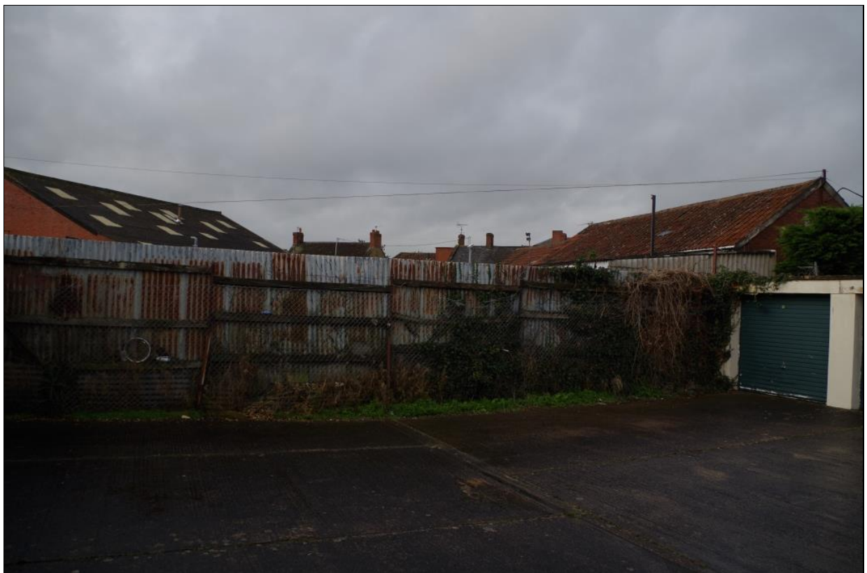
2. THE SOUTH-WEST BOUNDARY TO THE SITE, VIEWED FROM THE NORTH-EAST.
