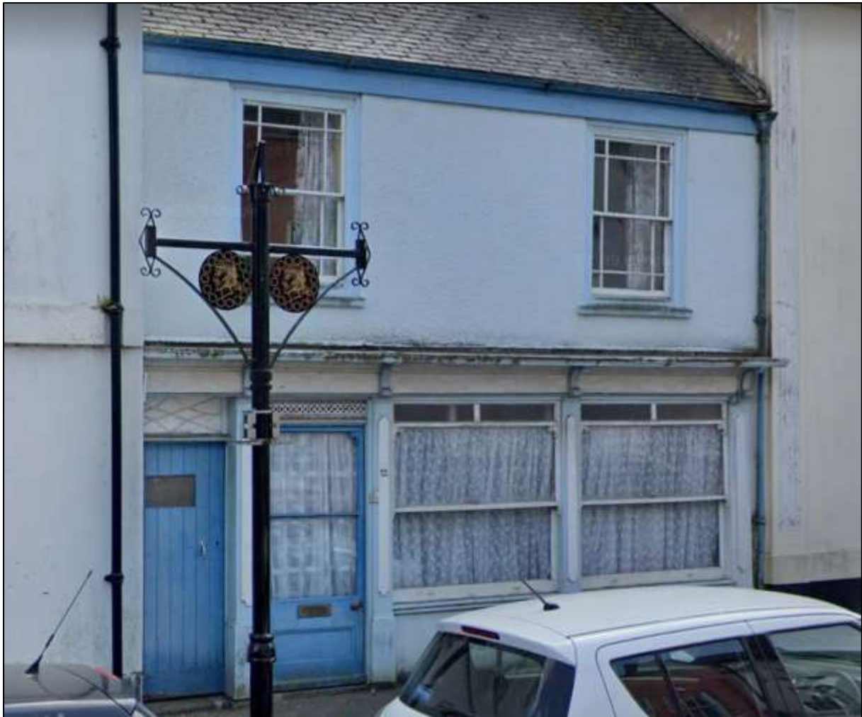
FIGURE 2: FRONT ELEVATION OF 22 BROAD STREET; VIEWED FROM THE NORTH (©GOOGLE STREETVIEW).
