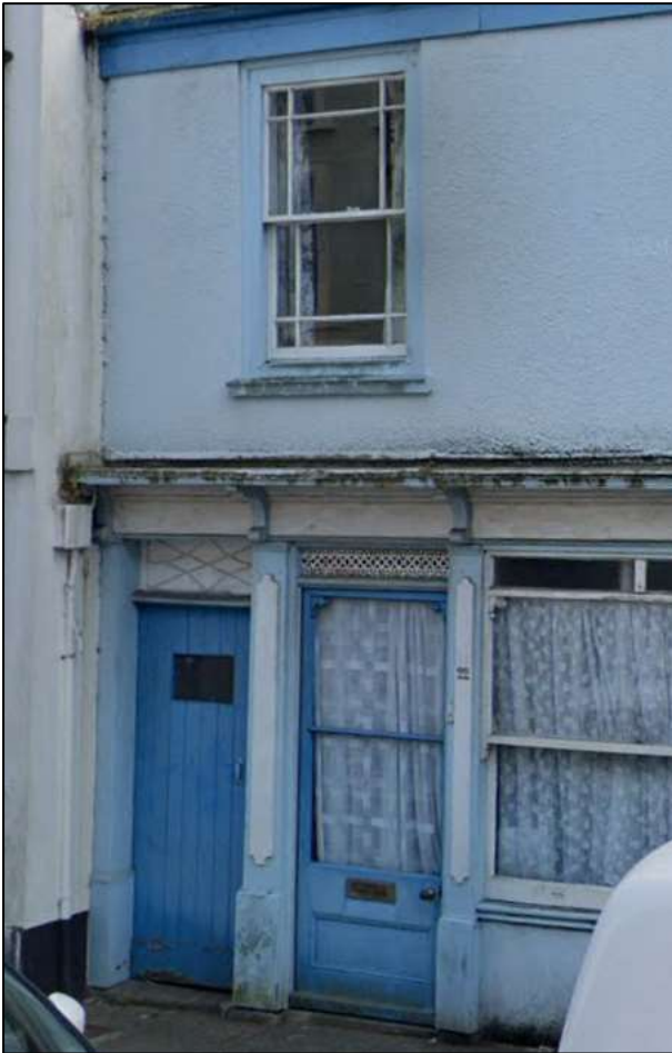
FIGURE 3: DETAIL OF EAST END OF FRONTAGE; VIEWED FROM THE NORTH-WEST. NOTE THE EARLIER 19 TH CENTURY INTERLACED TOPLIGHT OVER THE HOUSE DOOR TO LEFT, AND MID-19 TH CENTURY HORNLESS SASH WITH VERGE LIGHTS ABOVE. CAST IRON GRILLE OVER LATER 19 TH CENTURY SHOP DOOR FORMERLY CONTINUED ACROSS THE SHOP WINDOWS, NOW GLAZED (©GOOGLE STREETVIEW).
