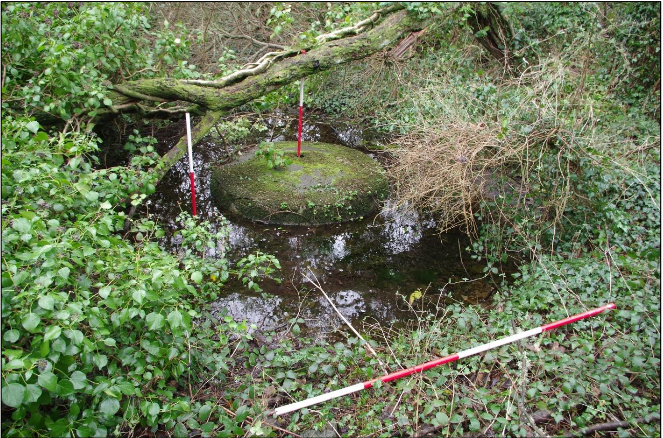
9. 1920s-30s ROUND BUDDLE ON WET DRESSING FLOOR DF3; VIEWED FROM THE SOUTH (SCALES 2M & 1M).
