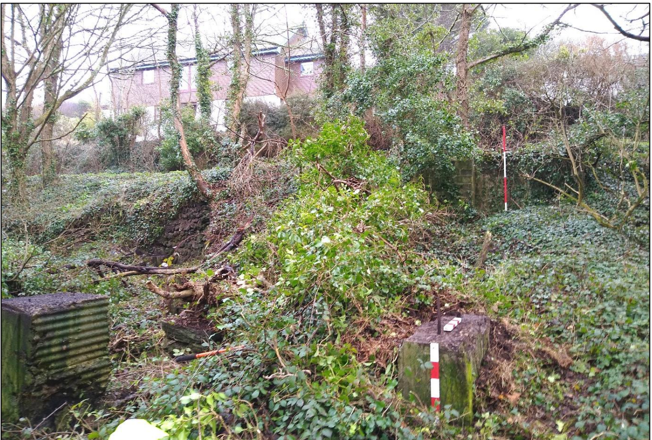
12. CONCRETE STANDS FOR 1920s-30s DRIVE-SHAFT IN FOREGROUND (0.5M SCALE) AND HEADER TANKS FOR WATER TURBINE AND WET DRESSING BESIDE ROAD BEYOND (2M SCALE). VIEWED FROM THE NORTH-WEST.
