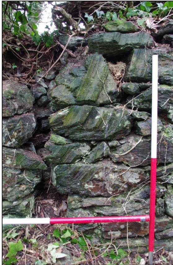
3. SCORE MARKS FROM A 10FT 6IN DIAMETER WATER WHEEL IN WP2; VIEWED FROM THE NORTH-EAST (SCALES 1M).
