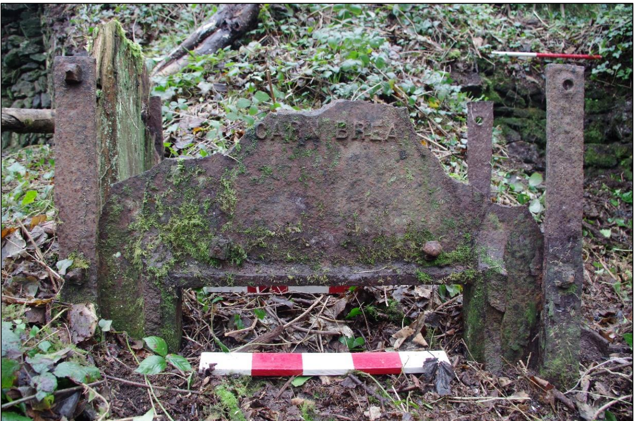
6. CAST IRON THROAT PLATE OF STAMPS BOX; VIEWED FROM THE NORTH-WEST (SCALE 0.5M).
