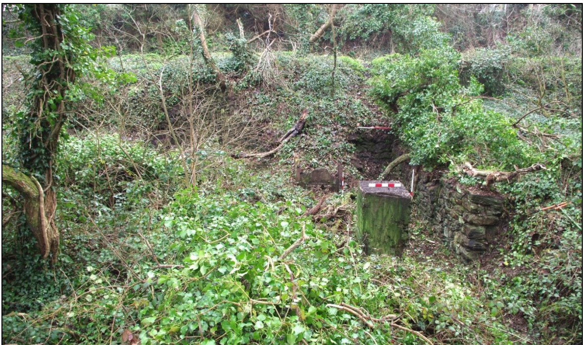
FIGURE 8: WHEEL PIT 2, GENERAL VIEW FROM NORTH-WEST WITH 1920s-30s CONCRETE STAND FOR DRIVE-SHAFT IN FRONT OF LATE 19 TH CENTURY MASONRY PIT. PERRANCOOMBE LANE RUNS ALONG THE TERRACE BEHIND.
