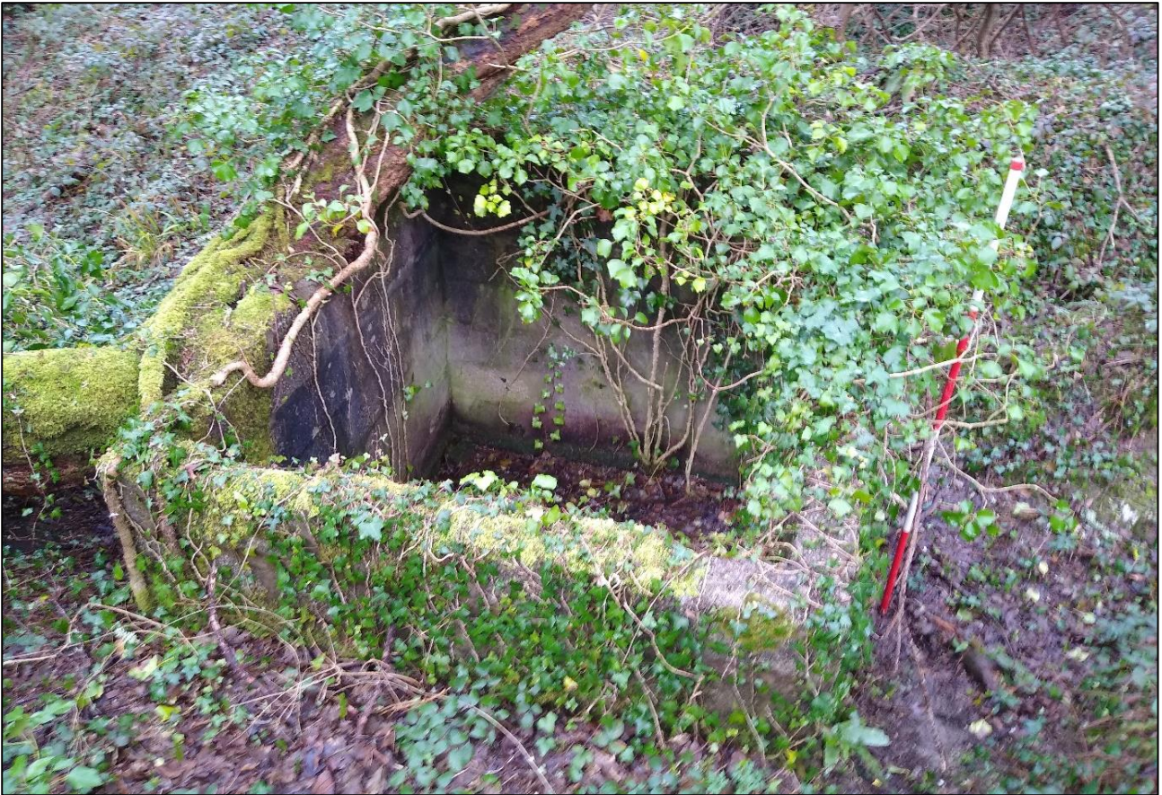
11. 1920s-30s CONCRETE TURBINE HOUSE WITH HOLES FOR AXLES; VIEWED FROM THE SOUTH-WEST (SCALE 2M).
