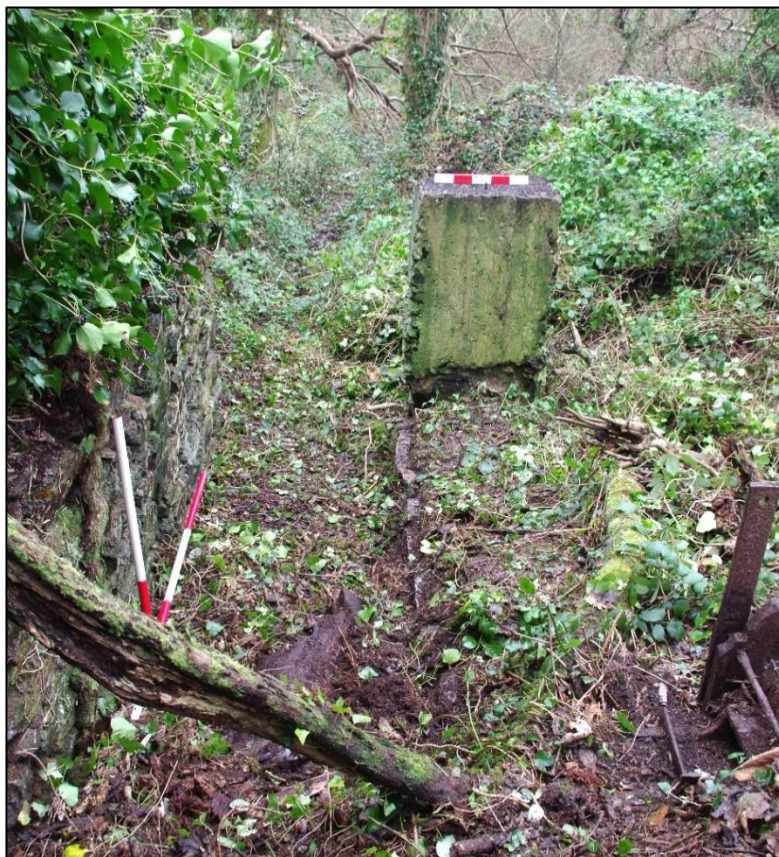
4. VIEW ALONG WATER WHEEL PIT 2 FROM THE SOUTH-EAST, WITH STAMPS BOX ON EXTREME RIGHT (SCALES 2M, 1M AND 0.5M).
