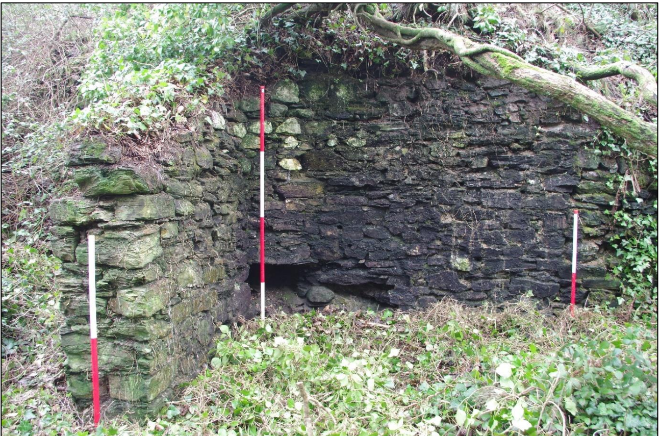
10. 19 TH CENTURY CRIB HUT B1 BUILT INTO THE RETAINING WALL OF THE TINNER'S SCARP; VIEWED FROM THE NORTH-WEST (SCALES 2M & 1M).
