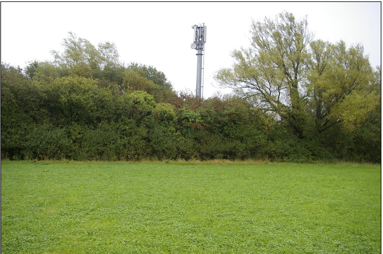
6. THE MAST WITHIN THE GAS DISTRIBUTION STATION; VIEWED FROM THE WEST (NO SCALE).
