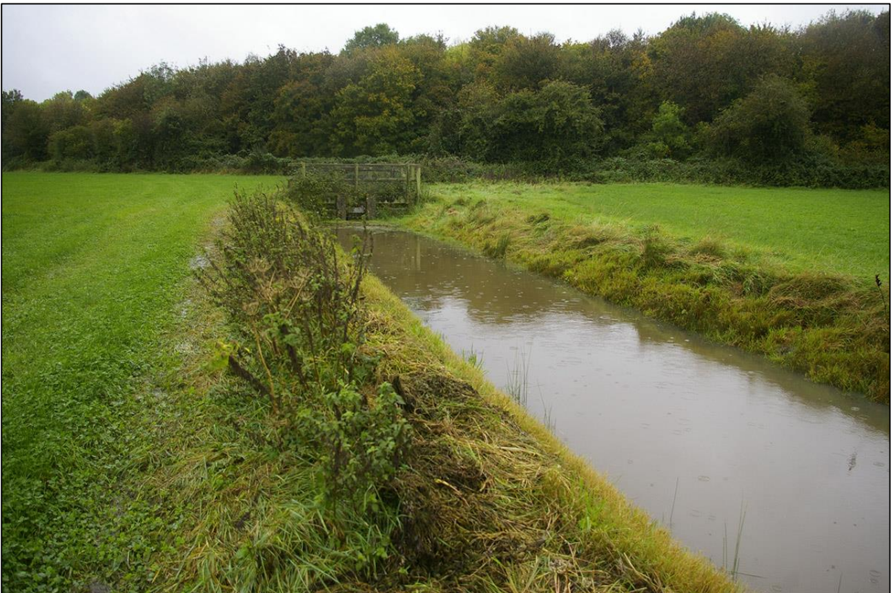
22. VIEW OF THE DRAIN AND SLUICE GATE AT THE END OF THE LARGE DITCH BETWEEN THE TWO FIELDS; VIEWED FROM THE NORTH-EAST (NO SCALE).
