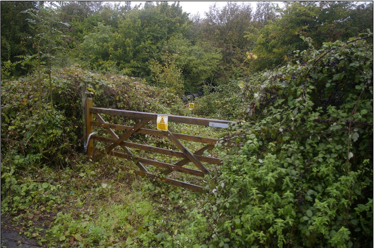
33. VIEW OF ACCESS TO THE PIPE THAT CROSSES THE RIVER BANWELL; VIEWED FROM THE NORTH-EAST (NO SCALE).
