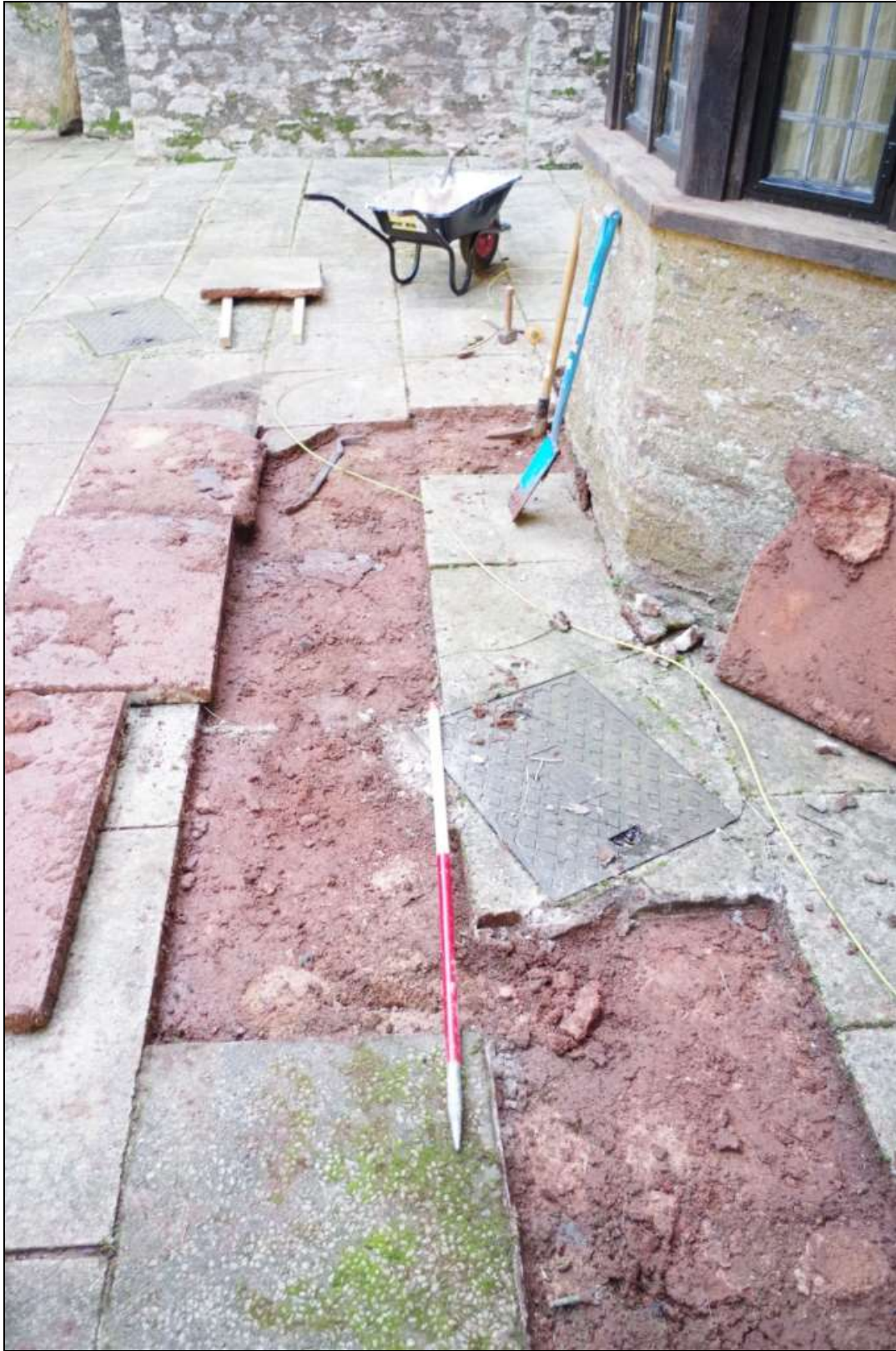
FIGURE 2: LIMIT OF EXCAVATIONS; VIEWED FROM SOUTH-WEST (1M SCALE).
