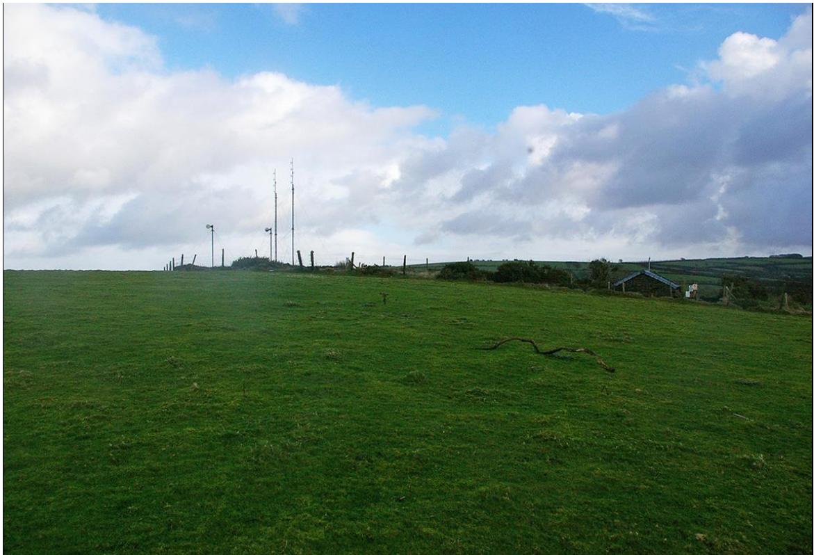
FIGURE 7: SEVERAL OTHER MASTS, A SUBSTATION AND ANTENNAE, SET ON THE FENCED WASTE GROUND AROUND THE QUARRY; VIEWED FROM THE SOUTH-WEST.
