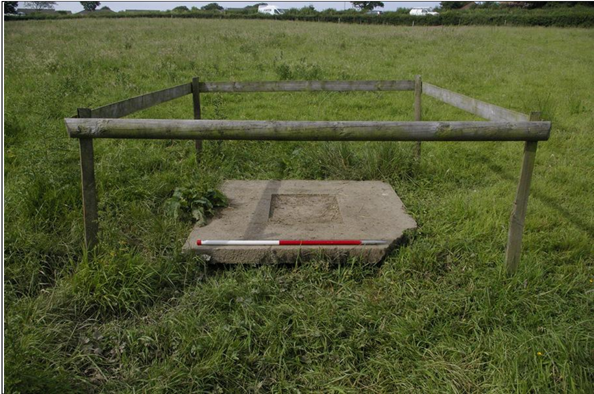
35. DETAIL OF A STORM DRAIN TOWARDS THE SOUTH-WEST CORNER OF F2; VIEWED FROM THE SOUTH (1M SCALE).
