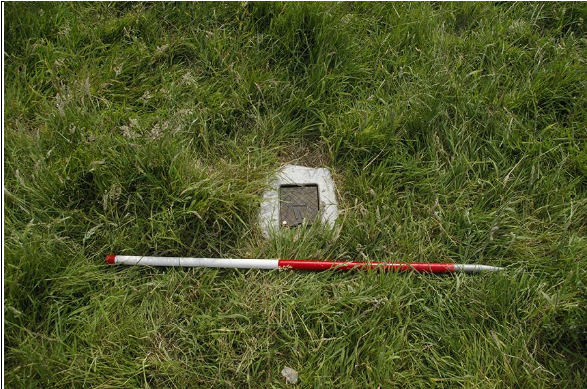
25. DETAIL OF A WATER INSPECTION POINT WITHIN F2; VIEWED FROM THE EAST (1M SCALE).
