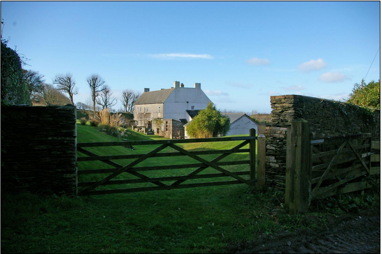
19. RAME BARTON, VIEWED FROM THE EAST-SOUTH-EAST.
