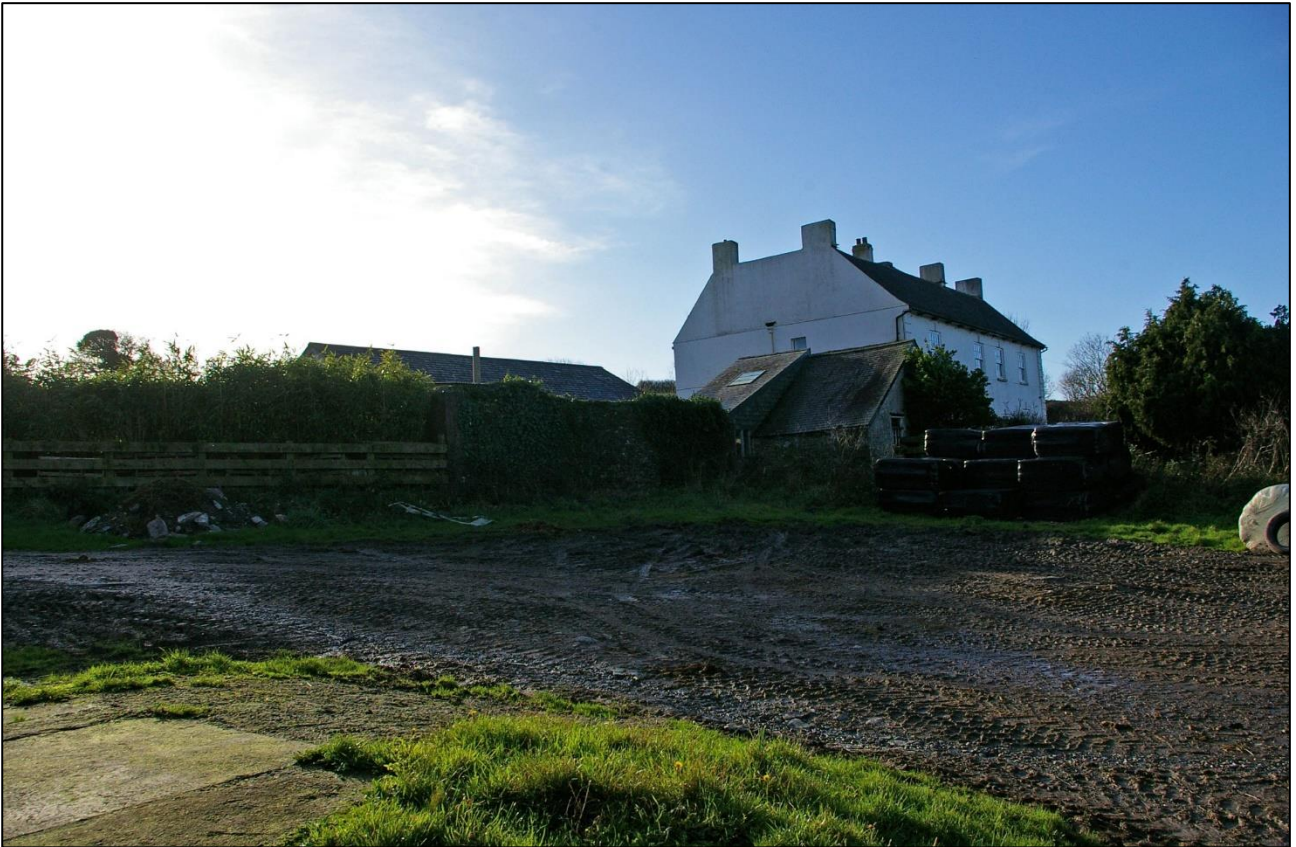
17. RAME BARTON, VIEWED FROM THE ADJACENT FARMYARD, VIEWED FROM THE EAST-NORTH-EAST.
