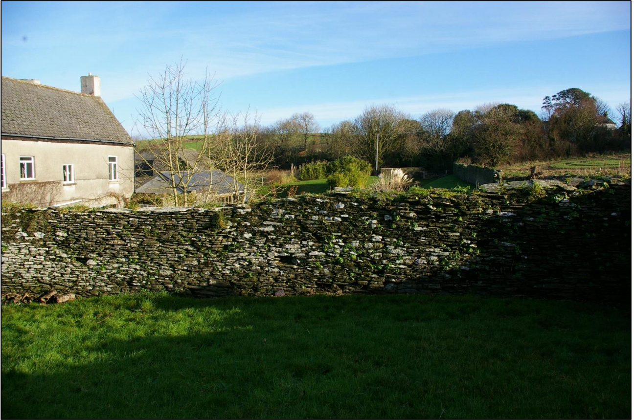
11. STONE WALL, FROM THE WEST.
