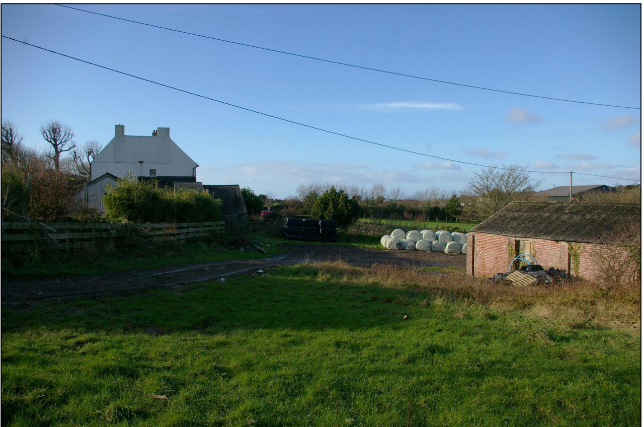
18. RAME BARTON AND ADJACENT FARMYARD, VIEWED FROM THE EAST.
