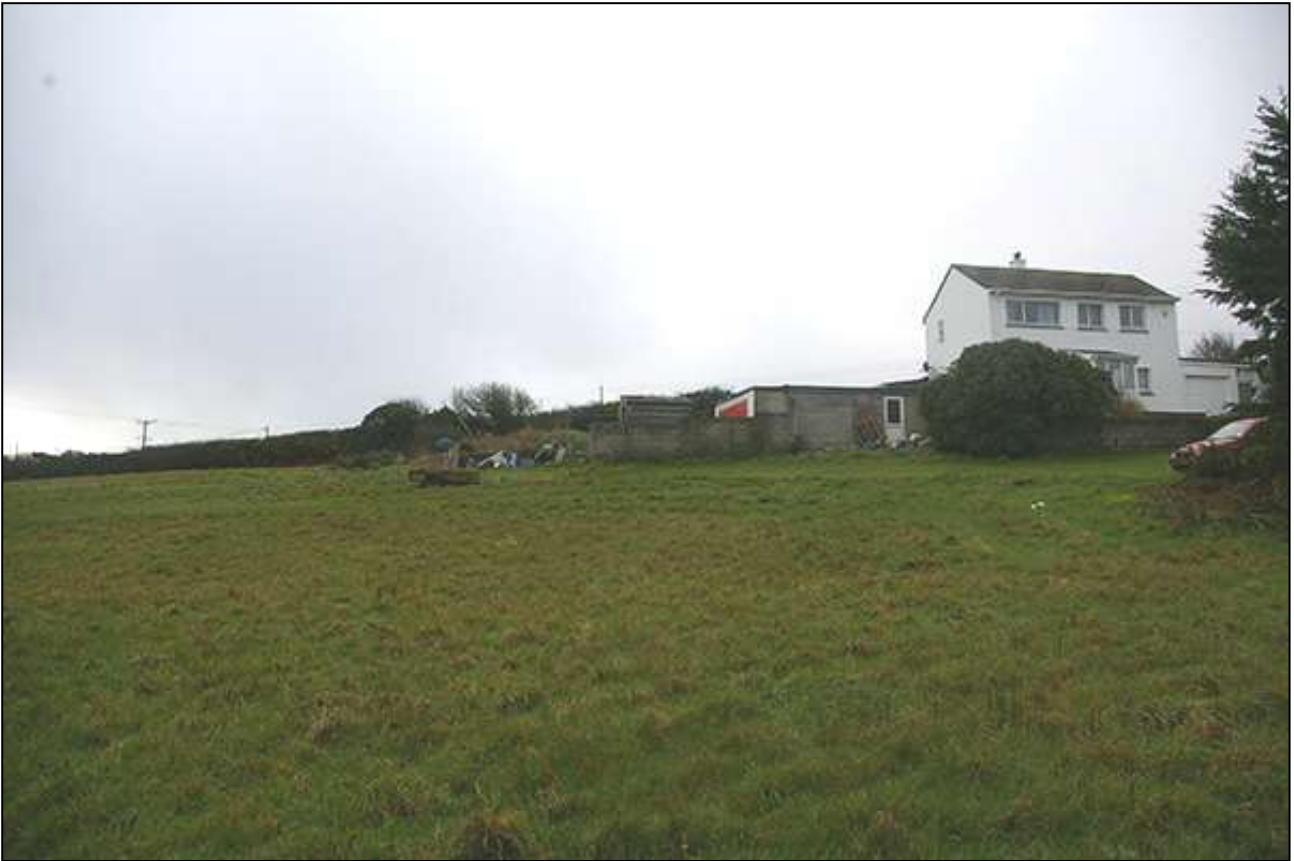
9. VIEW TO THE SOUTH, LOOKING TOWARDS WHITE HORSES HOUSE, WITH GARAGE TO EAST AND TERRACE GARDENS AREAS; VIEWED FROM THE NORTH.
