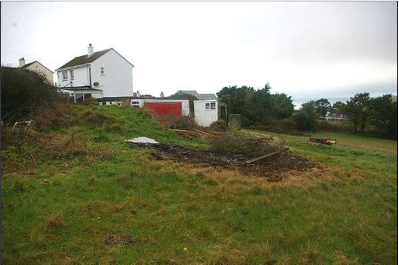
21. VIEW TO WHITE HORSES AND ITS DETACHED GARAGE; VIEWED FROM THE EAST-SOUTH-EAST.
