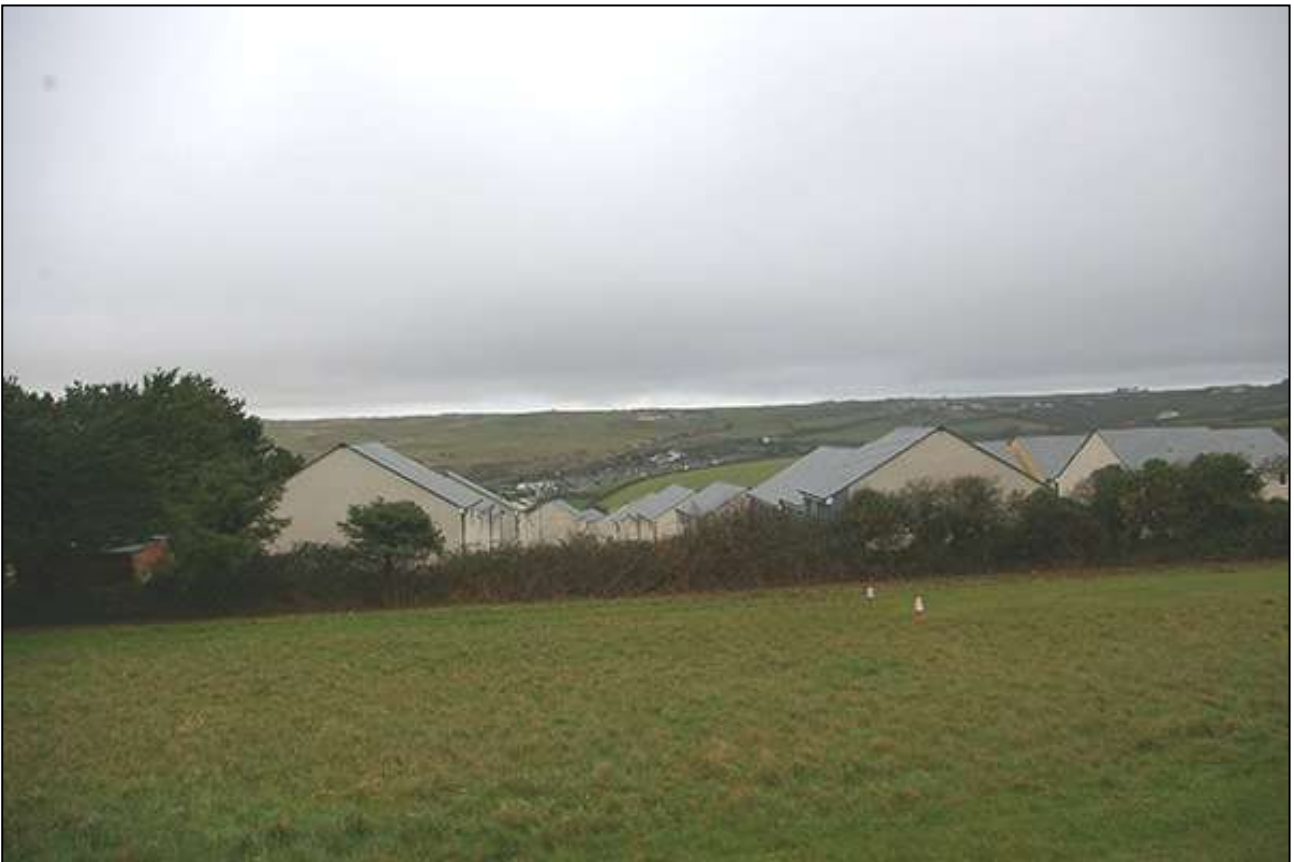
24. VIEW DOWN TO HENDRAWNA MEADOWS; VIEWED FROM THE SOUTH.
