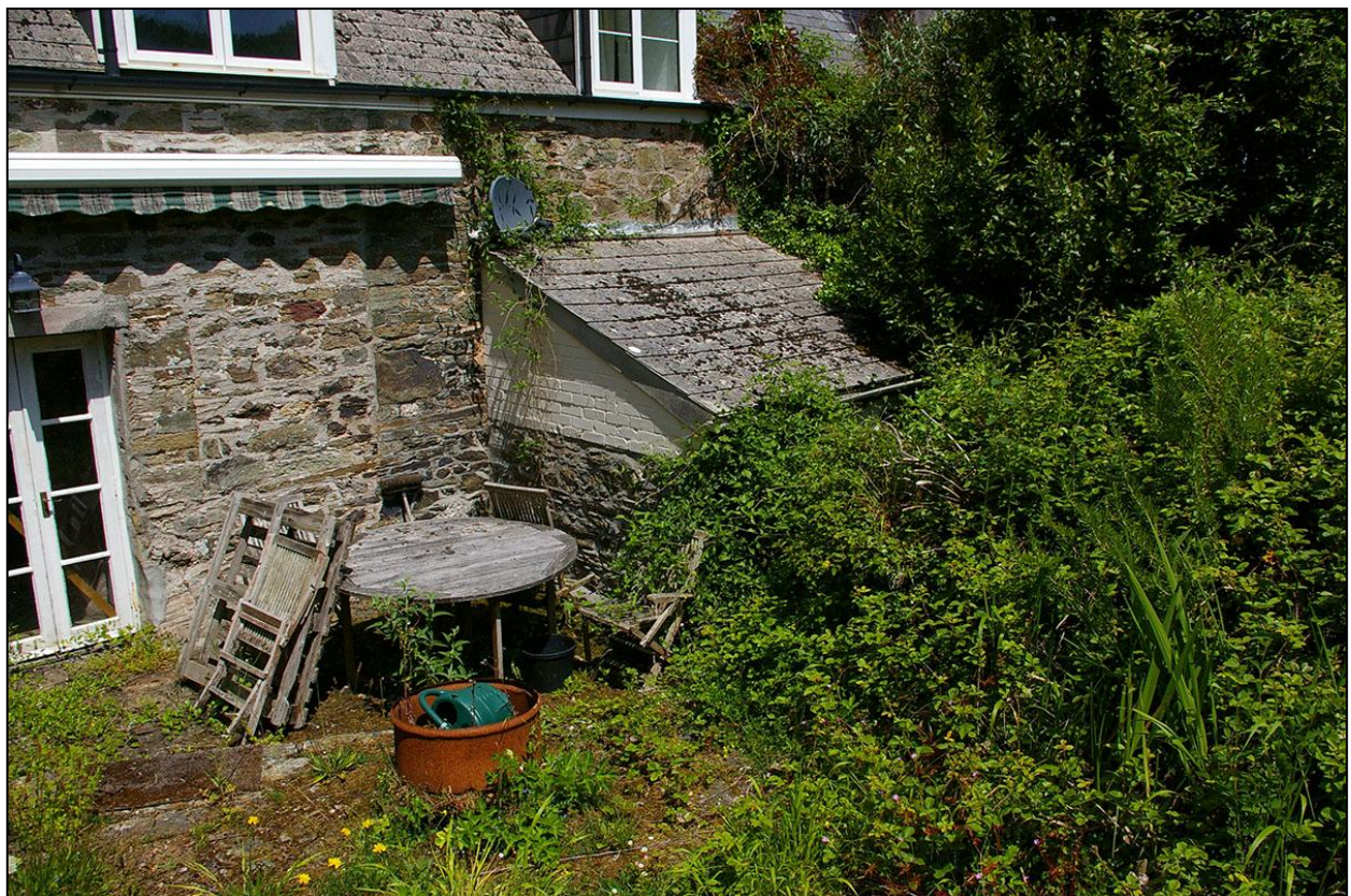
THE PROJECTING BLOCK, OF AN OLDER FORM OF PLATEY STONEWORK, OFF THE BACK OF THE SOUTH ELEVATION ACROSS THE JOIN BETWEEN COTTAGE AND FARMHOUSE; FROM THE SOUTH-WEST.
