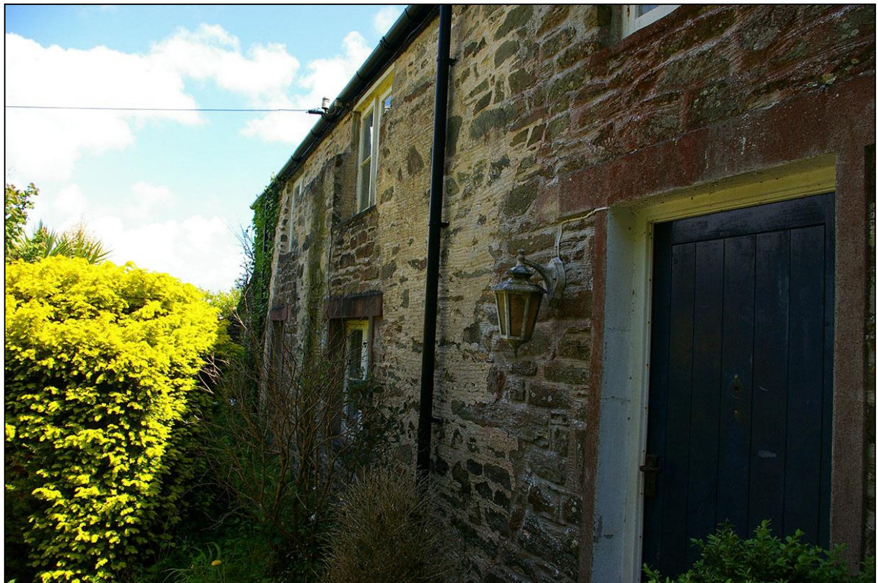
WIDER ANGLED VIEW SHOWING THE INCORPORATED RUINS AND FORCED FRONT DOOR, LEADING INTO THE INTERIOR; FROM THE WEST, NORTH-WEST.
