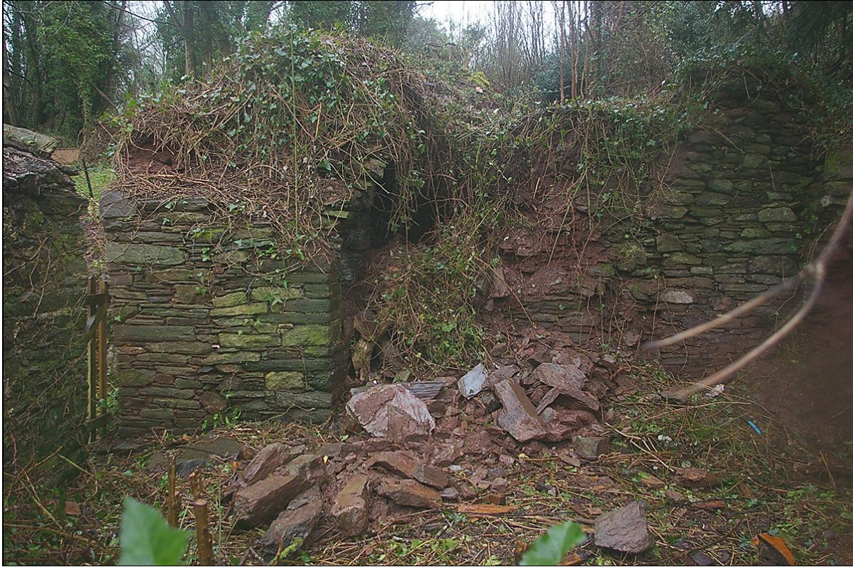
THE WEST WALL OF THE DETACHED MEDIEVAL BLOCK, SHOWING A LARGE OPEN FIREPLACE WITH OVEN TO THE SOUTH-WEST CORNER, FROM THE EAST.
