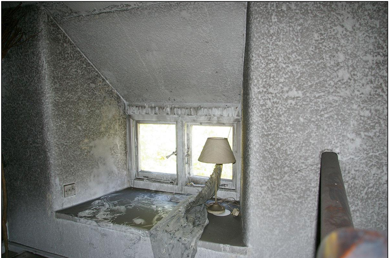
THE TWO LIGHT WINDOW SET INTO A BLOCKED LOADING DOOR IN THE FRONT WALL, CW4; FROM THE SOUTH-EAST.
