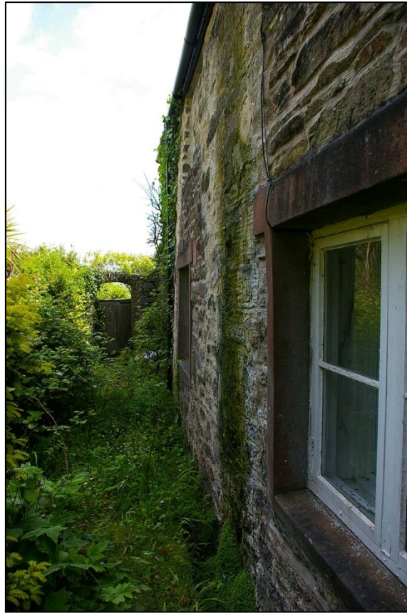
VIEW BACK ALONG THE INCORPORATED RUINED EARLIER BUILDING SHOWING THE SLIGHT BATTER TO THE WALL AND HOW THE WINDOWS AND RAISED EAVES ARE INSET BEHIND THE EARLIER WALLING, FORMING A LEDGE; FROM THE WEST.
