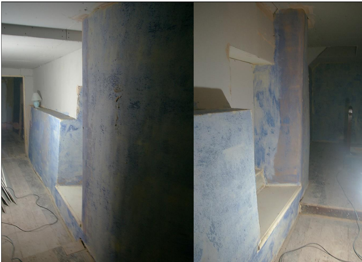
LEFT: THE SOUTH WALL OF THE FARMHOUSE, SHOWING THE BATTERED LOWER EARLIER SECTION OF WALL AND THE TALL ANGLED WEST PROJECTION, WITH DISTINCTIVE CURVE; FROM THE WEST-NORTH-WEST.
