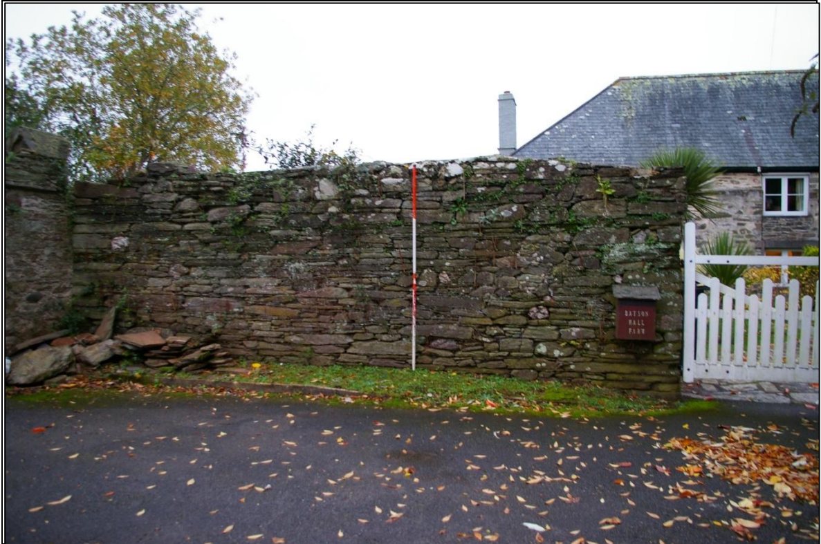
FIGURE 12: THE FRONT GARDEN WALL THE FORMER GABLE END OF A MEDIEVAL BUILDING, 2M SCALE, AUTUMN 2010; FROM THE NORTH-NORTH-WEST.
