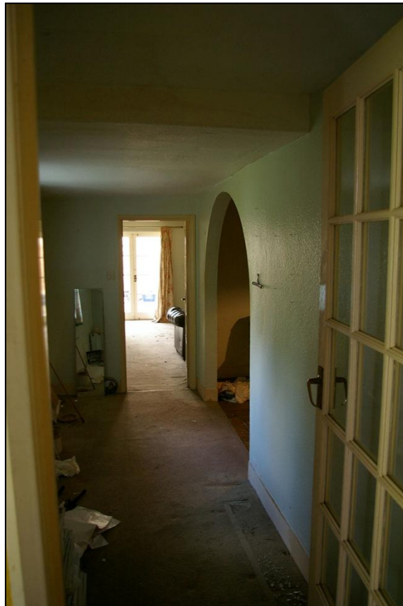
VIEW FROM THE HALLWAY INTO THE LOBBY/CORRIDOR CREATED BY ANOTHER MODERN PARTITION AND ARCHWAY, FORMING A FITTED KITCHEN, ALSO SHOWING FURTHER MODERN GLAZED DOORS AND MODERN FITTINGS; FROM THE WEST.
