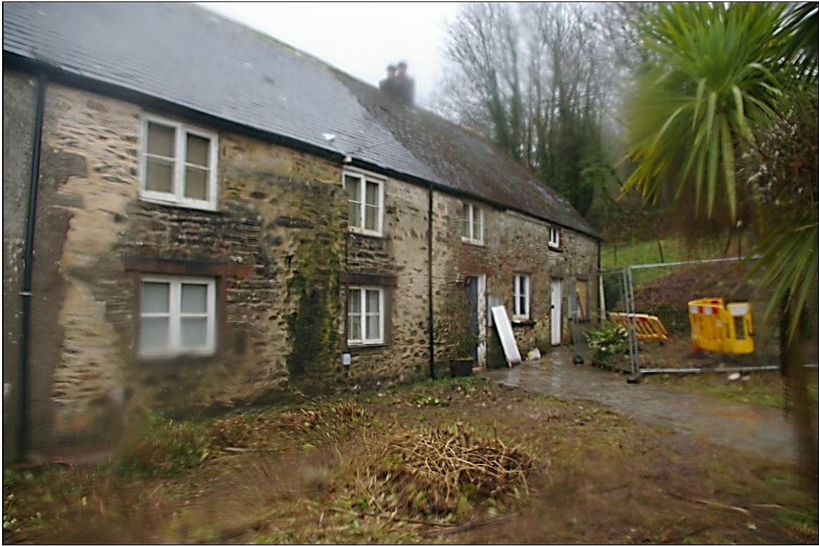
FIGURE 13: THE FRONT ELEVATION OF THE FARMHOUSE, CLEARED OF ALL VEGETATION, FEBRUARY 2020; FROM THE NORTH-EAST.
