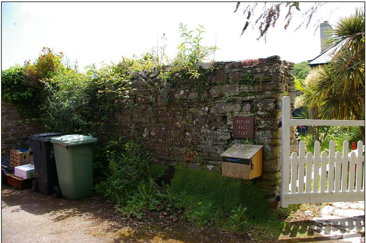
THE NORTH OUTER FACE OF THE HEAVY SLATESTONE WALL, WHICH IS THE FORMER GABLE END OF AN EARLY BUILDING; FROM THE NORTH-WEST.
