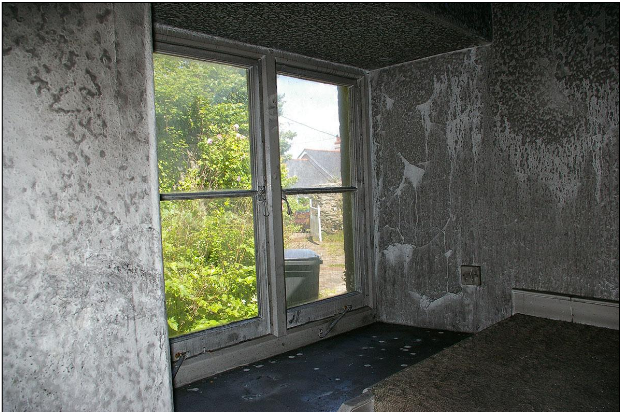
DEEP BEADED OPENING, PLANK SILL AND TWO LIGHT BEADED CASEMENT IN CHAMFERED PEGGED FRAME, A 19 TH CENTURY FEATURE CW1; FROM THE SOUTH-WEST.
