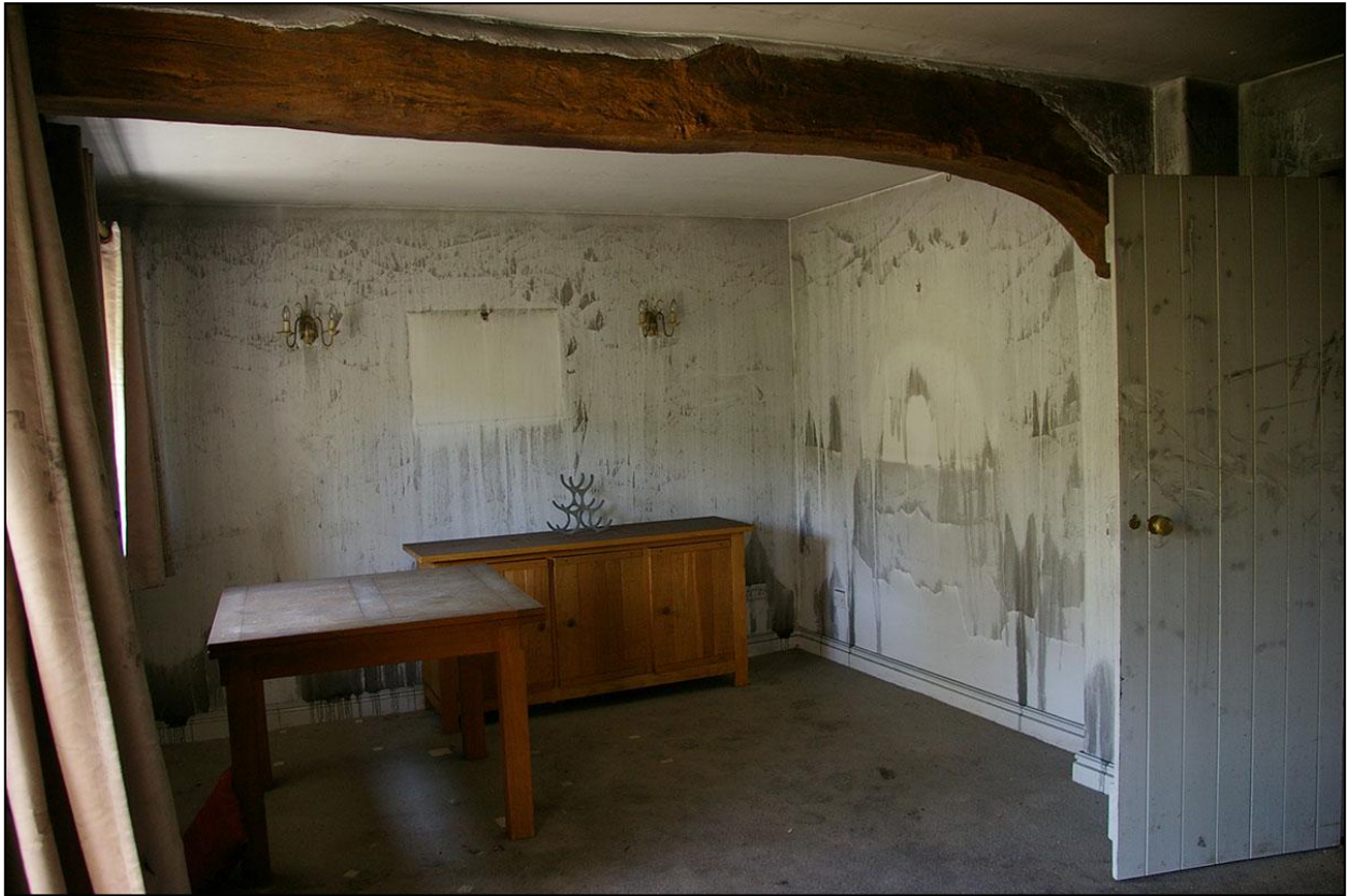
THE BEAM IN MORE DETAIL, BRACING A FORMER PARTITION LINE/WALL LINE; FROM THE SOUTH-EAST.
