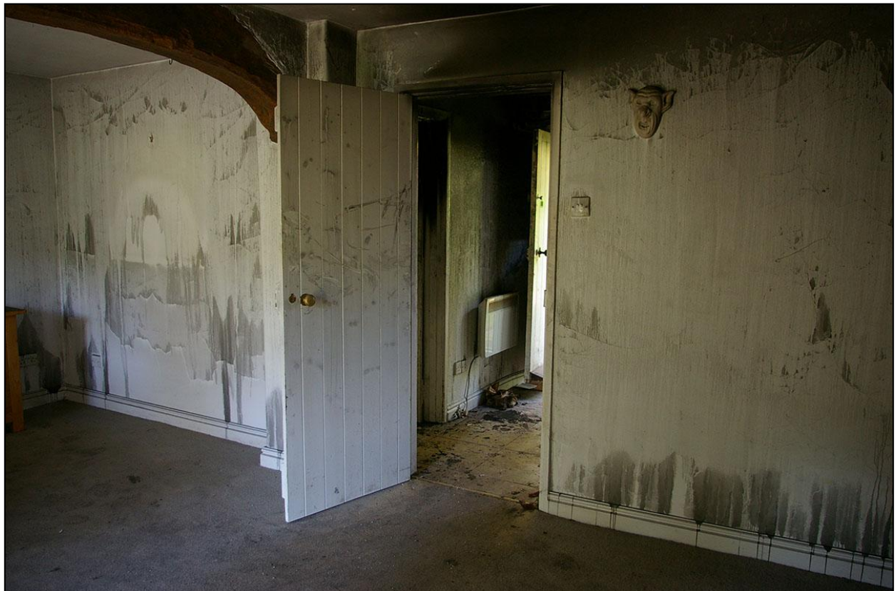
THE MODERN PARTITIONS, WITH A STUD OF EARLIER WALL BRACED BY A HACKED BACK BEAM IN CR3, THE SITTING ROOM, ALSO WITH DOOR BACK TO THE HALLWAY; FROM THE SOUTH-EAST.
