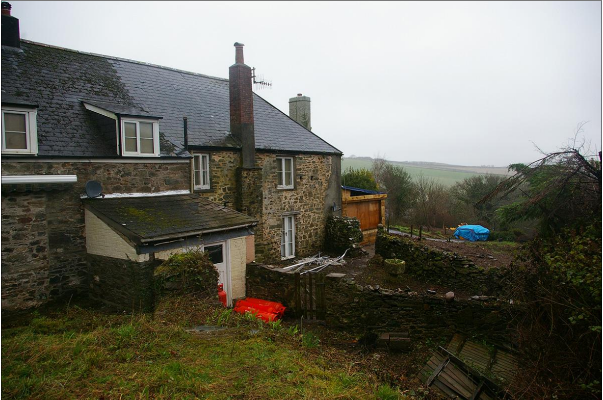
THE SOUTH ELEVATION OF THE FARMHOUSE, SHOWING THE PROJECTION TO THE WEST AND SMALL LATERAL STACK BUILT AGAINST THE EARLIER STONEMASONRY OF THE MEDIEVAL RUIN, WHICH OCCUPIES A SECTION TO THE CENTRE OF THE WALL, FROM THE SOUTH-WEST.
