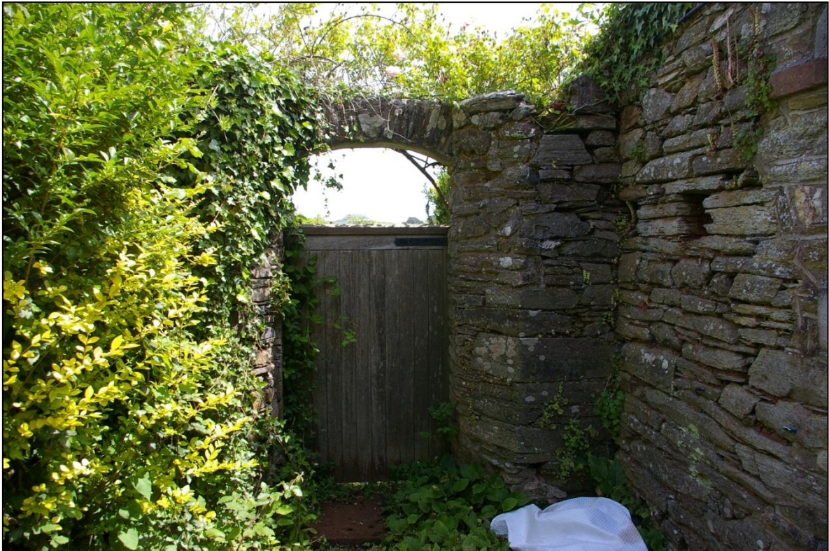
FIGURE 10: DETAILED VIEW OF THE FINE HEAVY SLATESTONE AND PUTLOGS, AND SLOPING EMBRASURES, WHICH IDENTIFY THESE GARDEN WALLS AS RUINS OF A 'FINE' MEDIEVAL BUILDING, JUNE 2019; FROM THE WEST-NORTH-WEST.
