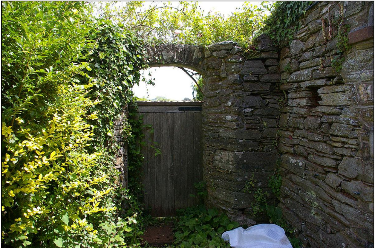
DETAILED VIEW OF THE FINE HEAVY SLATESTONE AND SOME DRESSED BLOCKS AND PUTLOGS, ALL OF WHICH IDENTIFY THESE GARDEN WALLS, AS IN FACT RUINS OF AN EARLIER QUITE FINE BUILDING, LIKELY PART OF THE COMPLEX WHICH SUPPORTED THE MANOR HOUSE WHICH STOOD ON THE SITE; FROM THE WEST.
