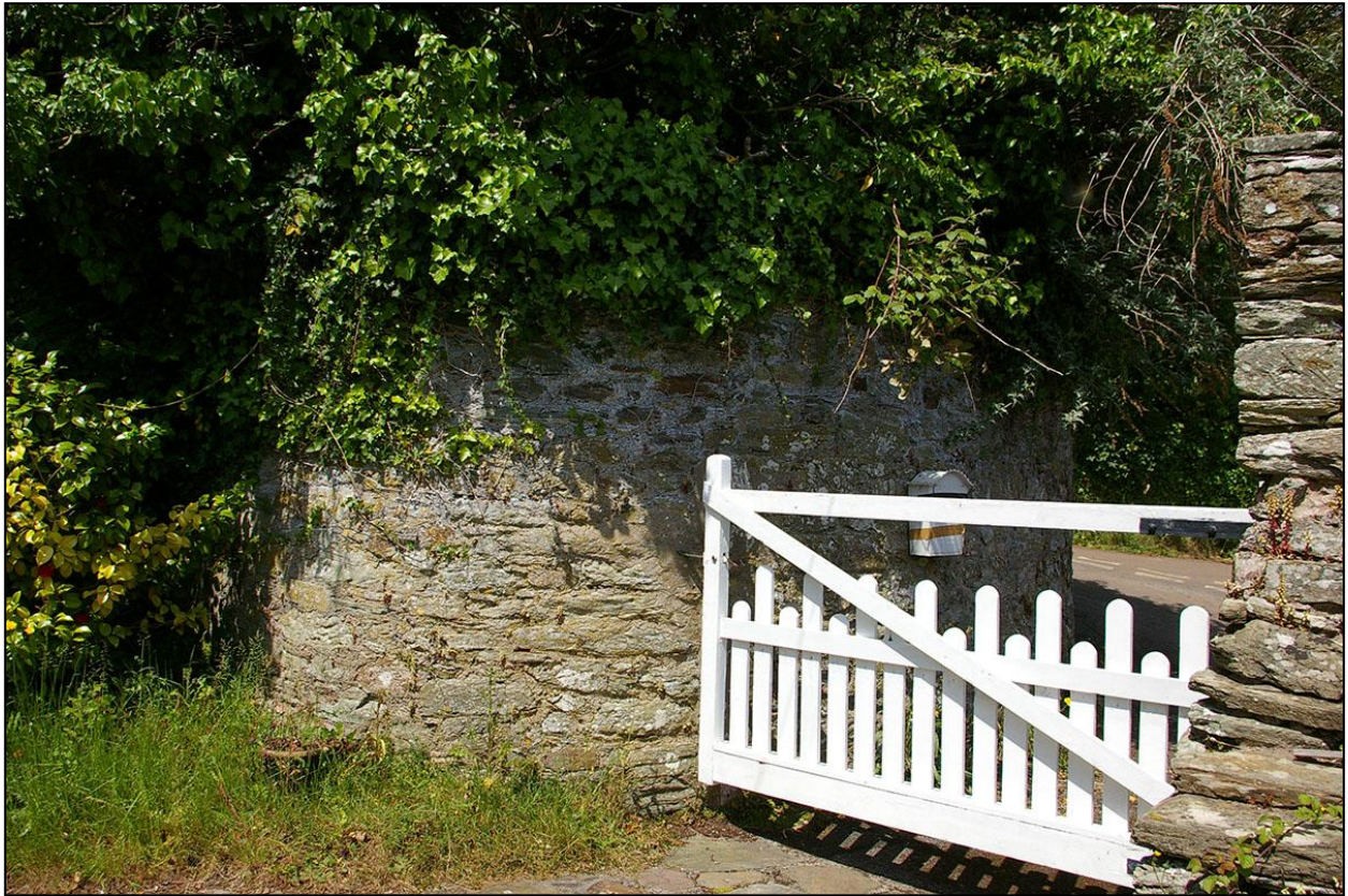
THE LOOSE RUBBLE 19 TH CENTURY GARDEN WALL IN A LIME MORTAR, ENCLOSING AN EMBANKED AREA AND FLANKING THE HEDGEBANK ALONGSIDE THE ROAD; FROM THE EAST.
