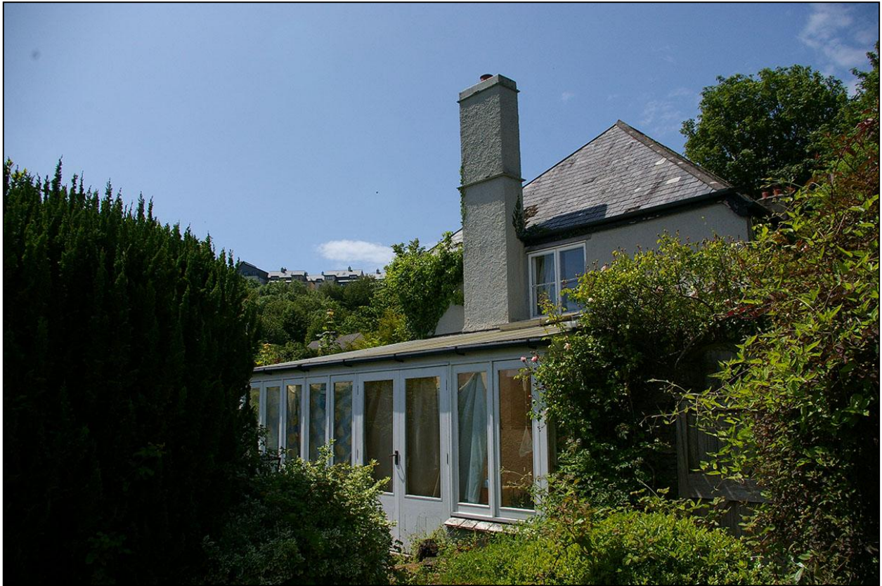
THE EAST GABLE END OF THE FARMHOUSE, WITH HIPPED ROOF, BOX STACK AND SHAFT AND LARGE MODERN CONSERVATORY; FROM THE NORTH-EAST.
