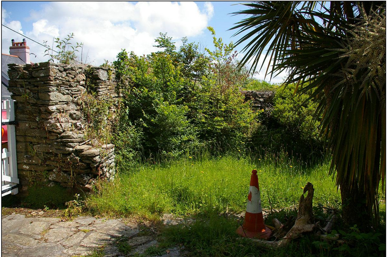
DETAIL OF THE NORTH GABLE END WALL OF THE EARLIER BUILDING, WHICH NOW FORMS THE GARDEN WALL, SHOWING A STUB RUNNING BACK TOWARDS THE HOUSE; FROM THE WEST, SOUTH-WEST.
