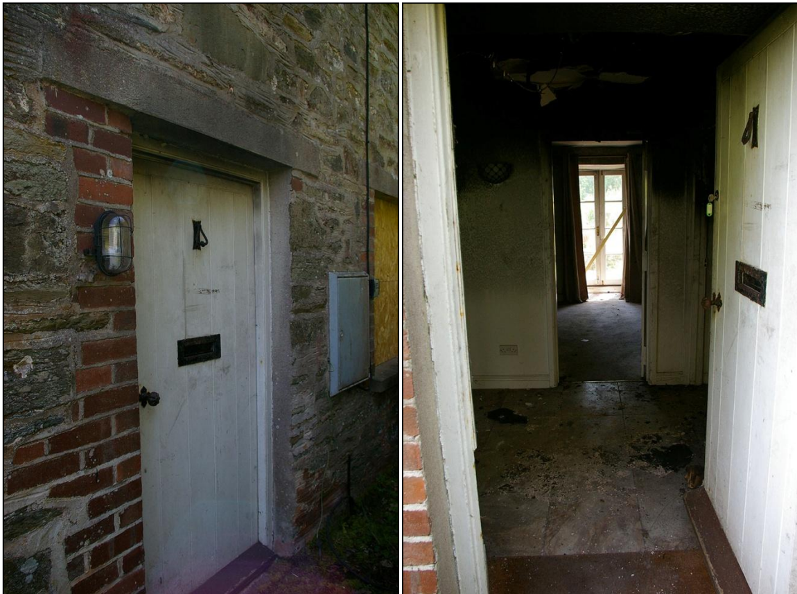
LEFT: THE FRONT DOOR TO THE COTTAGE, BRICK PATCHED REVEALS TO THE EAST, CONCRETE RENDER PATCHING TO THE WEST AND RENDERED LINTEL; FROM THE NORTH-EAST.
