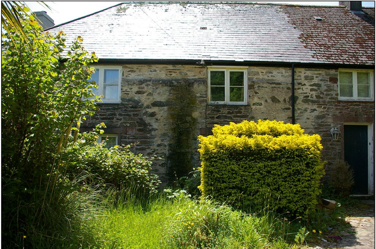
DETAILED VIEW OF THE THICKER LOWER SECTION OF WALLING WHICH DOMINATES THE NORTH FRONT OF THE FARMHOUSE, AT THE EAST END, THE REMAINS OF A RUINED EARLIER BUILDING; FROM THE NORTH.
