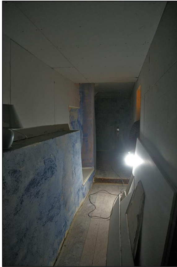
FIGURE 20: VIEW ALONG THE SOUTH CORRIDOR, SHOWING THE MEDIEVAL WALL REMAINS IN THE FOREGROUND, THE TALLER HEAVY BLOCK OF ANGLED MASONRY, WITH CURVING INNER PROFILE IN THE BACKGROUND TO THE PROJECTING BAY; FROM THE EAST.
