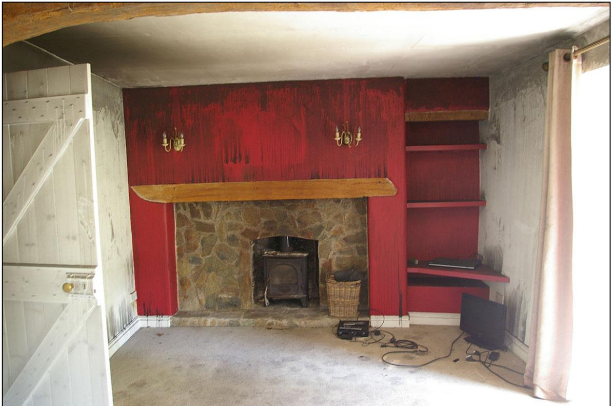
THE SHALLOW STACK AND BLOCKED FIREPLACE, WITH ALCOVE TO THE SOUTH, WITH TIMBER LINTEL; FROM THE WEST.
