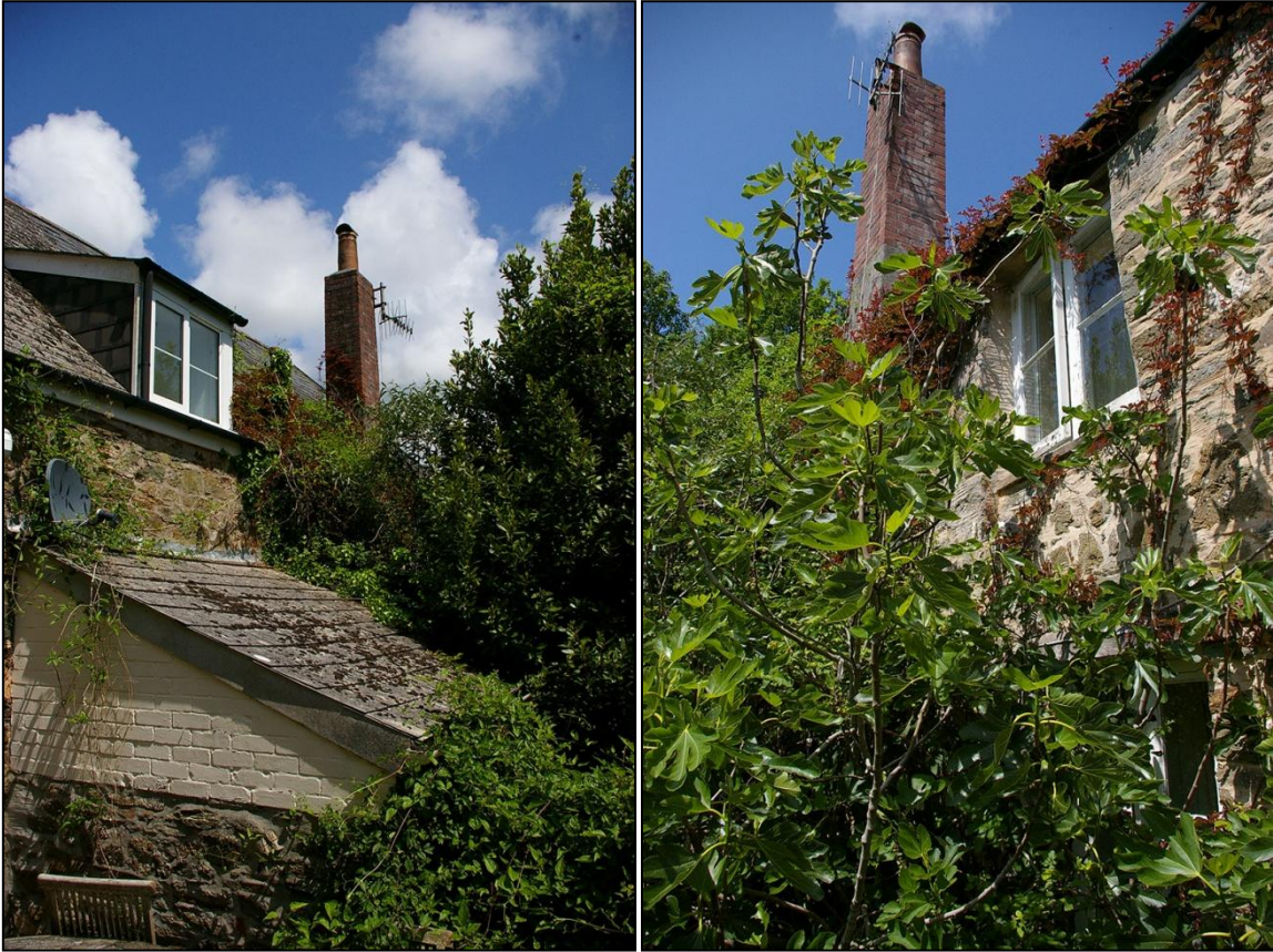
LEFT: VIEW BACK ALONG THE REAR OF THE FARMHOUSE, SHOWING LOOSE POST MEDIEVAL RUBBLE AT THE EAVES AND A REBUILT BRICK CHIMNEY SHAFT, AS WELL AS A DISTINCT CHANGE IN ALIGNMENT ON THE ROOF; FROM THE WEST, SOUTH-WEST.
