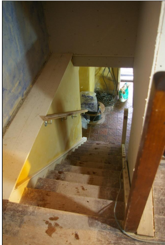
VIEW DOWN THE STAIRS IN THE FARMHOUSE, BUILT AGAINST THE THICK SLIGHTLY BATTERED FORMER GABLE WALL, SHOWING IT IS FAR THICKER TO THE GROUND FLOOR, WITH A MARKED LEDGE, WHERE THE MEDIEVAL WALL STOPS, HAVING BEEN RUINED AT SOME STAGE, FROM THE SOUTH.
