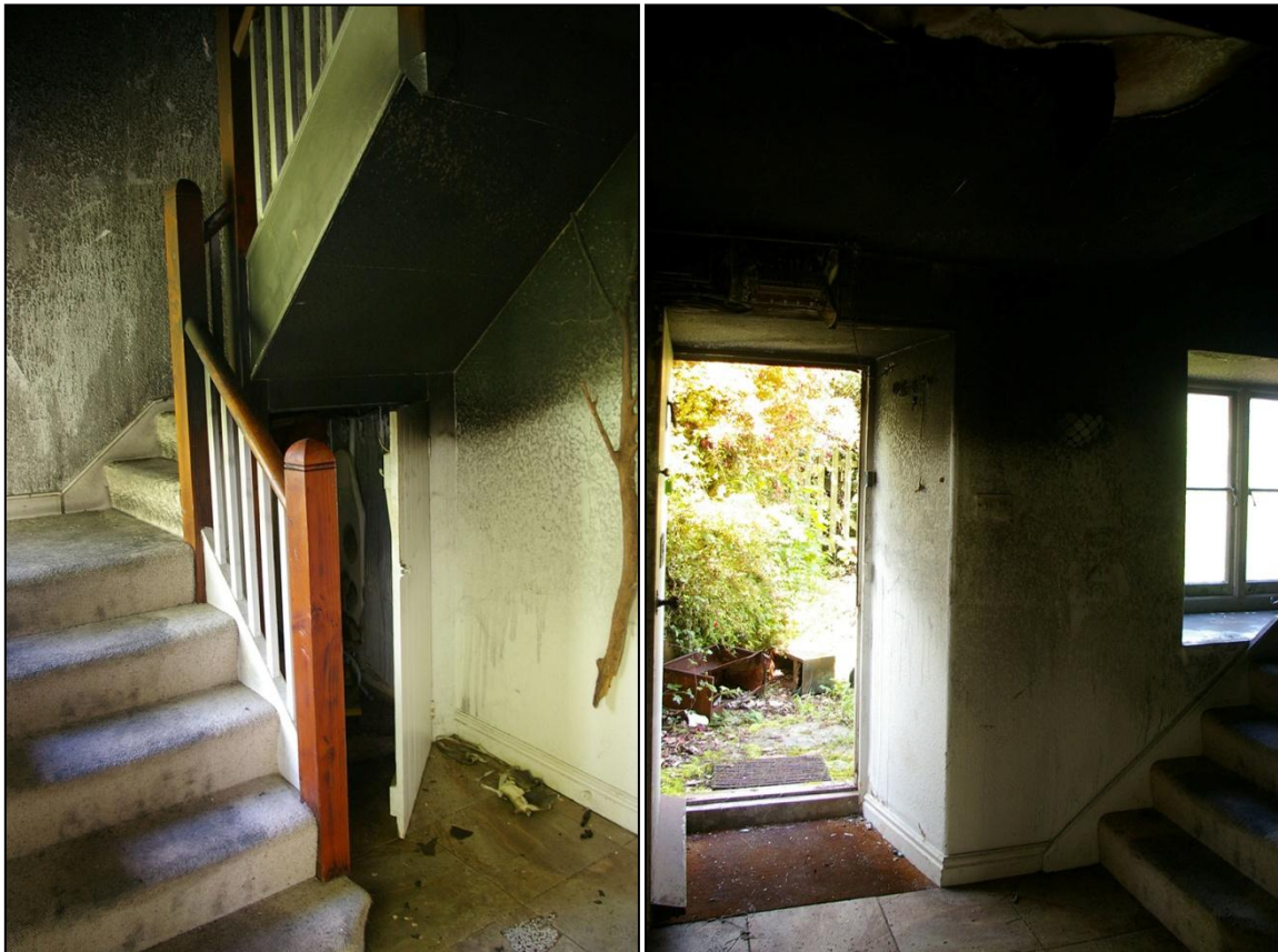
LEFT: VIEW OF THE LATE 20 TH CENTURY TIMBER STAIRCASE, HEAVILY SMOKE BLACKENED; FROM THE NORTH-WEST.
