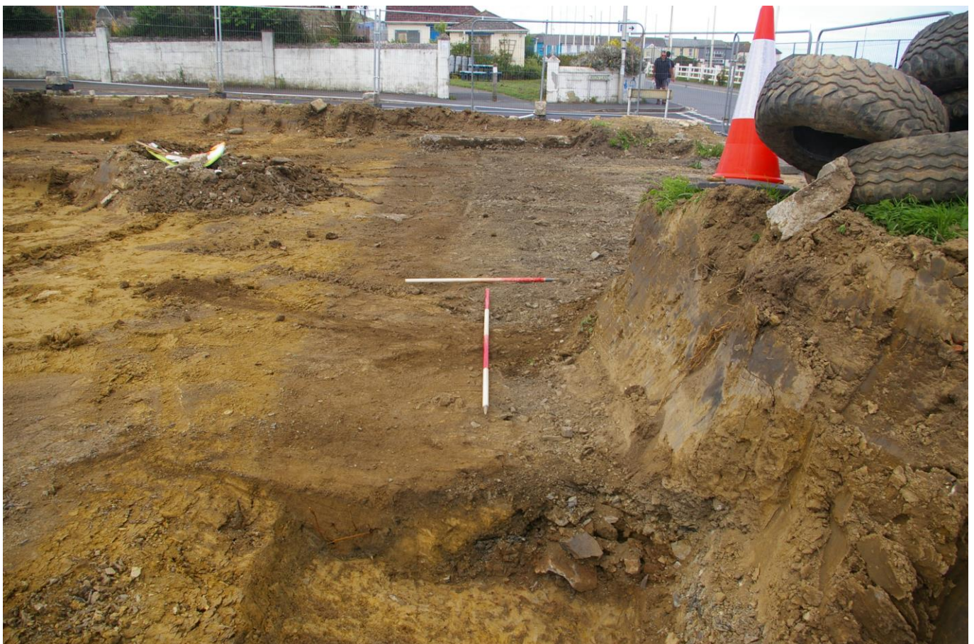
FIGURE 3: THE LINE OF THE FORMER BIDEFORD, WESTWARD HO! AND APPELORE RAILWAY AS REPRESENTED BY TRACK BED {121} AND ASSOCIATED DRAINAGE DITCH [122]; VIEWED FROM THE EAST (1M & 2M SCALES).
