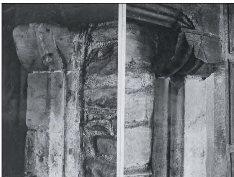
Figure 28: The corbels of the first floor front fireplace.
