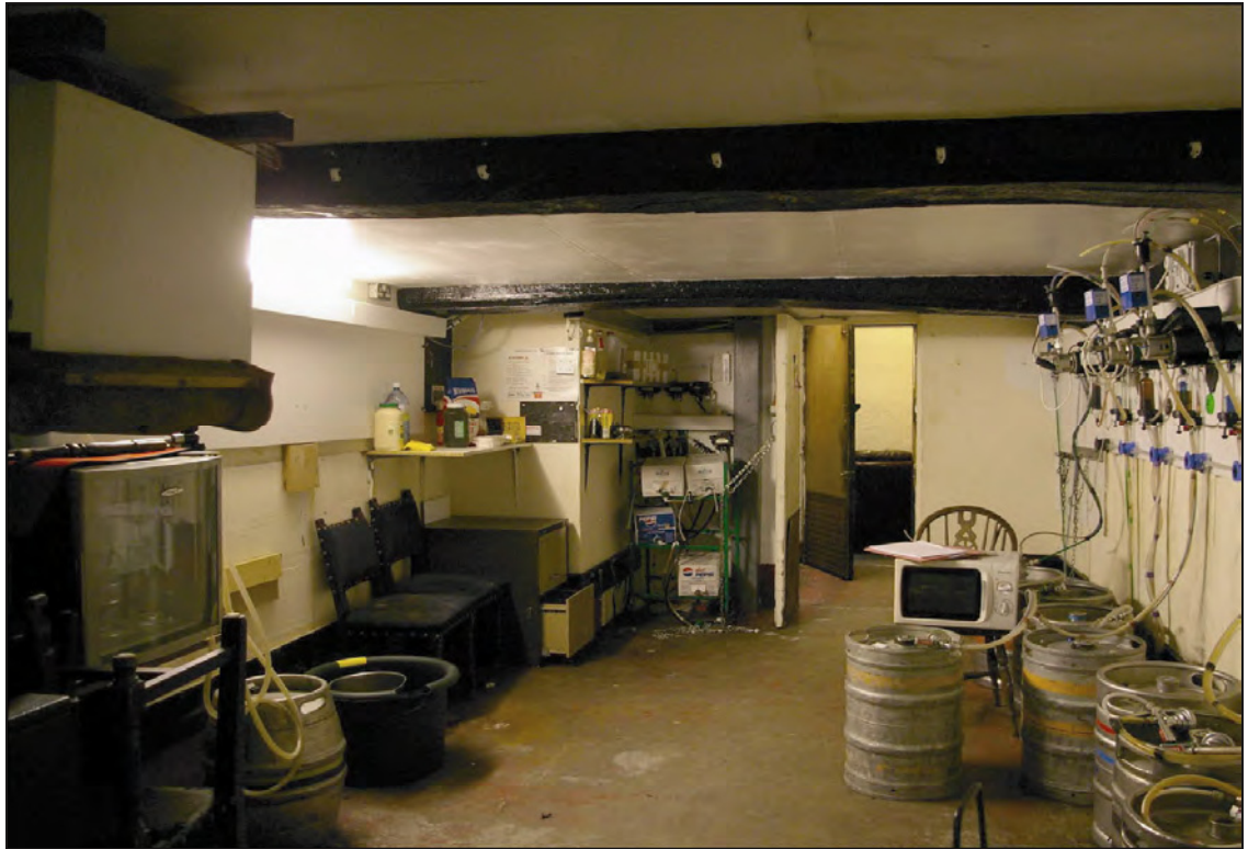
Figure 18: The back block (Room 7), viewed from the west.
