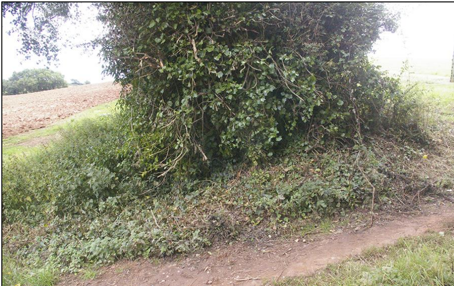
2. SOUTH BOUNDARY AT SITE ENTRANCE; VIEWED FROM THE WEST (NO SCALE).
