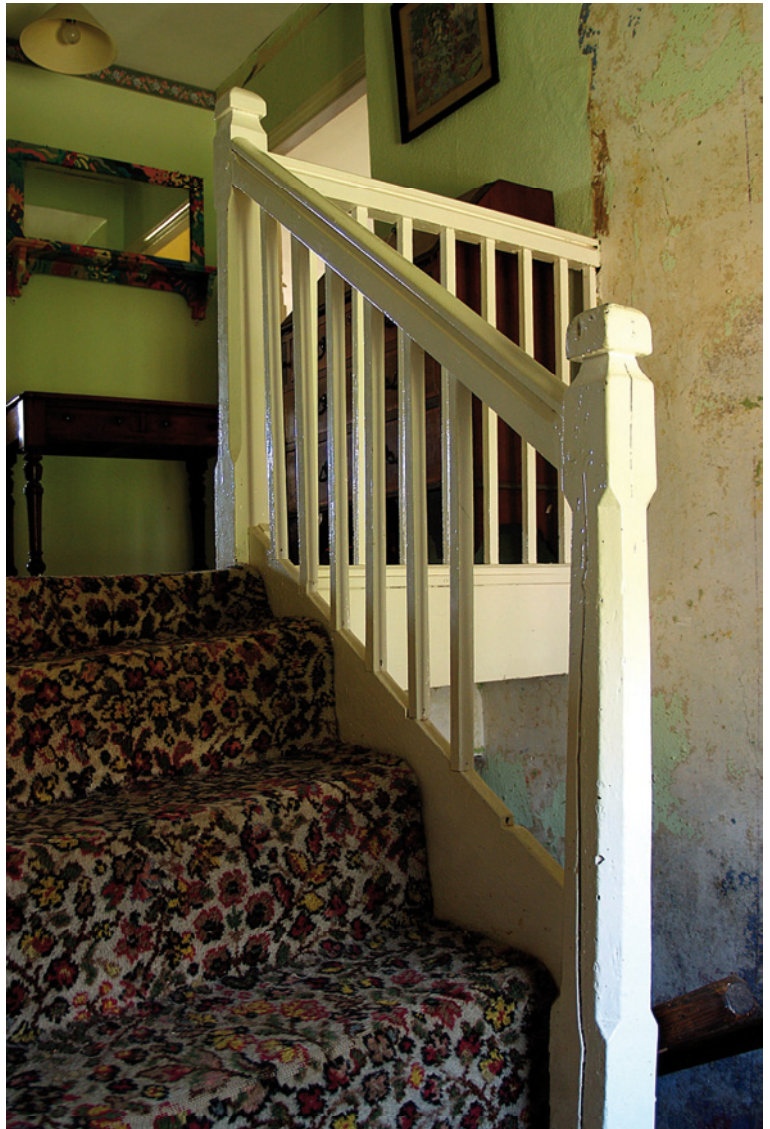
[15] The main stair was refurbished c1880, but the lower newel post may survive from the 18th century.
