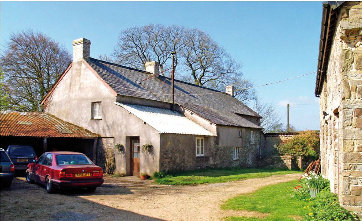
[10] The back of the house from the northeast. The nearest and lowest of the rear lean-tos is the potato store and, beyond is the dairy and then the stairblock under the same roof.
