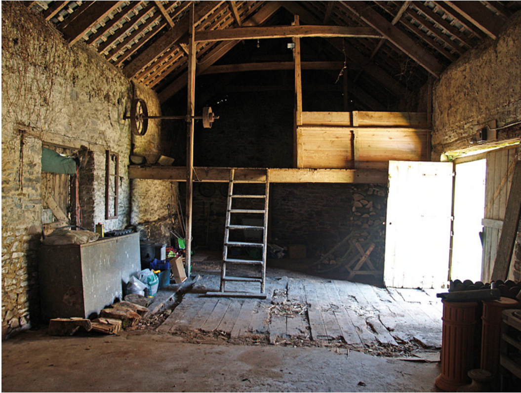
[21] The inside of the barn, looking south towards the lofted end, and showing the threshing floor in front. The driveshaft with belt drives and gearing comes through the the right-hand (east) side just beyond the threshing floor.
