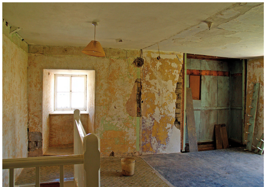
[16] The first floor chamber at the east end of the first floor level, looking east. A scar along the ceiling shows that there was once an axial partition dividing the space into two.
