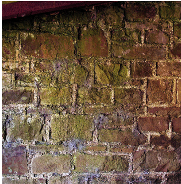
[17] Detail of the original pointing on the south end of the front, preserved within the cartshed.
