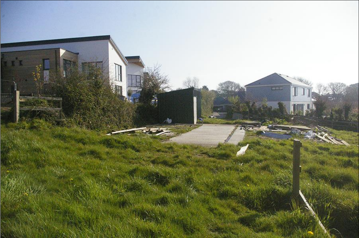
7. VIEW ALONG THE NORTH BOUNDARY OF THE NORTH FIELD SHOWING THE EXISTING CONCRETE PAD AND ACCESS THROUGH THE NORTH-EAST CORNER; VIEWED FROM THE WEST (NO SCALE).
