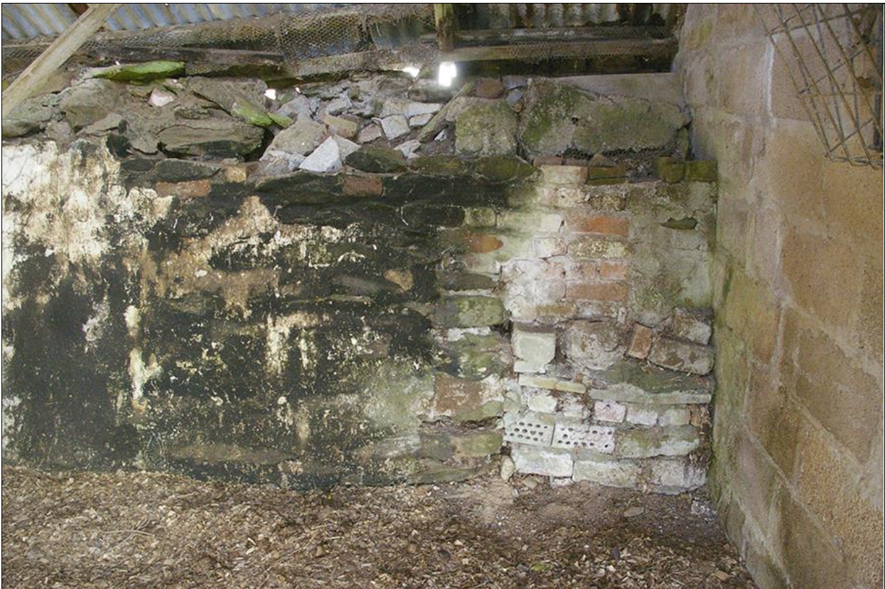
14. DETAIL OF THE EAST END OF THE WEST ROOM OF THE STRUCTURE IN THE NORTH-WEST CORNER OF THE SOUTH FIELD, SHOWING PATCHED REPAIRS; VIEWED FROM THE SOUTH (NO SCALE).
