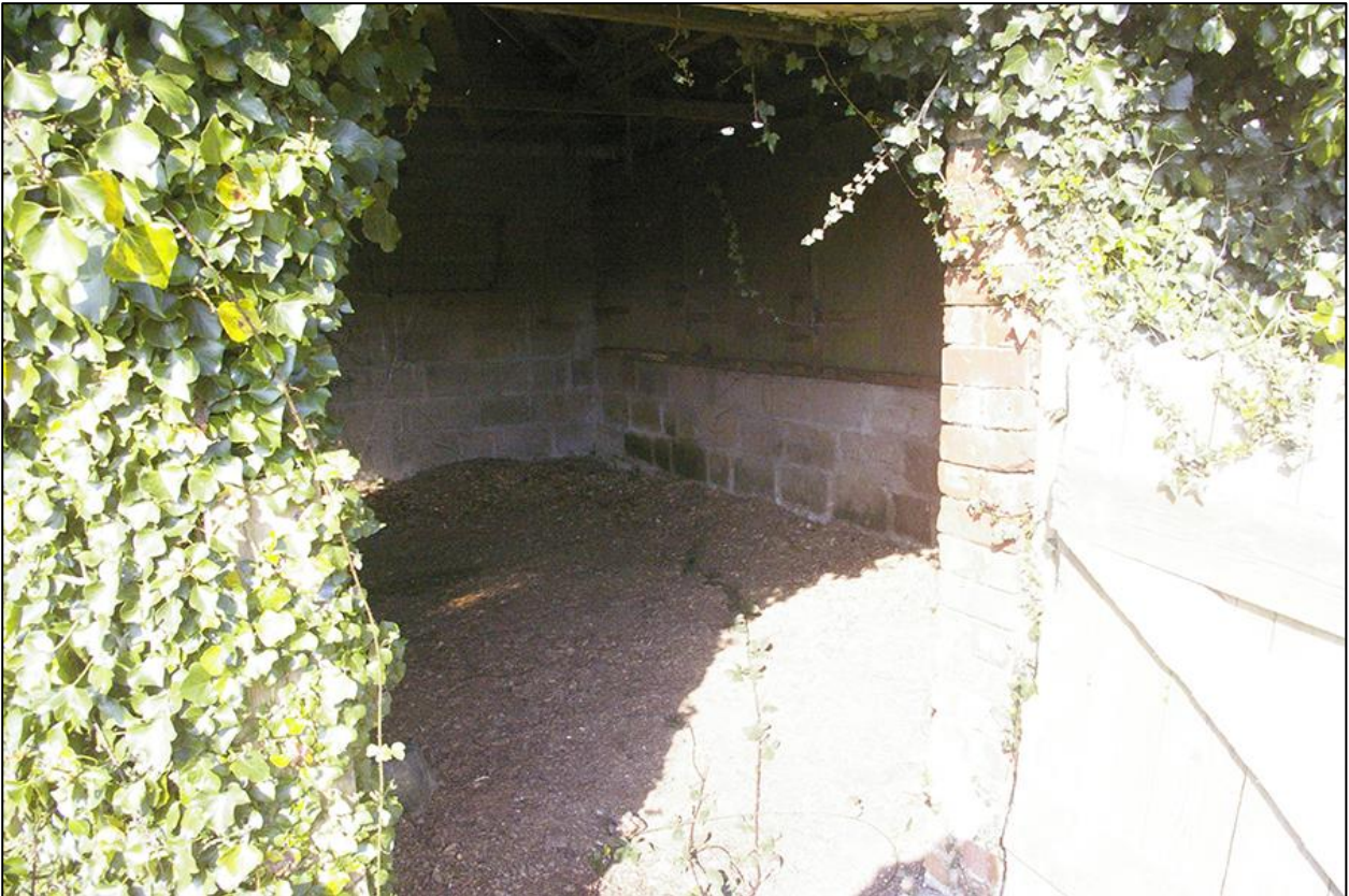
13. DETAIL OF THE EAST ROOM OF THE STRUCTURE IN THE NORTH-WEST CORNER OF THE SOUTH FIELD, SHOWING THE BLOCK AND BRICK WORK CONSTRUCTION; VIEWED FROM THE SOUTH-EAST (NO SCALE).
