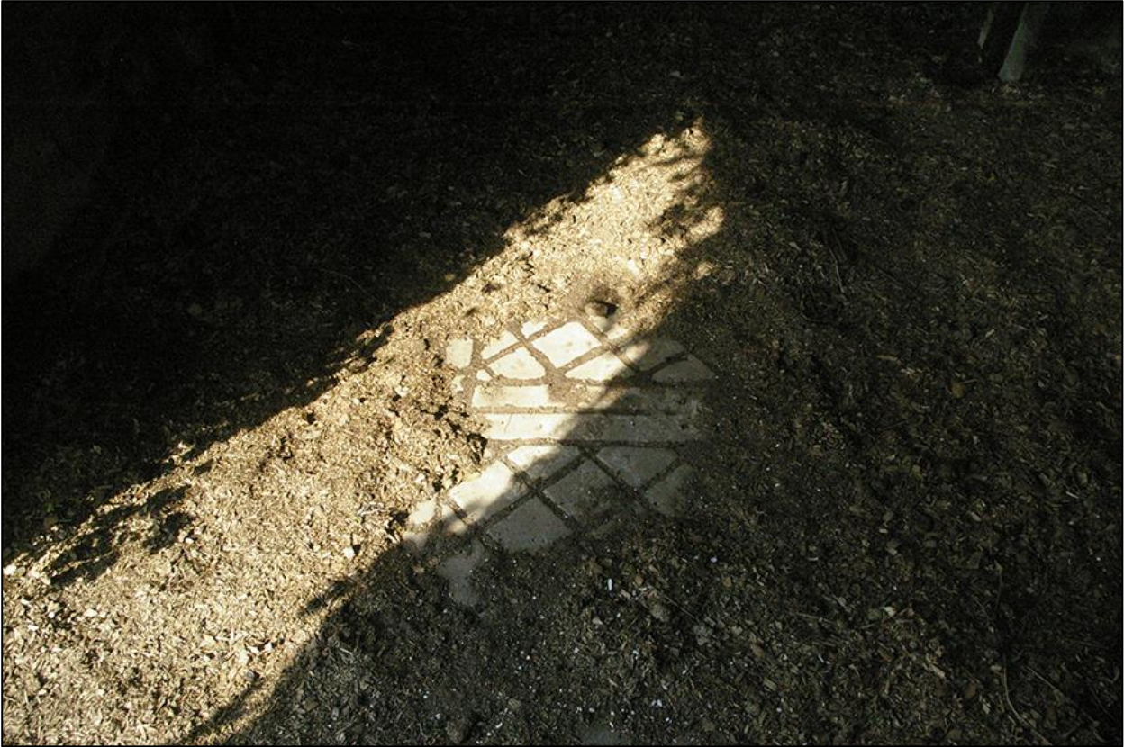
15. DETAIL OF PAVERS IN THE FLOOR OF THE STRUCTURE; VIEWED FROM THE EAST (NO SCALE).
