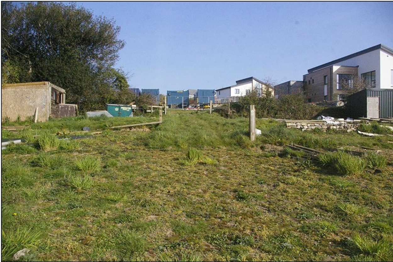
6. DETAIL OF THE NORTHERN END OF THE NORTH FIELD SHOWING THE ADJOINING BUILDING SITE; VIEWED FROM THE SOUTH (NO SCALE).
