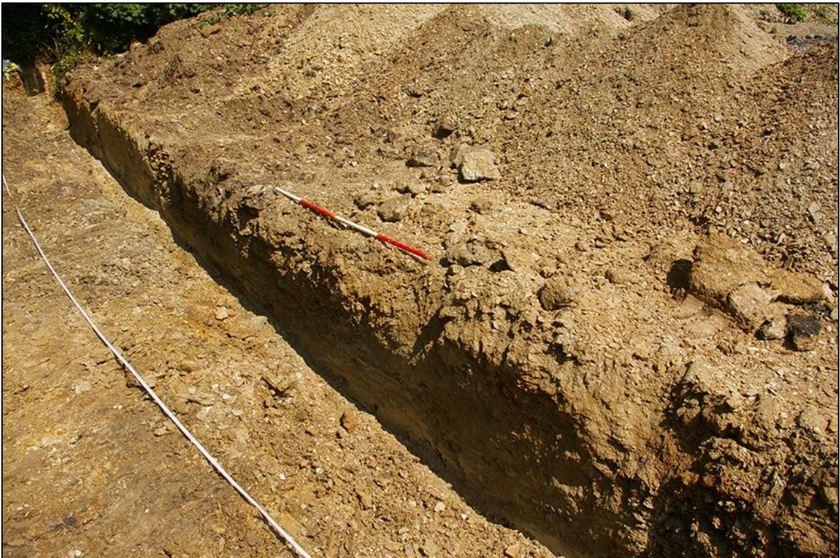
59. TRENCH 02, POST-EXCAVATION; VIEWED FROM THE SOUTH-WEST (2M SCALE).
