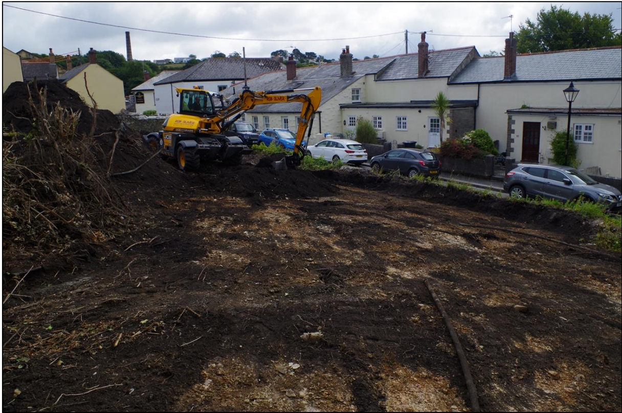
80. AREA 03, POST-EXCAVATION; VIEWED FROM THE NORTH-WEST (NO SCALE).
