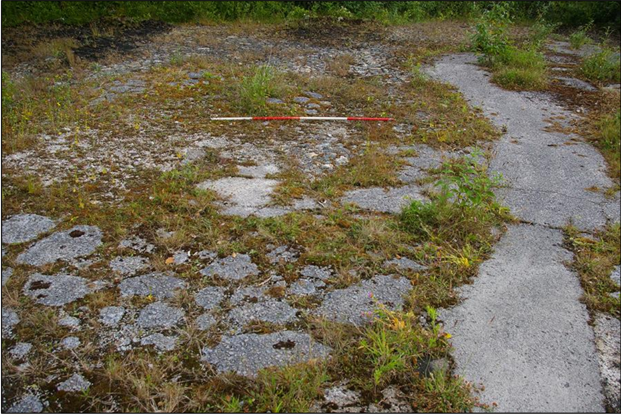
19. DETAIL OF COBBLE SURFACE (103) WITH CONCRETE REPAIRS (100), MIDDLE TO SOUTH-EAST CORNER; VIEWED FROM THE SOUTH (2M SCALE).
