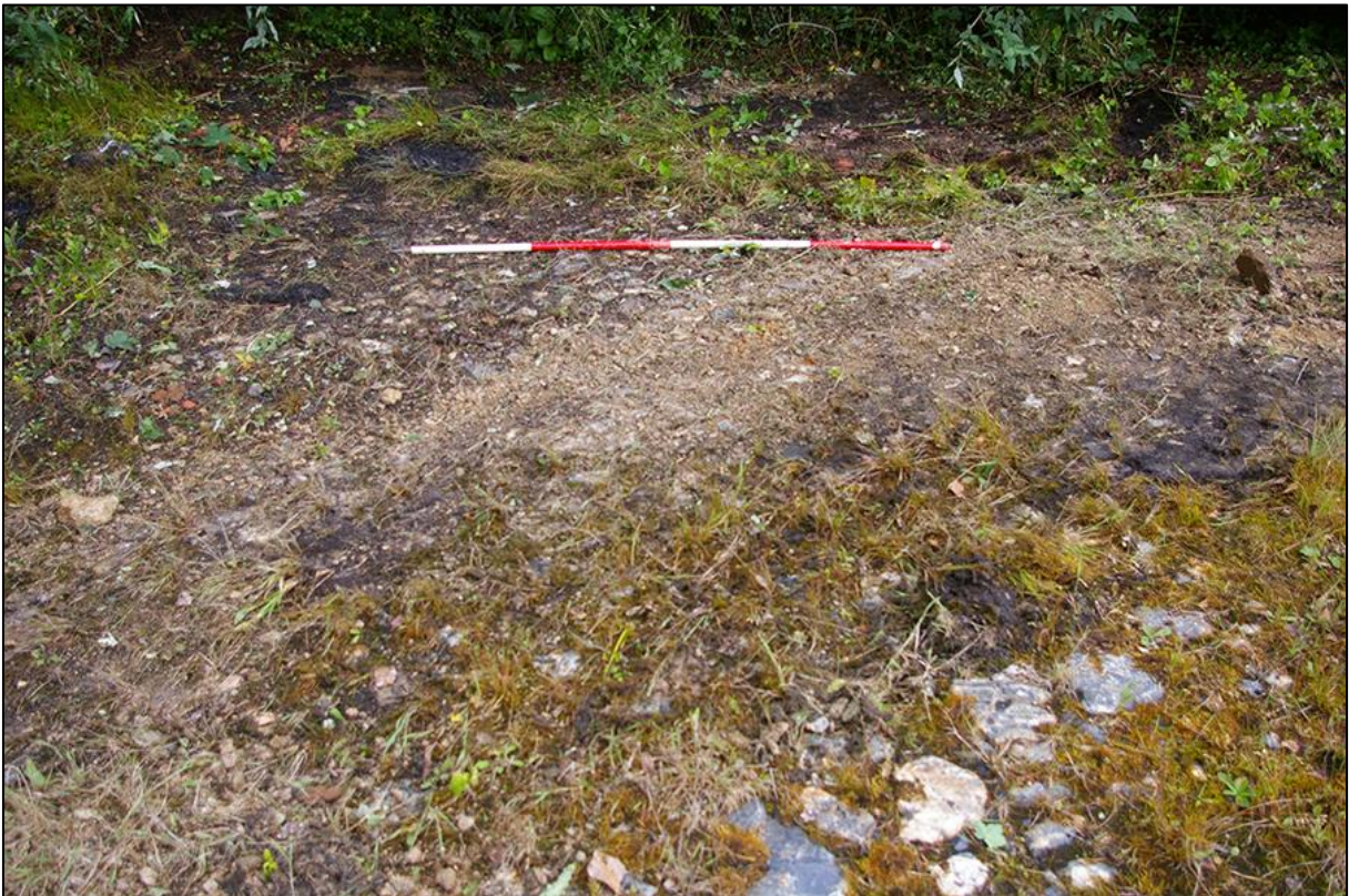
14. DETAIL OF COBBLE SURFACE (103), NORTH-WEST CORNER; VIEWED FROM THE SOUTH (2M SCALE).
