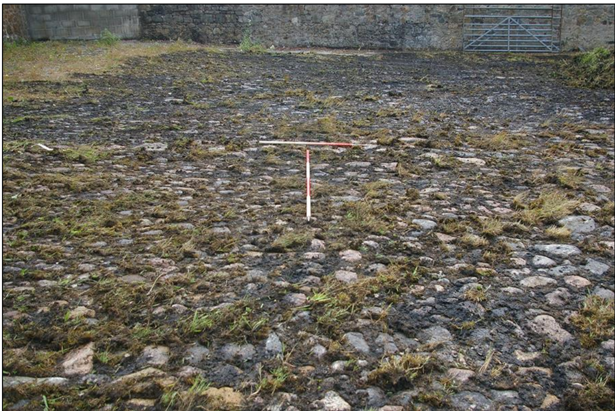
28. DETAIL OF COBBLE SURFACE OF THE SURVIVING ORE FLOOR IN THE NORTH-EAST CORNER OF THE SITE; VIEWED FROM THE WEST (1M & 2M SCALES).
