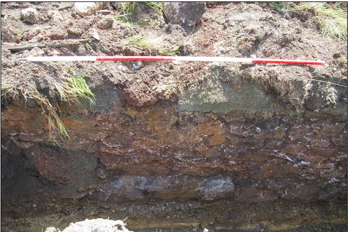
65. DETAIL OF WALL {148}/{149} WITH POSSIBLE FOUNDATION STONES {150}, NORTH FACING ELEVATION; VIEWED FROM THE NORTH (2M SCALE).
