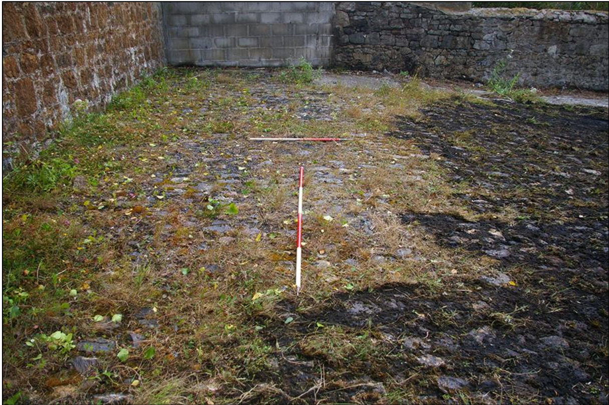
25. DETAIL OF COBBLE SURFACE OF THE SURVIVING ORE FLOOR IN THE NORTH-EAST CORNER OF THE SITE; VIEWED FROM THE WEST (1M & 2M SCALES).
