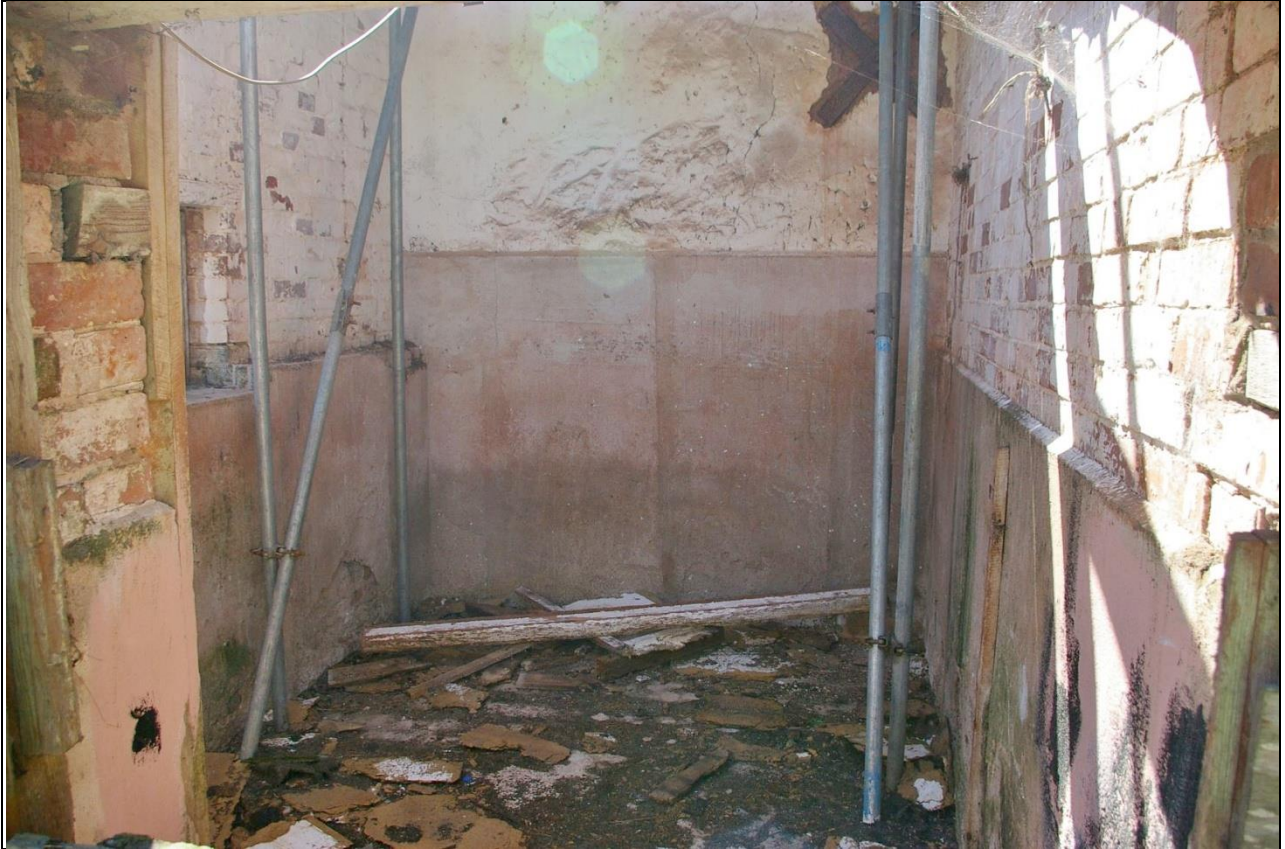
21. THE INSIDE OF B1.3; FROM THE NORTH.
