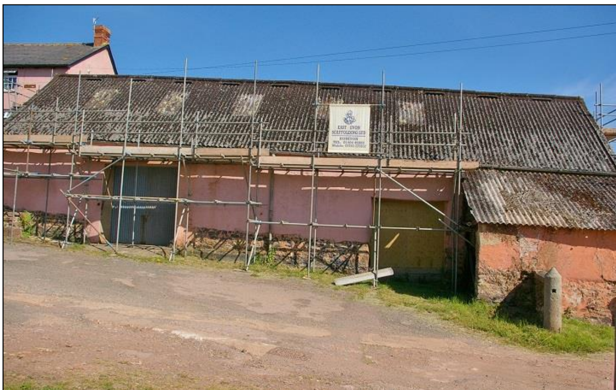
FIGURE 7: THE SOUTH ELEVATION OF LOWER RIXDALE BARN; FROM THE SOUTH.
