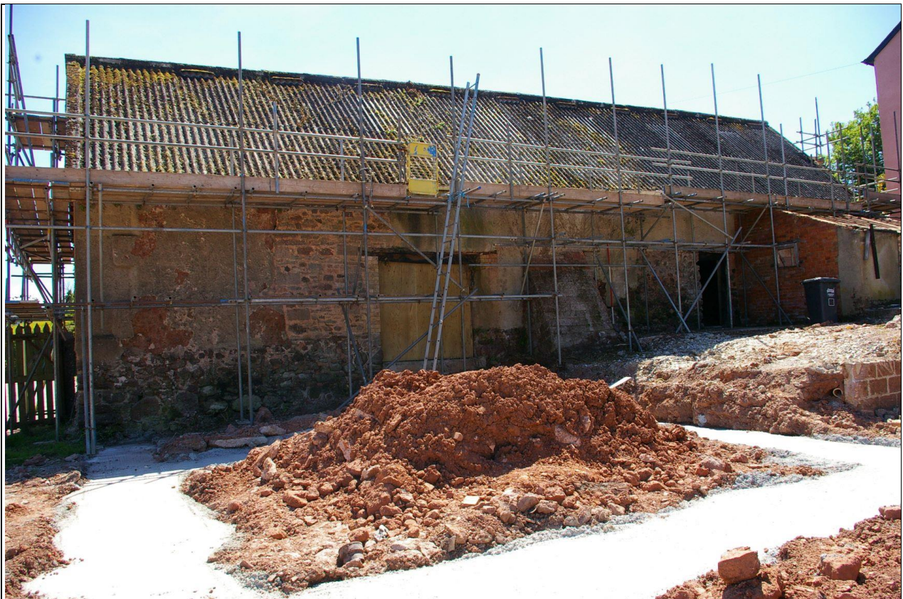
13. LOWER RIXDALE BARN, WITH 2M SCALE; FROM THE NORTH-EAST.
