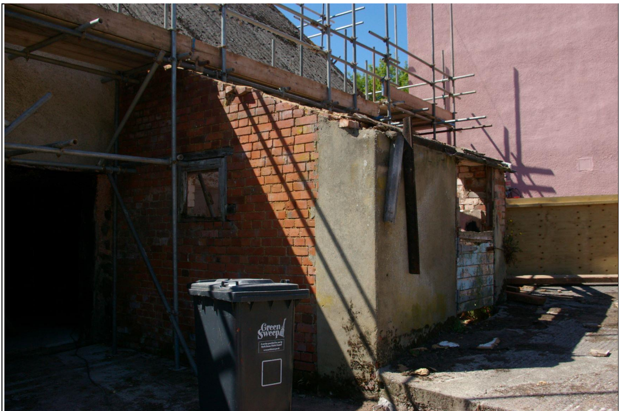
18. THE EAST WALL OF B1.3, THE BRICK OUTSHUT; FROM THE NORTH-EAST.
