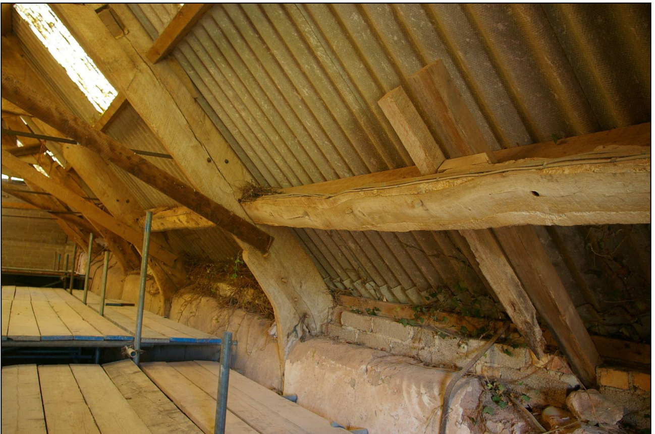
29. DETAIL OF THREADED BUTT PURLINS, FOR TRUSSES 3 AND 4, PEGGED TOGETHER IN THE SOCKET, FOR BAYS 4 AND 5; FROM THE SOUTH-EAST.
