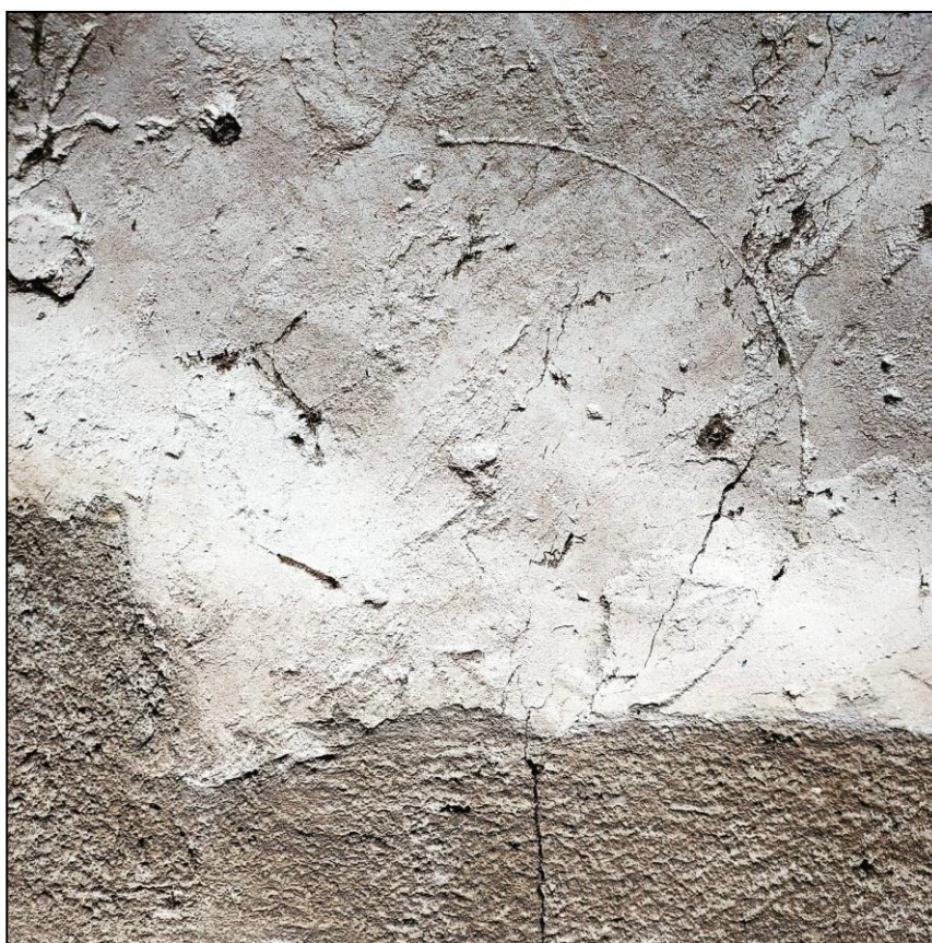
FIGURE 13: THE POTENTIAL DAISY-WHEEL ON THE NORTH WALL OF THE BARN, AT THE WEST END, WEST OF THE WINNOWING DOOR; FROM THE SOUTH.
