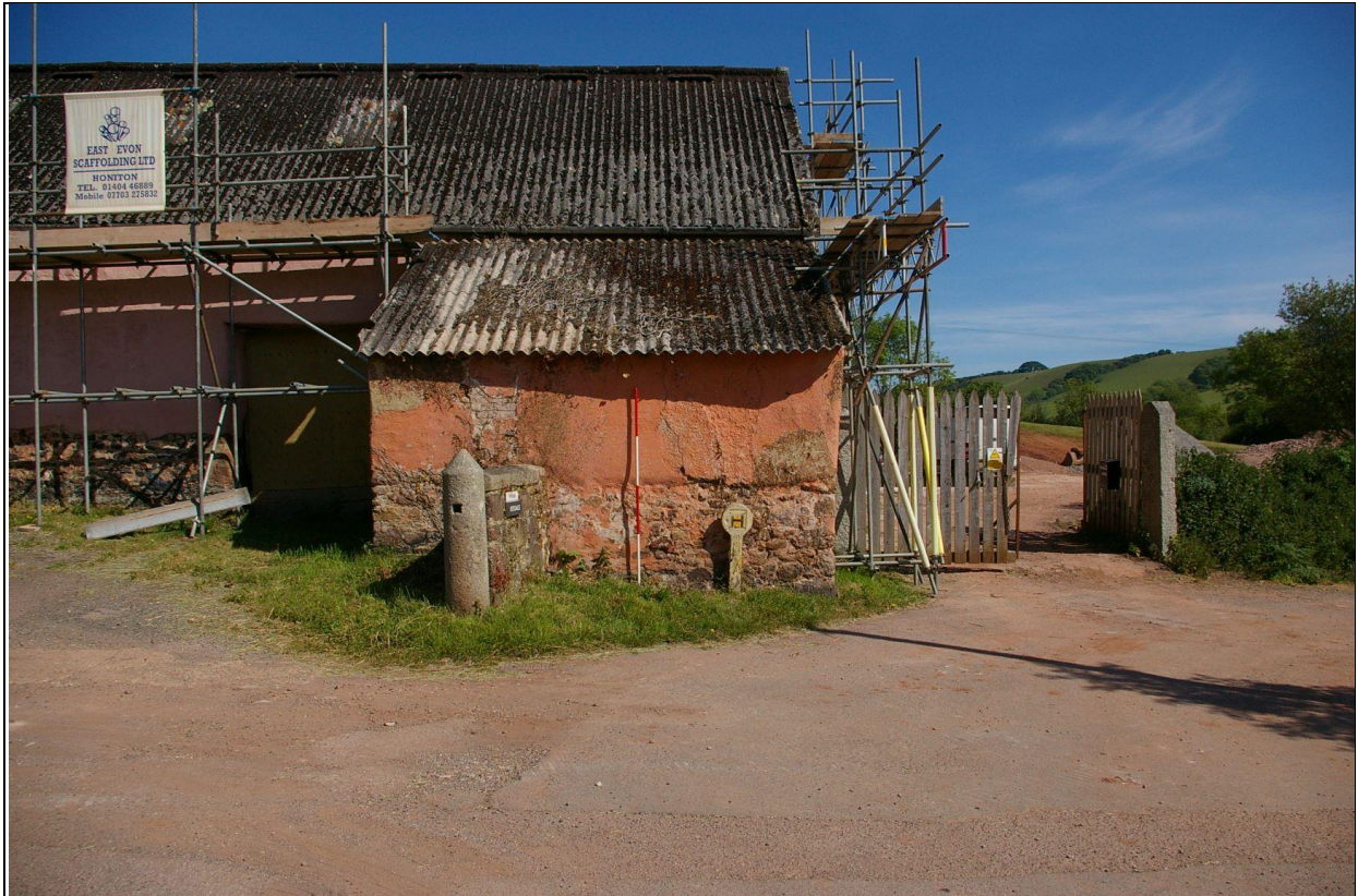
10. THE EQUIPMENT SHED, WITH 2M SCALE; FROM THE SOUTH.
