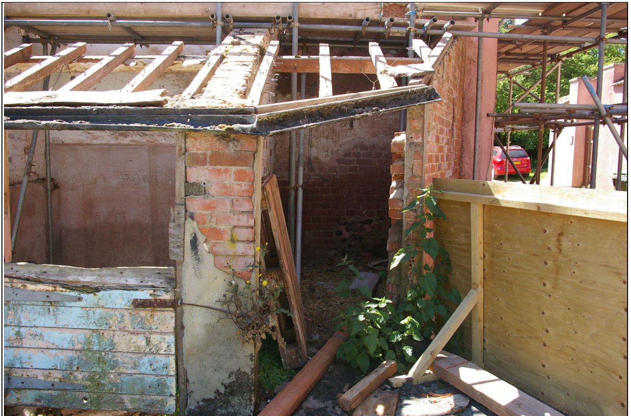
20. THE WEST SIDE OF B1.3; FROM THE NORTH.
