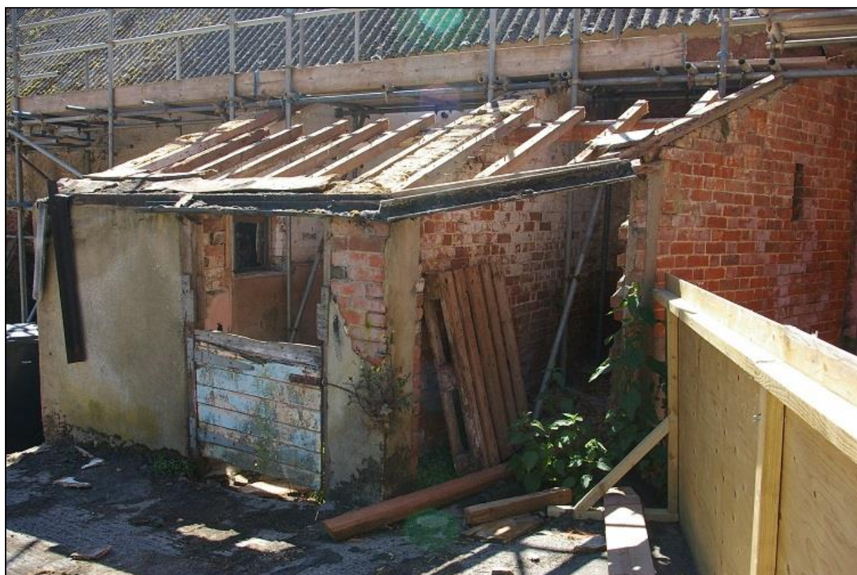
FIGURE 12: B1.3, RECTANGULAR BRICK OUTSHUT ADDED TO BARN AND ADDITIONAL SPACE FORMED IN ANGLE WITH BANK, WITH ADDITIONAL BRICK WALL, FOR STORAGE AND HOUSING MACHINERY; VIEWED FROM THE NORTH-WEST.
