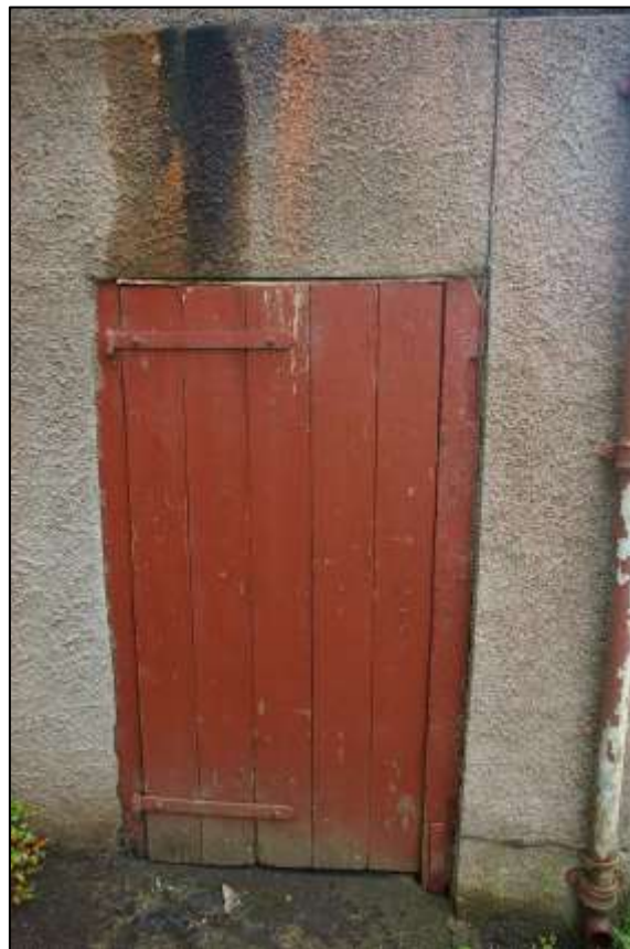
5. D3, ON THE NORTH GABLE ELEVATION; FROM THE NORTH-NORTH-WEST.
