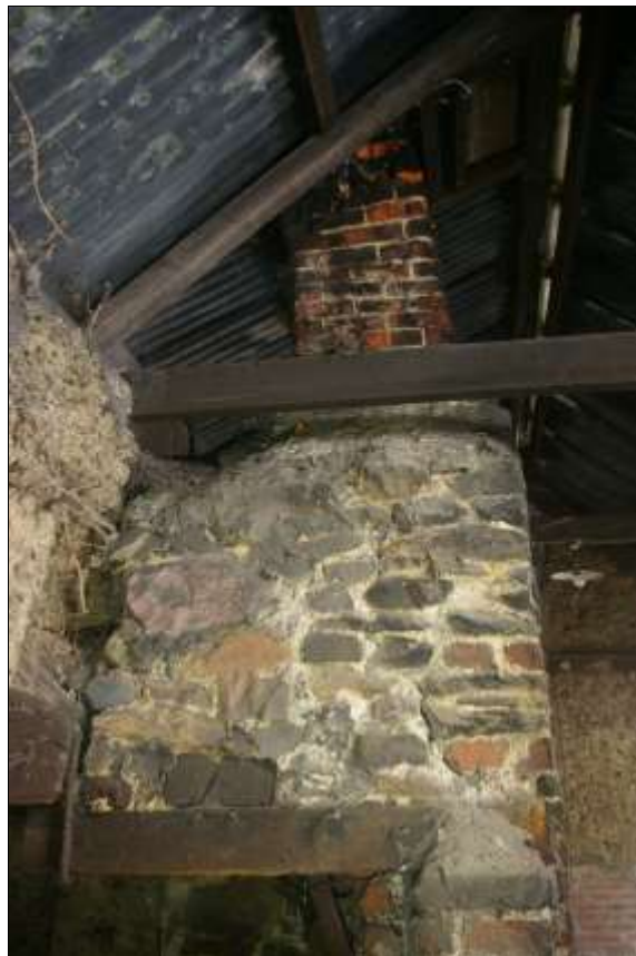
16. THE CHIMNEY TO THE FORGE, REBUILT IN BRICK; FROM THE NORTH.
