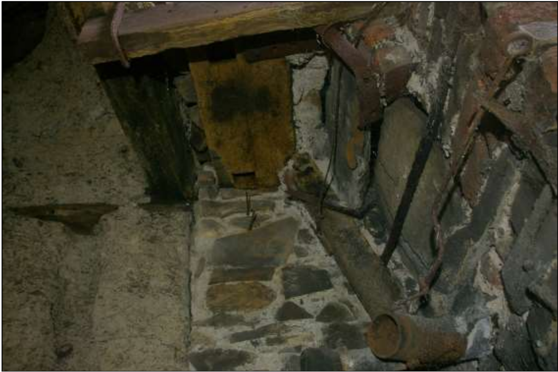
15. THE UNDERSIDE OF THE FORGE STRUCTURE.
