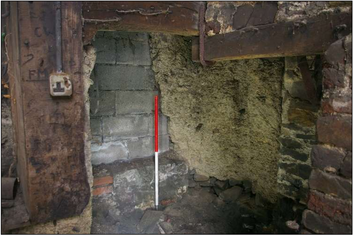
FIGURE 11: DETAIL OF THE FORGE AND EARLIER DOMESTIC FIREPLACE; FROM THE NORTH-WEST (1M SCALE).
