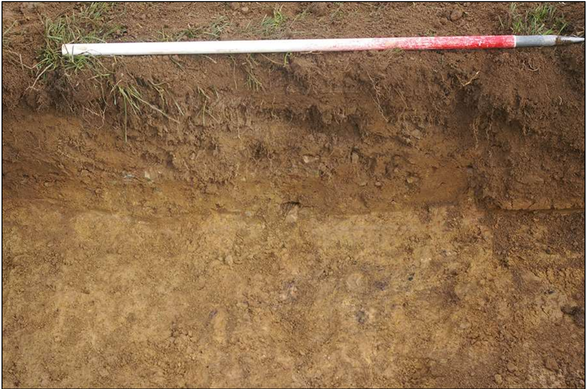
60. TRENCH 08, REPRESENTATIVE SOUTH FACING SECTION, EAST END; VIEWED FROM THE SOUTH (1M SCALE).
