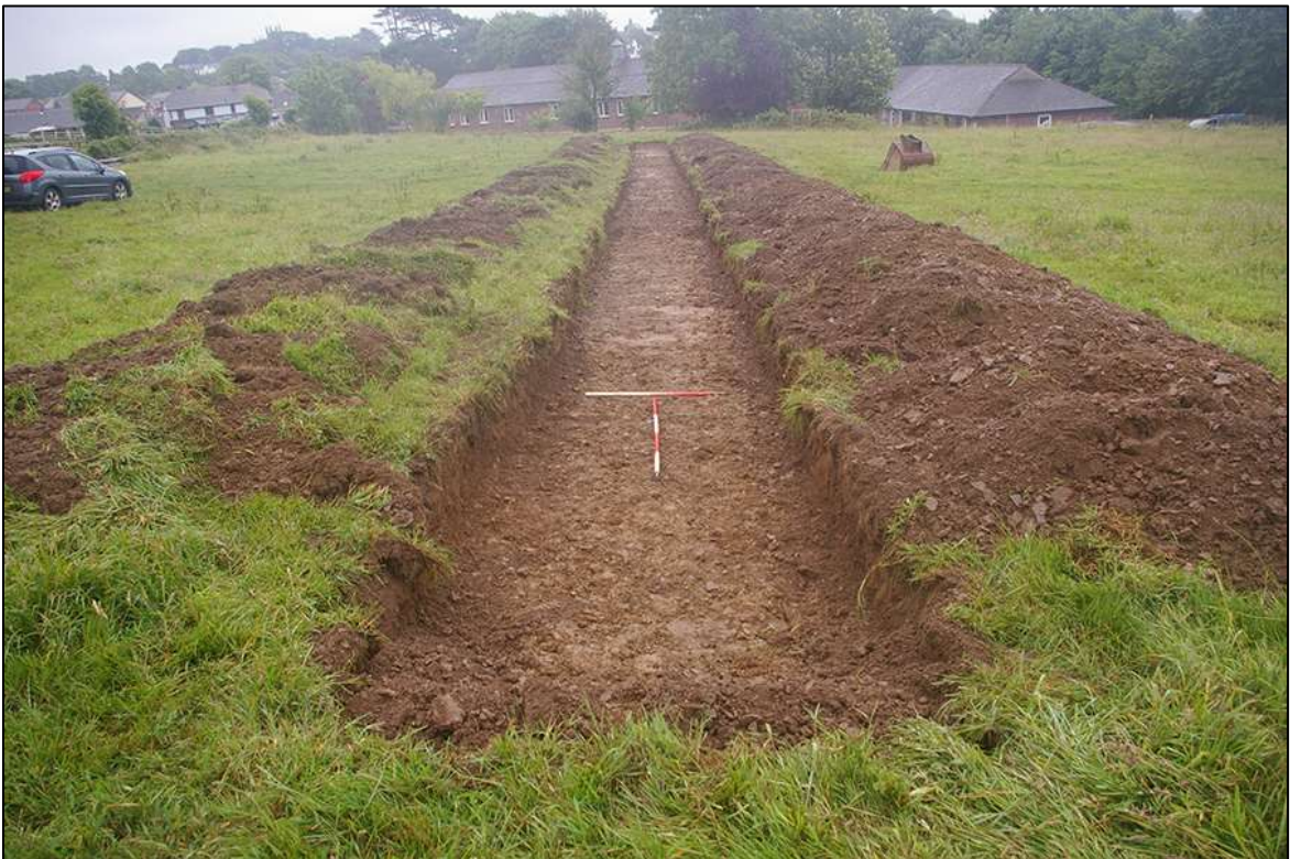
59. TRENCH 07, POST-EXCAVATION; VIEWED FROM THE NORTH-WEST (1M & 2M SCALES).
