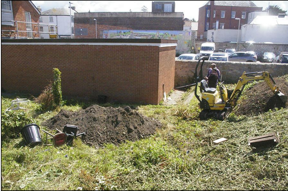
FIGURE 3: SITE SHOT, POST-EXCAVATION; VIEWED FROM THE WEST-SOUTH-WEST (NO SCALE).
