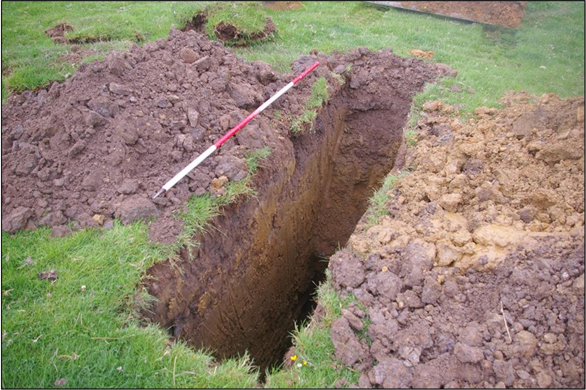
19. TRIAL-PIT 07, POST-EXCAVATION; VIEWED FROM THE EAST (2M SCALE).
