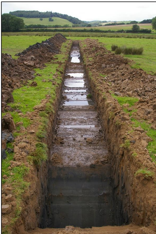
30. TRENCH 14, POST-EXCAVATION; VIEWED FROM THE SOUTH-EAST (2M SCALE).
