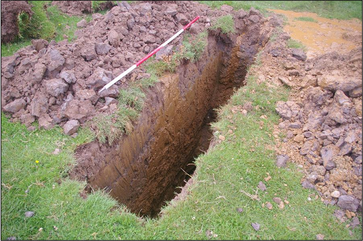
13. TRIAL-PIT 04, POST-EXCAVATION; VIEWED FROM THE EAST (2M SCALE).
