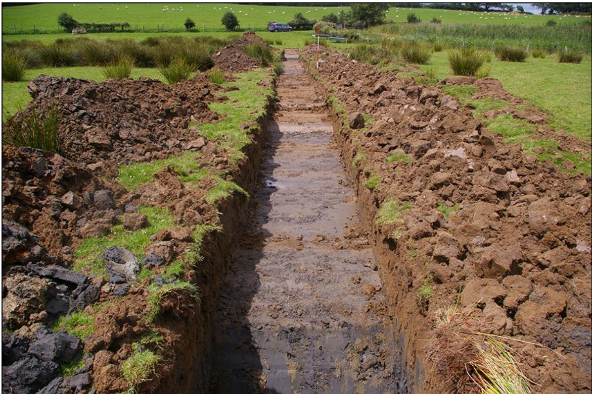
46. TRENCH 20, POST-EXCAVATION; VIEWED FROM THE SOUTH-EAST (2M SCALE).
