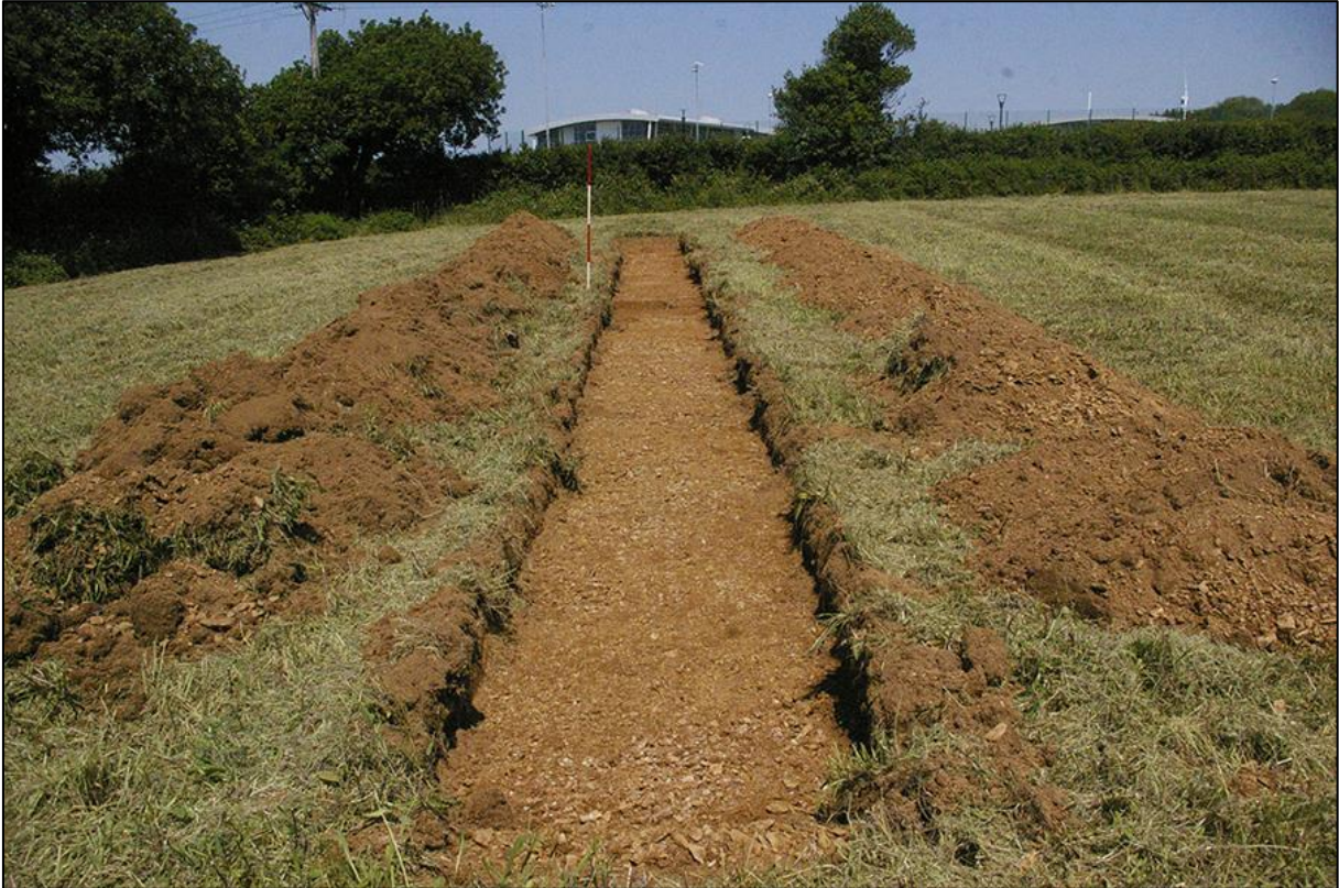
13. TRENCH 4, POST-EXCAVATION; VIEWED FROM THE SOUTH-WEST (2M SCALE).
