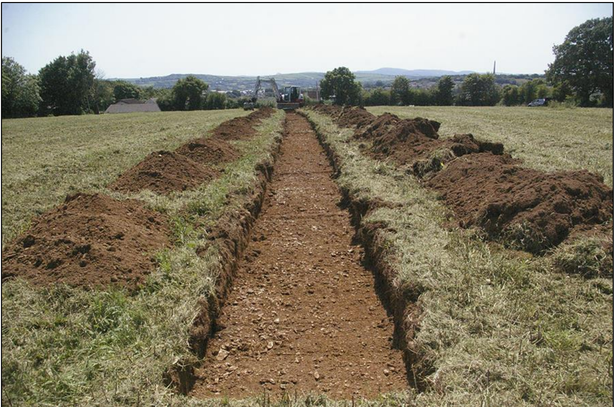
14. TRENCH 5, POST-EXCAVATION; VIEWED FROM THE NORTH-EAST (2M SCALE).
