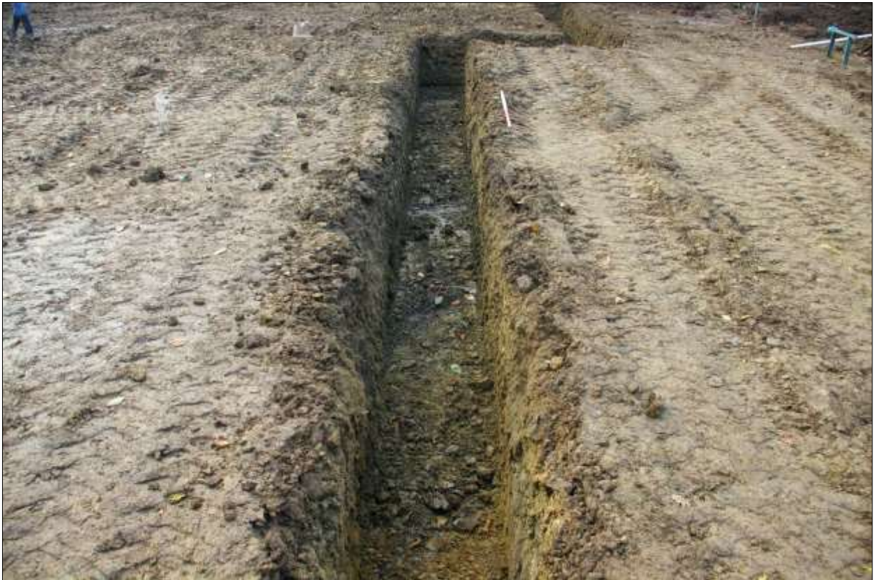
FIGURE 3: AREA STRIP FOR HOUSE PLOT FOOTINGS; FROM THE NORTH-EAST (1M SCALE).
