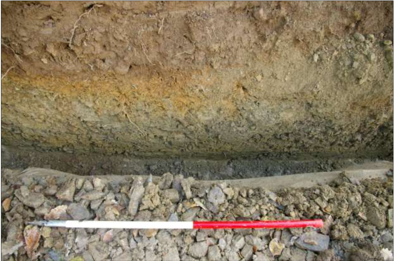
FIGURE 3: SAMPLE SECTION IN SERVICE TRENCH; FROM THE NORTH-EAST (1M SCALE).
