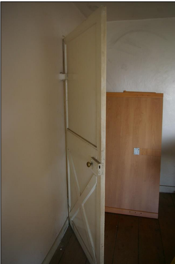
32. LEFT: R9, DETAIL OF THE TWO-PANEL DOOR; VIEWED FROM THE WEST.
