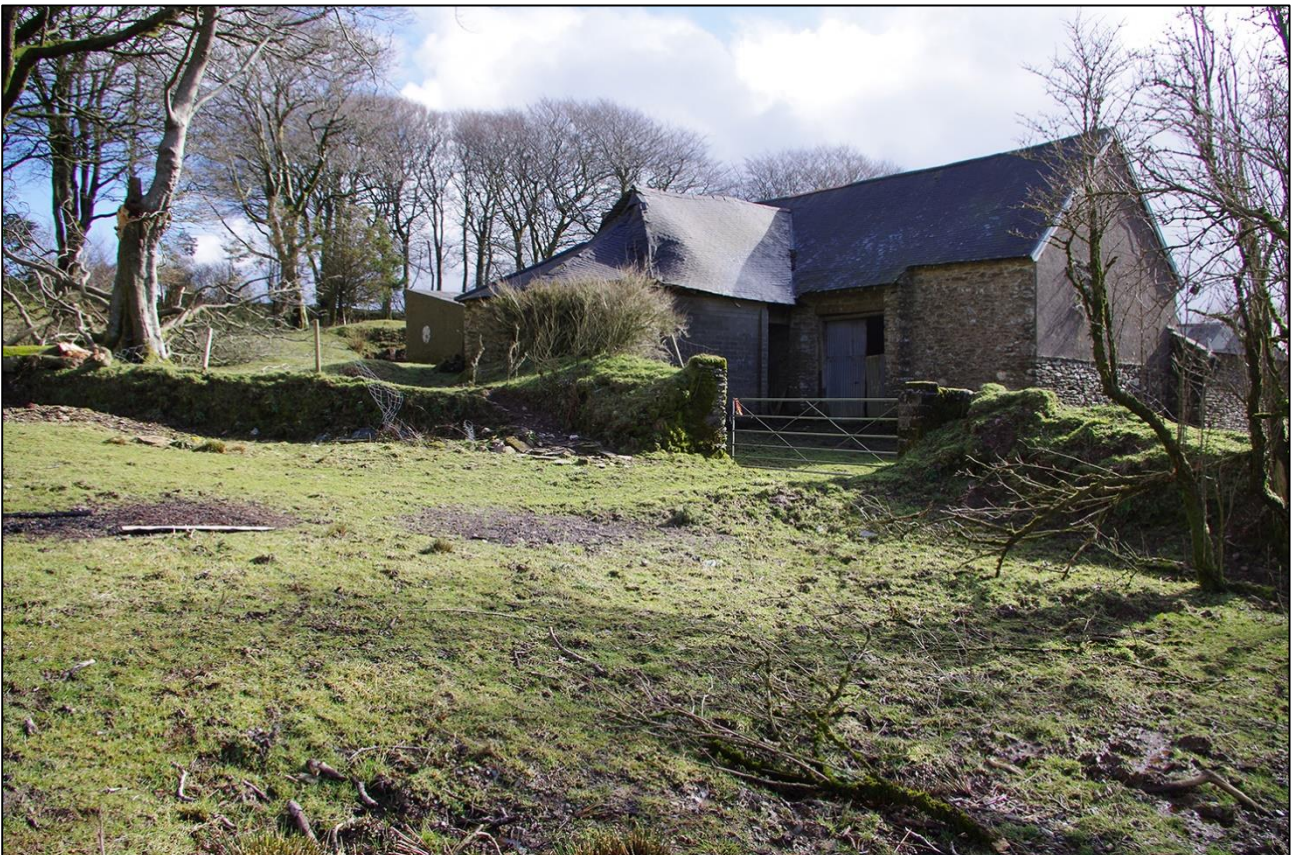
56. THE THRESHING BARN AND HORSE ENGINE HOUSE; VIEWED FROM THE NORTH-WEST.
