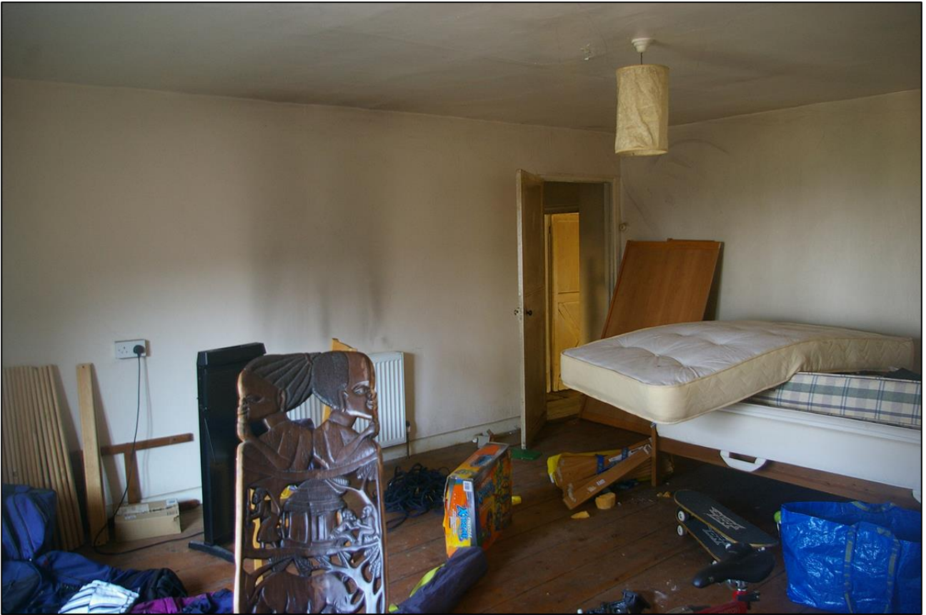
31. R9; VIEWED FROM THE SOUTH-WEST.
