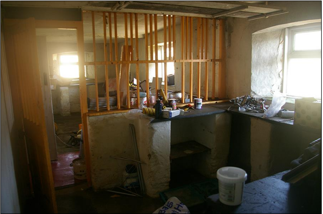
23. R5, LOOKING THROUGH FROM R5B TO R5A; VIEWED FROM THE SOUTH.
