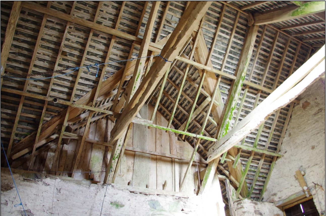
63. THE ROOF STRUCTURE IN THE THRESHING BARN; VIEWED FROM THE SOUTH-WEST.
