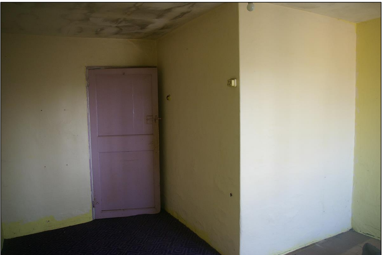
35. R10; VIEWED FROM THE NORTH-WEST.
