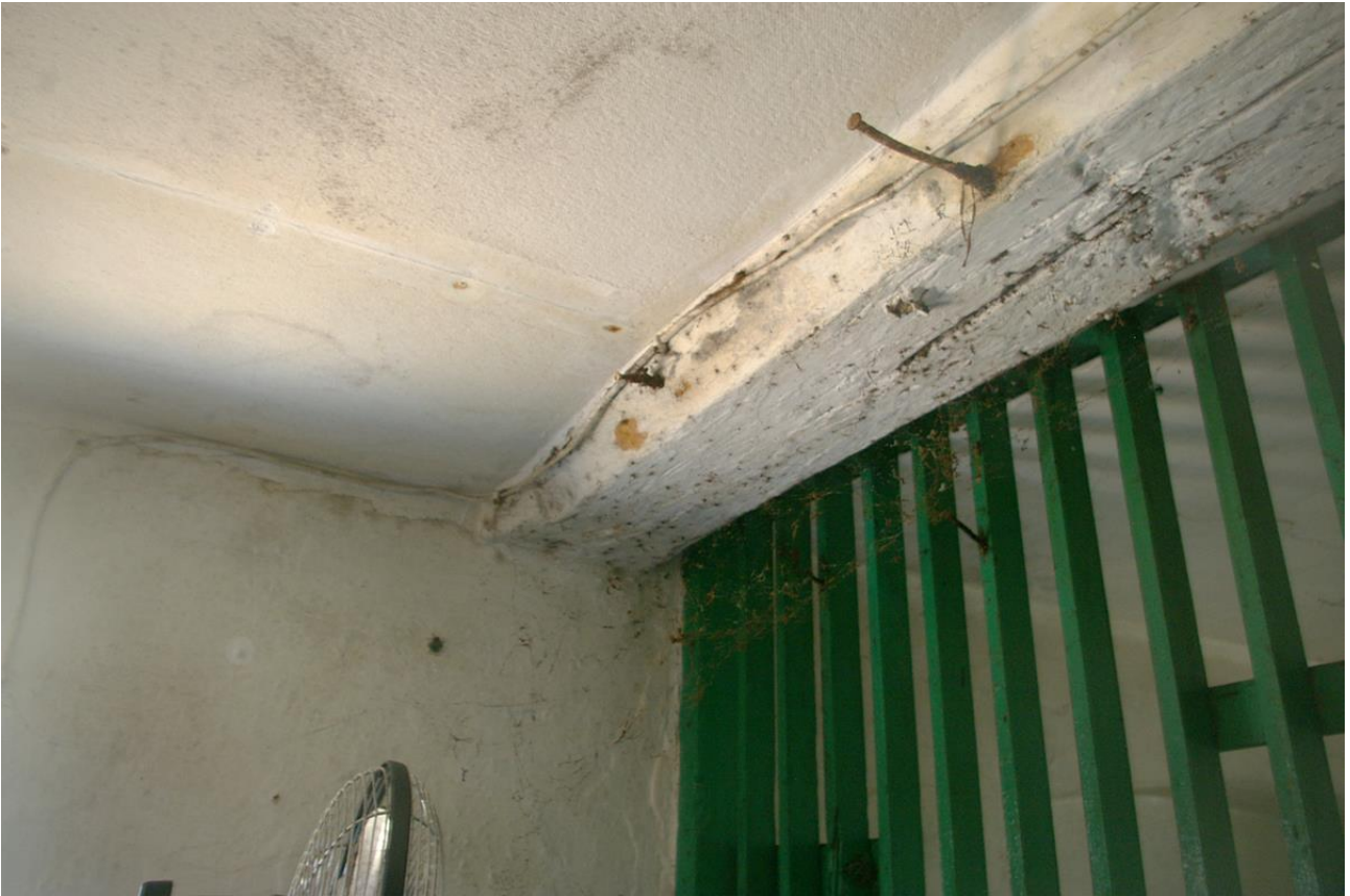
27. R5B, DETAIL OF THE RUN-OUT STOP ON THE RE-USED 17 TH CENTURY BEAM; VIEWED FROM THE WEST.
