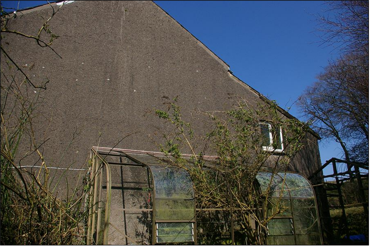
7. THE SOUTH ELEVATION OF THE FARMHOUSE; VIEWED FROM THE SOUTH.
