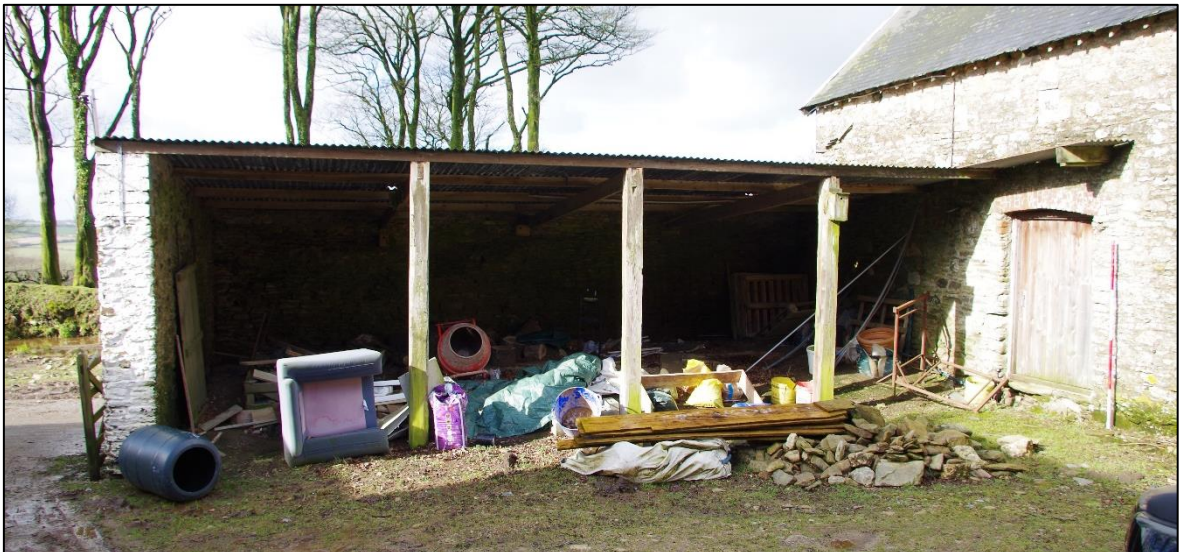
FIGURE 22: THE OPEN-FRONTED CARTSHED (B2.3); VIEWED FROM THE EAST (SCALE 2M).
