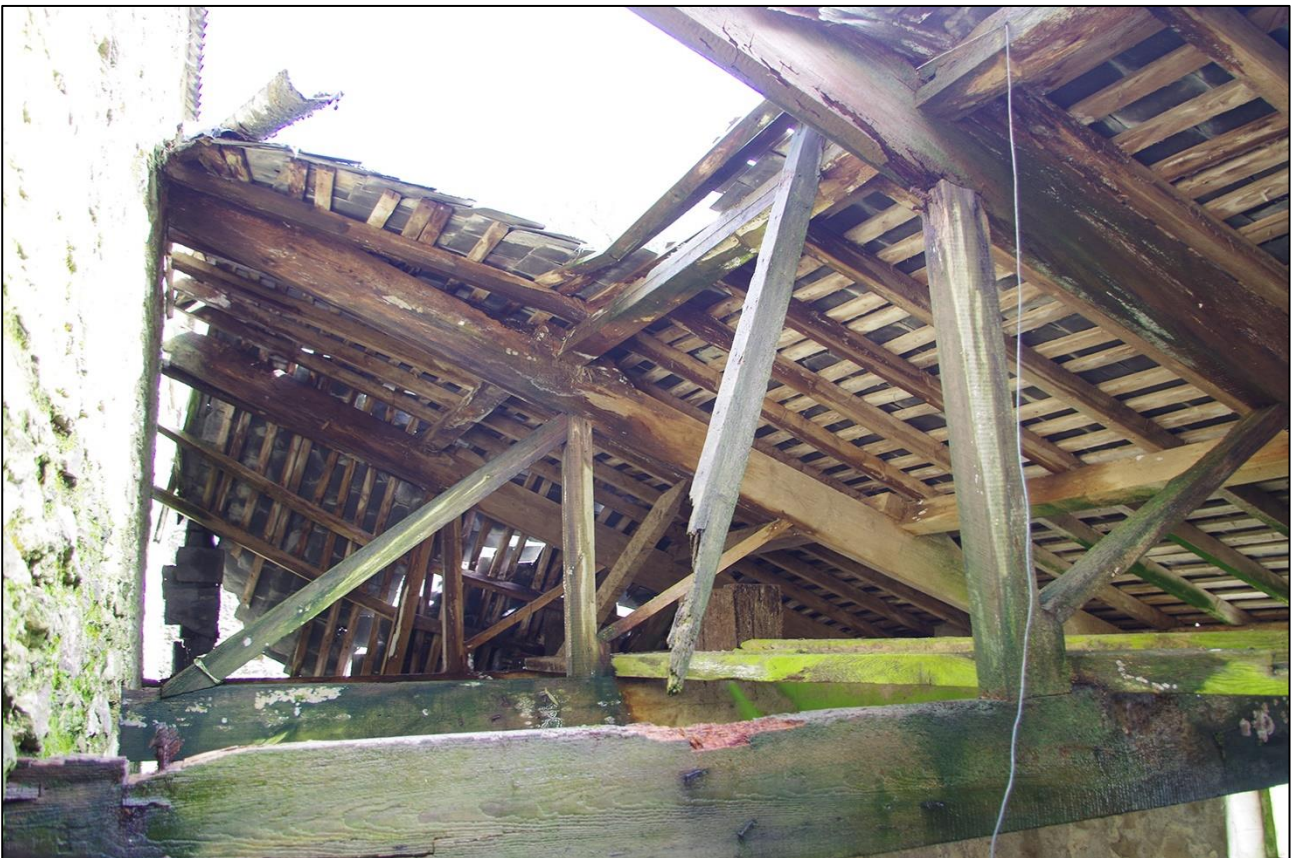
94. THE ROOF STRUCTURE OVER THE MILKING PARLOUR; VIEWED FROM THE WNW.
