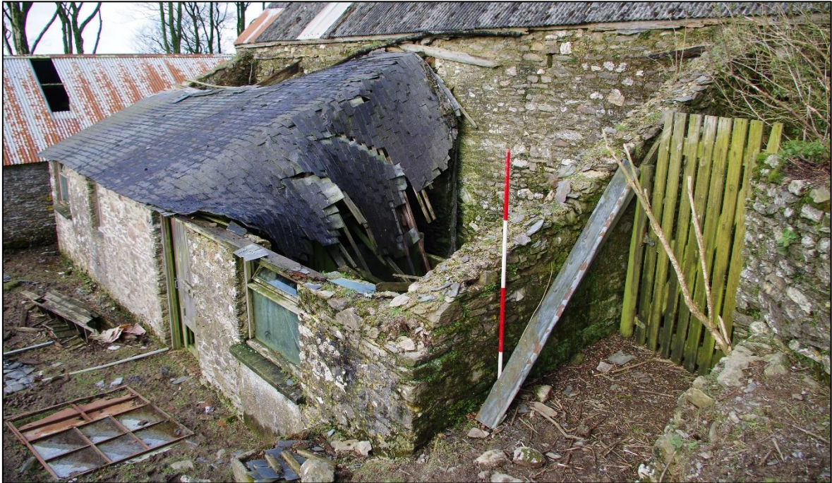
FIGURE 25: THE MILKING PARLOUR (B3.3); VIEWED FROM THE SOUTH-EAST (SCALE 2M).
