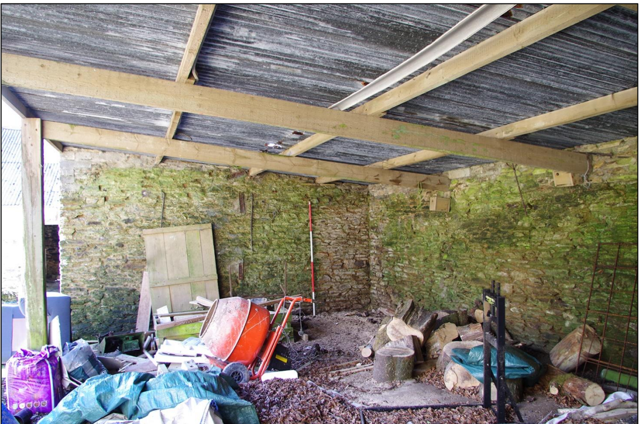
68. THE INTERIOR OF THE CARTSHED; VIEWED FROM THE NORTH (SCALE 2M).
