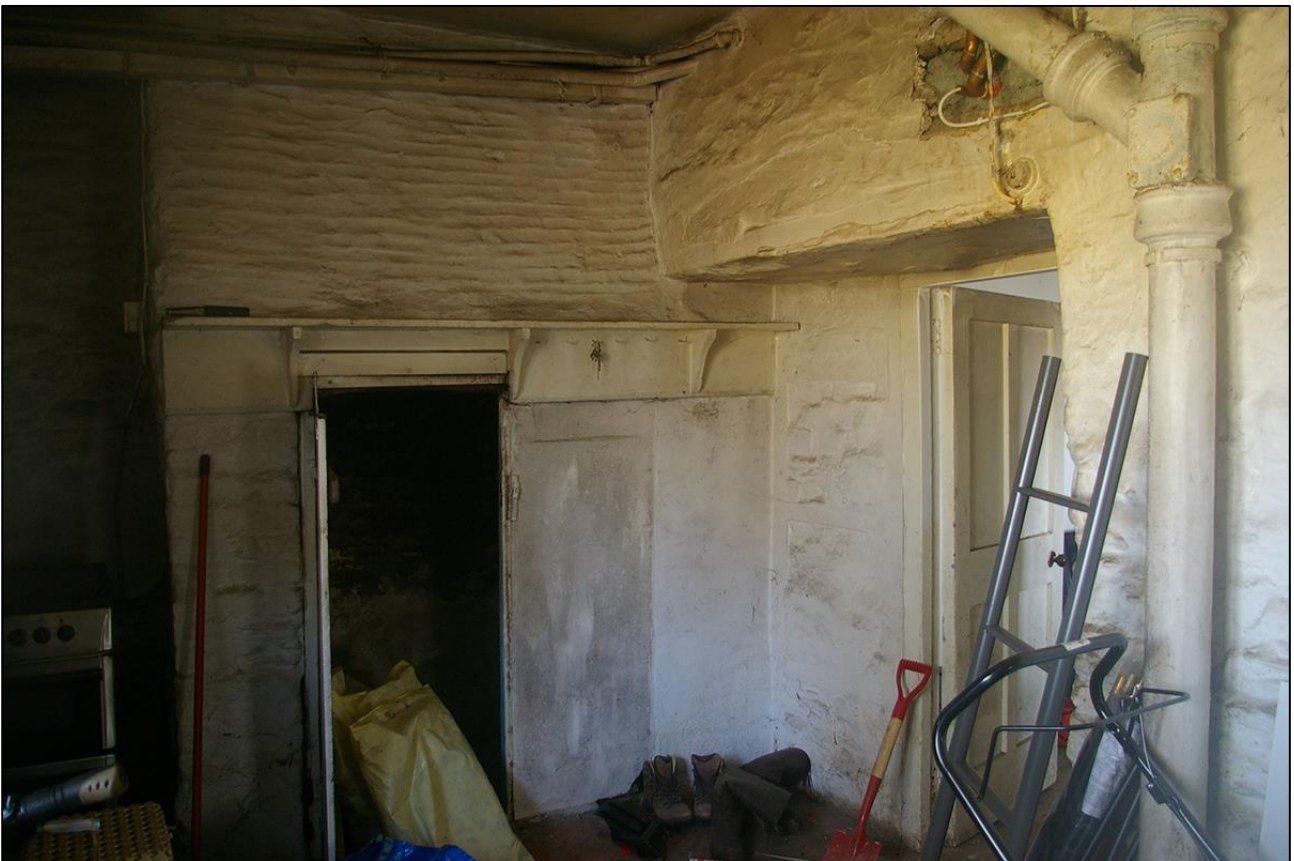
18. R6, DETAIL OF THE FORMER HEARTH; VIEWED FROM THE WEST.
