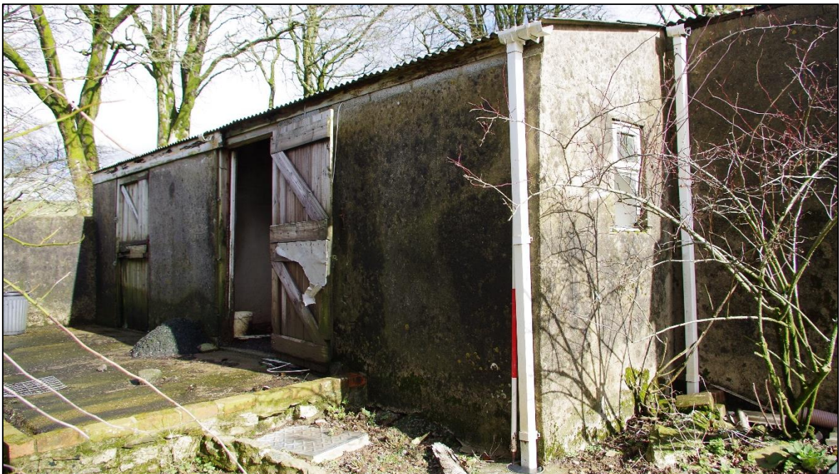
FIGURE 18: THE OUTBUILDING (B1.2); VIEWED FROM THE SOUTH-WEST (SCALE 2M).
