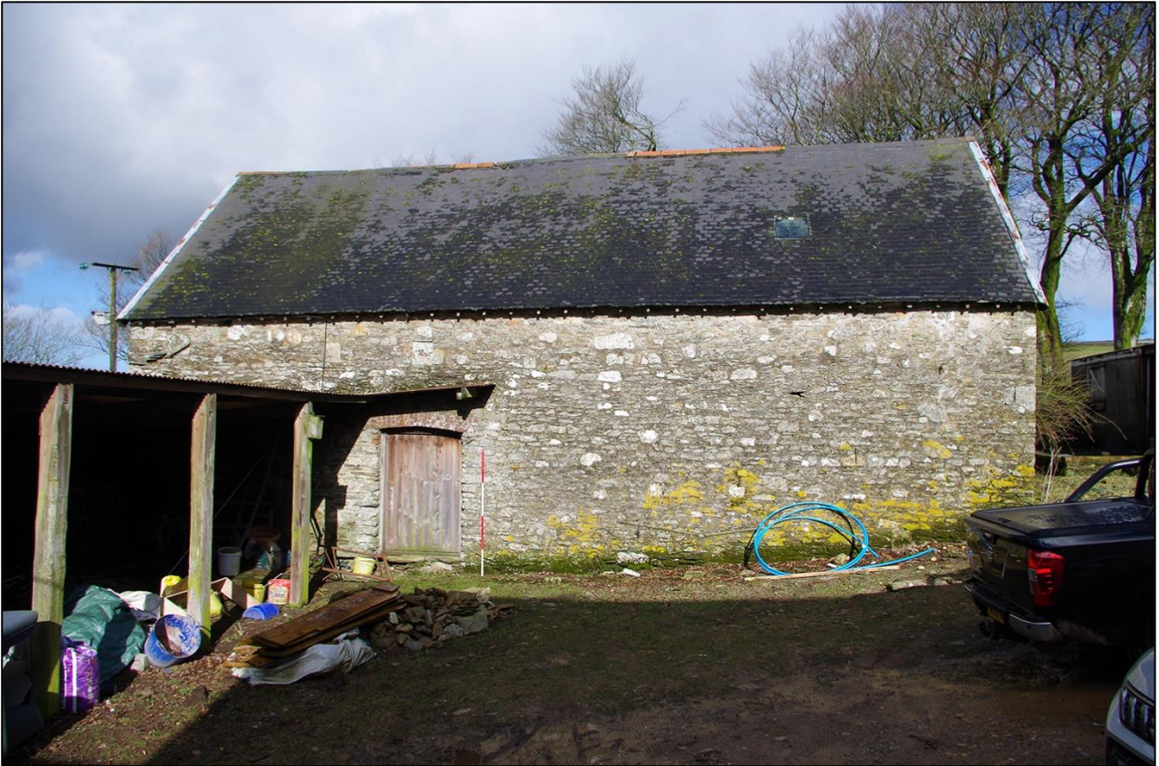
44. THRESHING BARN; VIEWED FROM THE SOUTH.
