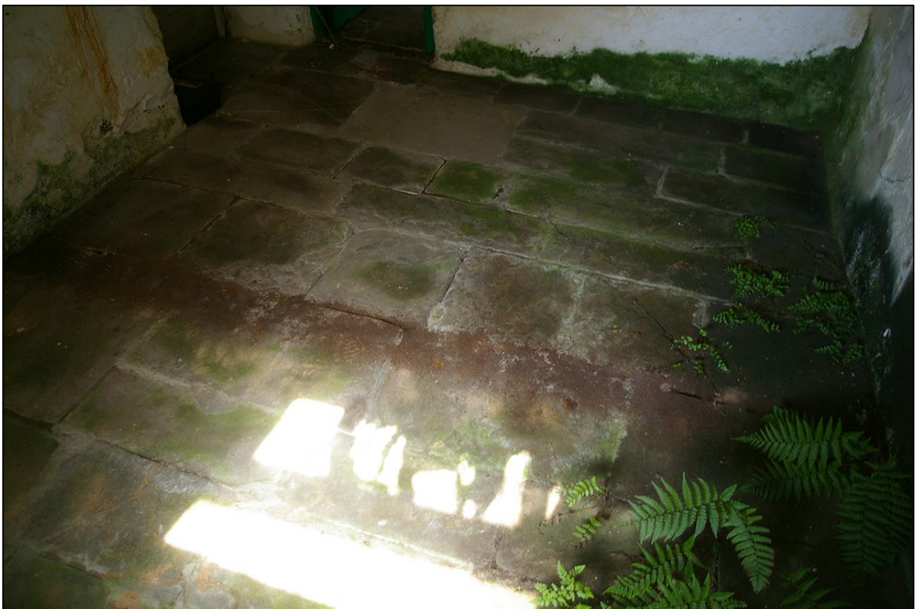
28. R5C, DETAIL OF THE SLATE FLAGSTONE FLOOR; VIEWED FROM THE SOUTH.
