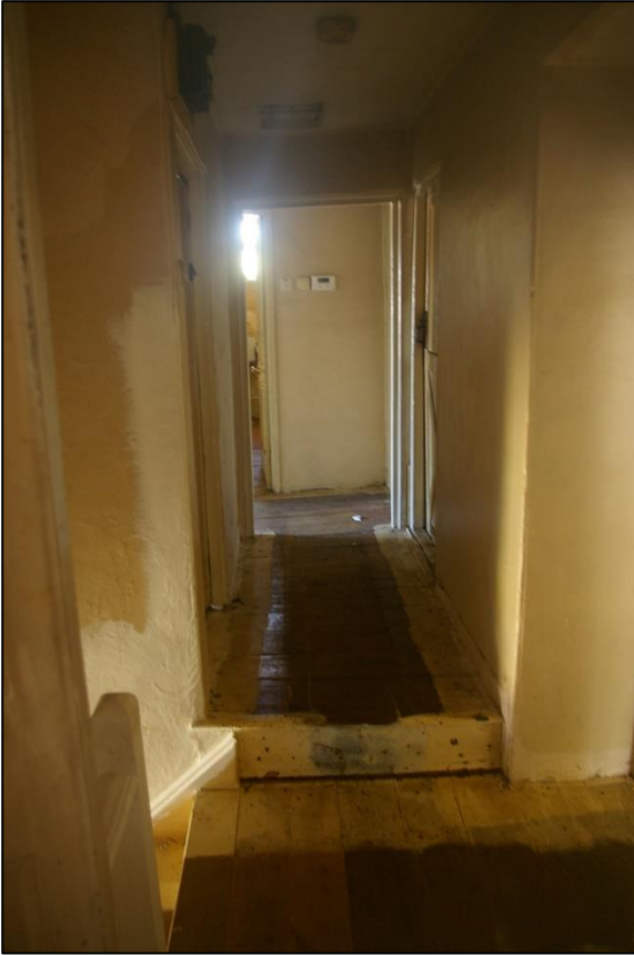
29. R8, THE FIRST-FLOOR LANDING; VIEWED FROM THE SOUTH.
