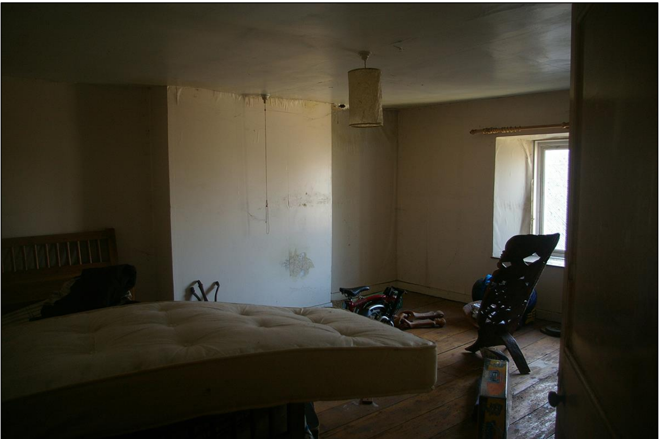
30. R9; VIEWED FROM THE NORTH-EAST.
