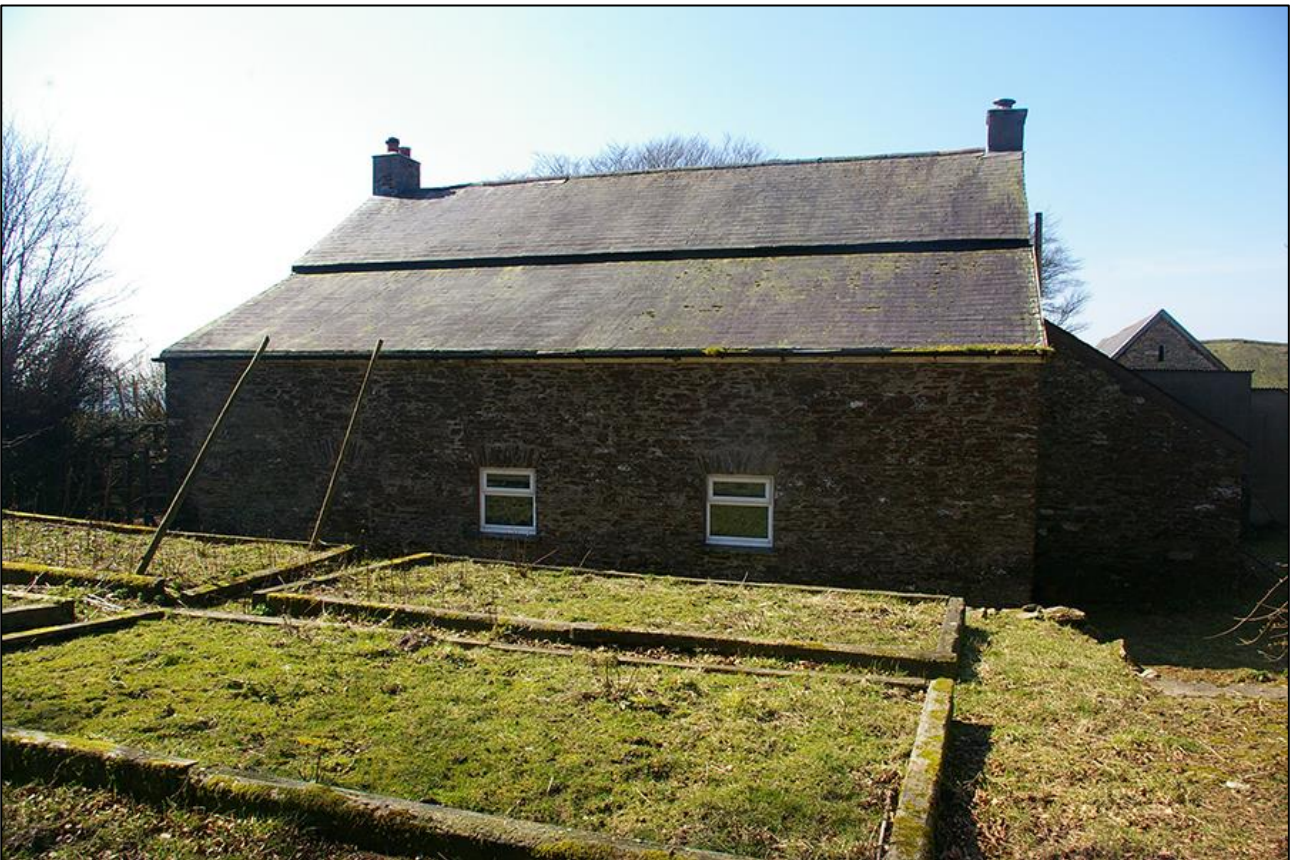
6. THE EAST ELEVATION OF THE FARMHOUSE; VIEWED FROM THE EAST.
