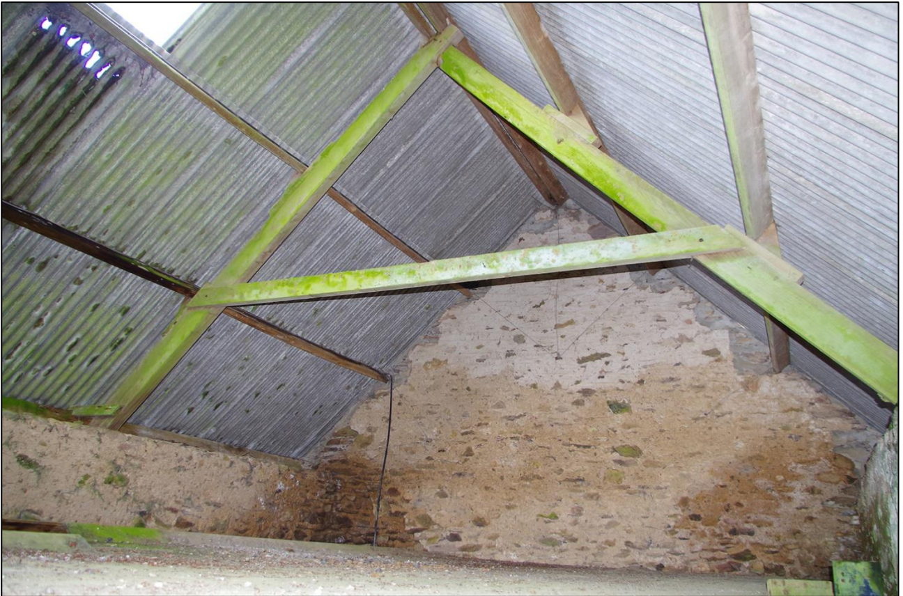
86. THE FIRST-FLOOR LOFT OVER THE STABLES; VIEWED FROM THE SSW.
