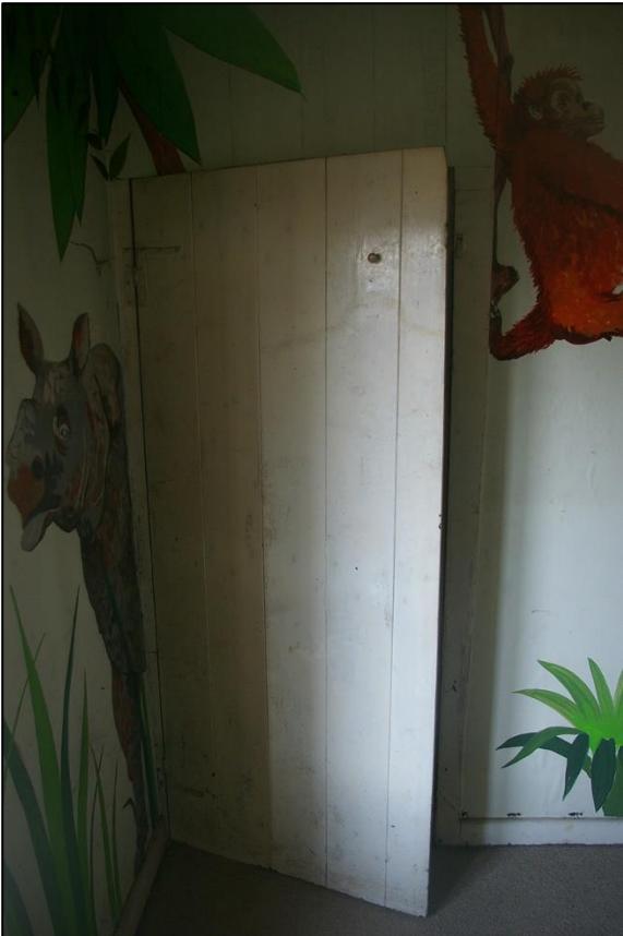
39. R12, DETAIL OF THE CUPBOARD DOOR TO THE WEST OF THE STACK; VIEWED FROM THE SOUTH.
