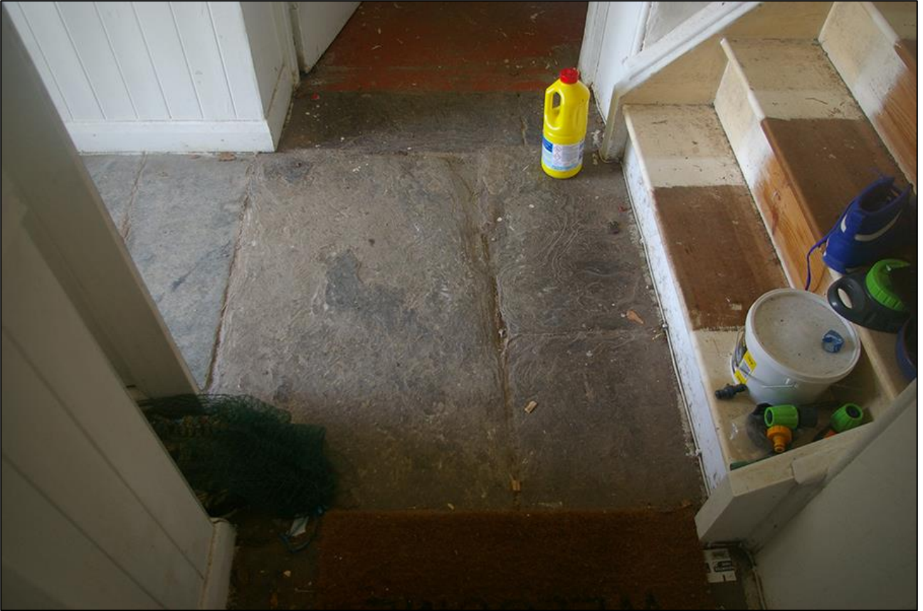
10. R2, DETAIL OF THE SLATE FLAGSTONES; VIEWED FROM THE SOUTH.
