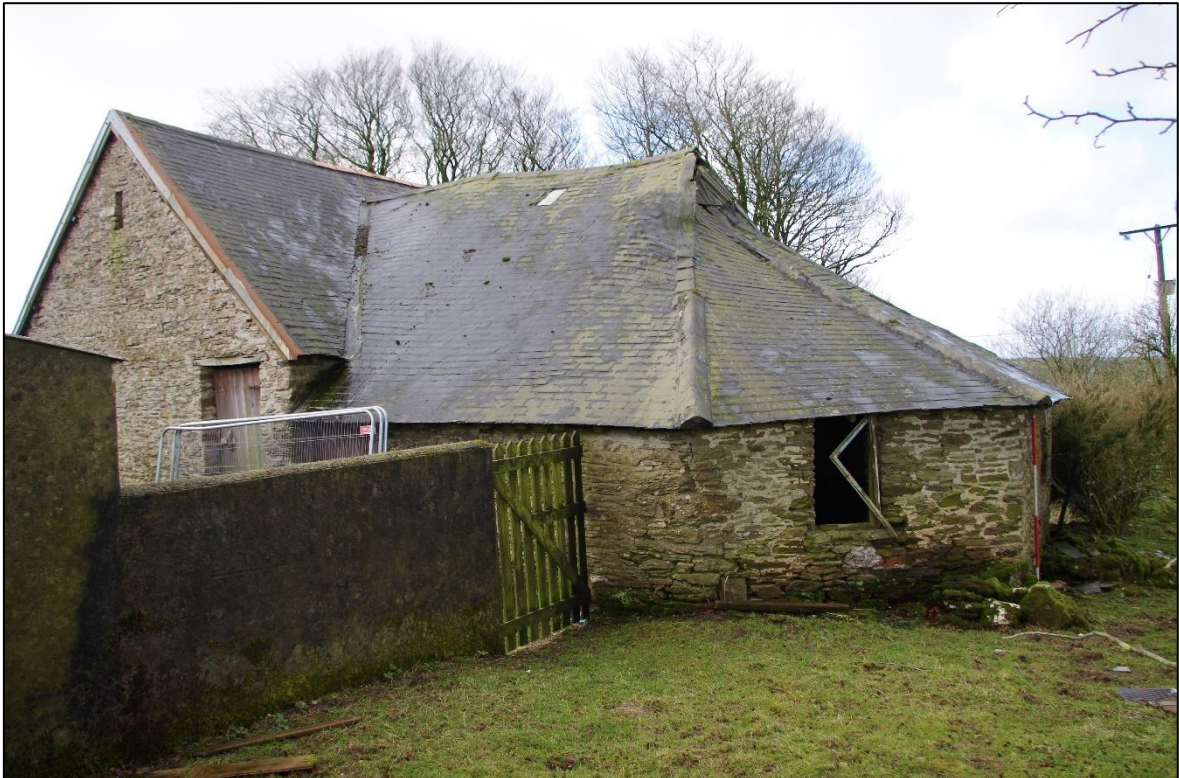
FIGURE 21: THE HORSE ENGINE HOUSE (B2.2); VIEWED FROM THE ENE (SCALE 2M).
