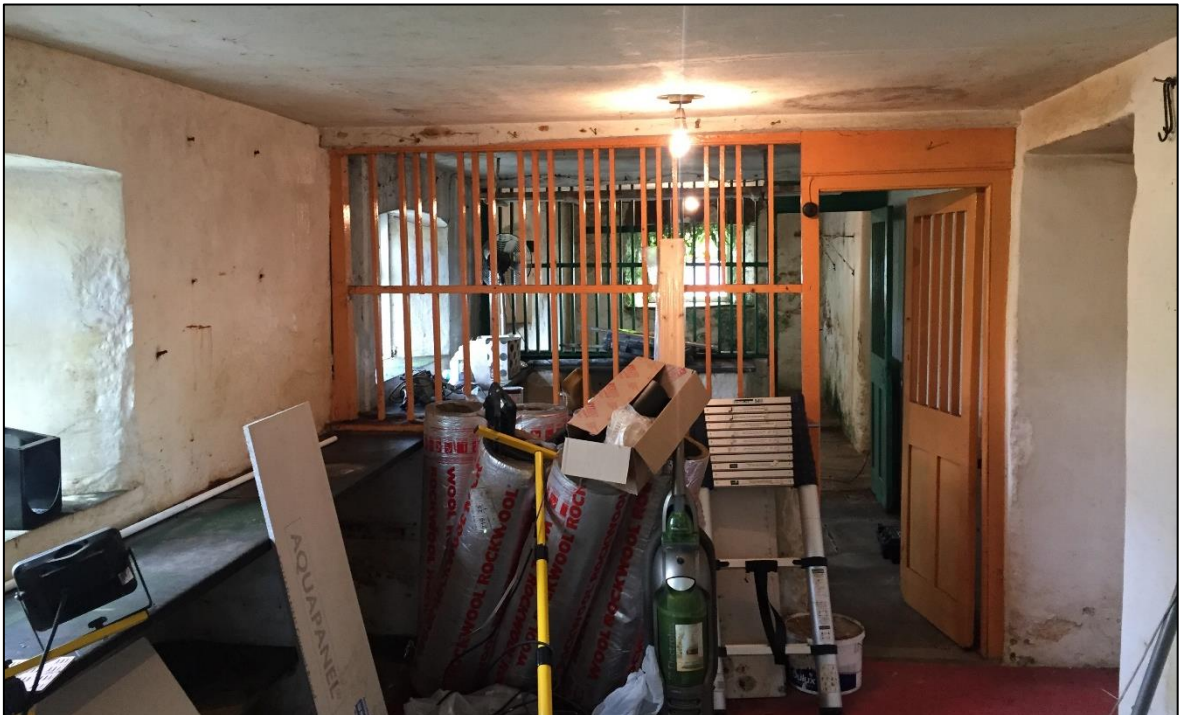
FIGURE 17: THE INTERIOR OF R15; VIEWED FROM THE NORTH.
