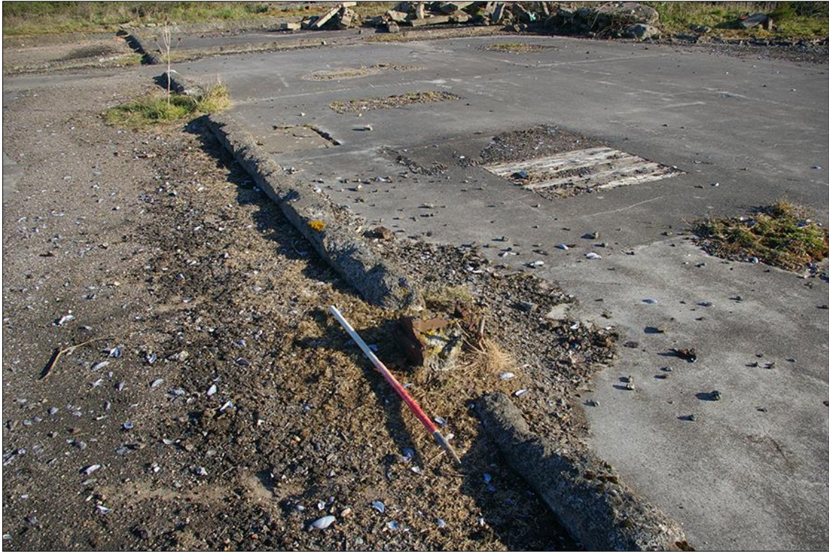
11. DETAIL OF ONE OF THE CONCRETE BUILDING FOOTPRINTS SURVIVING ON THE SITE, DEMONSTRATING SURVIVING STEEL FRAME CONSTRUCTION; VIEWED FROM THE SOUTH-WEST (1M SCALE).
