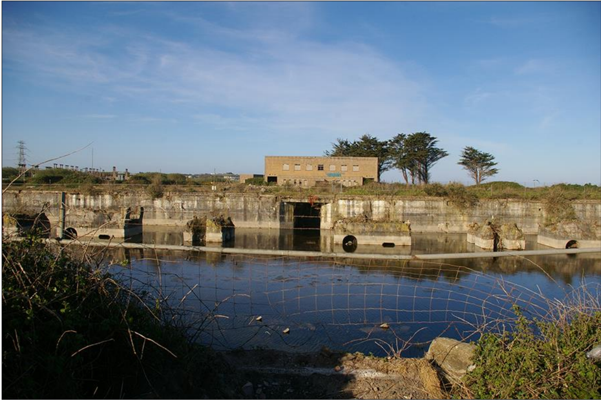
7. VIEW ACROSS THE FLOODED BOILER- AND TURBINE-HOUSE TO THE SWITCH-HOUSE; VIEWED FROM THE EAST (NO SCALE).
