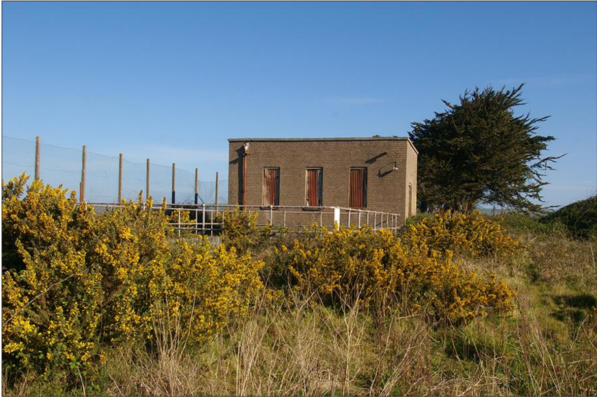
23. SOUTH EXTERNAL ELEVATION OF THE PUMP-HOUSE, WITH SETTLING TANK TO THE FOREGROUND; VIEWED FROM THE SOUTH-SOUTH-EAST (NO SCALE).
