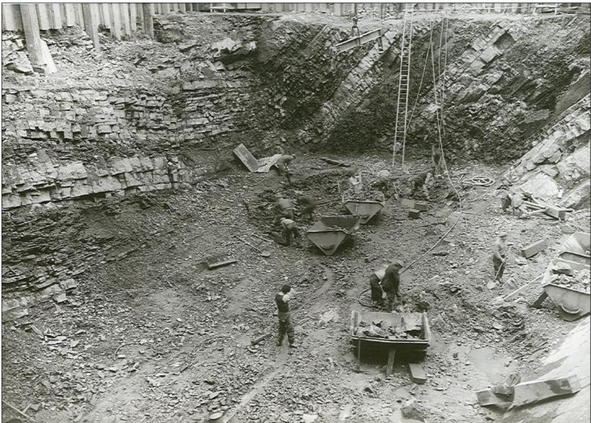
FIGURE 4: PHOTOGRAPH TAKEN DURING EXCAVATION OF ONE OF THE PUMP CHAMBERS (SOURCE: PRIVATE COLLECTION).
