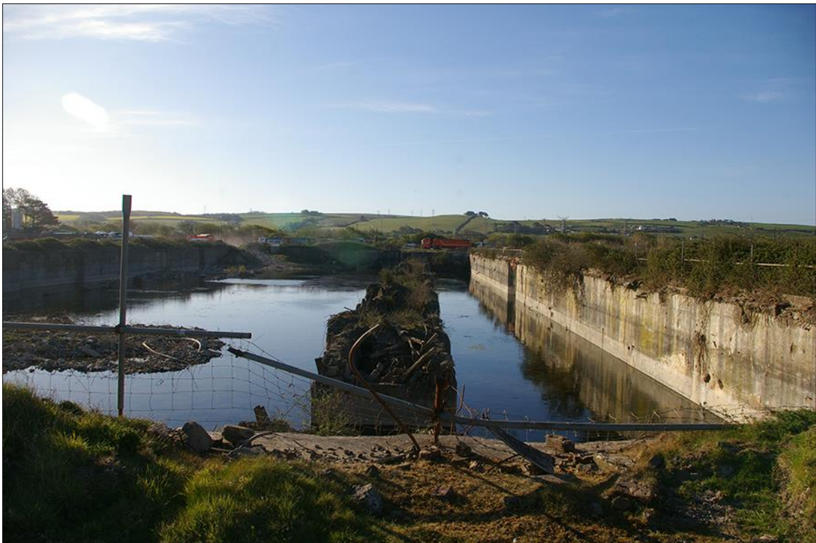
8. VIEW ACROSS THE FLOODED BOILER- AND TURBINE-HOUSE; VIEWED FROM THE NORTH (NO SCALE).
