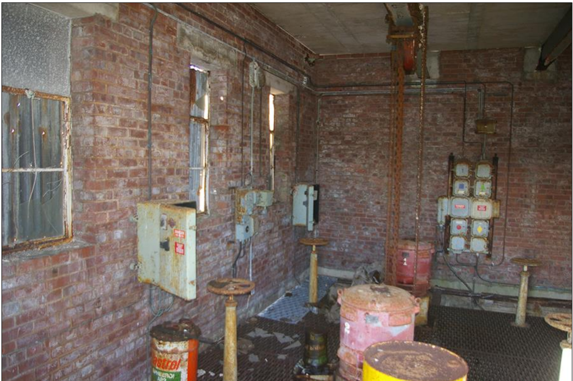
FIGURE 20: INTERIOR VIEW OF THE SURVIVING PUMP-HOUSE; VIEWED FROM THE EAST-NORTH-EAST.
