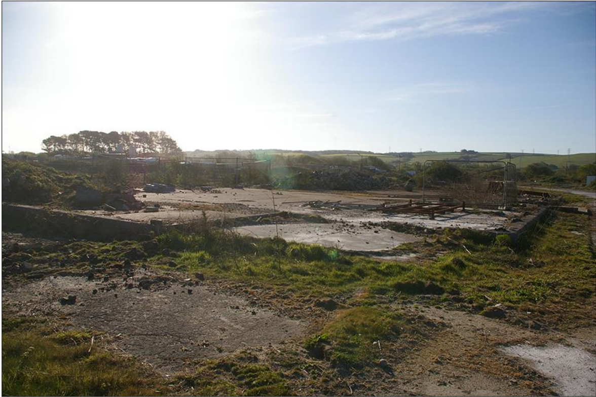
15. DETAIL OF THE SURVIVING FOOTPRINT OF THE CONTROL ROOM AND OFFICE BLOCK; VIEWED FROM THE NORTH-WEST (NO SCALE).
