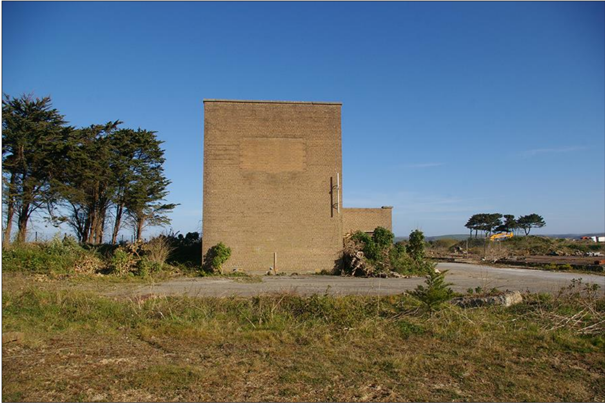
21. SOUTH EXTERNAL ELEVATION OF THE SWITCH-HOUSE; VIEWED FROM THE SOUTH (1M SCALE).
