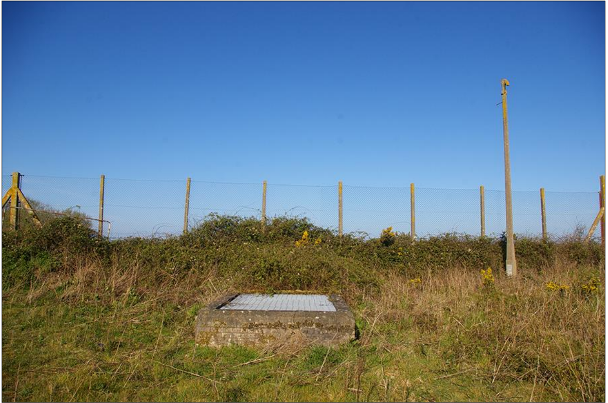
27. DETAIL OF THE COVERED INLET/OUTLET TUNNELS AT THE WESTERN END OF THE SITE; VIEWED FROM THE EAST (NO SCALE).
