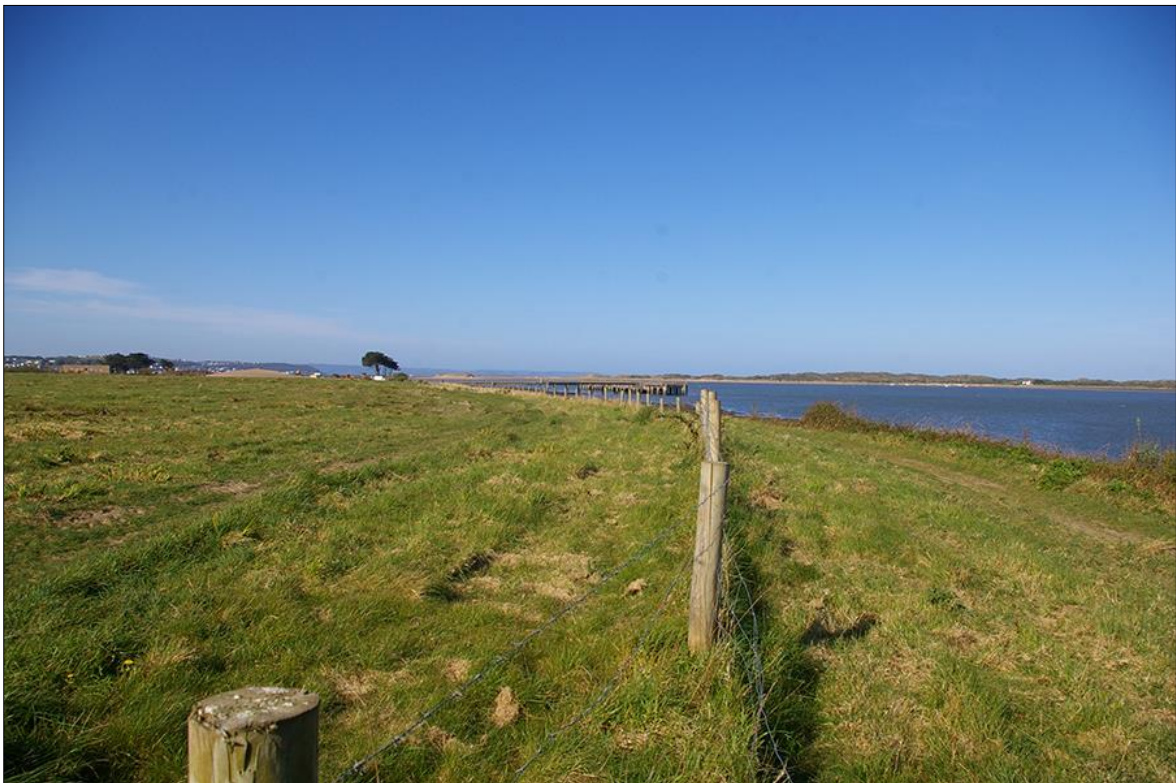
36. VIEW ALONG THE NORTHERN EDGE OF AREA 02 OF THE PROPOSAL SITE TOWARDS THE JETTY; VIEWED FROM THE EAST-SOUTH-EAST (NO SCALE).
