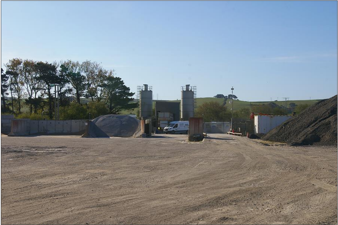
FIGURE 17: THE CONCRETE PROCESSING AREA OF THE SOUTH-EAST QUADRANT; VIEWED FROM THE NORTH-WEST.
