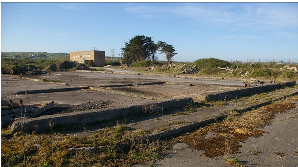
FIGURE 21: DETAIL OF THE SURVIVING BUILDING FOOTPRINTS, DEMONSTRATING STEEL FRAME AND CONCRETE CONSTRUCTION; VIEWED FROM THE NORTH-EAST.
