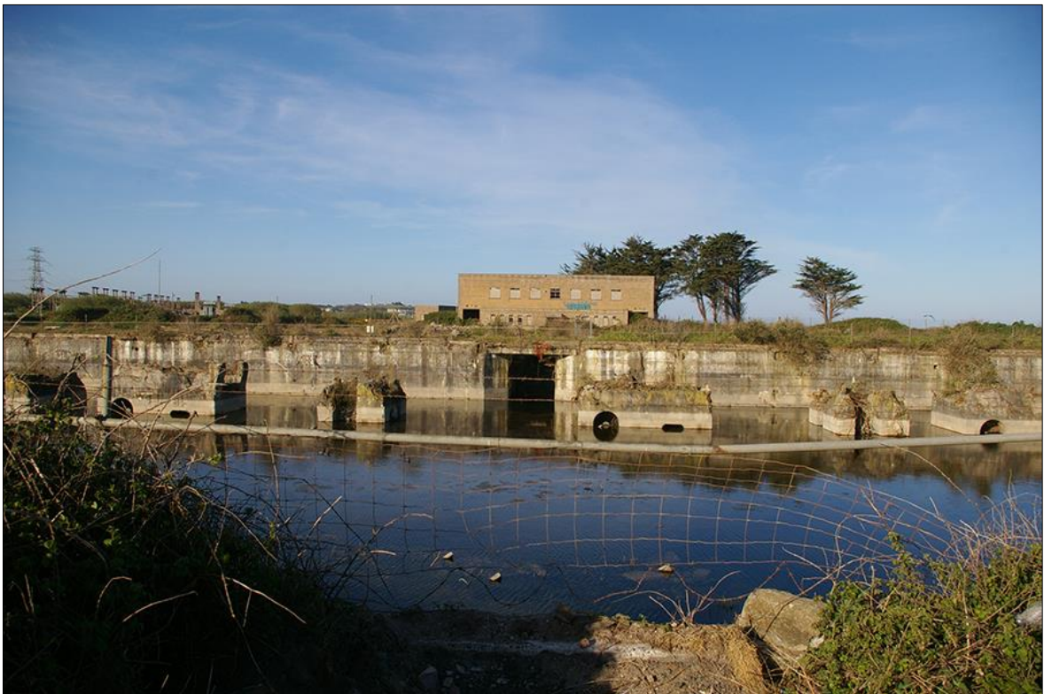
FIGURE 18: VIEW ACROSS THE FLOODED BASEMENT LEVELS OF THE DEMOLISHED BOILER- AND TURBINE-HOUSE TO THE STANDING SWITCH-HOUSE (CENTRE) AND PUMP-HOUSE (CENTRE-LEFT) STRUCTURES; VIEWED FROM THE EAST.
