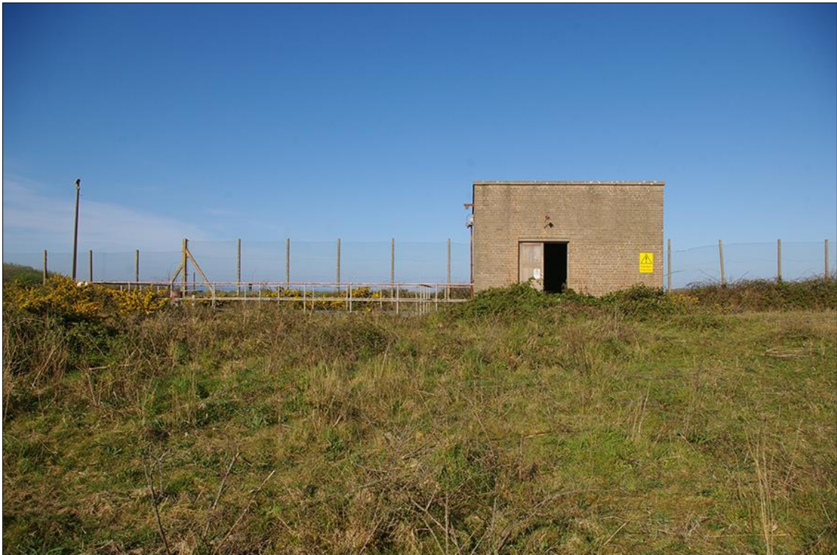
24. EAST EXTERNAL ELEVATION OF THE PUMP-HOUSE AND SETTLING TANK; VIEWED FROM THE EAST (NO SCALE).
