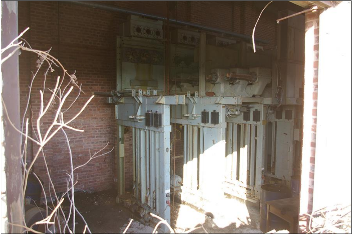
FIGURE 19: INTERIOR OF THE SWITCH-HOUSE, SHOWING SURVIVING MACHINERY; VIEWED FROM THE SOUTH-EAST.
