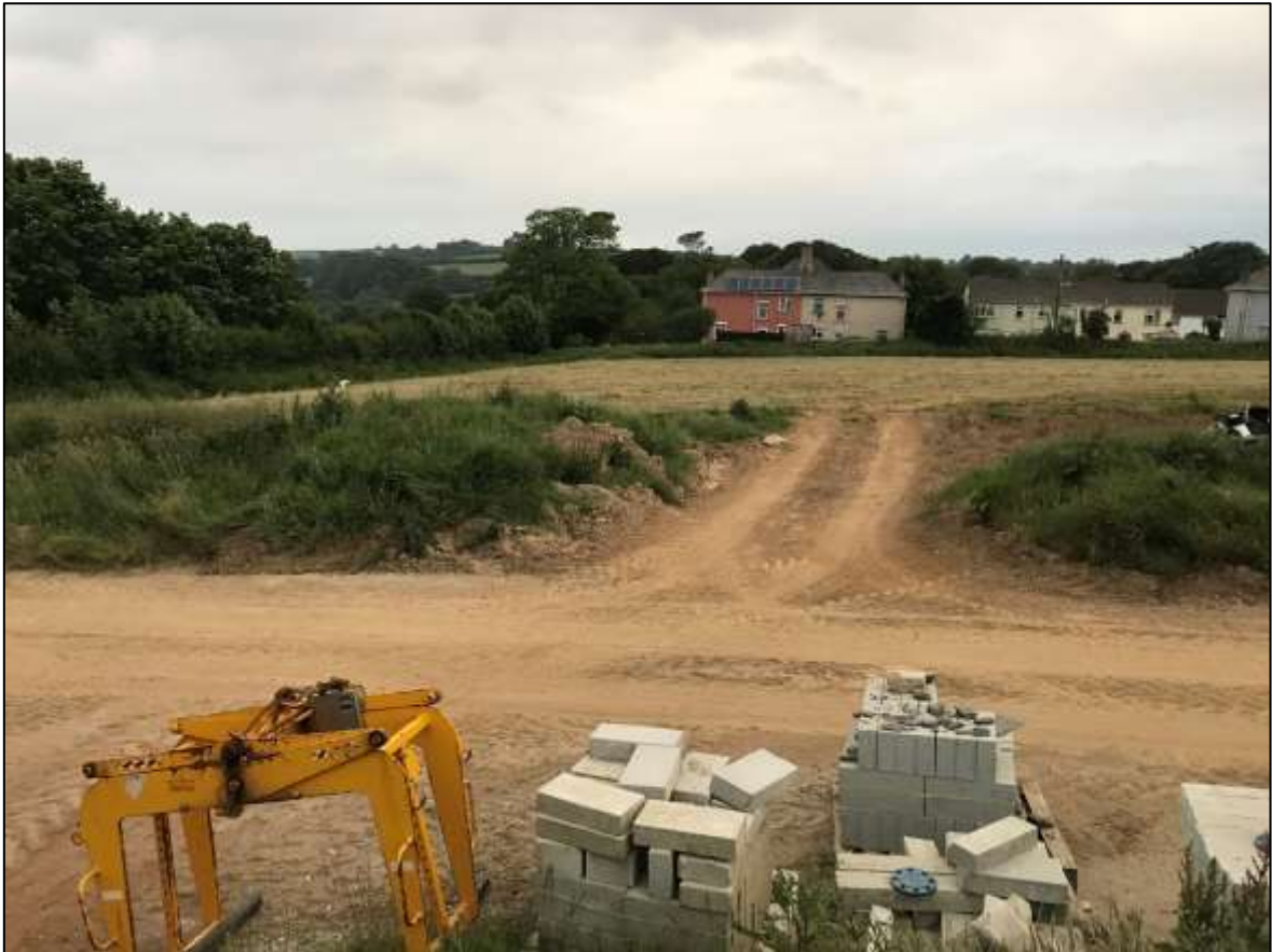
FIGURE 2: VIEW ACROSS THE SOUTHERN PART OF THE PHASE 2 SITE SHOWING THE TRACK; VIEWED FROM THE EAST.
