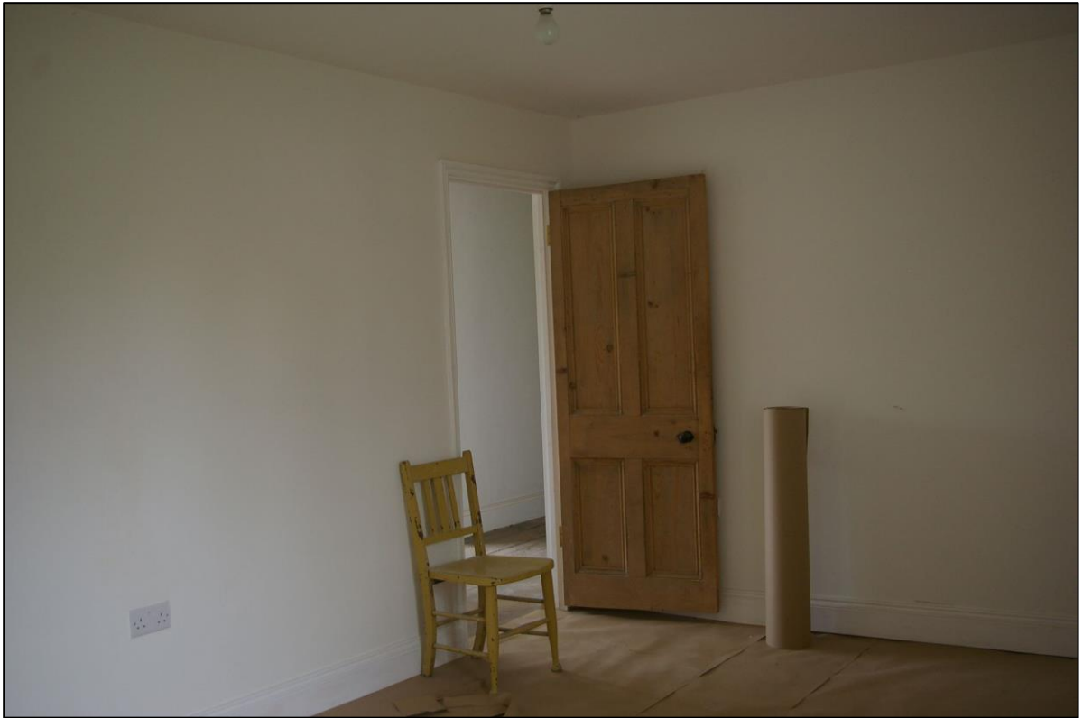
55. ROOM 17 WITH THE PANELLED DOOR TO R13; FROM THE NORTH-EAST.
