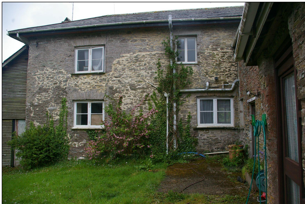
FIGURE 5: THE NORTH ELEVATION OF THE MAIN RANGE; FROM THE NORTH-NORTH-WEST.
