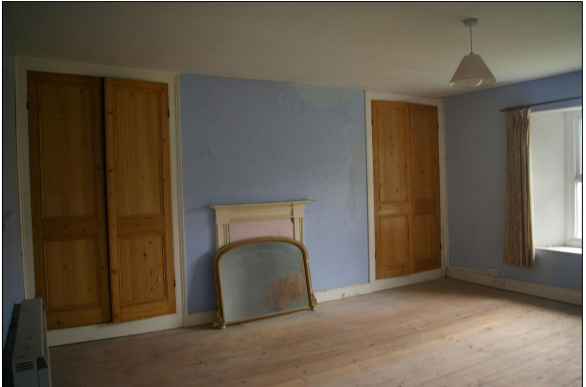
51. ROOM 15, IN THE EXTENSION, WITH GOOD FIREPLACE AND CUPBOARDS; FROM THE NORTH-WEST.
