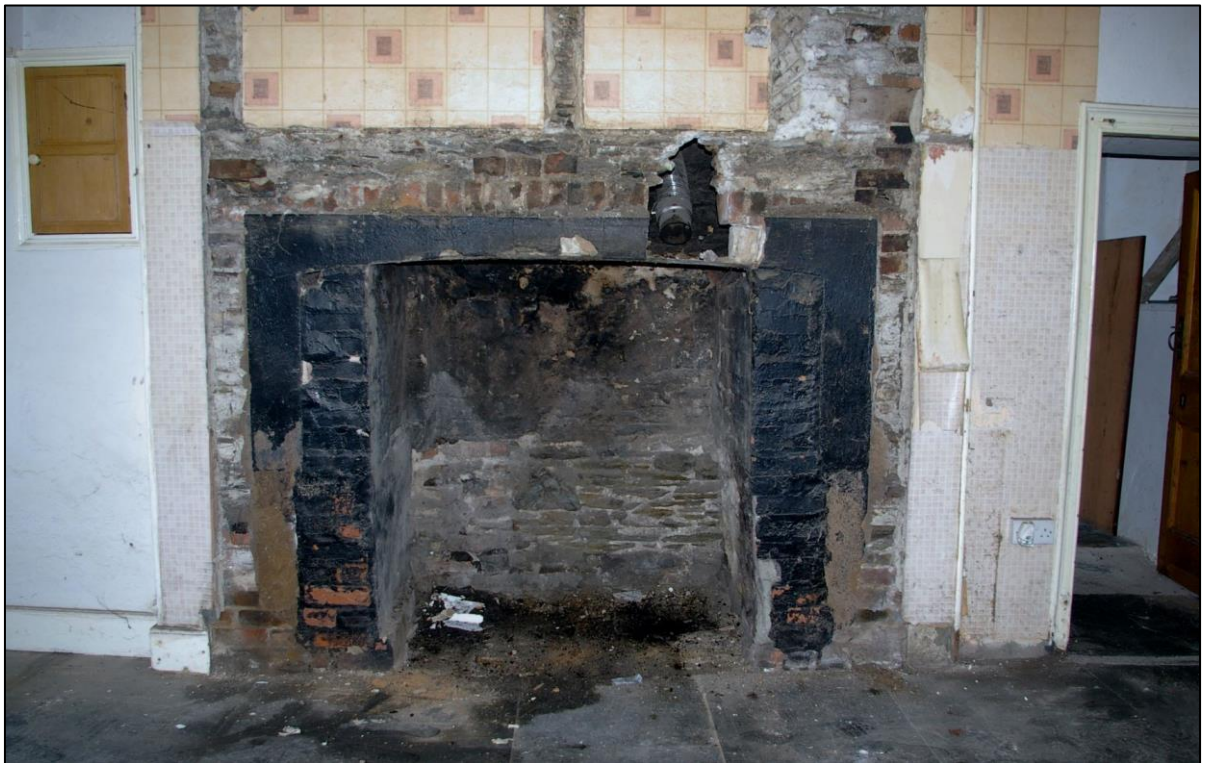
19. THE FIREPLACE IN R2A, FORCED INTO THE BACK OF AN EARLIER STACK; FROM THE EAST.
