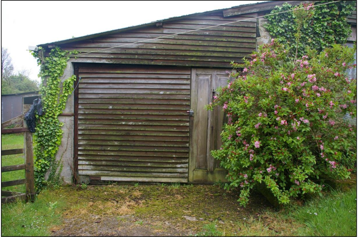
5. OB2, THE NORTH FRONT, SHOWING BOARDING; FORM THE NORTH.
