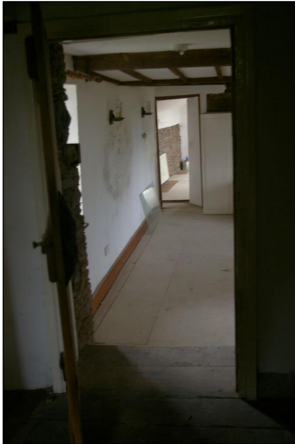
60. VIEW THROUGH THE DOORWAY INTO THE REAR SERVICE WING; FROM THE SOUTH.
