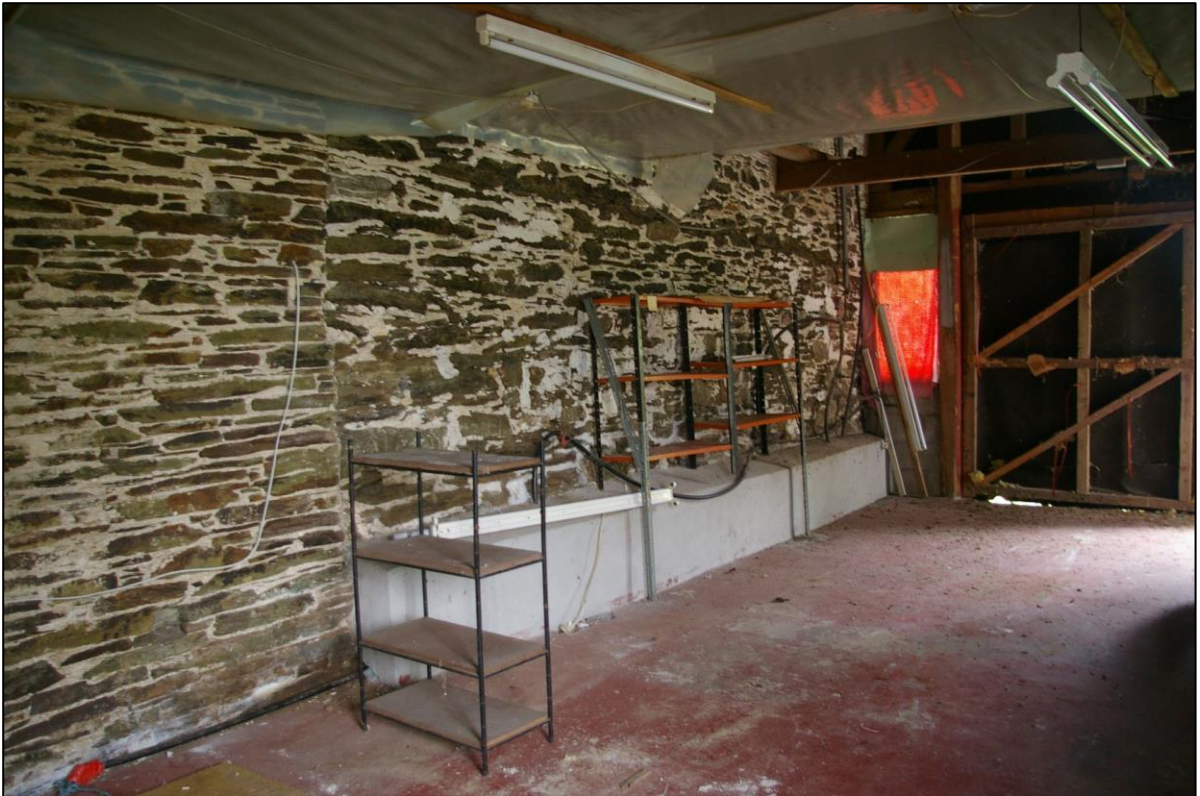
9. THE EAST WALL OF THE HOUSE, SHOWING THE BUILD LINE IN THE EAST WING; FROM THE SOUTH-EAST. FROM WITHIN OB1.
