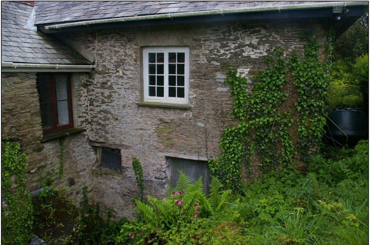
13. THE NORTH WALL OF THE WEST CROSS-WING; FROM THE NORTH-WEST.
