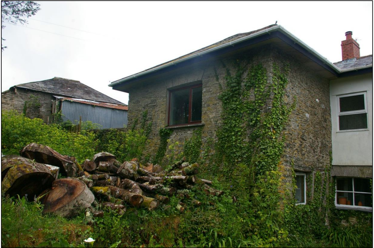
1. THE WEST WING AT TREVEDDA; FROM THE SOUTH-WEST.
