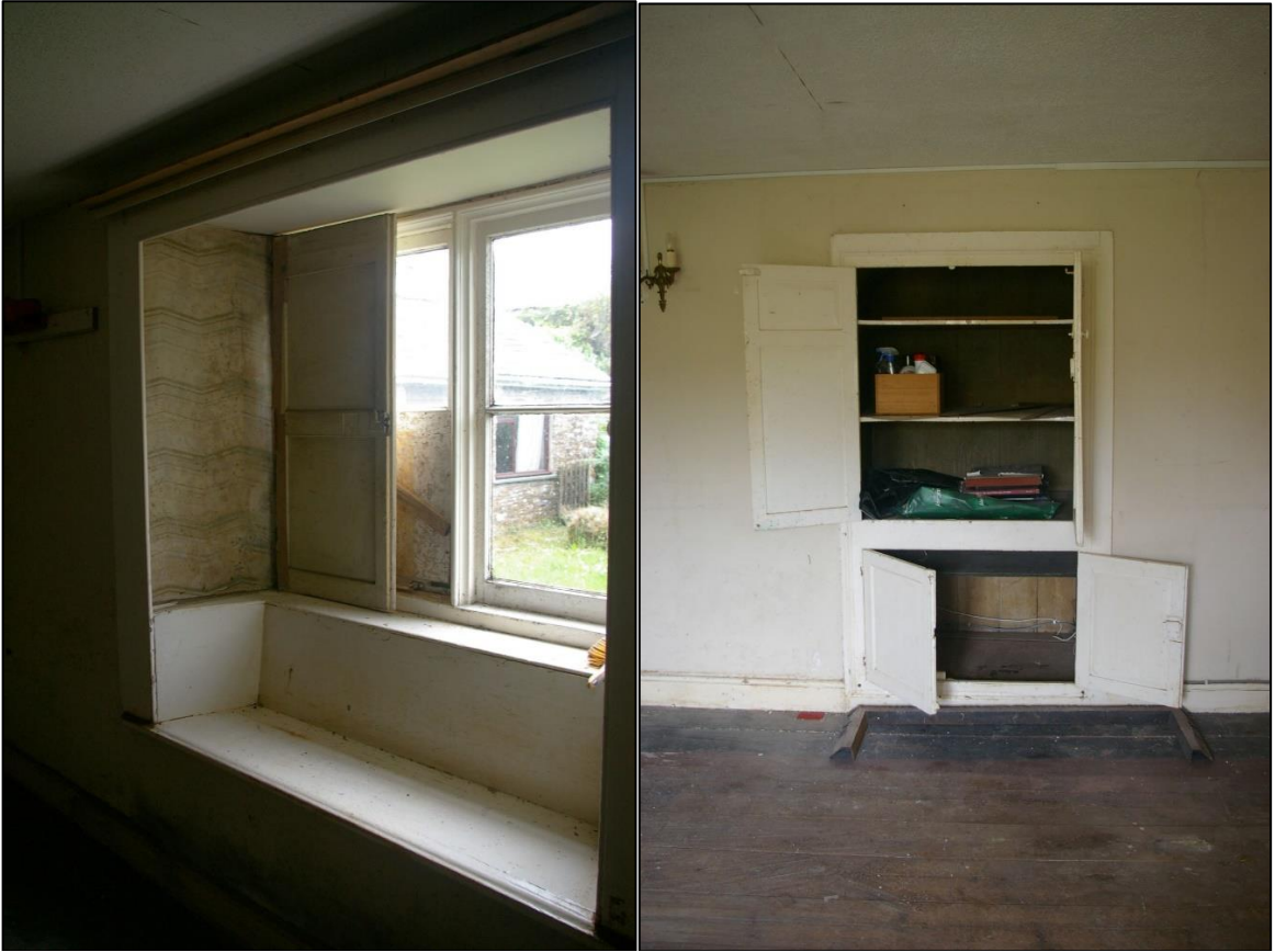
26. LEFT: THE WINDOW IN THE NORTH WALL OF R3, WITH GOOD PANELLED CASEMENT, WINDOW SEAT AND SHUTTERS; FROM THE EAST. 27. RIGHT: THE CUPBOARD IN R3, IN THE SOUTH WALL, IN A BLOCKED DOORWAY; FROM THE NORTH.
