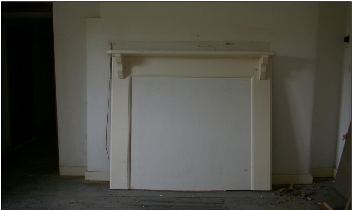
59. THE FIREPLACE SURROUND IN R19; FORM THE WEST.
