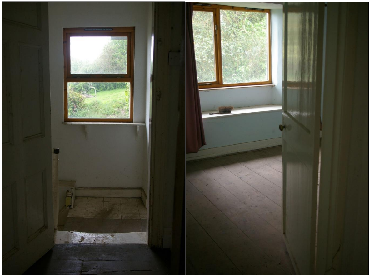
43. LEFT: ROOM 9, THE LANDING AT THE TOP OF THE WEST STAIRS; FROM THE NORTH.
