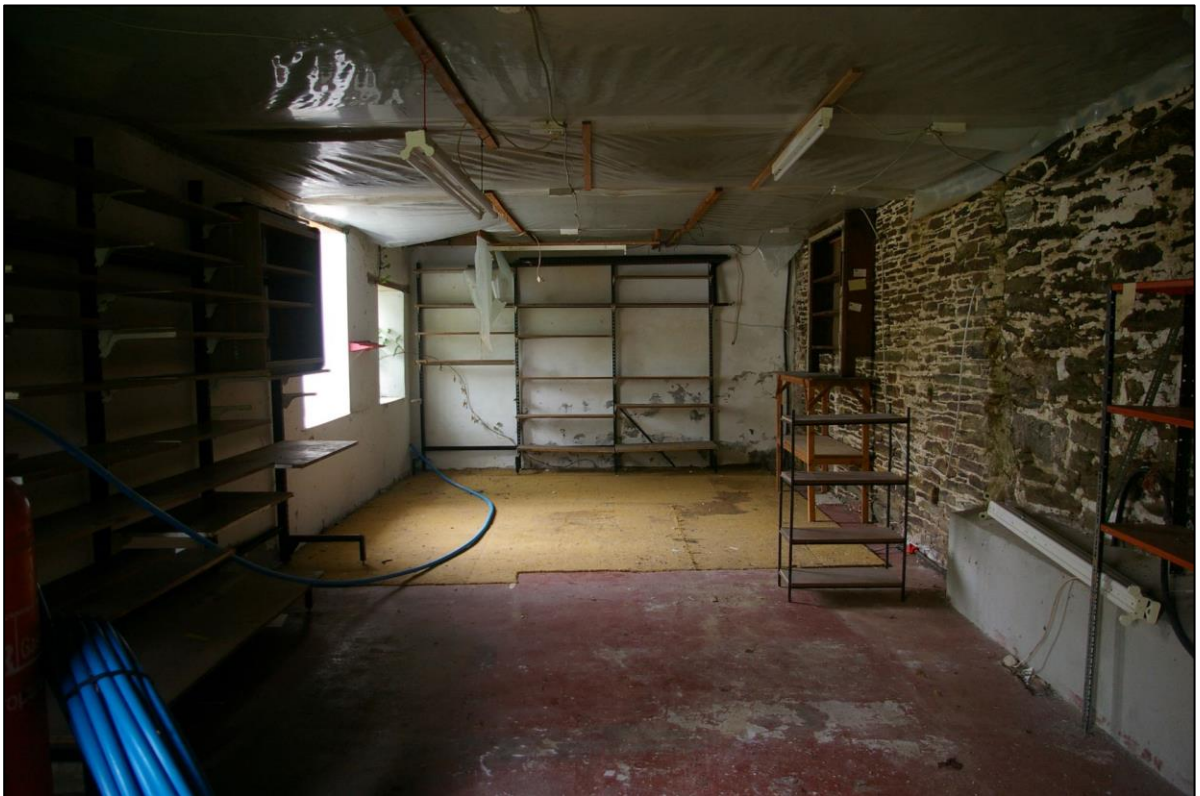
8. THE INTERIOR OF OB1; FROM THE NORTH.
