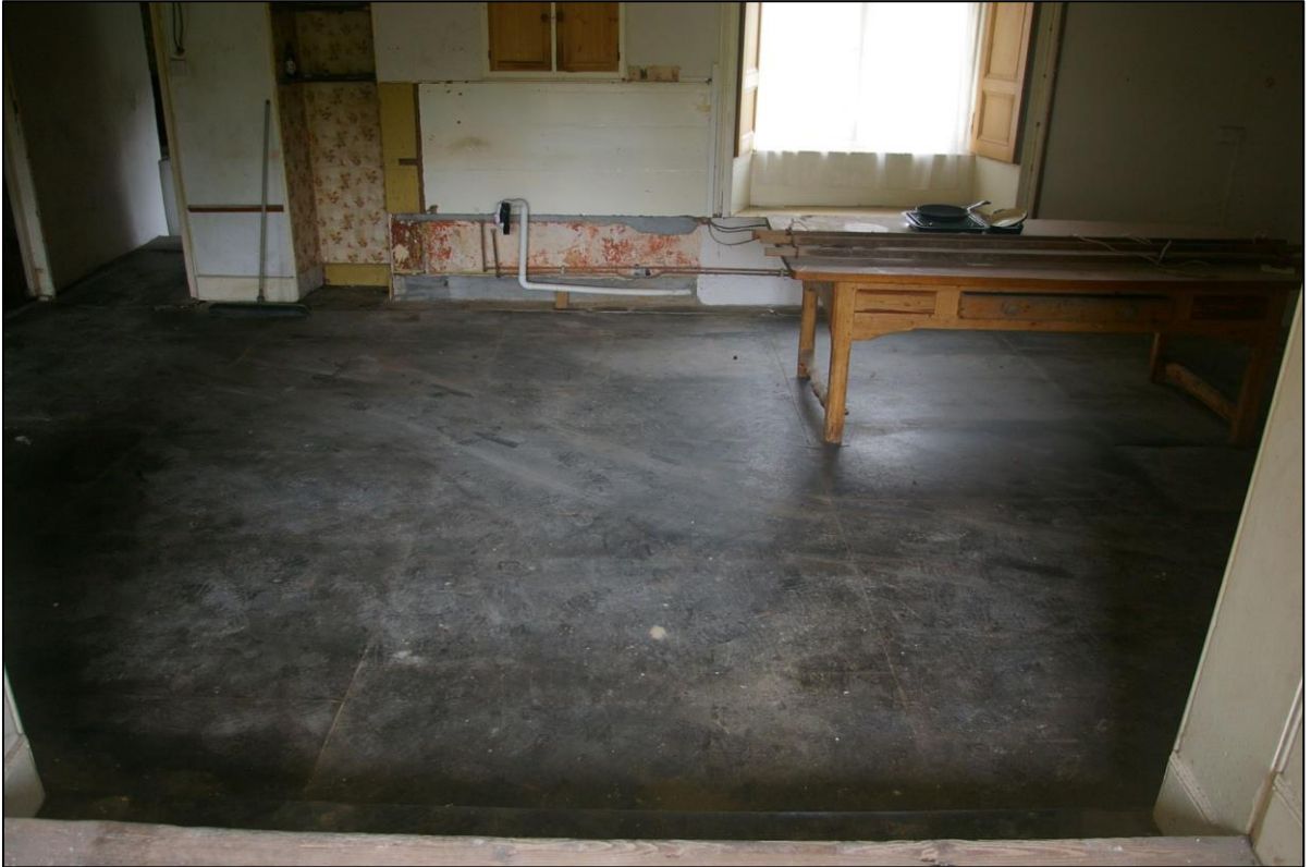
22. THE FLOOR OF R2A; FROM THE SOUTH.
