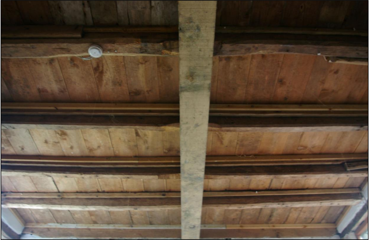
34. THE CEILING OF R5; FROM THE NORTH.
