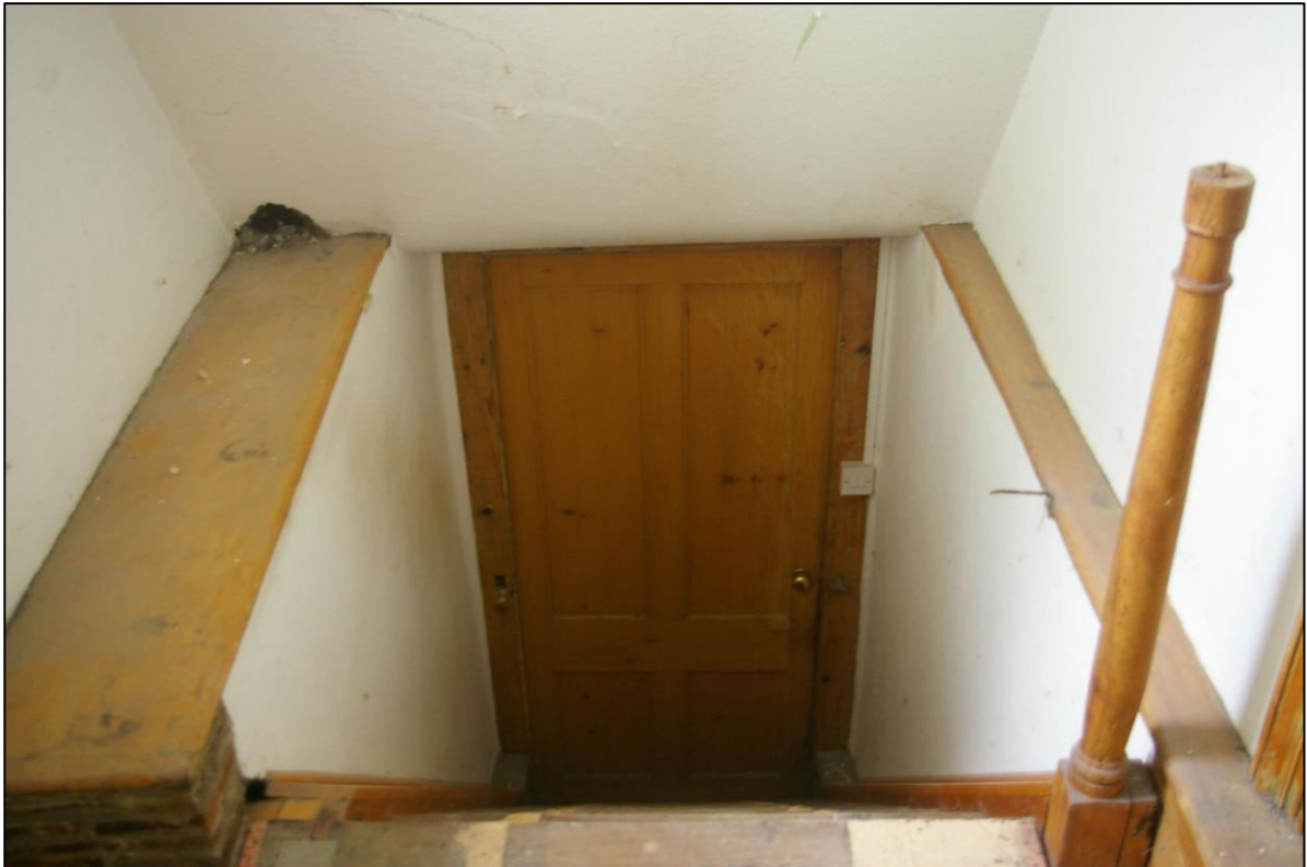
49. VIEW BACK DOWN THE EAST STAIRS, R14; FROM THE EAST.
