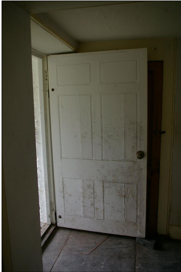
15. THE FRONT DOOR, BETWEEN R1 AND R2A; FROM THE EAST.
