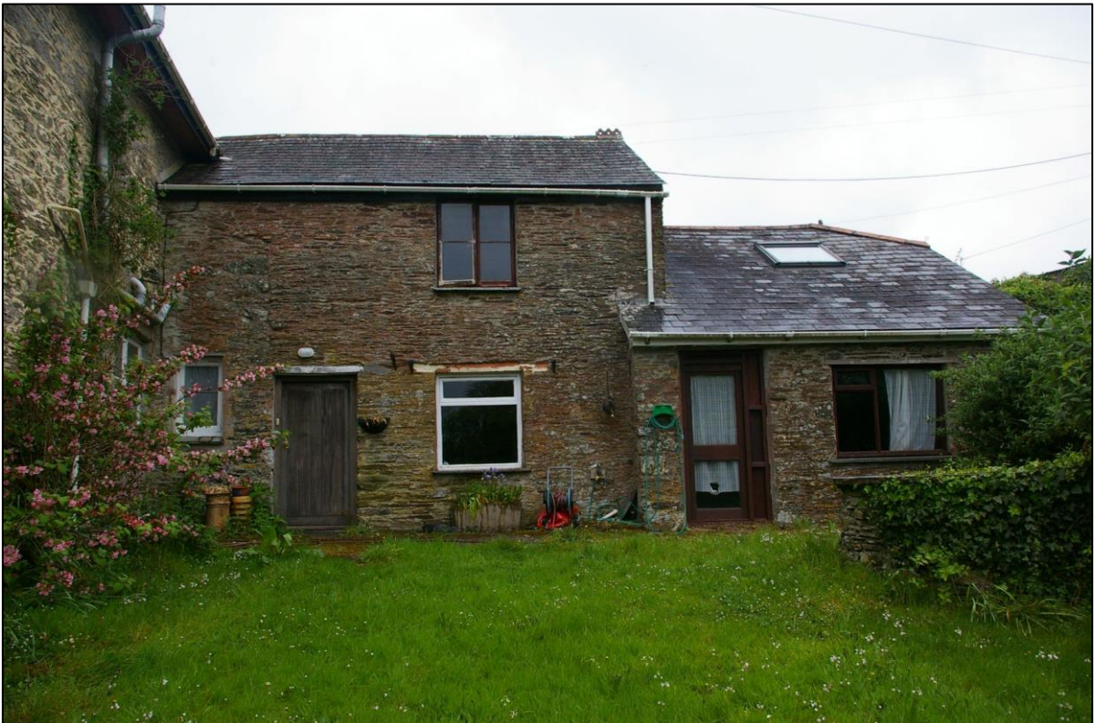
10. THE EAST WALL OF THE REAR SERVICE WING; FROM THE EAST.
