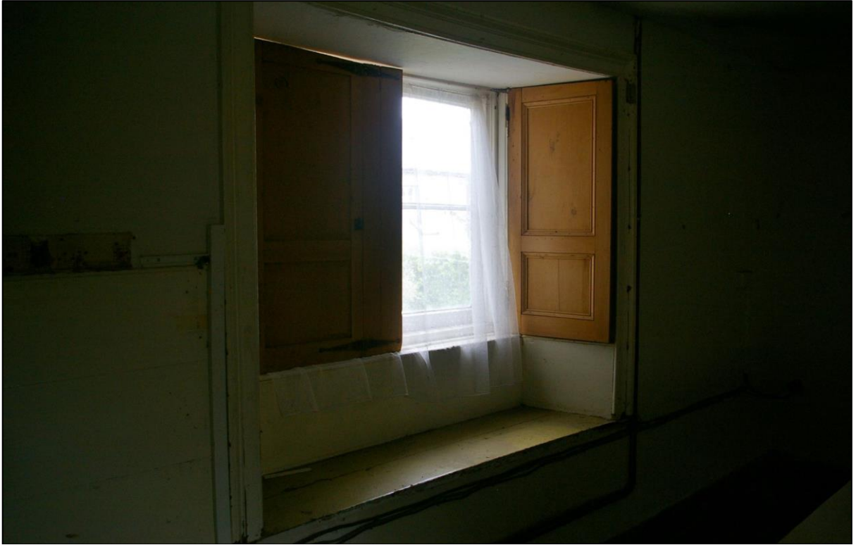
18. THE WINDOW WITH GOOD PANELLED CASEMENT AND WINDOW SEAT AND GOOD WINDOW FRAME, IN R2A; FROM THE SOUTH-WEST.
