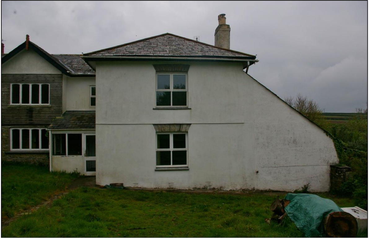
3. THE EAST WING AT TREVEDDA; FROM THE SOUTH.
