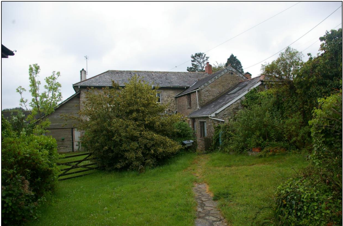
12. THE FARMHOUSE FROM THE REAR, NORTH.
