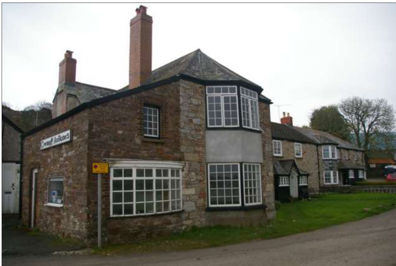
2. THE NORTH AND EAST ELEVATIONS OF THE COTTAGE; VIEWED FROM THE NORTH-EAST.
