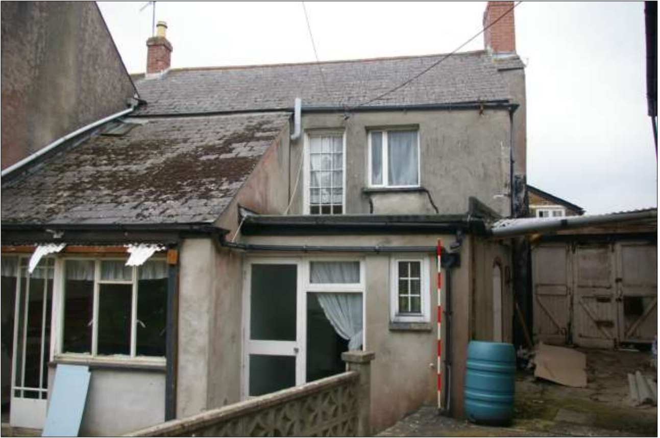
5. AS ABOVE; VIEWED FROM THE SOUTH-SOUTH-EAST (SCALE 2M).
