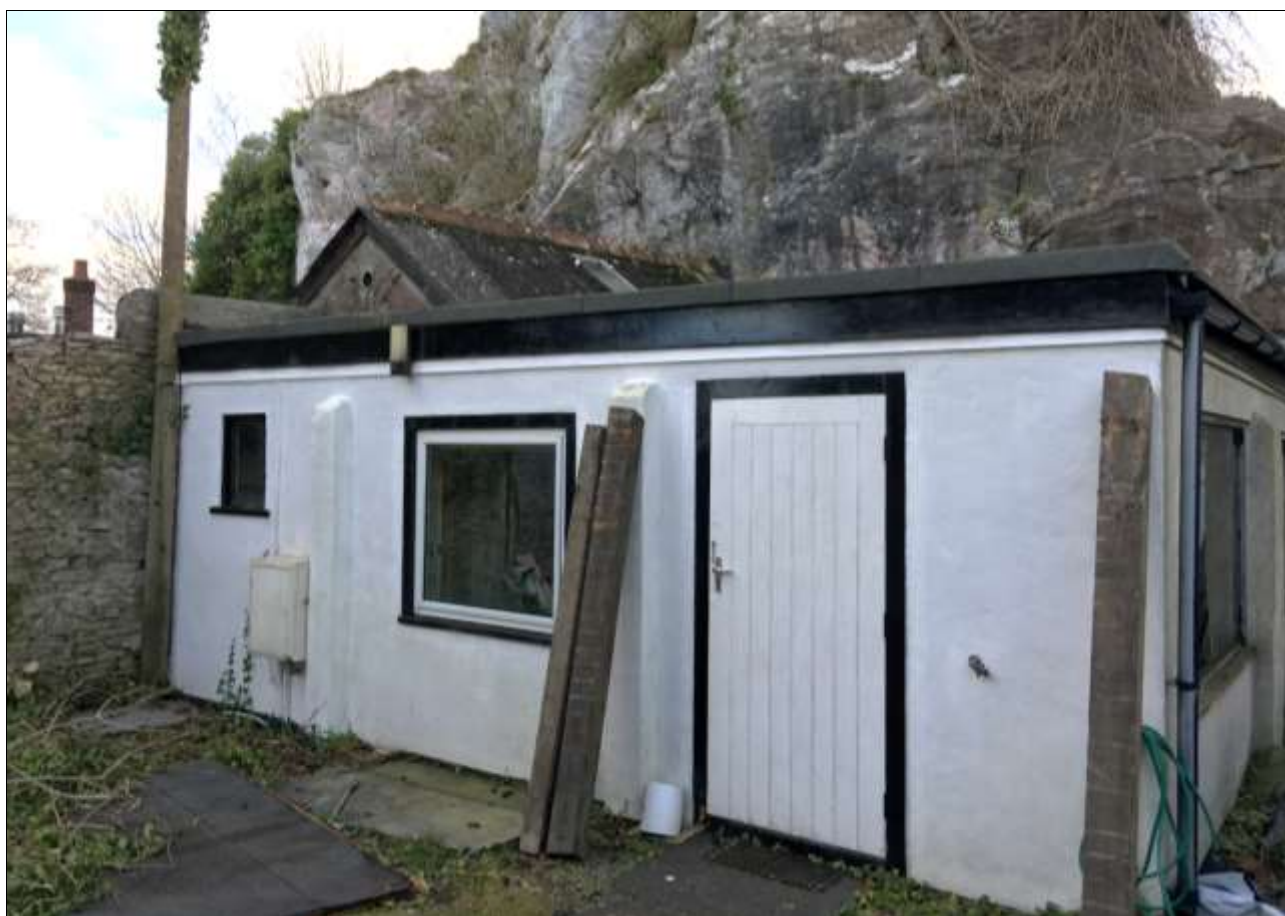
9. THE WORKSHOP IN MORE DETAIL, SHOWING IT ENVELOPING EARLIER SHED BEHIND; VIEWED FROM THE NORTH-WEST.
