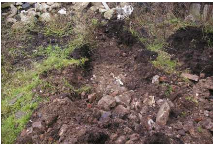
FIGURE 4: MADE-GROUND ON EAST SIDE OF SITE BELOW SITE FORMATION LEVEL IN TEST PIT, MID-EXCAVATION; VIEWED FROM THE SOUTH-WEST (NO SCALE).
