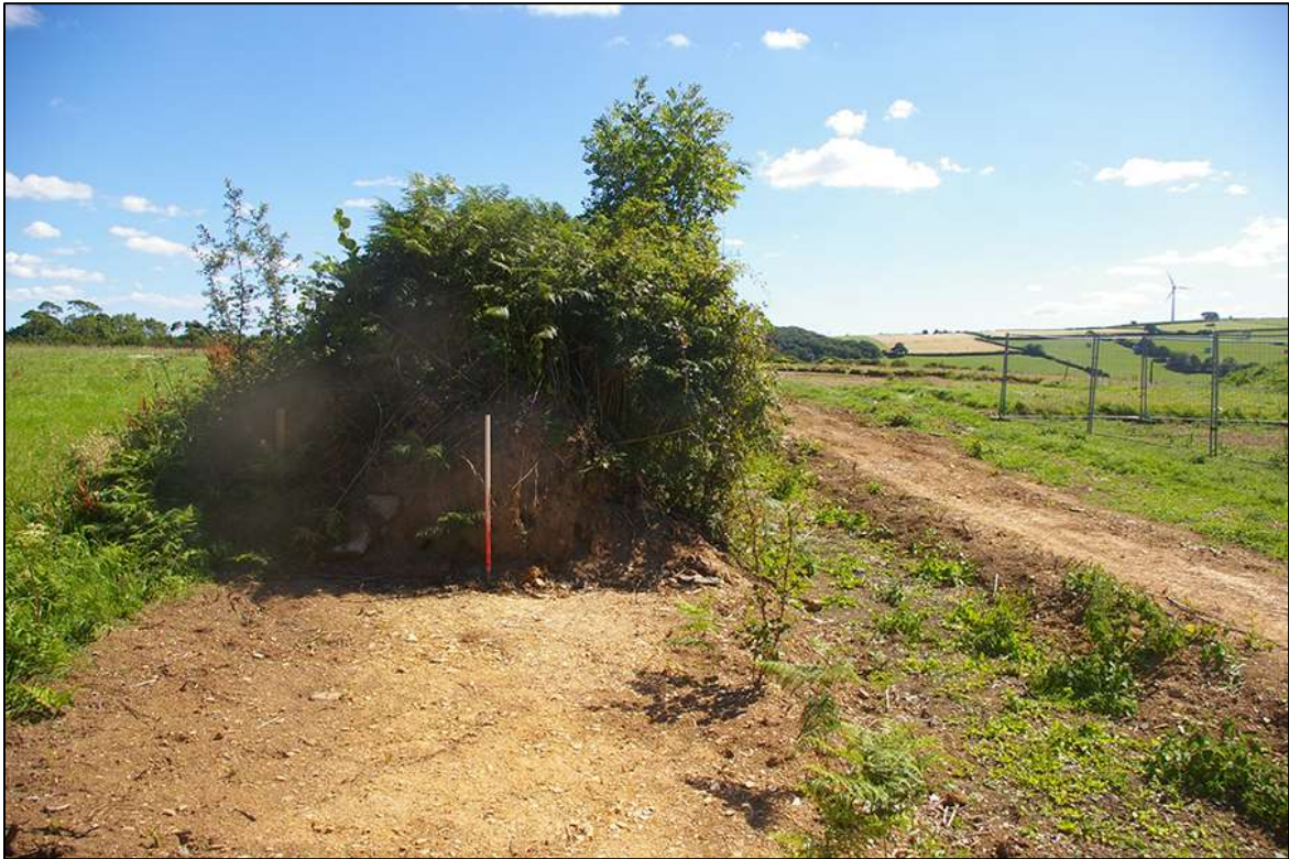
105. NORTH FACING PROFILE OF EAST HEDGEBANK BOUNDARY TO F4; VIEWED FROM THE WEST (1M SCALE).
