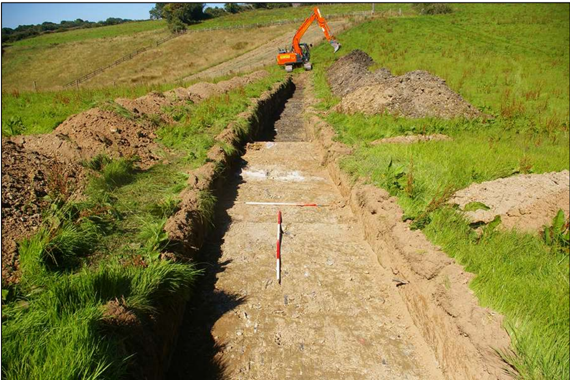
4. TRENCH 01, POST-EXCAVATION; VIEWED FROM THE EAST (1M & 2M SCALES).
