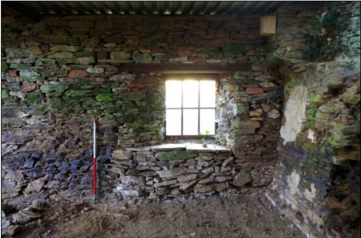
FIGURE 9: RE-BUILT WINDOW OPENING, VIEWED FROM THE NORTH-WEST (1M SCALE).
