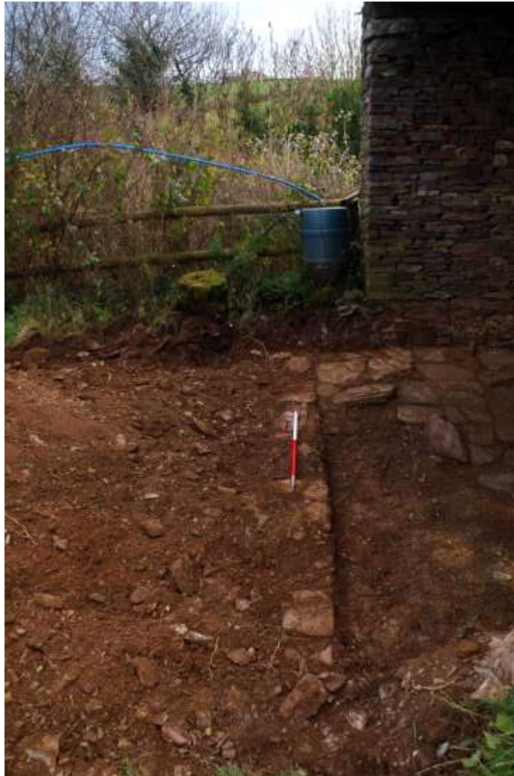
19. SURVIVING FOOTINGS OF THE DEMOLISHED NORTH-EAST ELEVATION, VIEWED FROM THE NORTH-WEST (1M SCALE).
