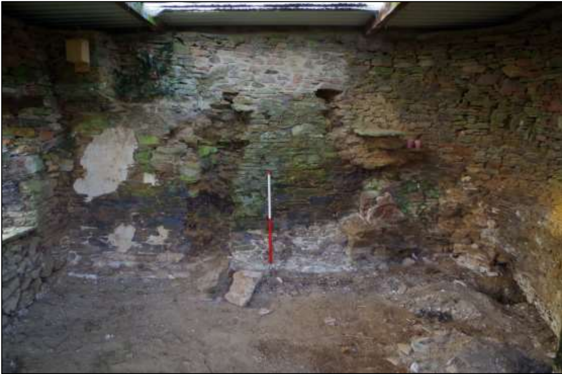
5. SCAR OF FIREPLACE WITH RE-BUILD ABOVE, VIEWED FROM THE NORTH-EAST (1M SCALE).
