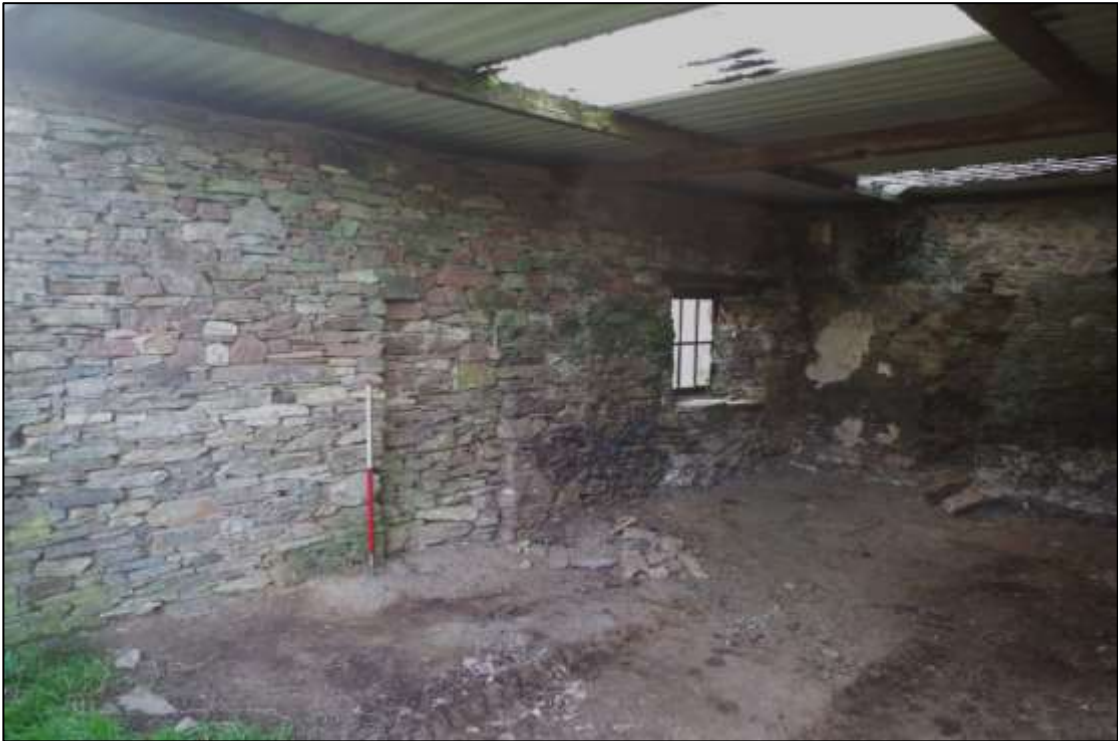
13. INTERNAL SPACE, VIEWED FROM THE NORTH (1M SCALE).
