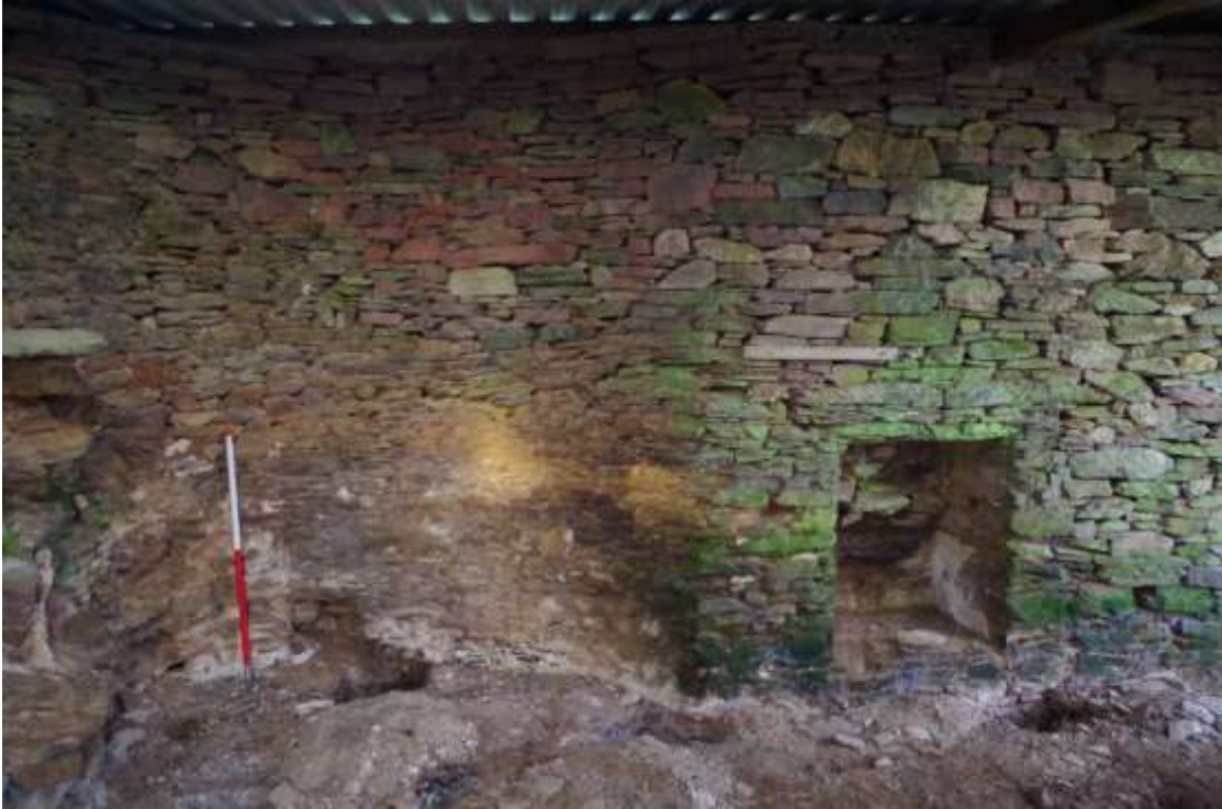
9. BLOCKED OPENING AND (?)STAIR, VIEWED FROM THE SOUTH-EAST (1M SCALE).
