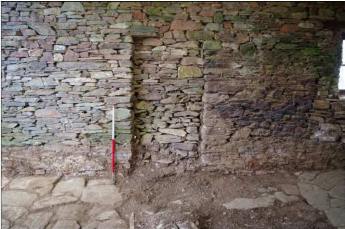
12. BLOCKED CENTRAL DOOR FOLLOWING EXCAVATION, VIEWED FROM THE NORTH-WEST (1M SCALE).
