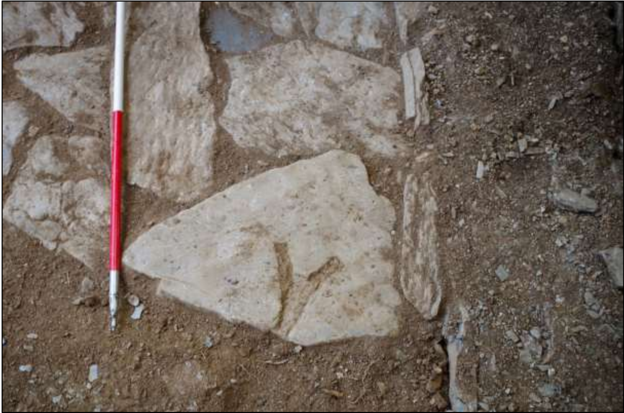
FIGURE 12: RE-USED STONE IN PAVED FLOOR TO THE EAST, THE INCISED 'Y' COULD RELATE TO A FORMER USE AS PART OF A CHEESE PRESS, VIEWED FROM THE NORTH-WEST (1M SCALE).
