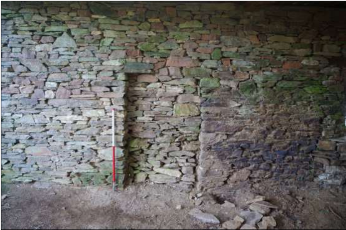
11. BLOCKED CENTRAL DOOR, VIEWED FROM THE NORTH-WEST (1M SCALE).
