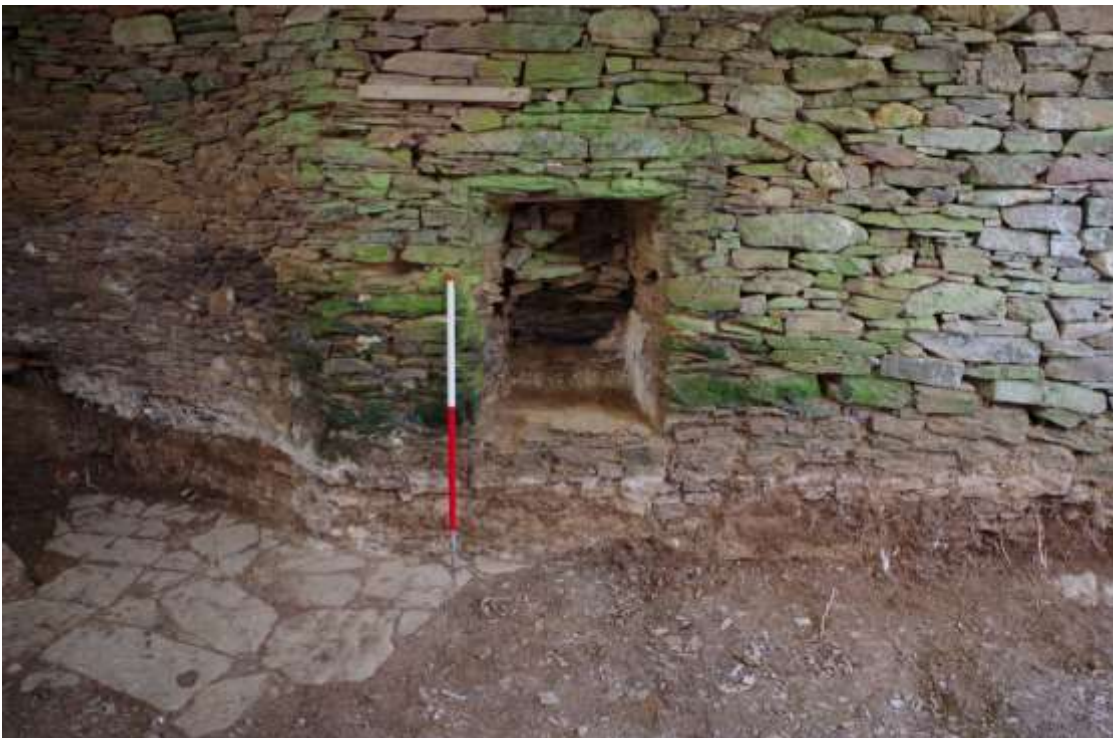
10. AS ABOVE, POST-EXCAVATION, VIEWED FROM THE SOUTH-EAST (1M SCALE).
