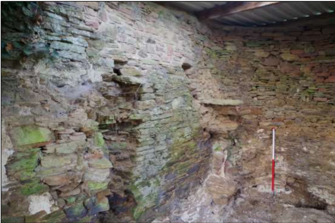
8. DETAIL OF STACK, VIEWED FROM THE EAST (1M SCALE).
