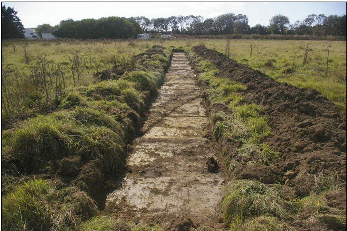
4. TRENCH 3, MODERN TRENCH LINE [305] IN FOREGROUND; VIEWED FROM THE NORTH-EAST (2M SCALE).
