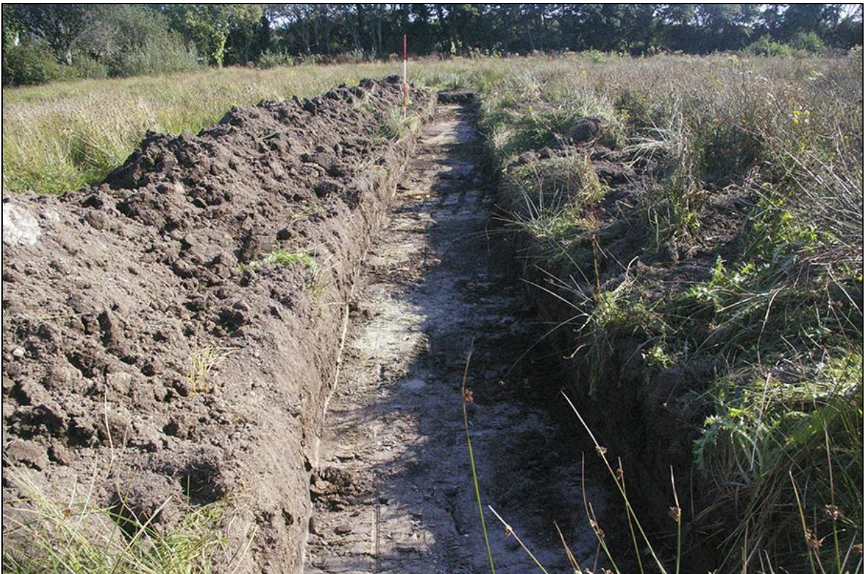
14. TRENCH 5; VIEWED FROM THE NORTH-WEST (2M SCALE).
