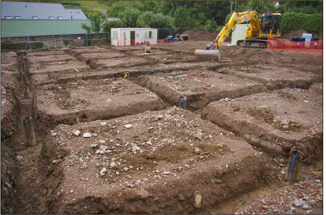
FIGURE 2: AREA 01, POST-EXCAVATION; VIEWED FROM THE NORTH-EAST (1M & 2M SCALES).
