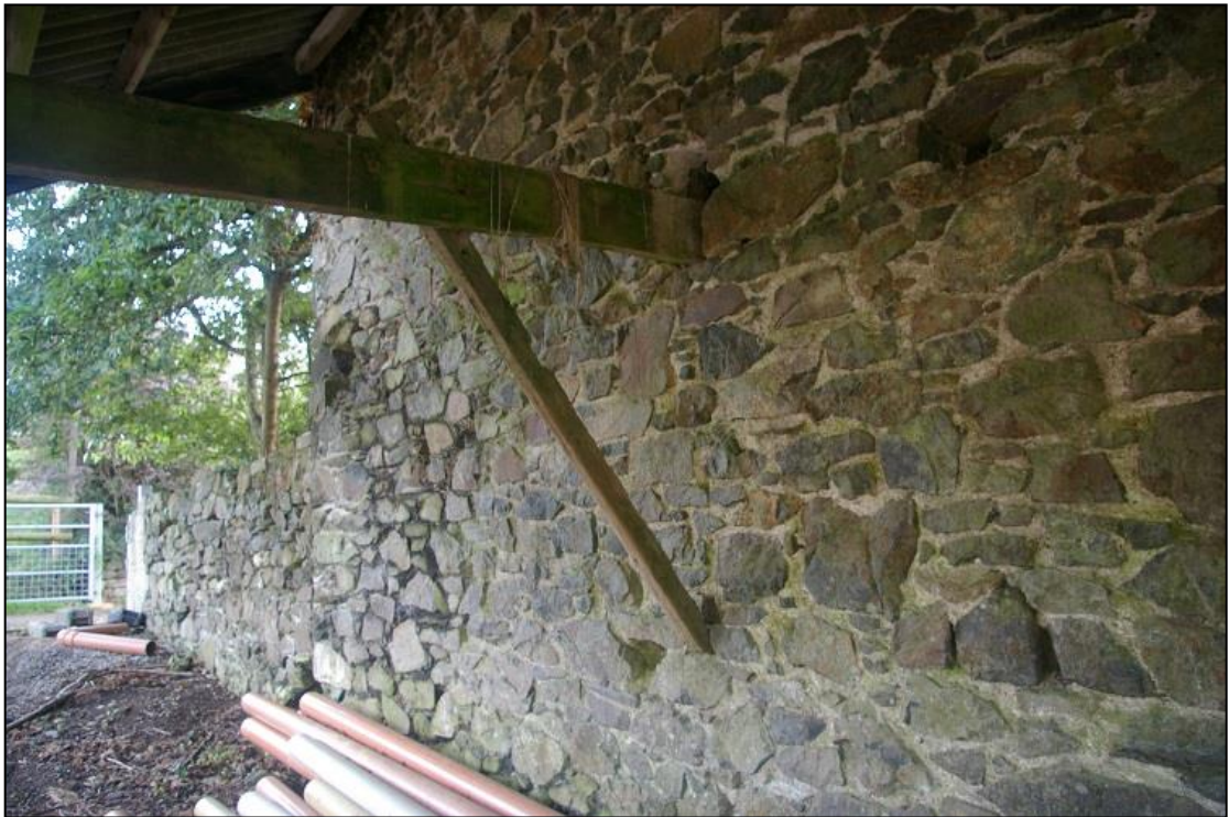
16. BRACING TIMBER FOR HAYRICKS IN B1B.
