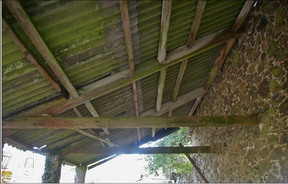
15. THE ROOF OVER B1B; FROM THE WEST.
