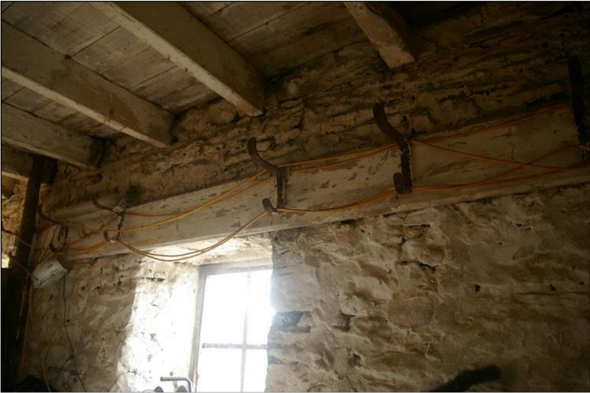
9. CHAMFERED PLANK FITTINGS WITH SADDLE AND HARNESS TREES ON THE SOUTH WALL OF THE STABLE.
