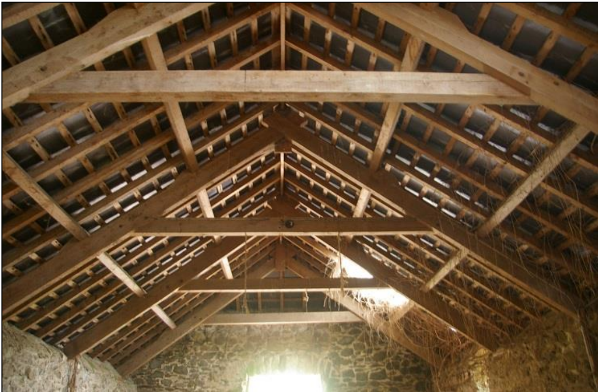
14. THE ROOF OVER B1A.
