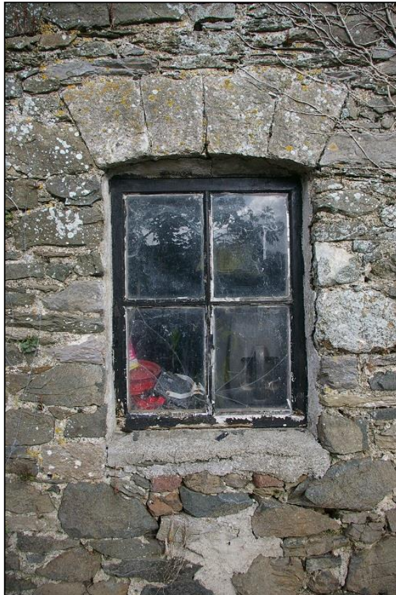
4. THE WESTERN WINDOW ON THE SOUTH ELEVATION; SHOWING ARCHITECTURAL DETAILS.
