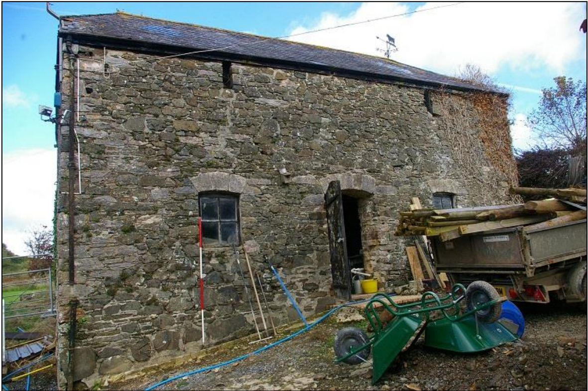
FIGURE 10: THE FRONT ELEVATION OF THE STABLES, B1A, WITH 2M SCALE.
