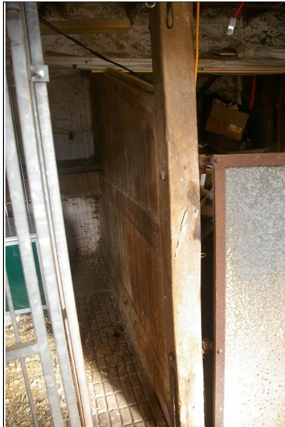
8. DETAIL OF THE BOARDED STALL PARTITIONS.
