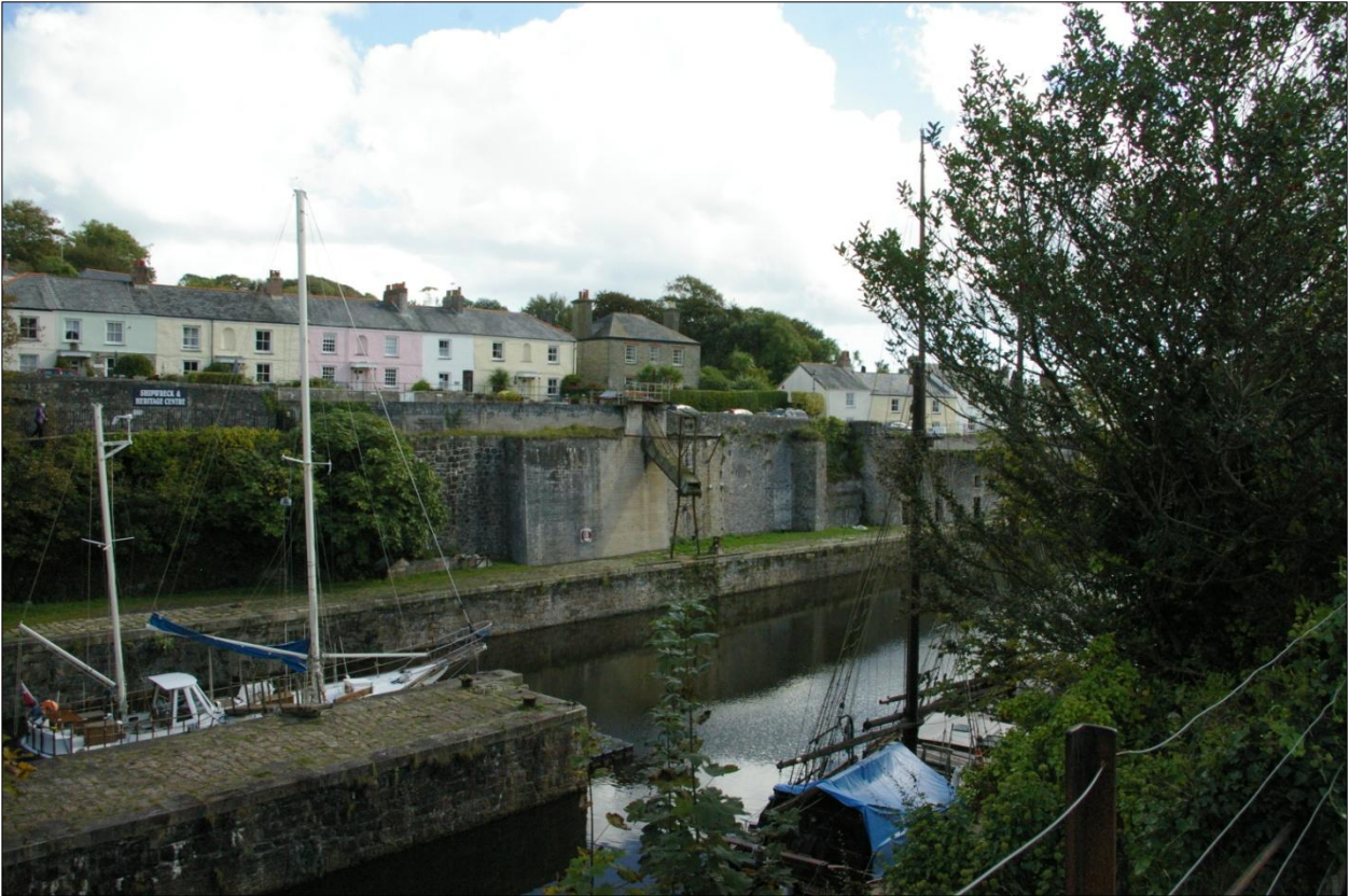
VIEW OF THE CHARLESTOWN HARBOUR INNER BASIN WALLS FROM THE HARBOUR APPROACH OF THE TOWN; VIEWED FROM THE NORTH-WEST.
