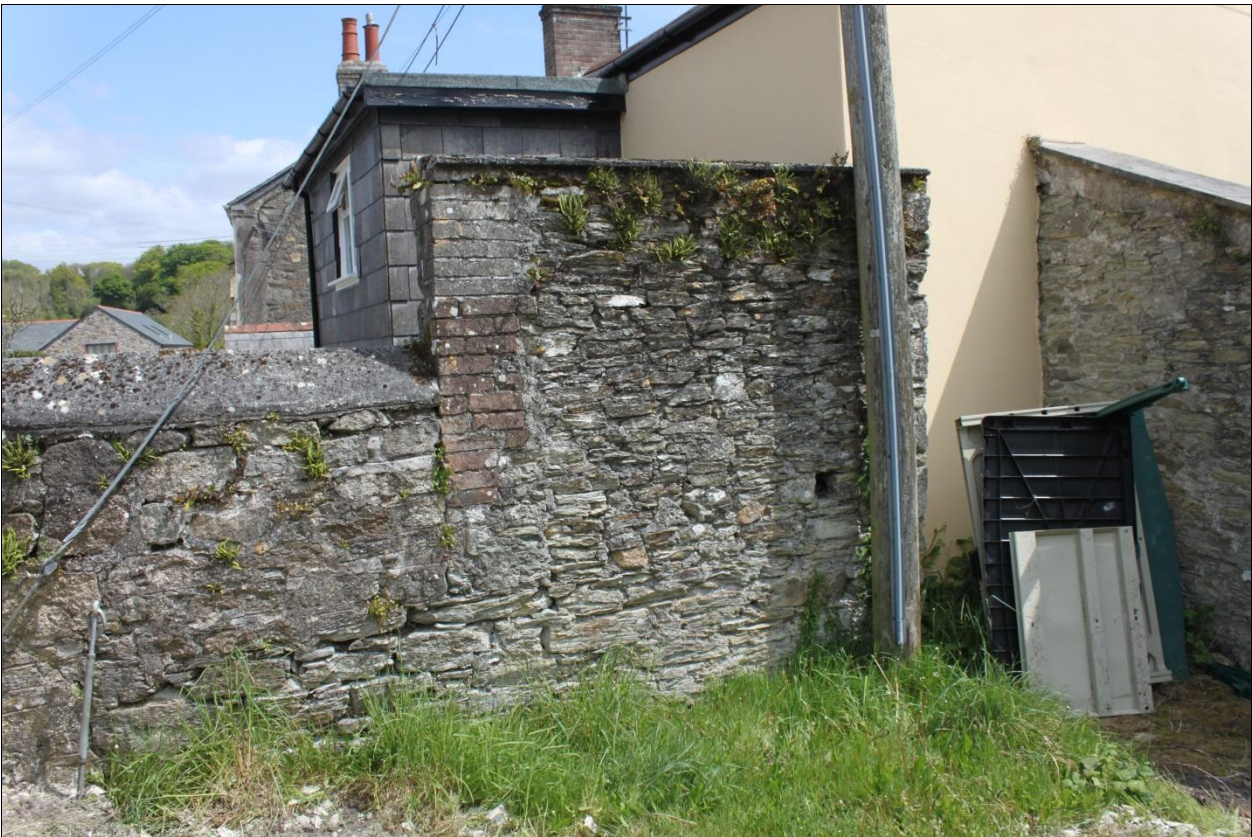
PHASING EVIDENT IN THE EASTERN BOUNDARY OF THE FORMER YARD, VIEWED FROM THE WEST.
