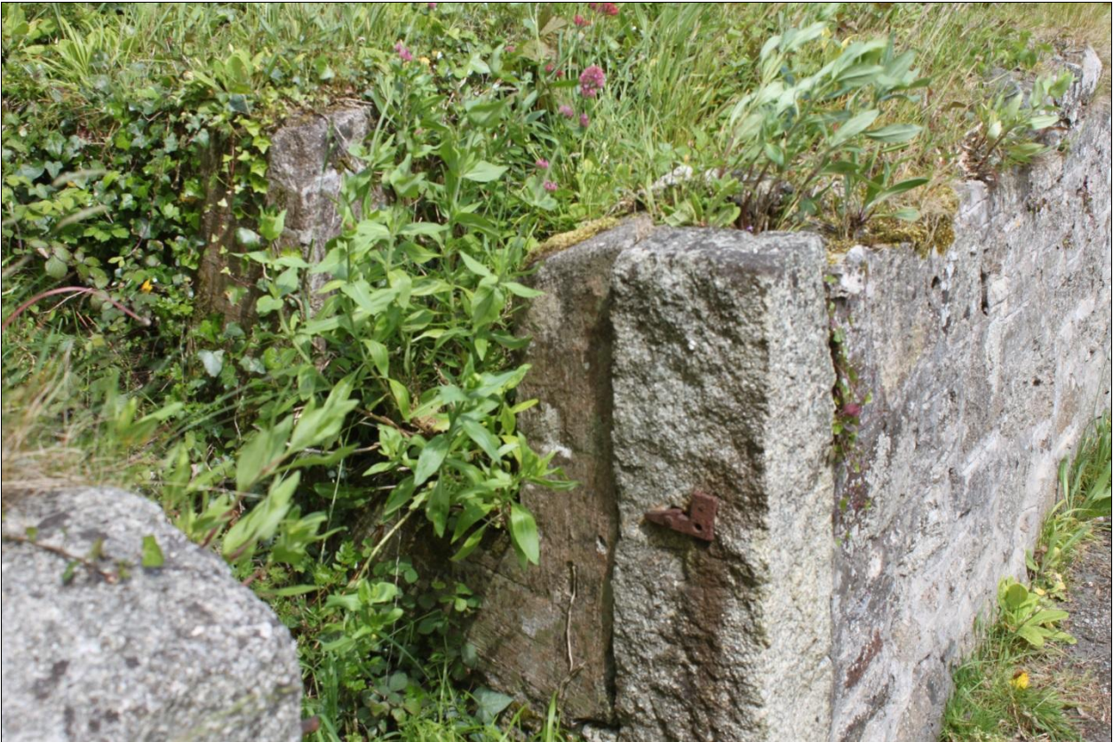
SHOT SHOWING THE REMAINS OF CAST IRON GATE FITTINGS NOTED ON EACH SET OF GRANITE GATE POSTS, AND THE STEP WHICH LED UP TO THE EASTERN GARDEN FROM EACH ACCESS POINT, VIEWED FROM THE WEST-SOUTH-WEST.
