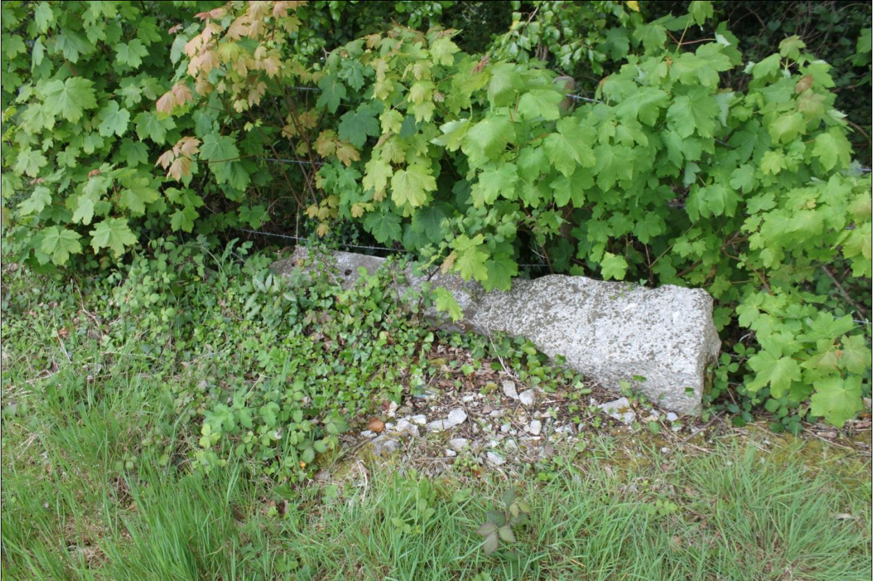
SHOT OF SURVIVING PORTION OF THE GRANITE COPING TO THE WESTERN BOUNDARY OF THE SOUTHERN ORE YARD, VIEWED FROM THE EAST.
