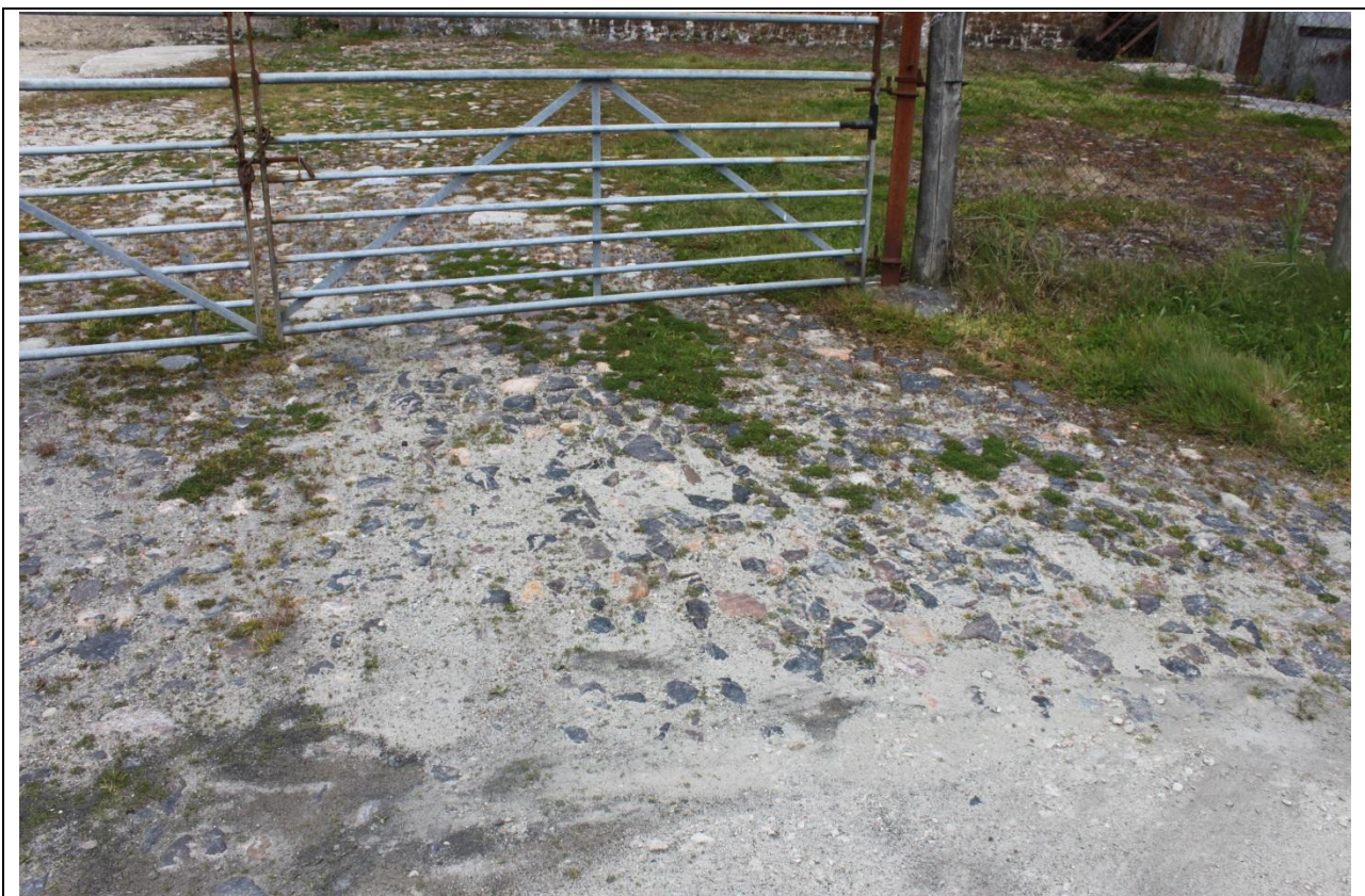
SHOT OF THE REMNANT OF THE COBBLED ORE FLOOR BETWEEN THE TWO YARDS, VIEWED FROM THE SOUTH.
