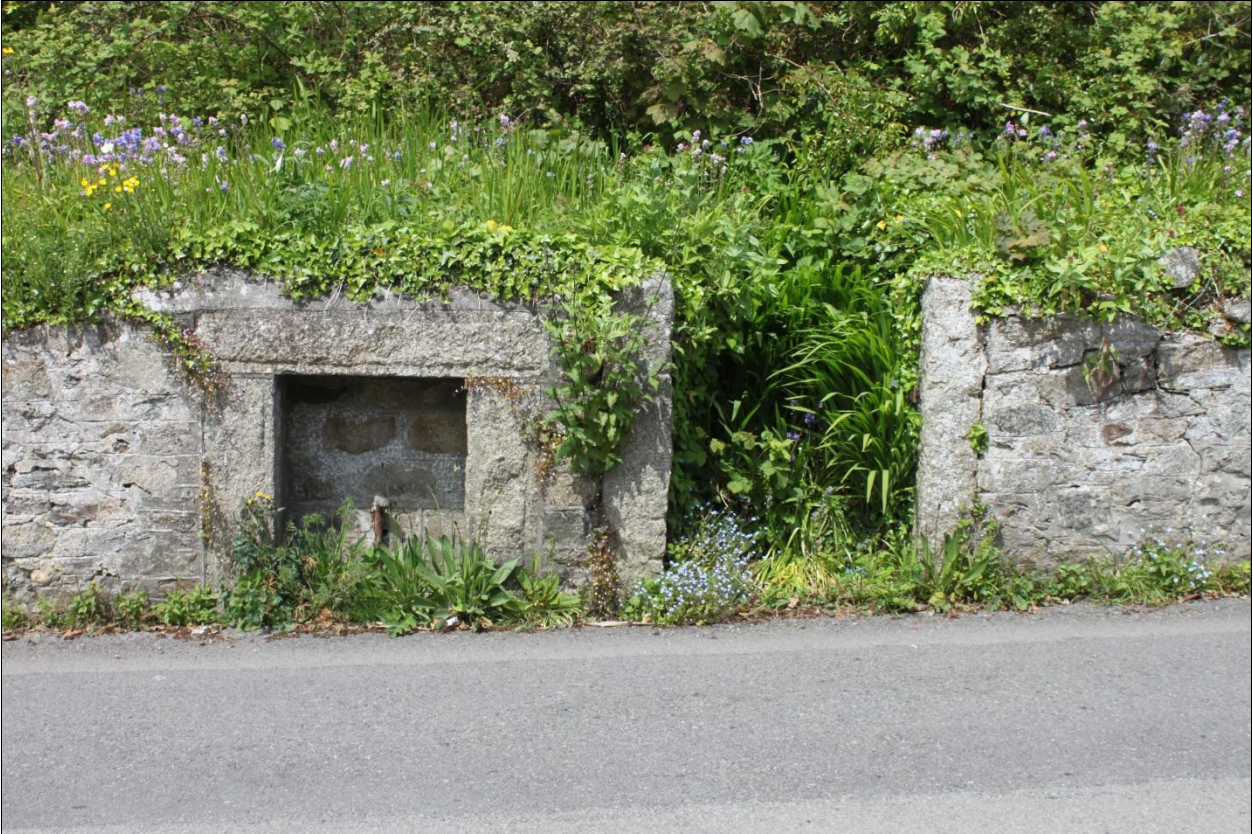
SHOT OF THE WATER POINT AND ADJACENT GATE OPENING, VIEWED FROM THE SOUTH.
