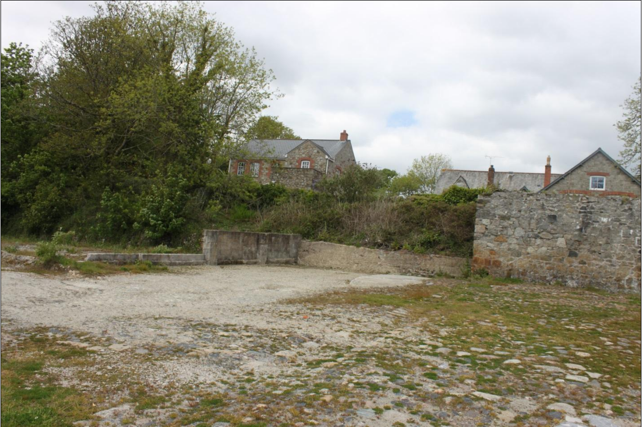
SHOT OF THE GENERALLY BETTER CONDITION, THOUGH WORN NATURE OF THE NORTHERN ORE FLOOR, VIEWED FROM THE SOUTH.
