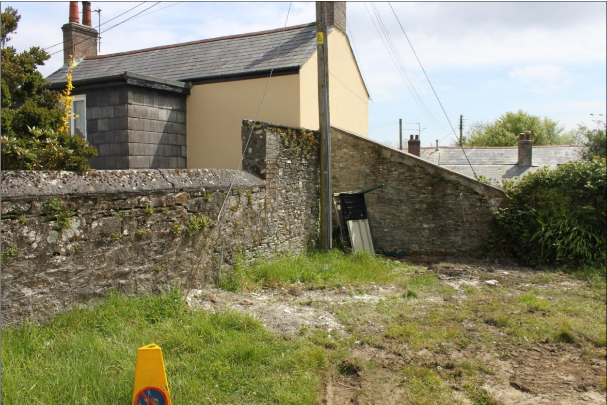
VIEW OF THE SOUTH-EASTERN CORNER OF THE FORMER YARD, VIEWED FROM THE NORTH-WEST.
