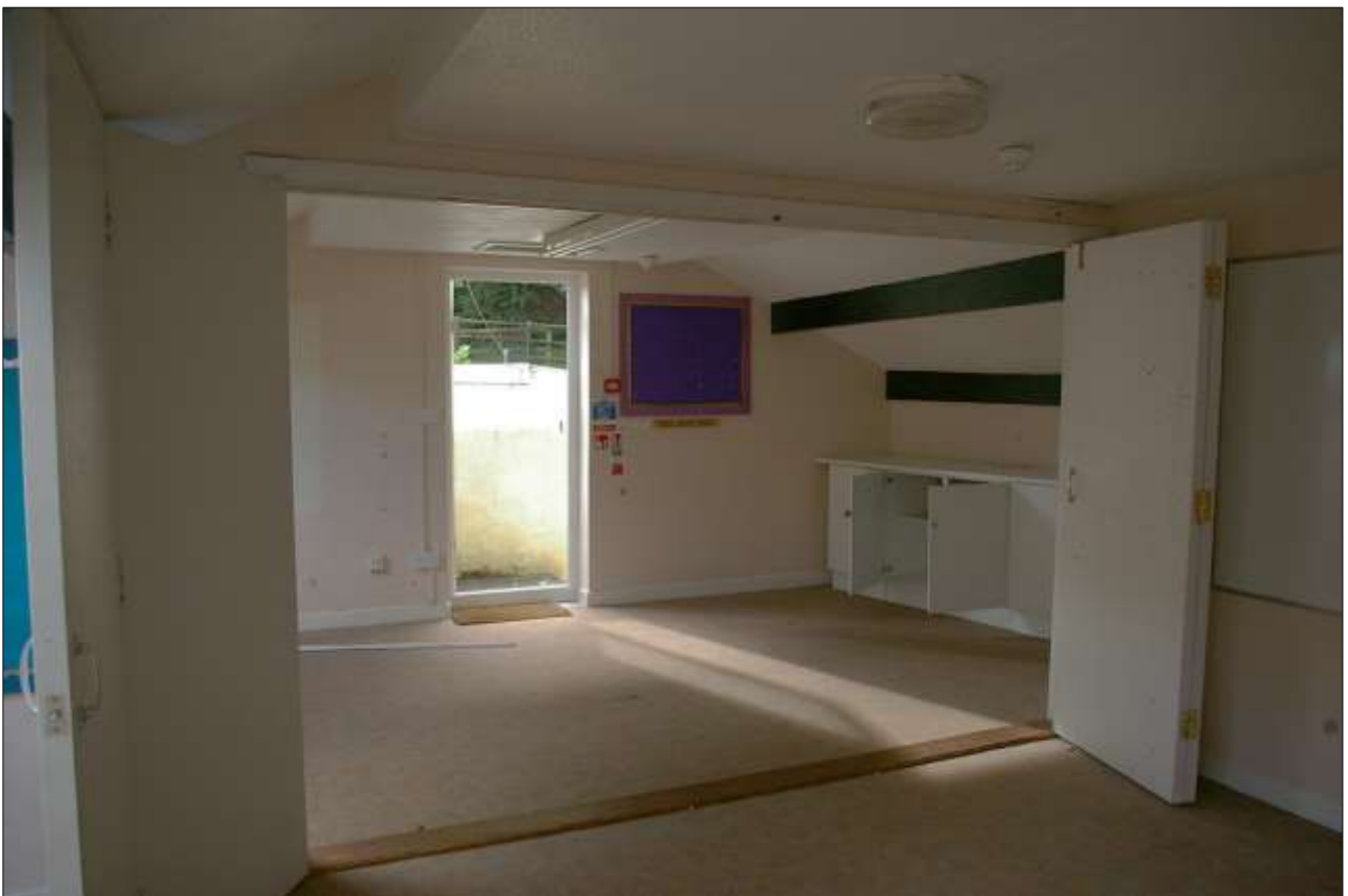
38. THE LOFT IN BLOCK 4B; VIEWED FROM THE NORTH-WEST
