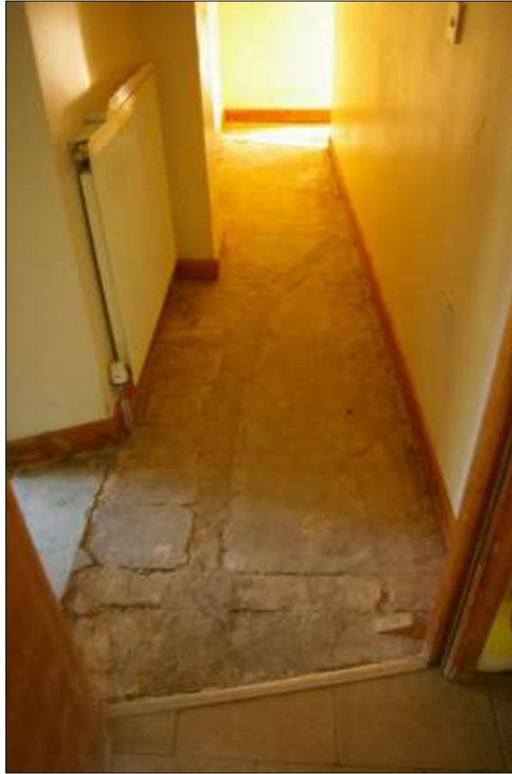
FIGURE 23: REMAINS OF A FLOOR OF STONE FLAGS IN BLOCK 1A; VIEWED FROM THE SOUTH.
