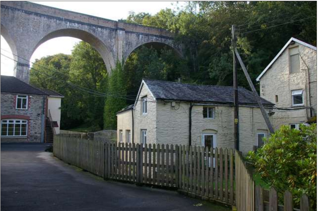
31. THE SETTING OF BLOCK 4 WITH THE VIADUCT BEHIND; VIEWED FROM THE WNW.
