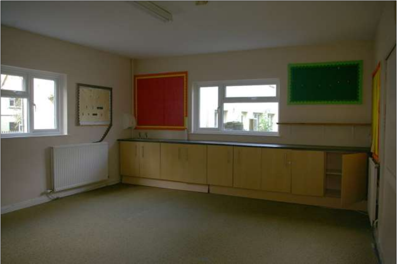
21. THE INTERIOR OF ONE OF THE SCIENCE CLASSROOMS IN BLOCK 2; VIEWED FROM THE ENE.
