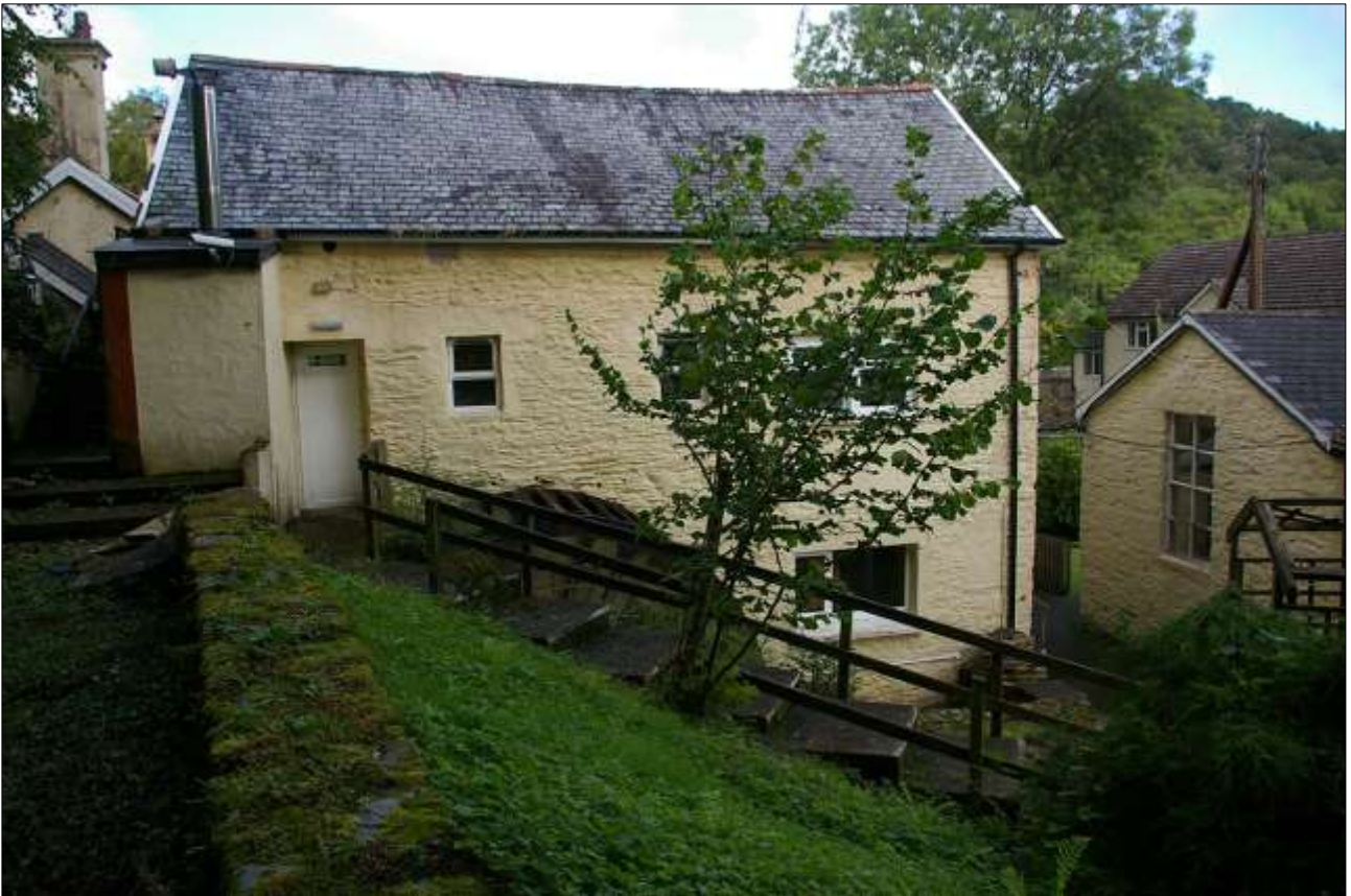
53. BLOCK 6, TERRACED INTO THE BANK WITH THE LEAT IN THE FOREGROUND; VIEWED FROM THE EAST.
