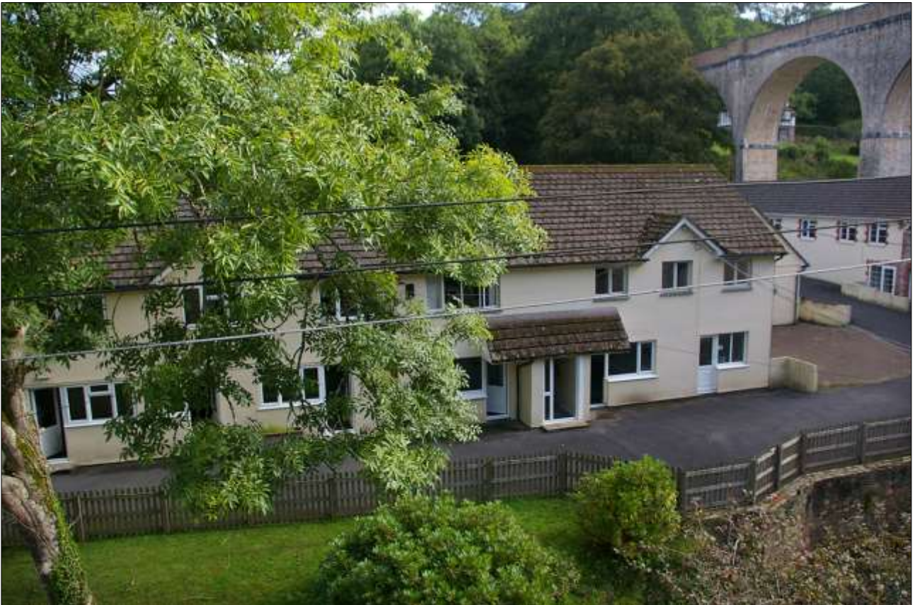
24. BLOCK 3 FROM ABOVE; VIEWED FROM THE SOUTH-WEST.
