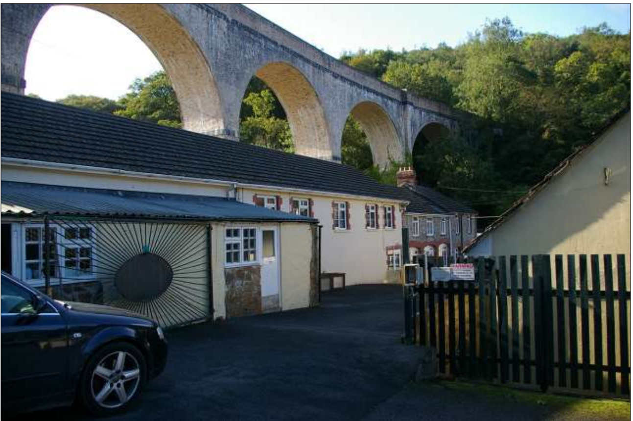
8. BLOCK 1 WITH THE VIADUCT BEHIND; VIEWED FROM THE NORTH-WEST.
