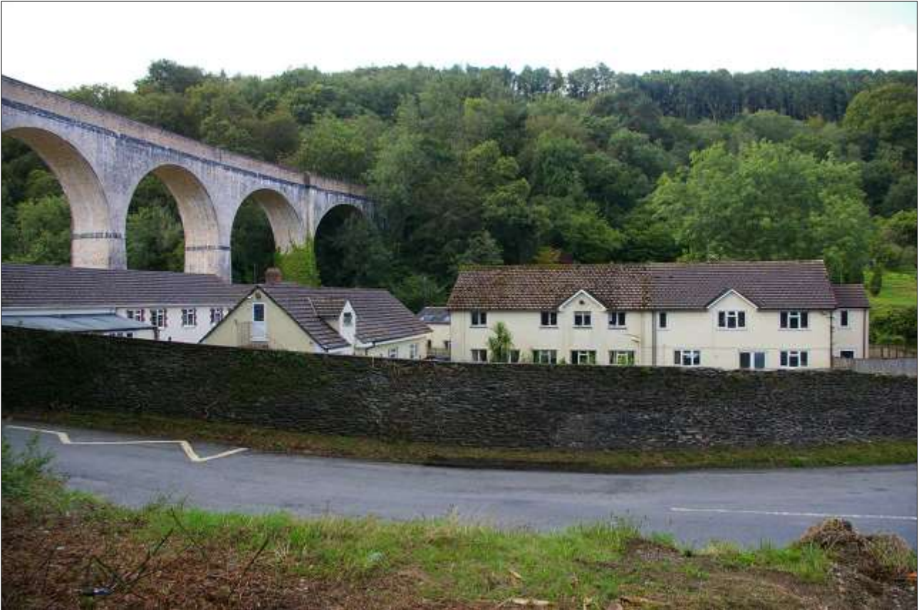
3. VALLEY VIEW OF THE SITE AND THE VIADUCT; VIEWED FROM THE NNW.
