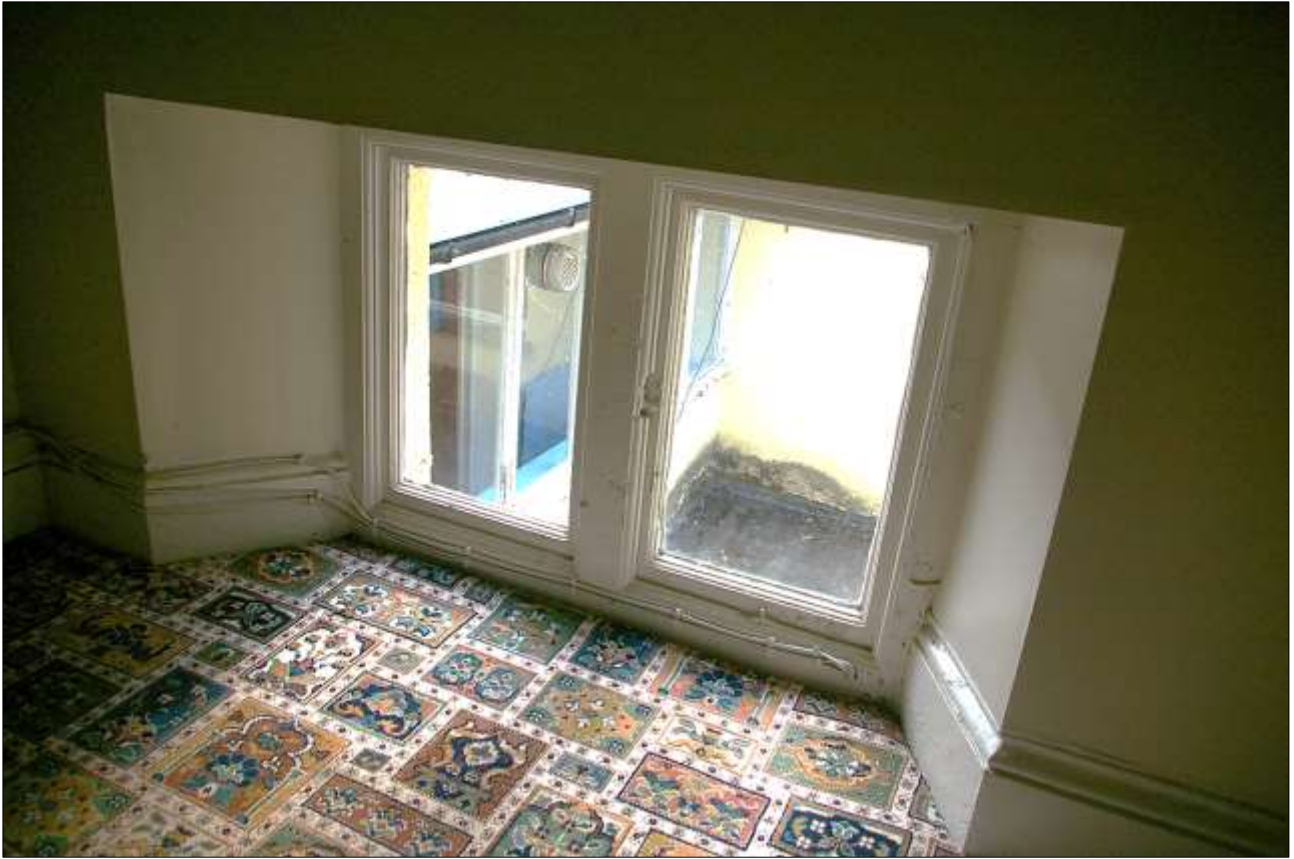
86. THE WINDOW AT THE TOP OF THE STAIR, CUT BY AN INSERTED HALF-LANDING IN BLOCK 7A; VIEWED FROM THE WSW.
