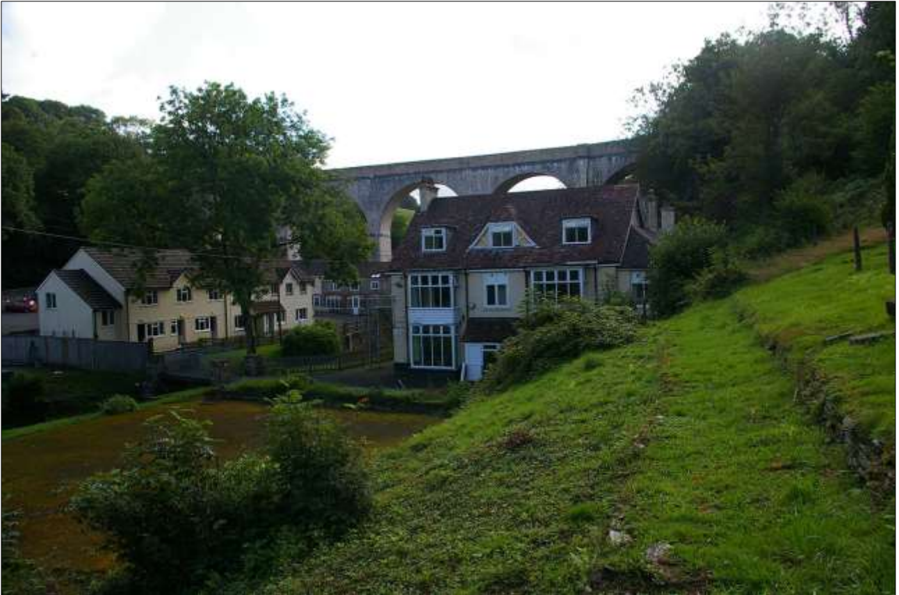
65. THE WHOLE SITE; VIEWED FROM THE SOUTH WEST.
