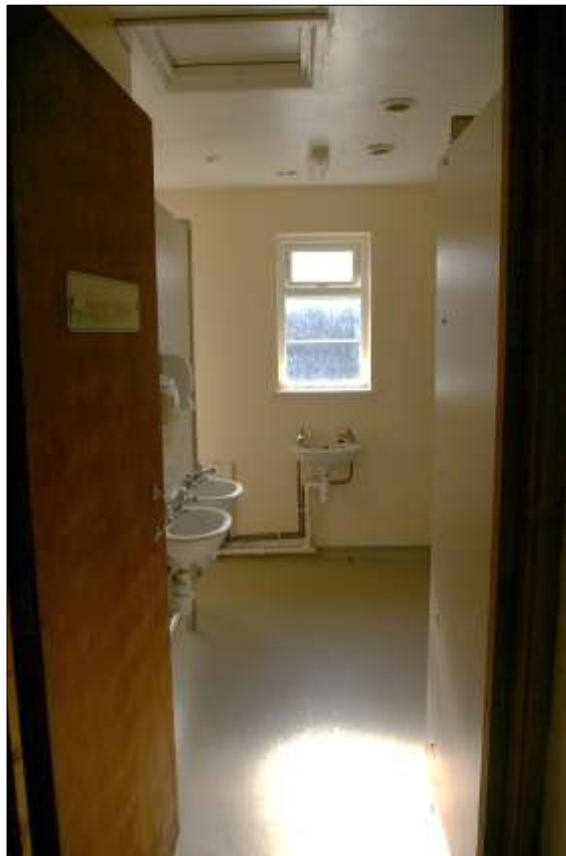
18. ONE OF THE MODERN BATHROOMS IN BLOCK 1; VIEWED FROM THE WEST.
