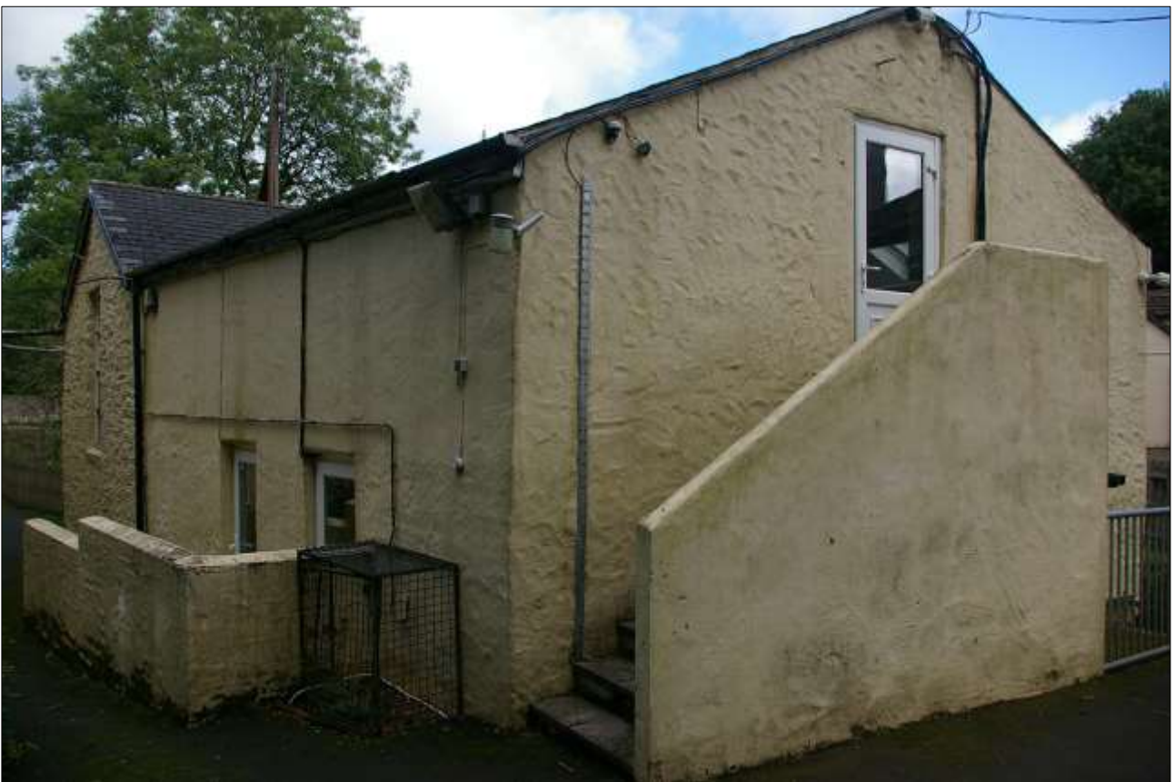
34. BLOCK 4B WITH STEPS TO LOFT; VIEWED FROM THE ESE.
