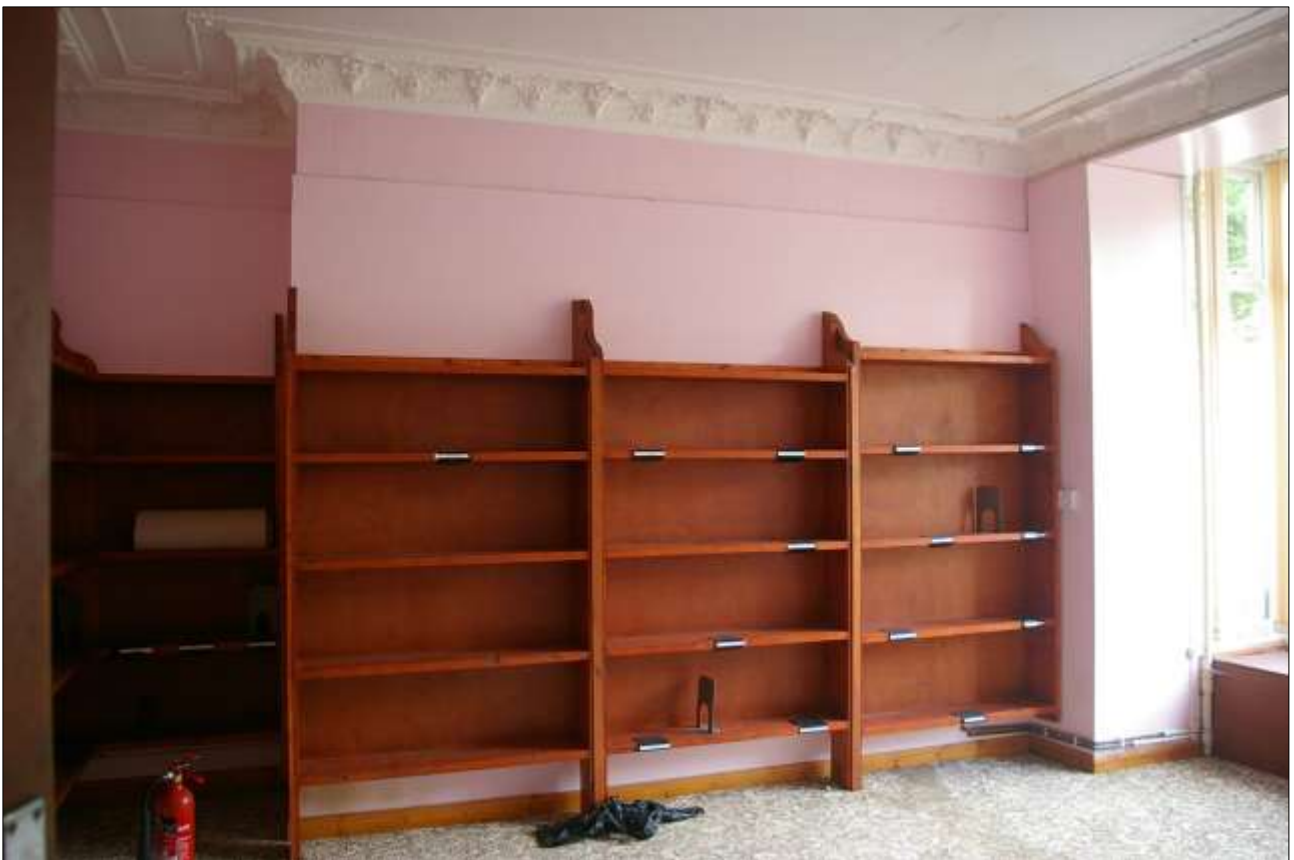
72. THE LARGE (BLOCKED) CHIMNEY BREAST IN THE LIBRARY, THE SECOND OF THE LARGE RECEPTION ROOMS; VIEWED FROM THE NORTH-EAST.
