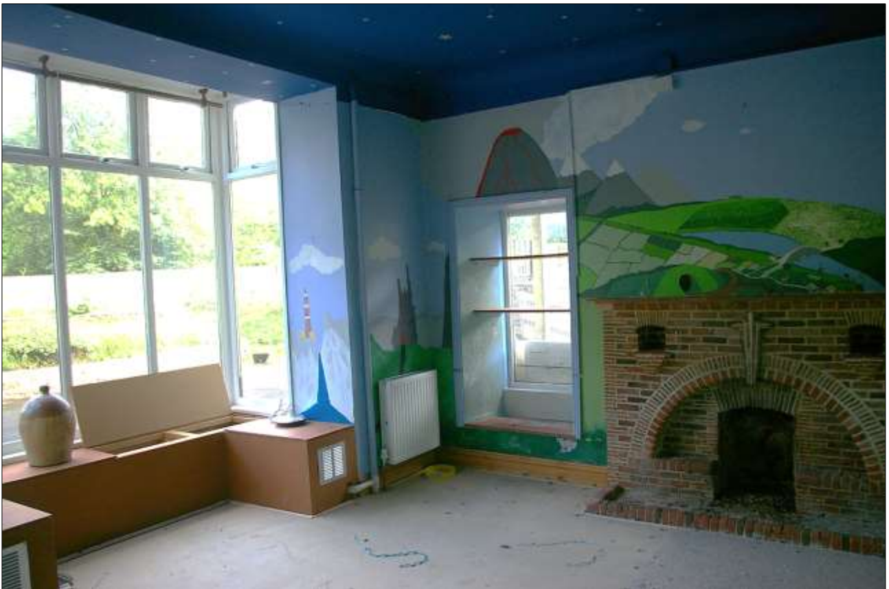
70. ONE OF THE MAIN RECEPTION ROOMS OF BLOCK 7A, SHOWING AN ALTERED ART DECO FIREPLACE AND LARGE WINDOW (PVC FRAMES); VIEWED FROM THE SOUTH-EAST.
