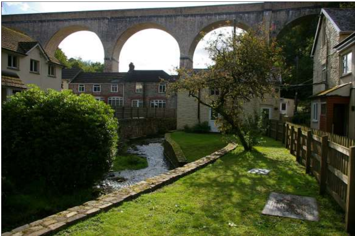
FIGURE 30: THE VIADUCT WITH THE CANALISED RIVER RUNNING BETWEEN BLOCK 1 AND BLOCK 4; FROM THE WEST-SOUTH-WEST.
