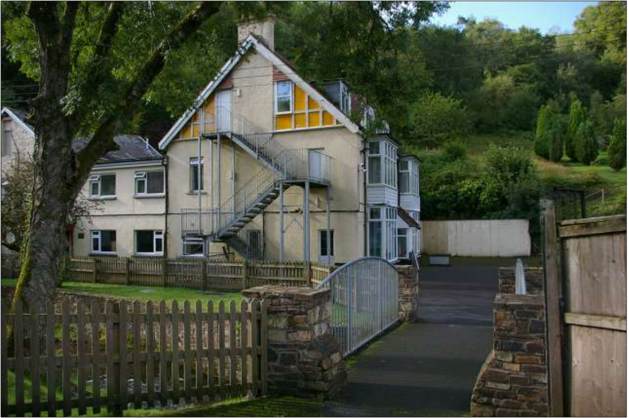
63. BLOCK 7A, THE HOUSE, VIEWED FROM ACROSS THE FOOTBRIDGE (THE OLD BRIDGE WAS WASHED AWAY BY FLOODS); VIEWED FROM THE NNW.
