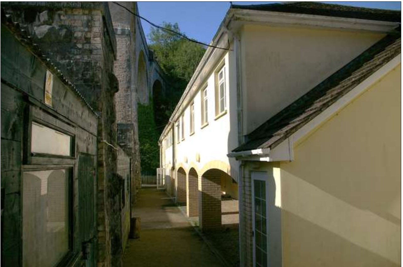
14. VIEW ALONG THE REAR SIDE OF BLOCK 1; VIEWED FROM THE NORTH.
