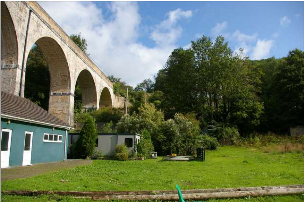
92. THE LARGE EASTERN GARDEN FIELD AREA, SHOWING THE VARIOUS STATIC CARAVANS AND SHEDS SET UNDER THE VIADUCT; VIEWED FROM THE SOUTH.
