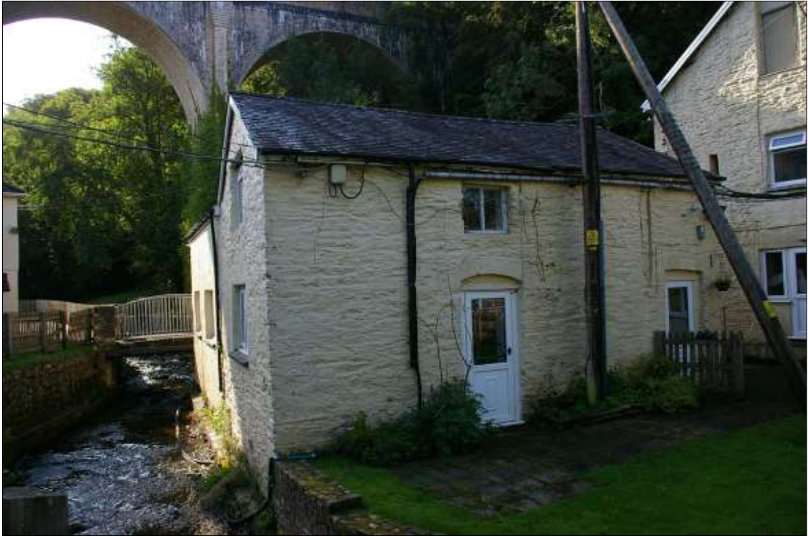
FIGURE 25: THE WEST AND NORTH ELEVATIONS OF BLOCK 4A; VIEWED FROM THE WNW.
