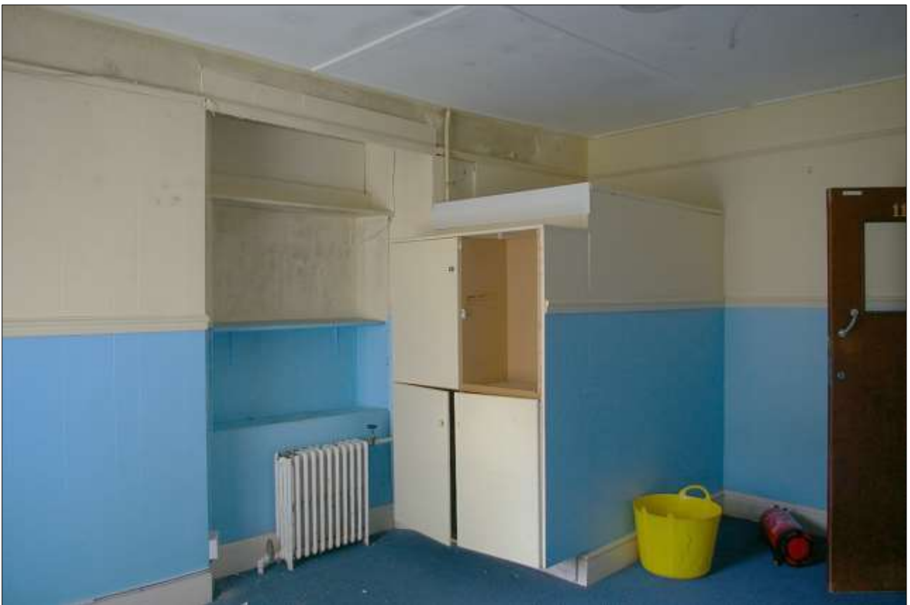
81. ONE OF THE LARGE FIRST-FLOOR BEDROOMS IN BLOCK 7A, WITH BLOCKED WINDOW AND FITMENTS FOR A DORMITORY; VIEWED FROM THE NORTH-EAST.
