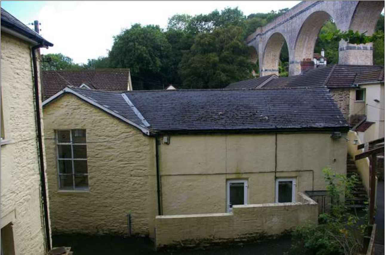
33. BLOCK 4 FROM THE SOUTH, SHOWING A TALL STAIR WINDOW FORCED INTO THE WALL OF BLOCK 4A; VIEWED FROM THE SOUTH.
