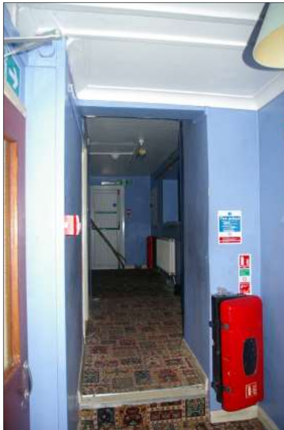
58. THE FORCED DOORWAY IN THE FIRST-FLOOR WEST WALL OF THE MILL THAT PROVIDES ACCESS TO BLOCK 7B; VIEWED FROM THE WEST.
