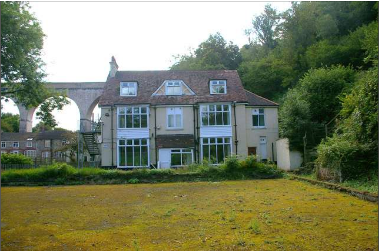
64. BLOCK 7A; VIEWED FROM THE WEST.
