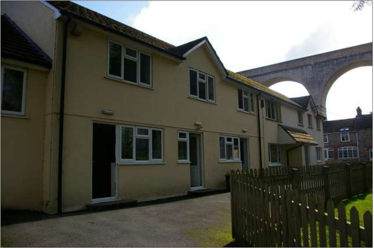
23. BLOCK 3 (3B TO THE FOREGROUND), SHOWING THE GROUND FLOOR CLASSROOMS WITH FIRST FLOOR OFFICES; VIEWED FROM THE SOUTHWEST.
