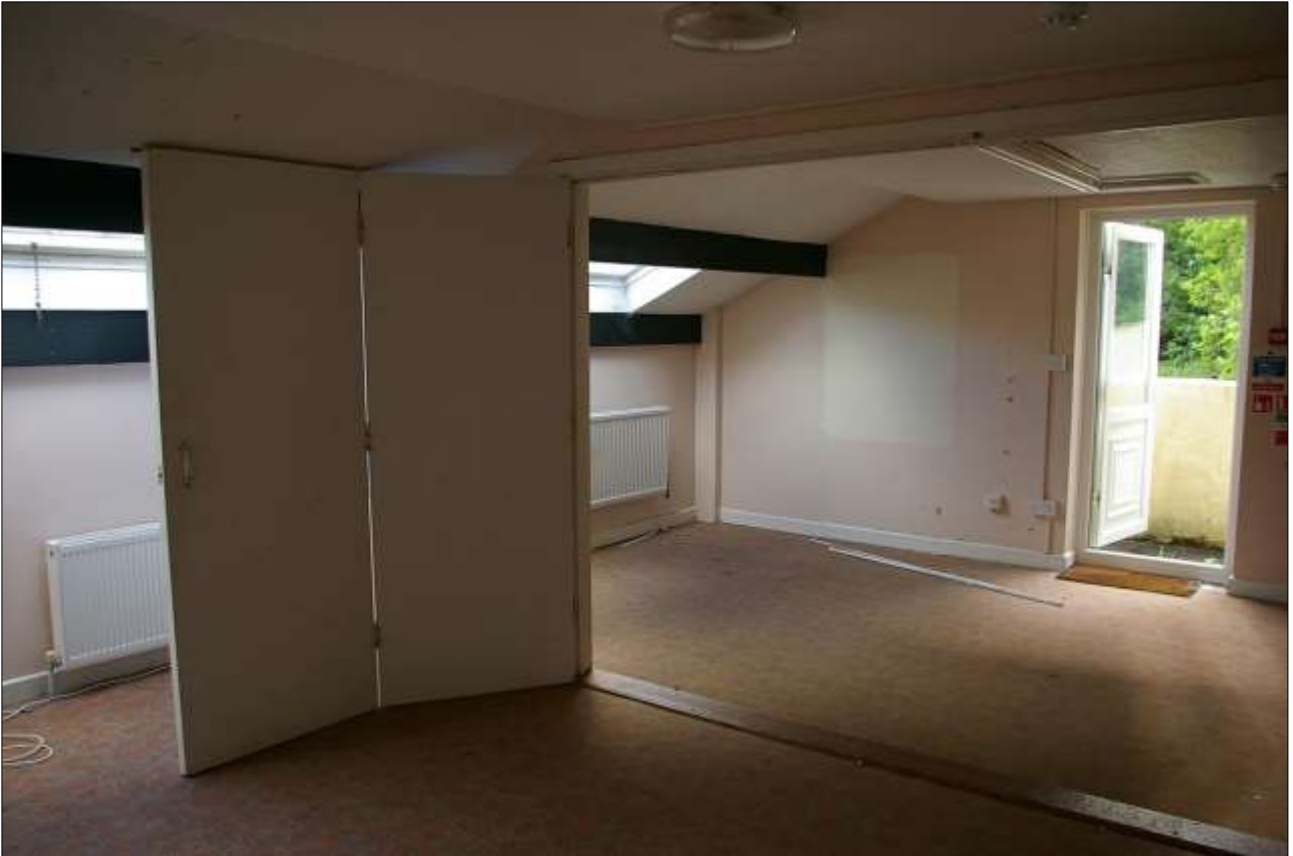
39. THE LOFT IN BLOCK 4B; VIEWED FROM THE SOUTH-WEST.
