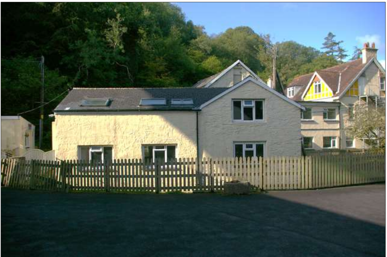
30. BLOCK 4, WITH BLOCK 4A TO THE WEST AND BLOCK 4B (THE EXTENSION) TO THE EAST; VIEWED FROM THE NORTH.
