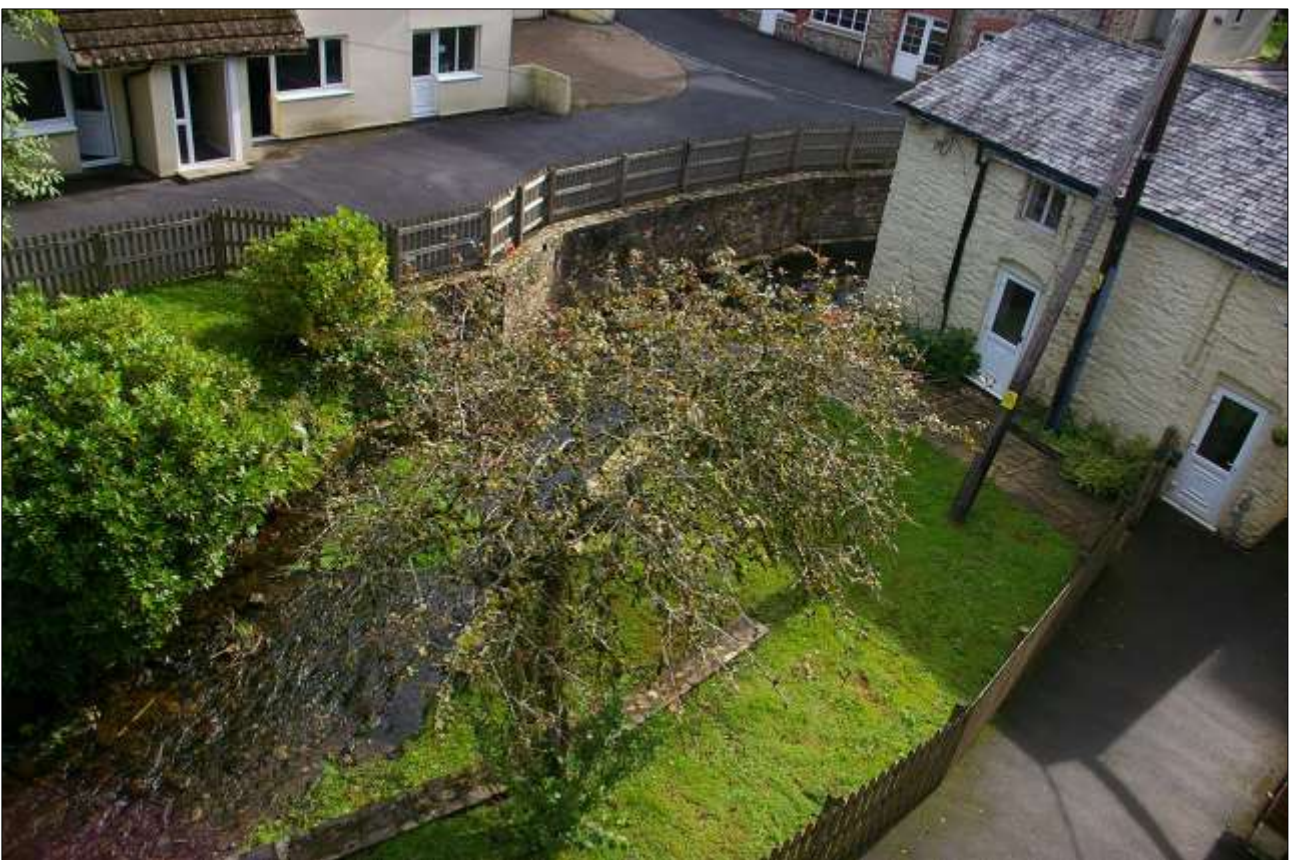
32. VIEW OF THE CANALISED RIVER RUNNING PAST BLOCK 4; VIEWED FROM ABOVE.
