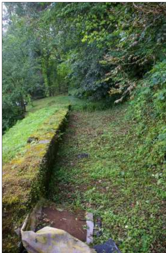
52. THE SILTED-UP LEAT LEADING TO THE OVERSHOT WATERWHEEL, JUST SOUTH-EAST OF BLOCK 6; VIEWED FROM THE WEST.
