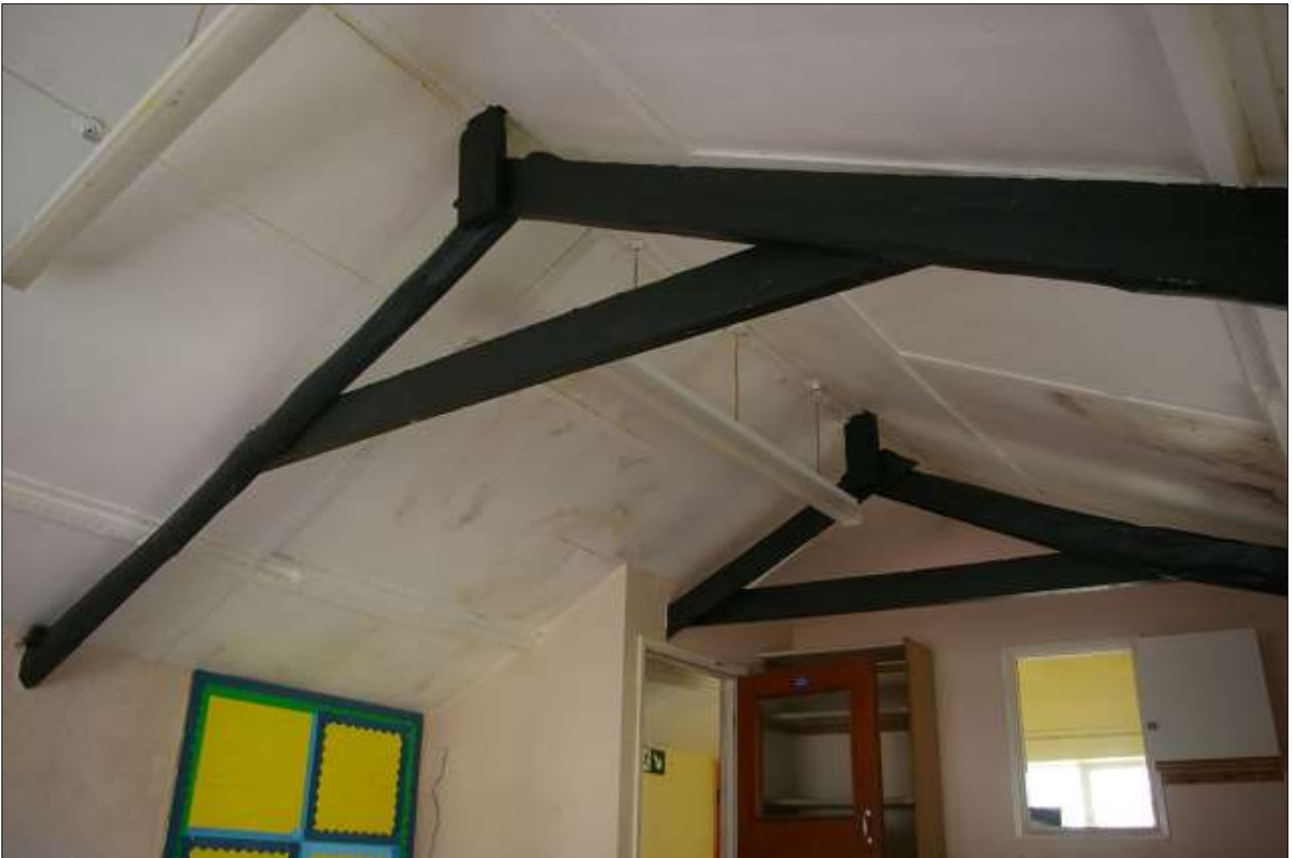
41. THE TWO A-FRAME TRUSSES OVER BLOCK 4A; VIEWED FROM THE NORTH-WEST.
