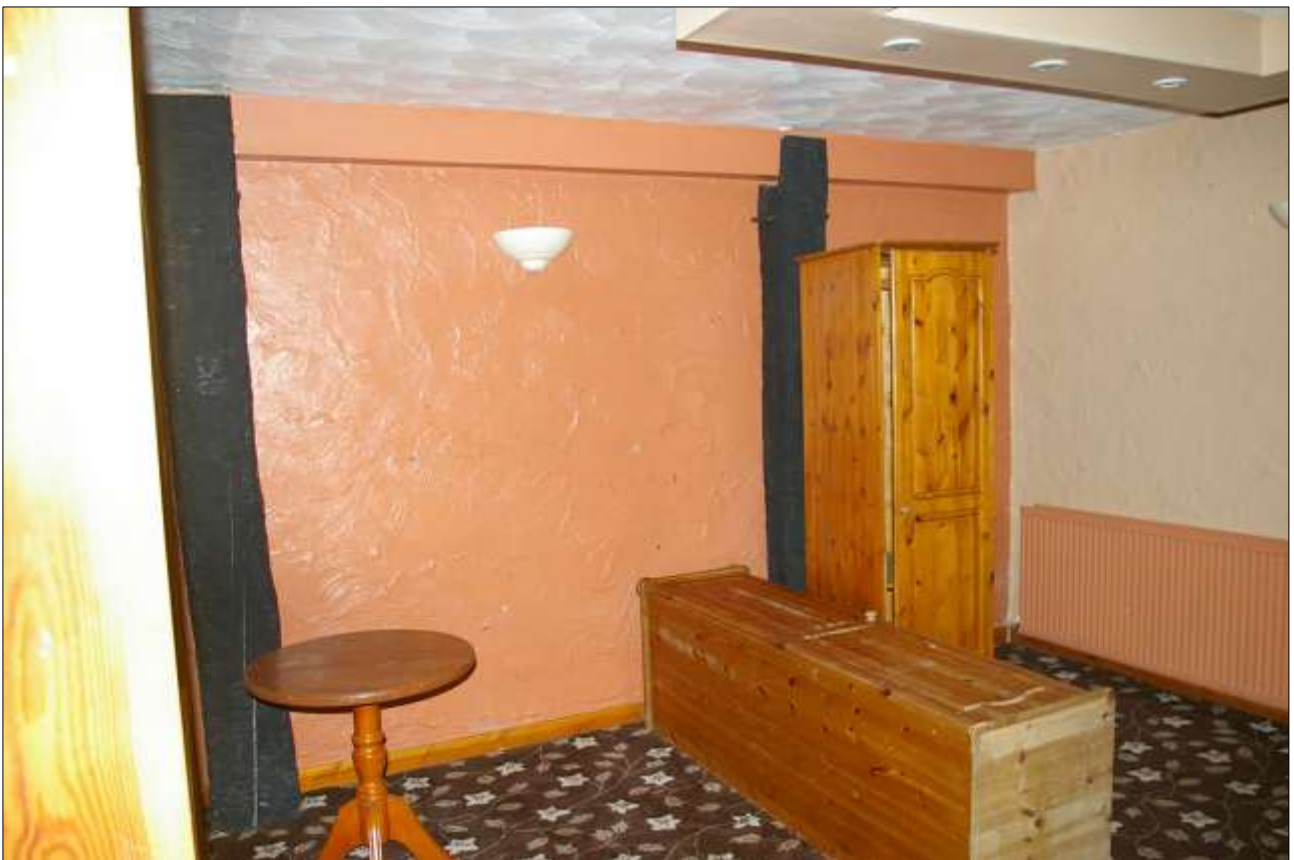
56. BEAMS ON THE INTERIOR OF THE EAST WALL BRACING THE WATERWHEEL ON THE EXTERIOR OF BLOCK 6; VIEWED FROM THE WNW.
