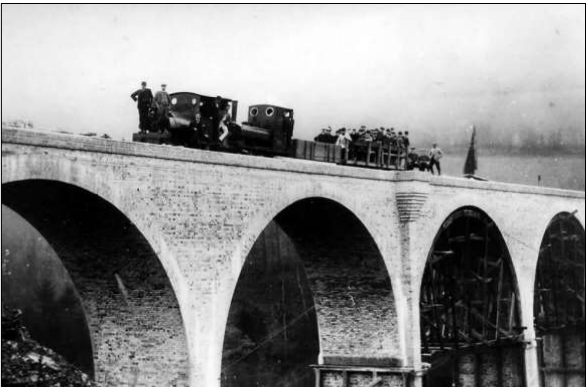
FIGURE 10: PHOTOGRAPH OF THE VIADUCT UNDER CONSTRUCTION IN 1896; VIEWED FROM THE NORTH-WEST (©LYNTON & BARNSTAPLE RAILWAY WEBSITE).
