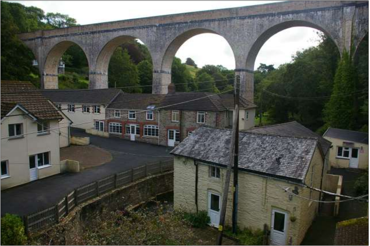
35. THE WIDER SETTING OF BLOCK 4 WITHIN THE SITE, SHOWING THE PHYSICAL DOMINANCE OF THE VIADUCT; VIEWED FROM THE SOUTH-WEST.
