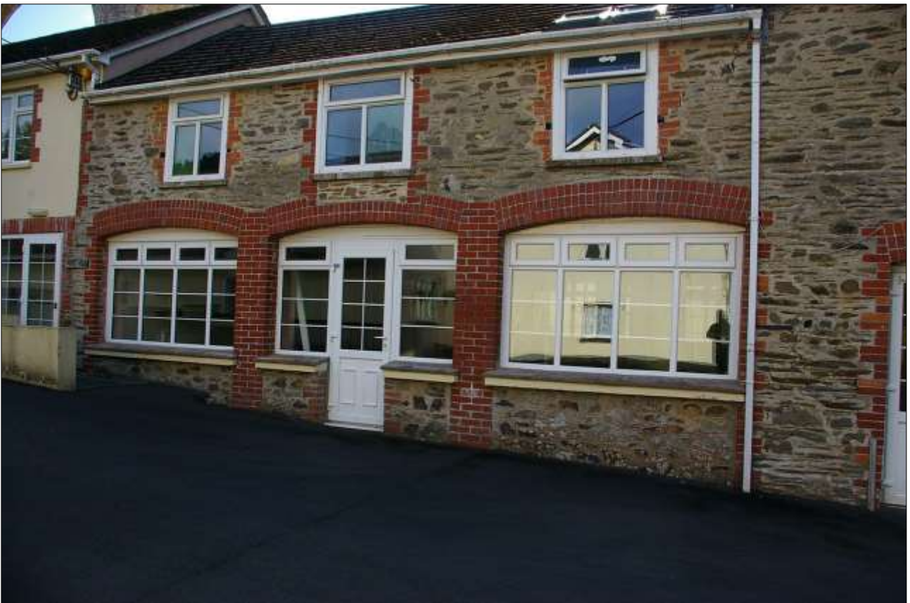
10. DETAIL OF THE BRICK ARCHES IN BLOCK 1A; VIEWED FROM THE WSW.
