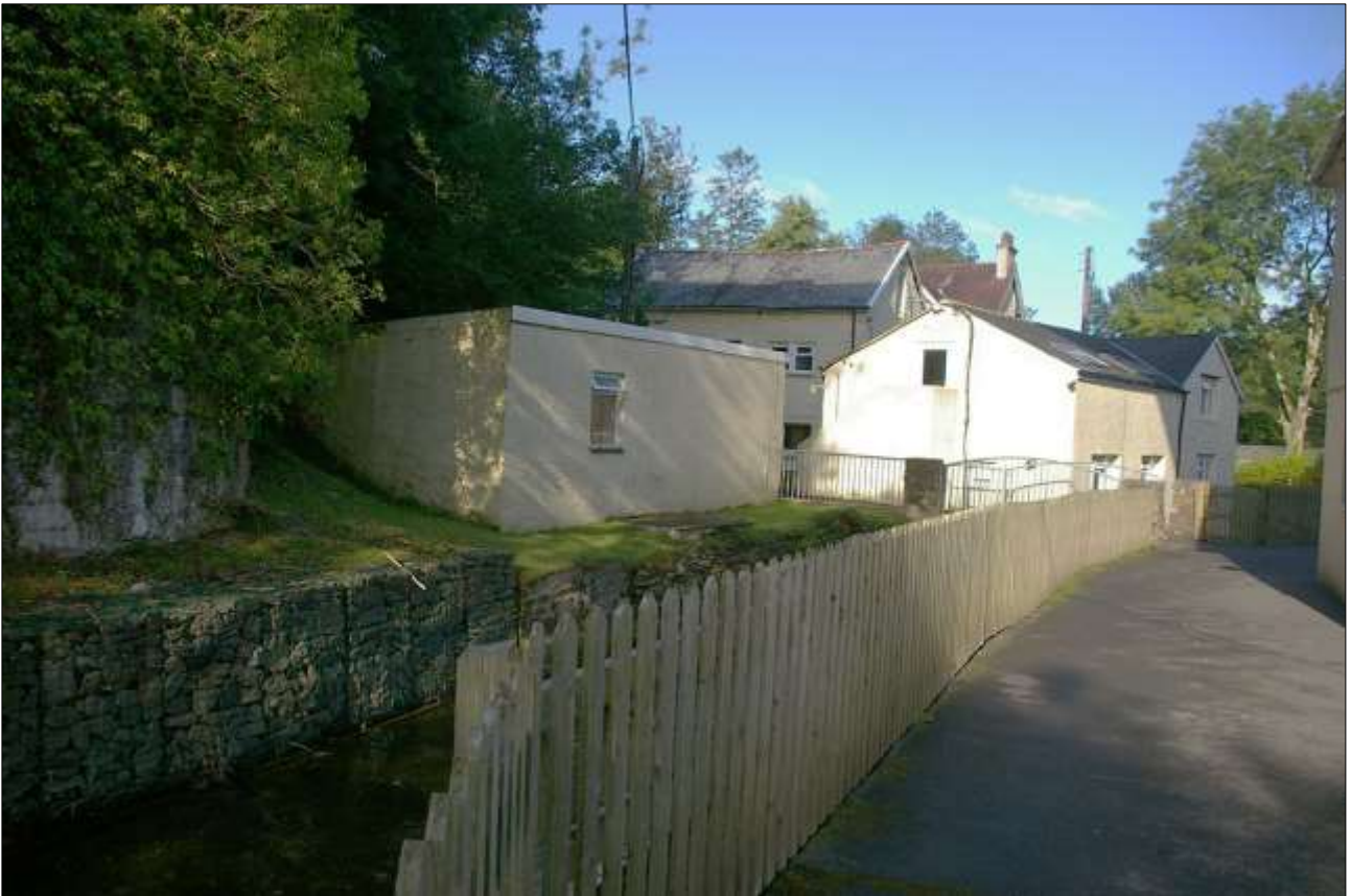
43. BLOCK 5, WITH THE RIVER RUNNING PAST, VIEWED FROM UNDER THE VIADUCT; VIEWED FROM THE NORTH.
