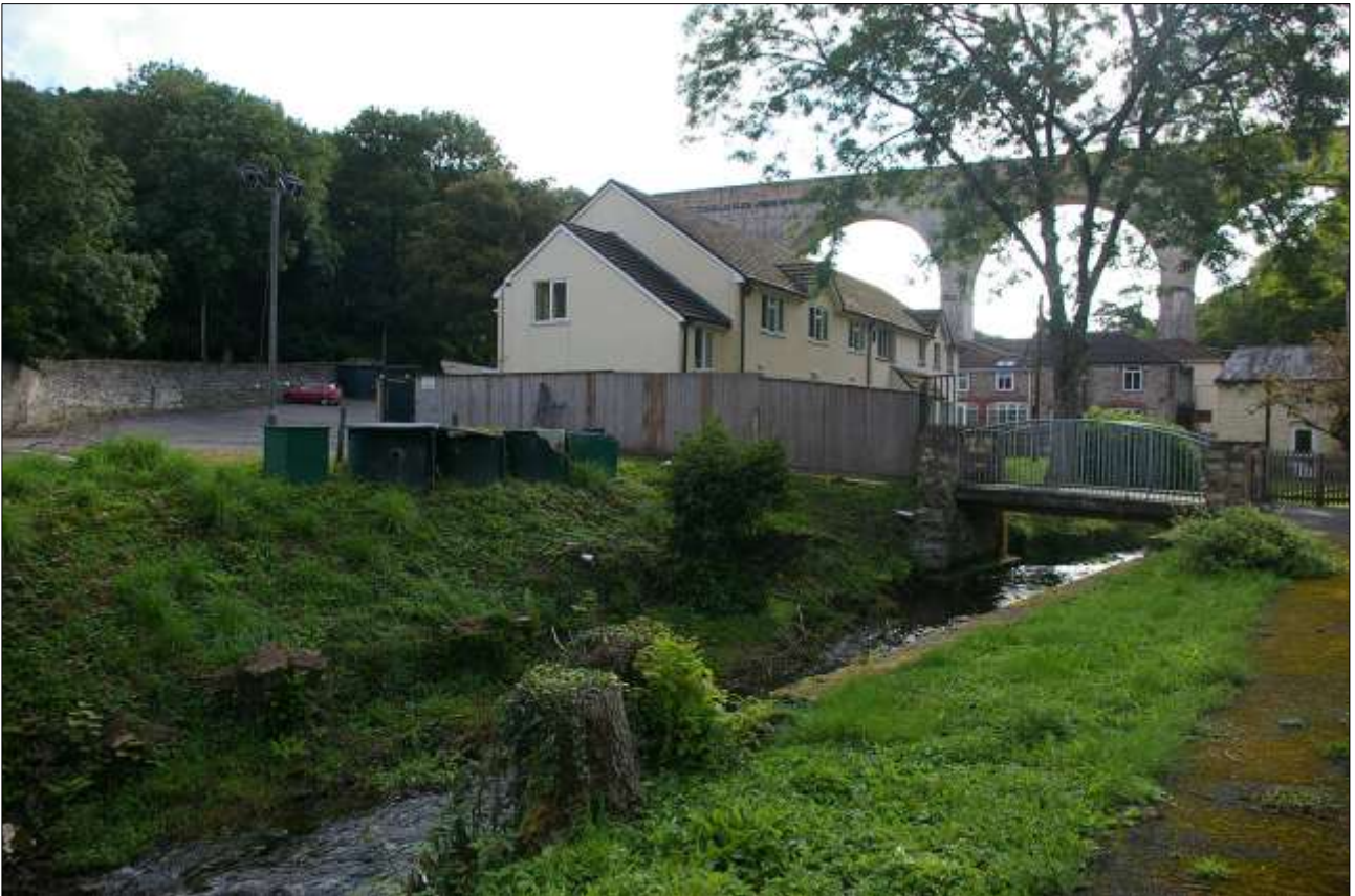
48. THE SITE AND RIVERBANK; VIEWED FROM THE SOUTH WEST.
