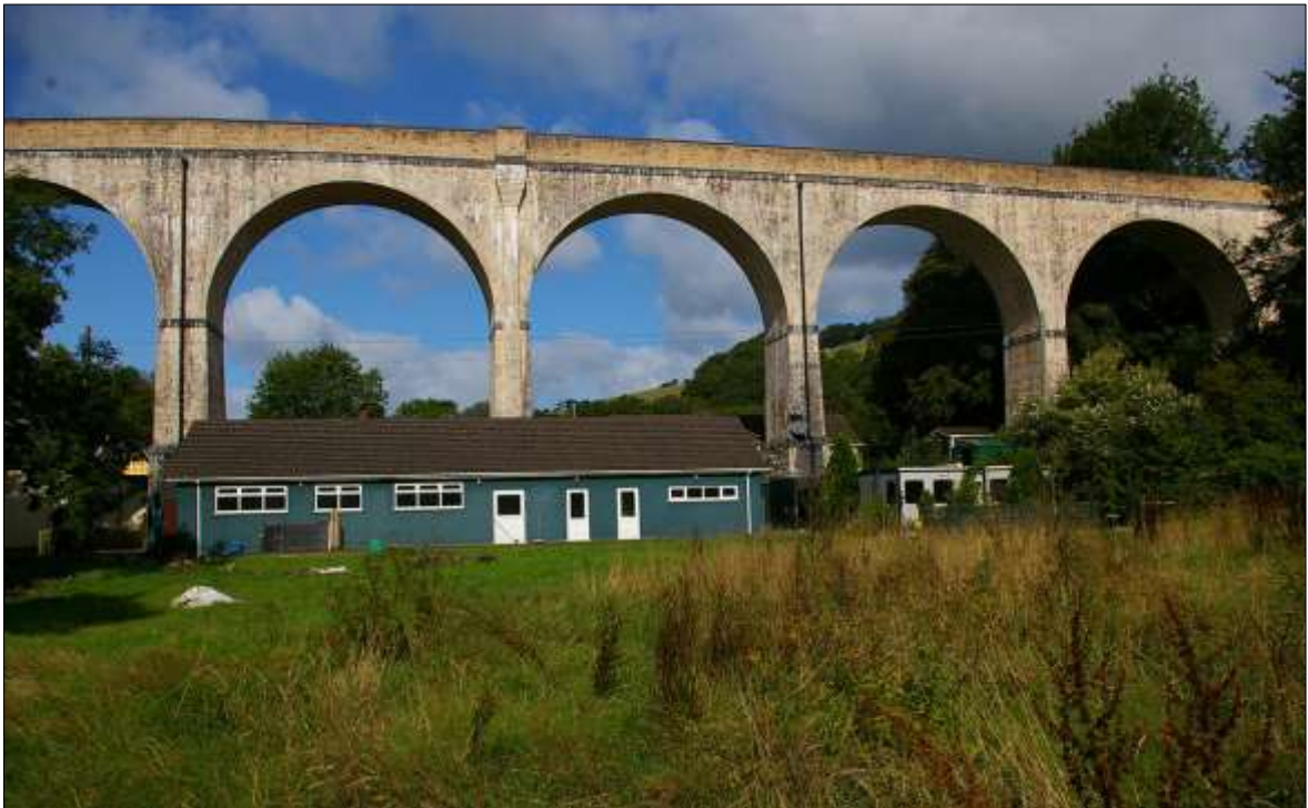
FIGURE 29: BLOCK 8, TO THE EAST OF THE VIADUCT; VIEWED FROM THE EAST.
