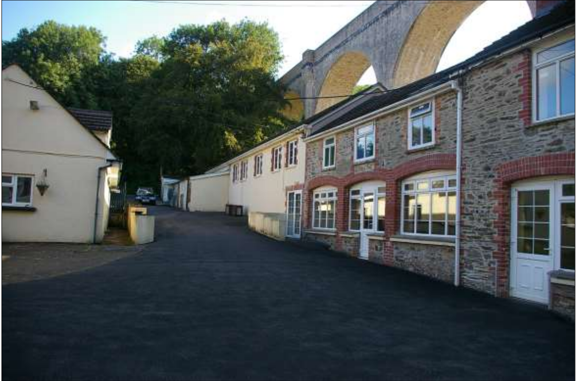
FIGURE 22: BLOCK 1 (RIGHT) AND BLOCK 2 (LEFT); VIEWED FROM THE SSW.
