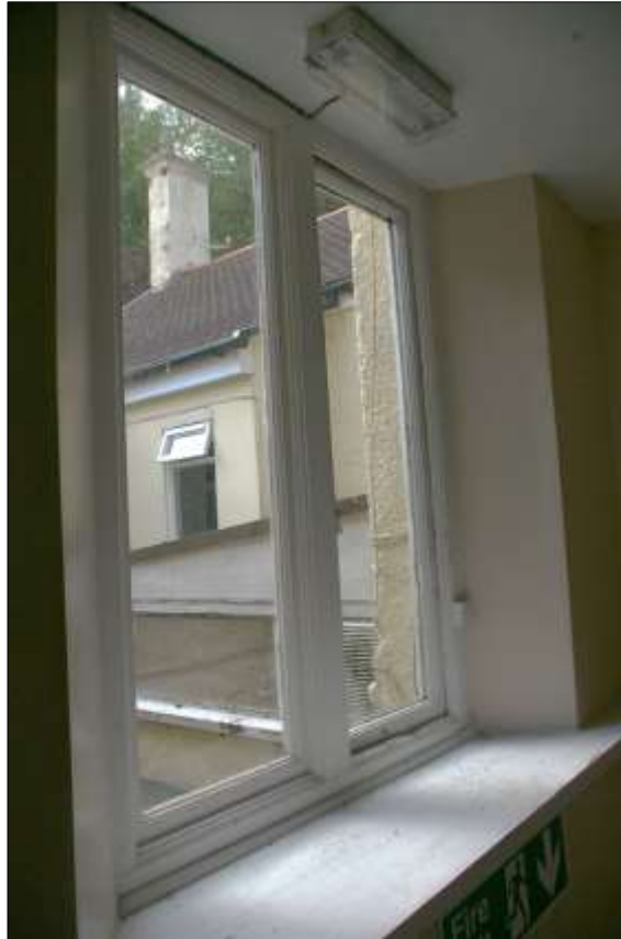
80. THE STAIR WINDOW TO BLOCK 7A; VIEWED FROM THE NORTH.
