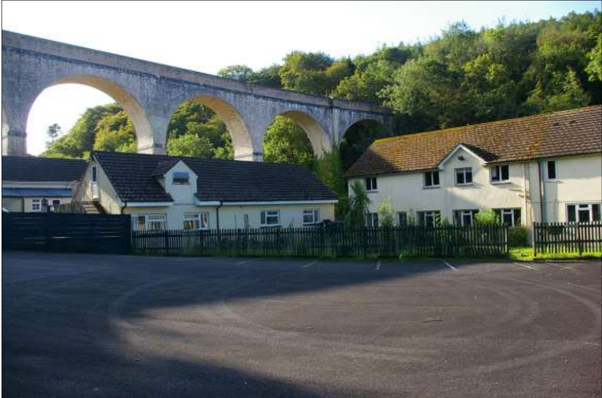
FIGURE 24: BLOCK 2 (LEFT) AND BLOCK 2 (RIGHT); VIEWED FROM THE NORTH-WEST.
