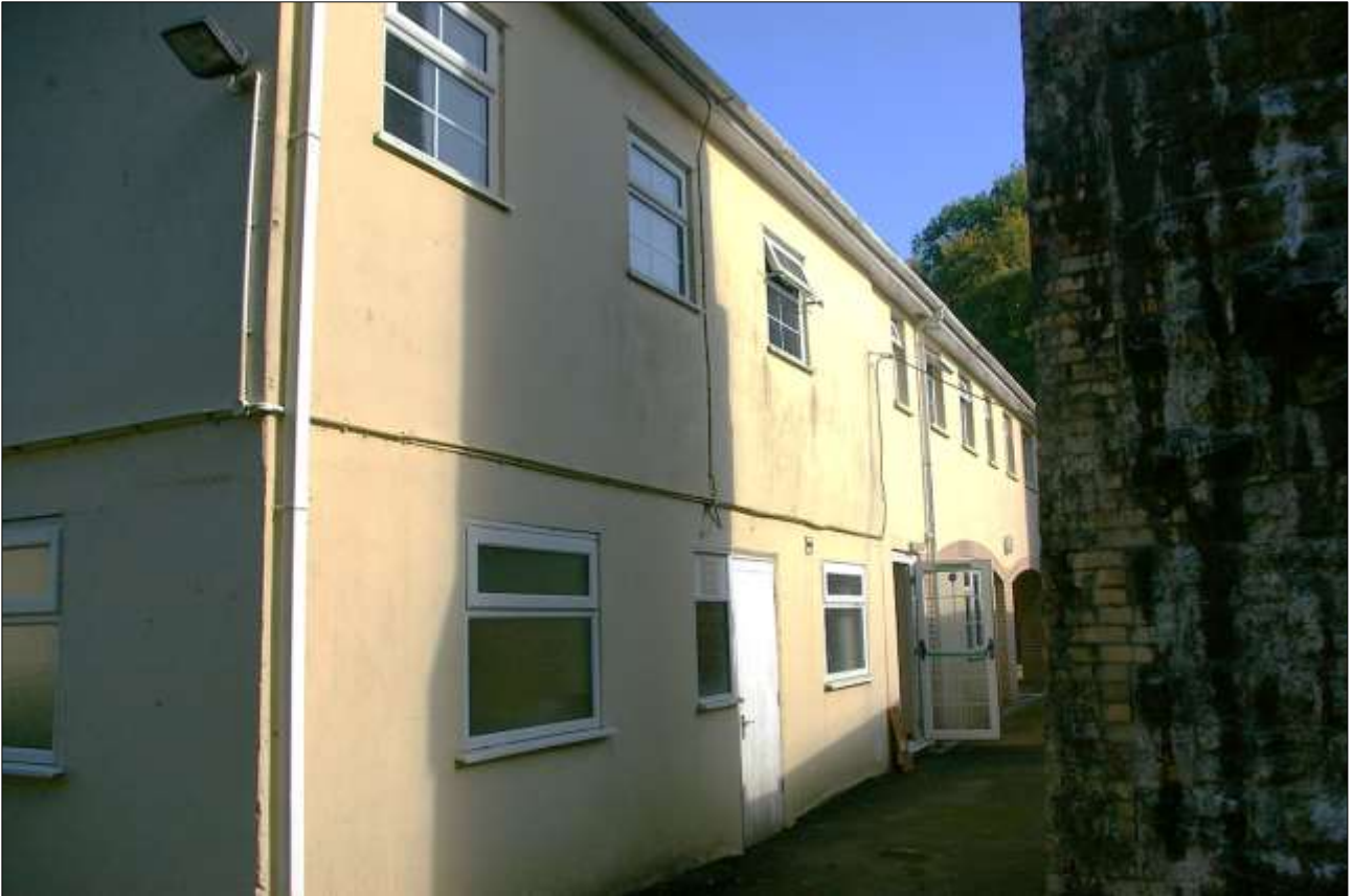
11. THE REAR ELEVATION OF BLOCK 1, SHOWING THE CLOSE PROXIMITY TO THE VIADUCT; VIEWED FROM THE SOUTH-EAST.
