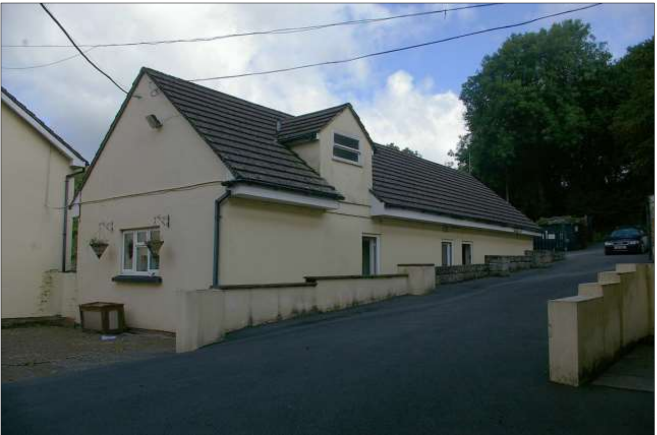
20. THE NORTH ELEVATIONS OF BLOCK 2 AND 3 BEHIND; VIEWED FROM THE NNE.
