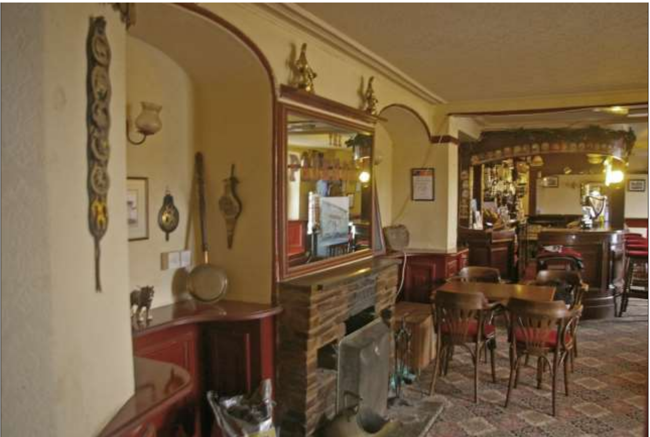
16. R2, DETAILED PROFILE VIEW OF THE BASKET ARCHES AND ALTERED FIREPLACE (FP1); VIEWED FROM THE SOUTH-SOUTH-EAST.
