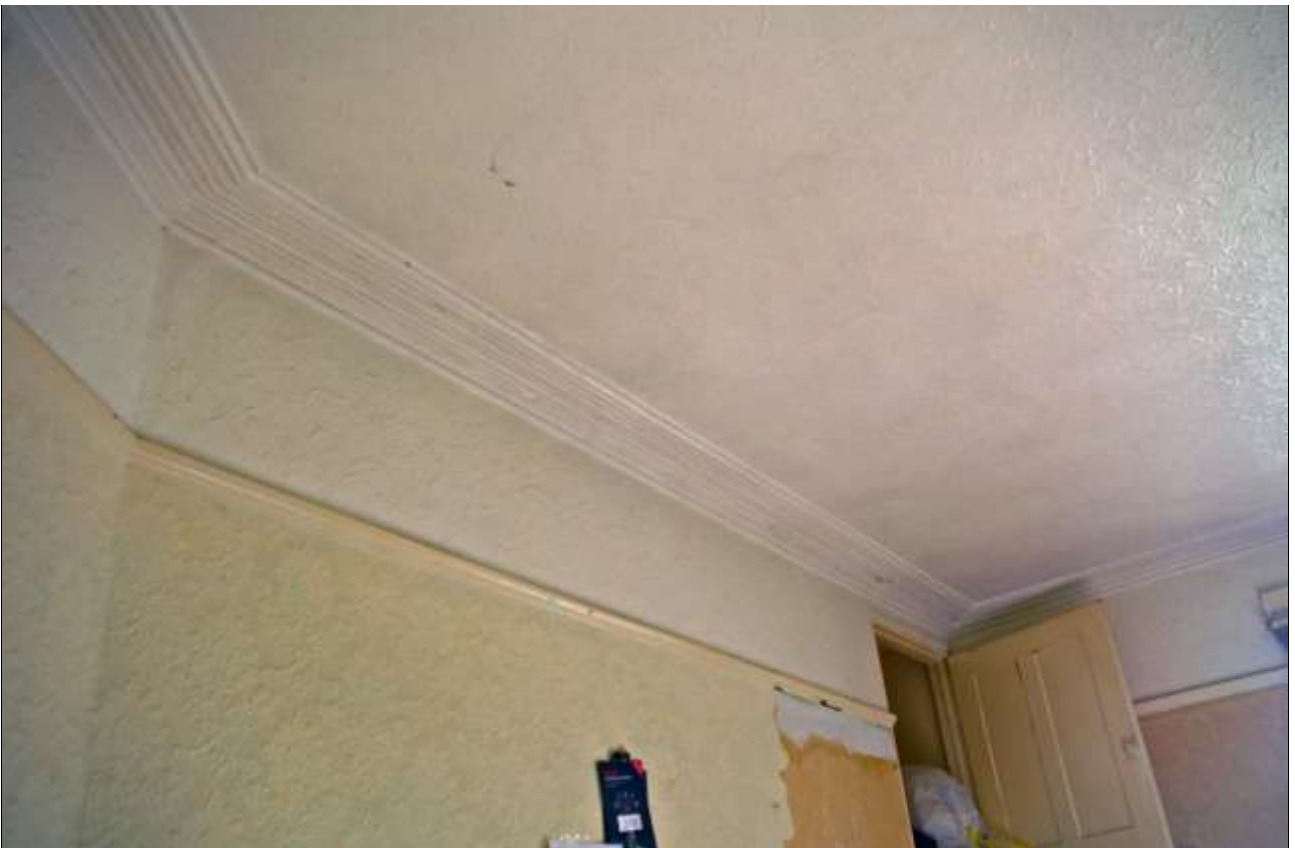
41. R14, DETAIL OF THE REEDED CORNICE; VIEWED FROM THE NORTH-WEST.
