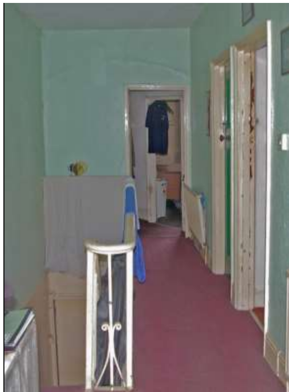
35. LEFT: R7, VIEW DOWN THE STAIRS WITH RAMPED HOGS-BACK HANDRAIL AND STICK BALUSTERS; VIEWED FROM THE NORTH-NORTH-WEST.
