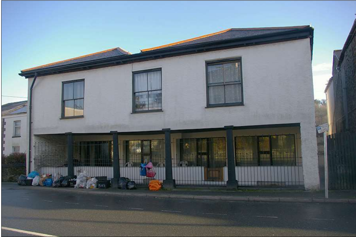
FIGURE 21: THE FORMER MARKET HOUSE SHOWING THE OPEN FRONTING AND JETTIED 1 ST FLOOR; VIEWED FROM THE WEST-SOUTH-WEST.
