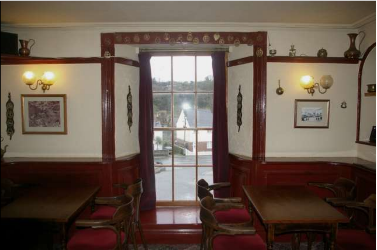
15. R2, DETAIL OF W1 IN THE EAST WALL, WITH FINE REEDED TIMBER SURROUND, CUT OFF BELOW TO ACCOMMODATE THE MODERN 'HERITAGE STYLE' PUB PANELLING; VIEWED FROM THE WEST.
