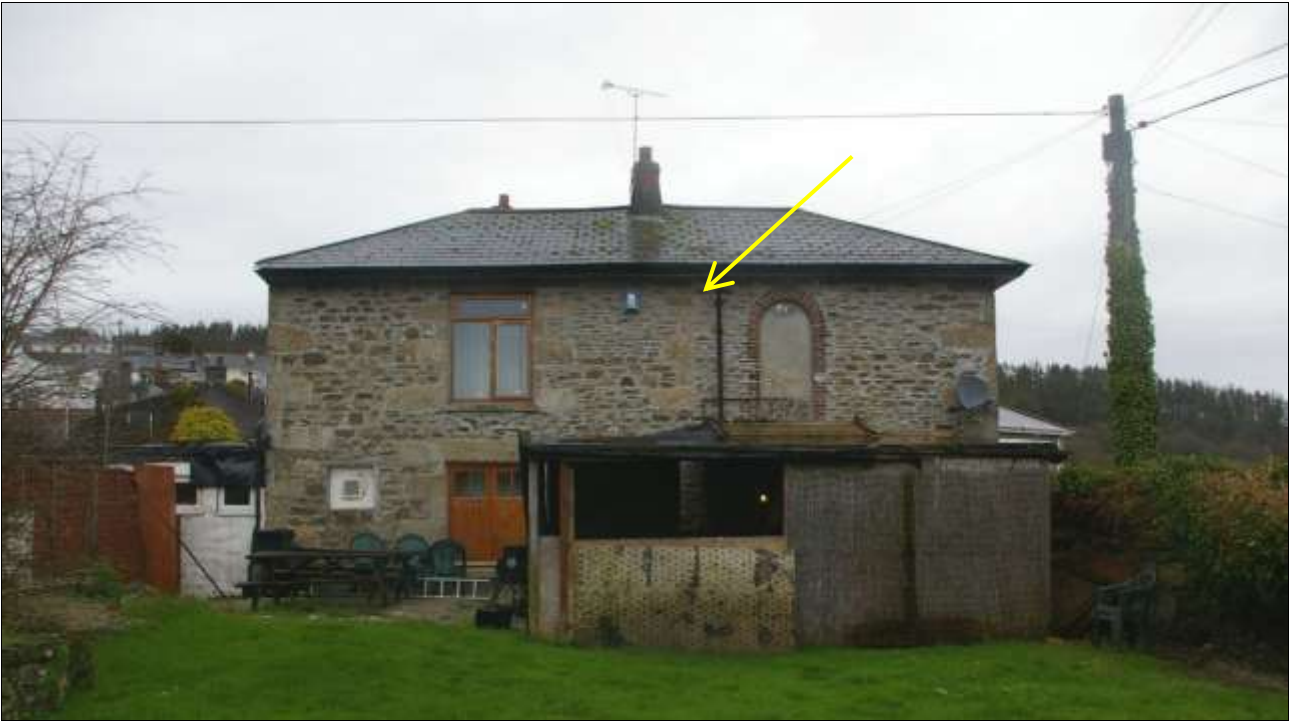
5. THE SOUTH ELEVATION OF THE INN SHOWING CLEAR PHASING; THE EAST BLOCK (LEFT) ABUTS THE QUOINS OF THE EARLIER WEST BLOCK (LEFT), AS INDICATED; VIEWED FROM THE SOUTH.
