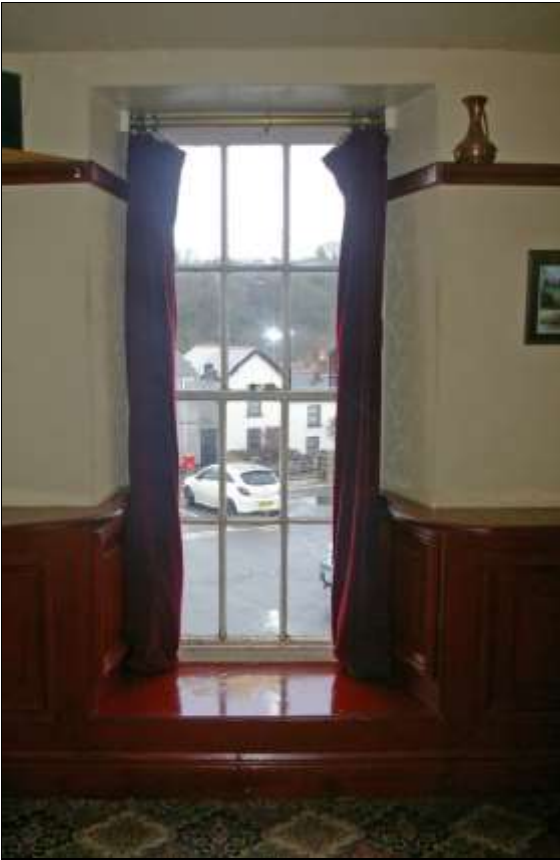
21. R3B, DETAIL OF W3 IN THE EAST WALL; VIEWED FROM THE WEST.
