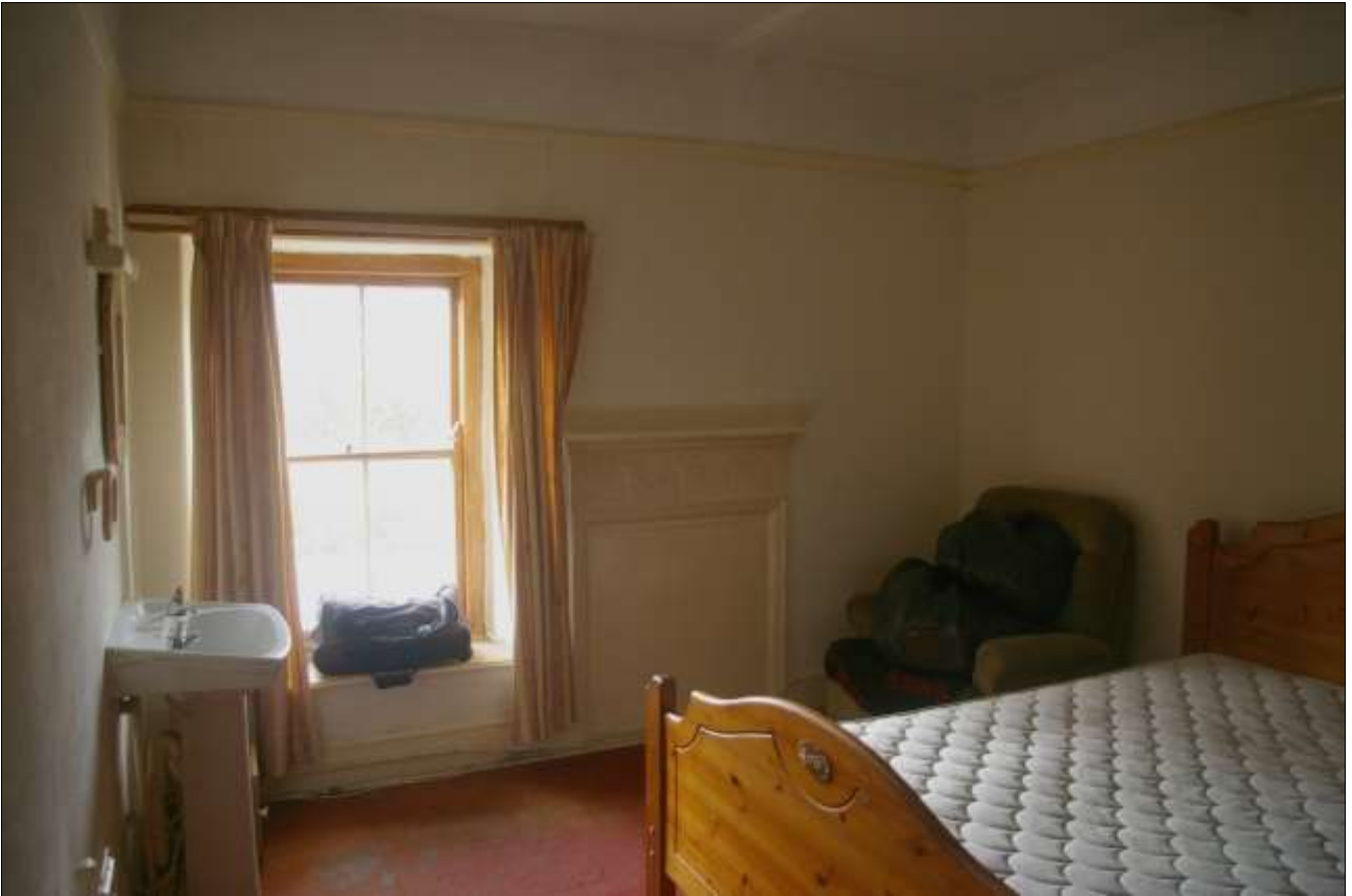
40. R11, REDUCED IN THE 20 TH CENTURY WITH NEW PICTURE RAIL AND BOARDED CEILING INSTALLED, BUT OLDER FIREPLACE SURROUND TO BLOCKED HEARTH RETAINED (FP3); VIEWED FROM THE EAST-SOUTH-EAST.
