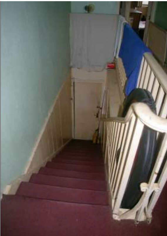
35. LEFT: R7, VIEW DOWN THE STAIRS WITH RAMPED HOGS-BACK HANDRAIL AND STICK BALUSTERS; VIEWED FROM THE NORTH-NORTH-WEST.
