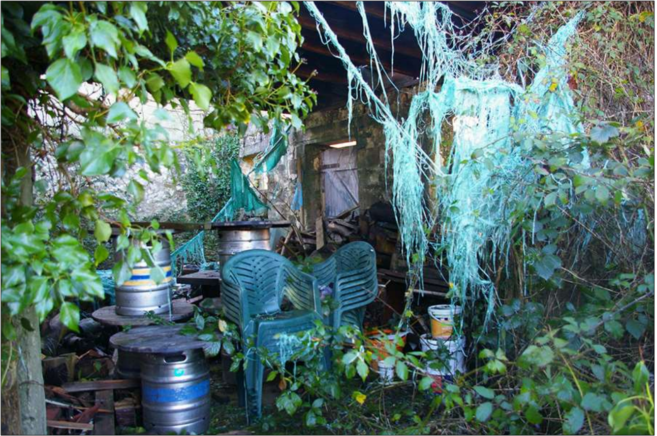
51. DETAIL OF THE INTERIOR OF THE DERELICT OUTBUILDING; VIEWED FROM THE NORTH-EAST.
