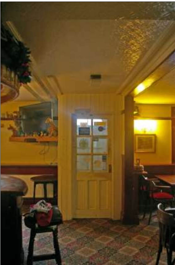
6. LEFT: R1, THE PLANK PARTITION WEATHER PORCH AROUND THE FRONT DOOR (D2) AND PRESENCE OF THE REEDED CORNICE, SHOWING THE LINE OF THE REMOVED PARTITION WALLS; VIEWED FROM THE WEST. 7. RIGHT: R1, THE DOORWAY IN THE WEST WALL (D3), LEADING INTO THE REAR WEST BLOCK (R5), WITH DOORFRAME ETC. REMOVED; VIEWED FROM THE EAST.
