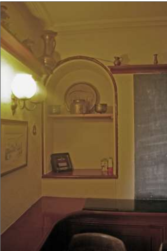
14. R2, THE ROUND-HEADED SHELVED ALCOVE IN THE SOUTH-EAST CORNER, A GOOD LATE GEORGIAN/REGENCY DETAIL; VIEWED FROM THE NORTH-NORTH-WEST.
