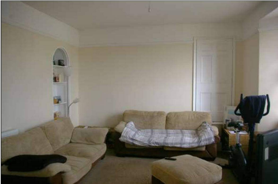
FIGURE 16: THE ROUND ARCHED ALCOVE AND PANNELLED DOOR TO CUPBOARD IN ROOM 15C; VIEWED FROM THE SSE.
