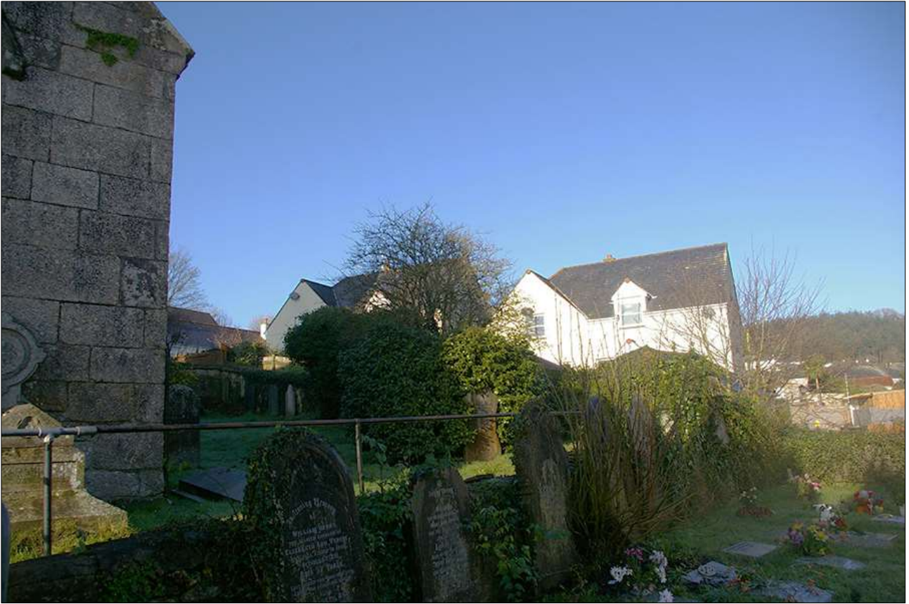
68. VIEW OF THE MODERN DEVELOPMENT OF CHURCHFIELD PLACE FROM THE CHURCHYARD; VIEWED FROM THE SOUTH-SOUTH-EAST.
