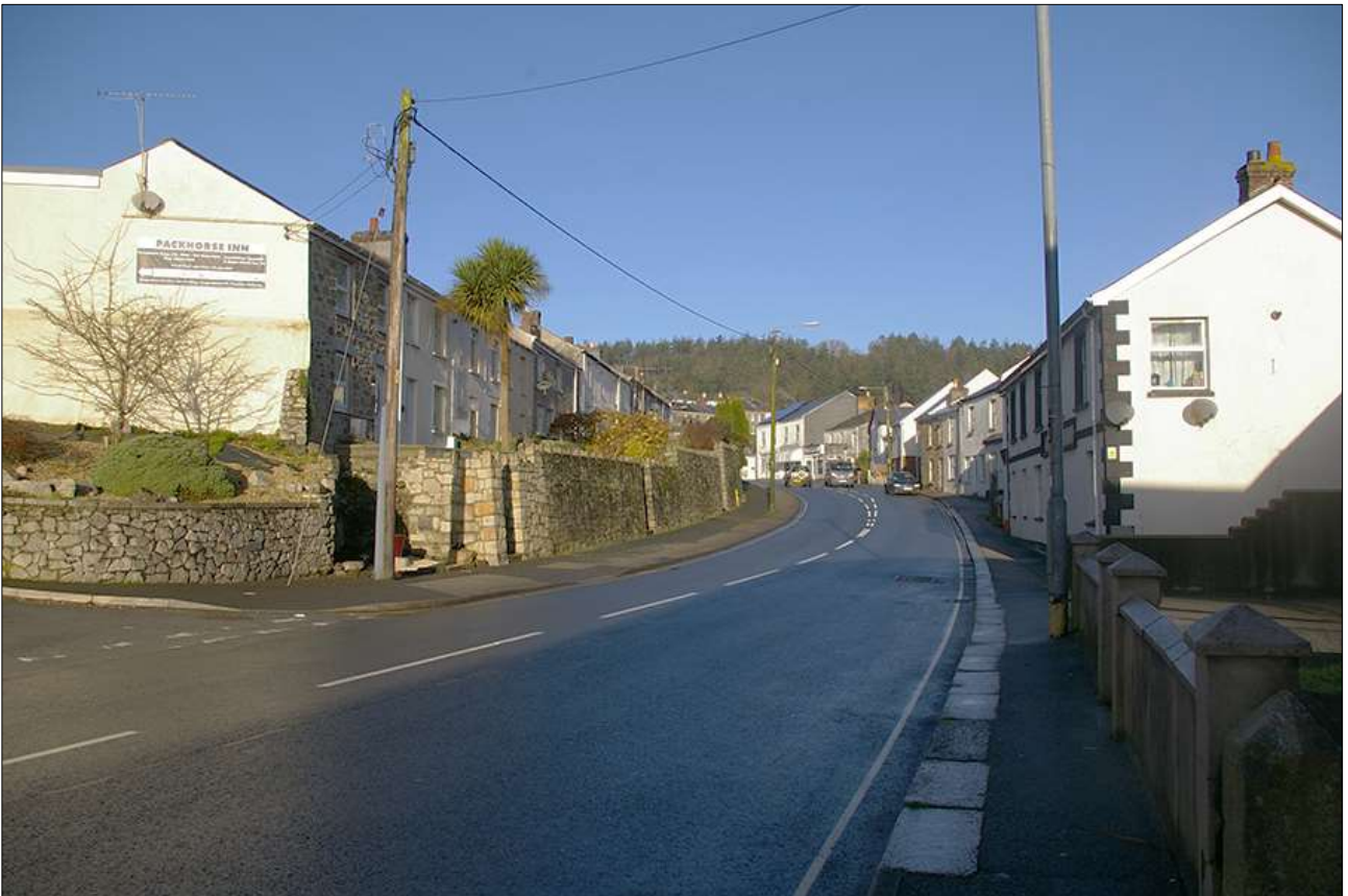
63. VIEW ALONG FORE STREET TOWARDS THE TOWN SQUARE; VIEWED FROM THE SOUTH-SOUTH-EAST.
