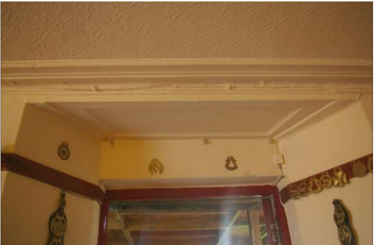
12. R2, THE PANELLED PLASTER DETAIL ABOVE A FORMER WINDOW IN THE SOUTH WALL (D4), WITH REEDED CORNICE TO CEILING; VIEWED FROM THE NORTH.
