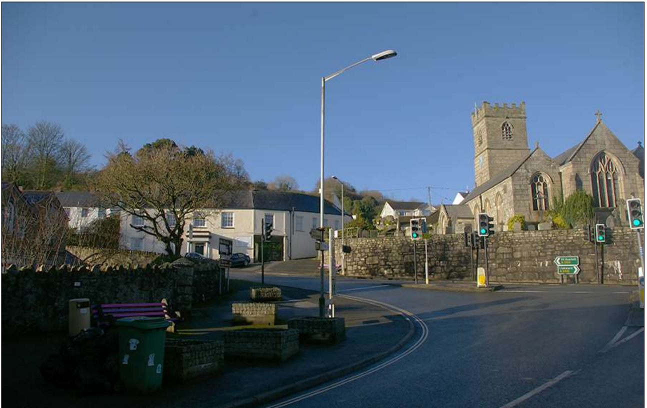
64. VIEW ACROSS THE JUNCTION OF FORE STREET, STATION ROAD AND DUKE STREET, SHOWING THE CHURCH OF ST BLAISE AND CORNISH ARMS INN IN RELATION TO THE INTRUSIVE ROAD FURNITURE; VIEWED FROM THE EAST.
