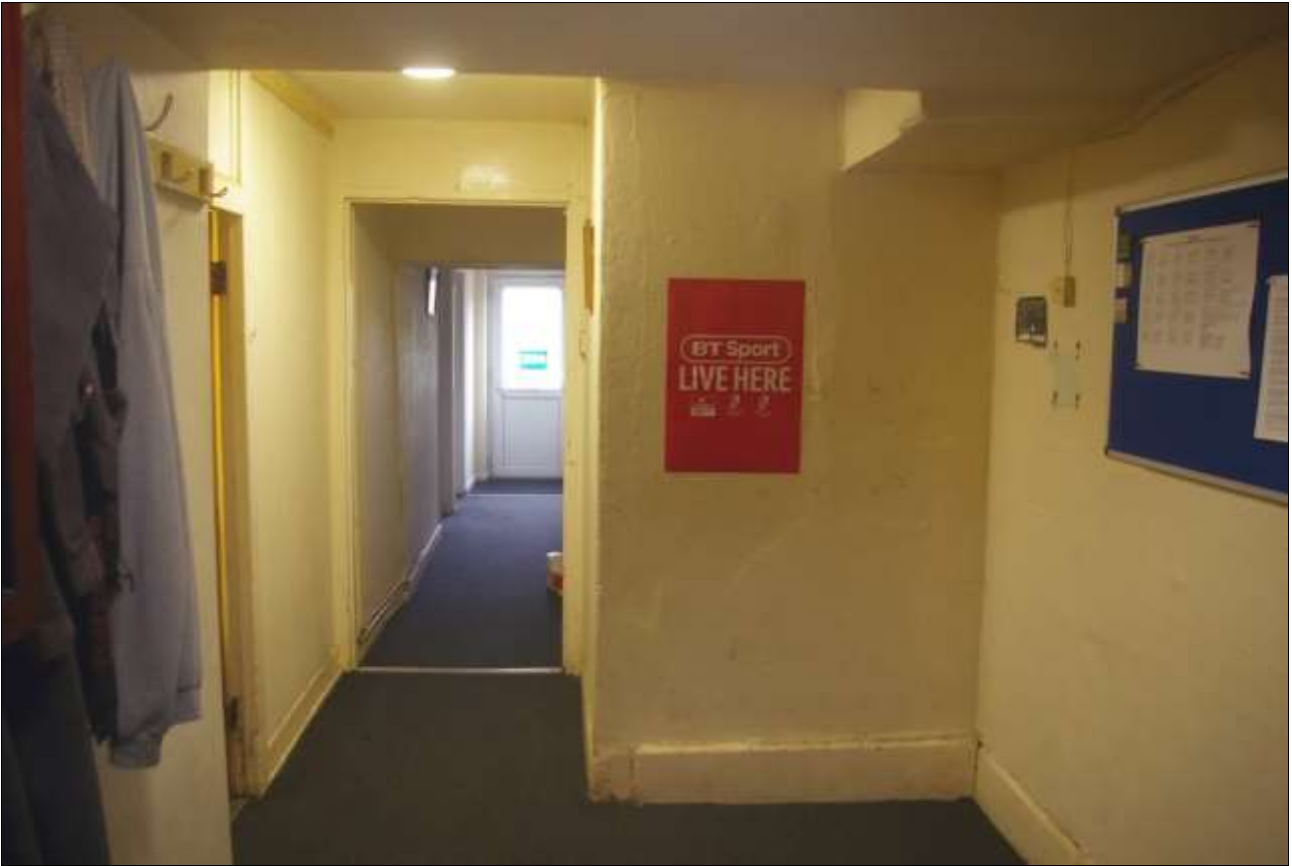
27. R5, SHOWING THE DOGLEG SECTION OF WALL WITH BLOCK OF MASONRY (STACK?) AND SCAR FOR FORMER RISING STAIR (CENTRE). GOOD DOORWAY (D7) TO LEFT; VIEWED FROM THE EAST.
