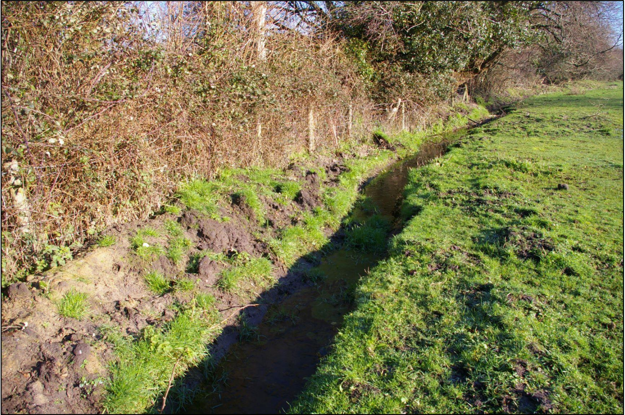
7. MODERN DRAIN (RE)CUT ALONG NORTHERN BOUNDARY OF THE SITE, VIEWED FROM THE SOUTH-WEST.
