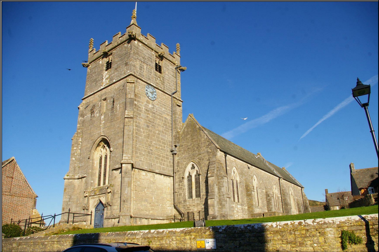
11. ST EDWARD, KING & MARTYR CHURCH, VIEWED FROM THE SOUTH-WEST.
