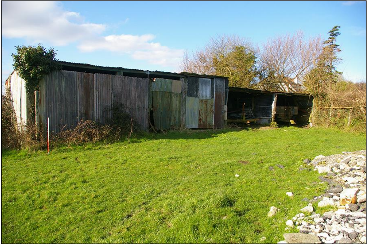
31. DETAIL OF METAL STRUCTURE IN THE NORTH-WEST CORNER OF F3; VIEWED FROM THE SOUTH-EAST (1M SCALE).
