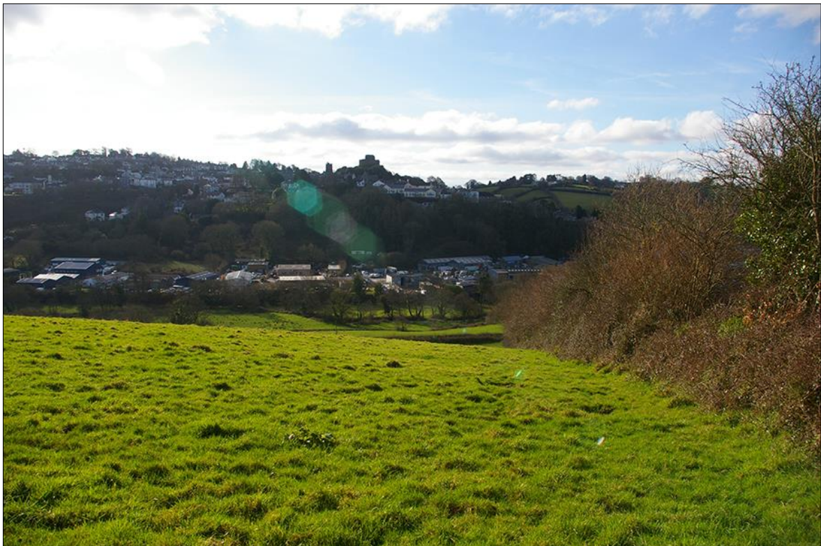
42. VIEW ACROSS F4 TO LAUNCESTON FROM THE NORTH-WEST CORNER, NOTE THE PROMINENCE OF LAUNCESTON CASTLE AND CHURCH OF ST MARY MAGDALENE; VIEWED FROM THE NORTH-EAST (NO SCALE).
