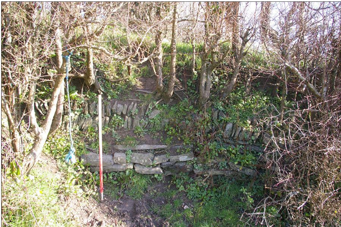
34. DETAIL OF THE STONE FACED HEDGEBANK NORTHERN BOUNDARY OF F4; VIEWED FROM THE SOUTH-WEST (1M SCALE).
