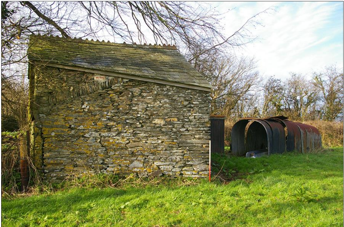
6. SOUTH-EAST ELEVATION OF THE STRUCTURE ALONG THE WESTERN BOUNDARY OF F1, WITH METAL STIES BEHIND; VIEWED FROM THE SOUTH-EAST (1M SCALE).
