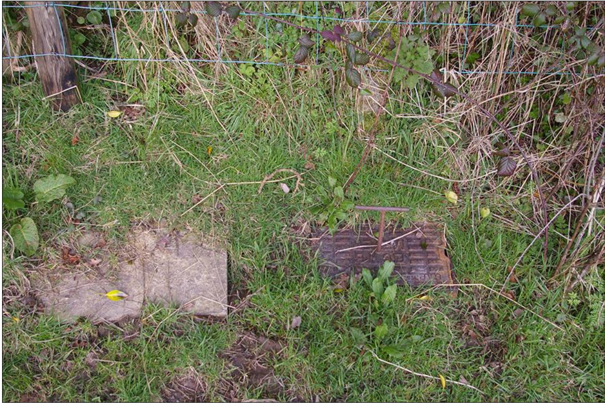
11. DETAIL OF THE MODERN SERVICE MANHOLE COVER IN THE NORTH-WEST CORNER OF F1; VIEWED FROM THE SOUTH-WEST (NO SCALE).
