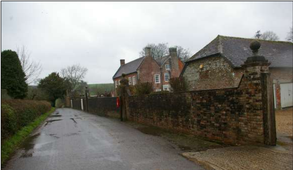
FIGURE 20: THE MANOR, WALLS AND GARAGE AT ALVEDISTON; VIEWED FROM THE SSW.
