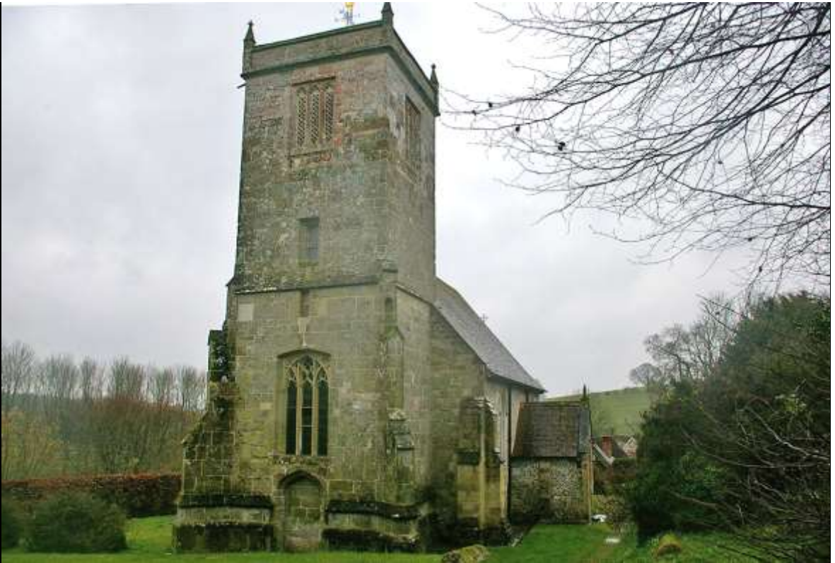
FIGURE 19: EBBESBOURNE WAKE CHURCH: FROM THE WEST-SOUTH-WEST.
