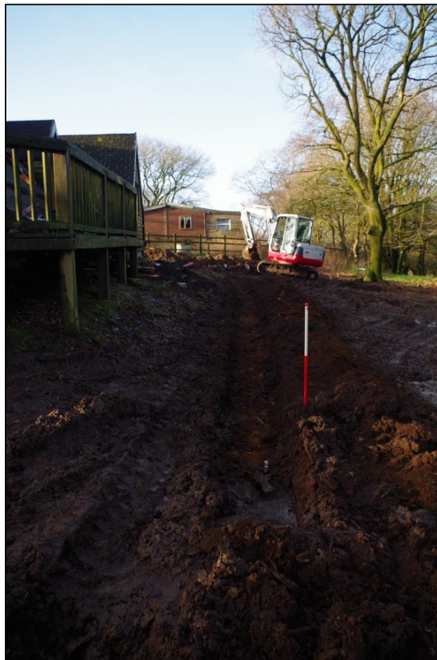
FIGURE 3: NORTHERN PORTION OF TRENCH, VIEWED FROM THE EAST (1M SCALE).
