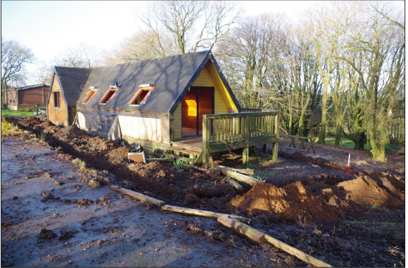
FIGURE 2: WORKS IN PROGRESS, VIEWED FROM THE EAST (1M SCALE).
