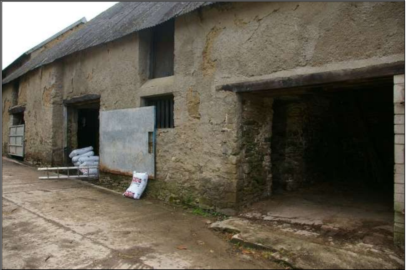
7. EAST FRONT ELEVATION OF B1B; VIEWED FROM THE NORTH-EAST.
