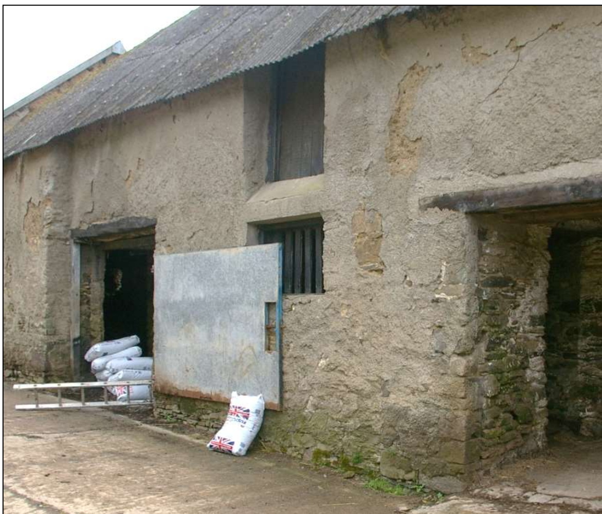
FIGURE 12: WEST ELEVATION OF B1B; VIEWED FROM THE NORTH-EAST. NOTE THE STEP IN THE WALL TO LEFT WHERE B1B ABUTS B1C, AND THE VERTICAL JOINT TO THE CENTRE RIGHT WHERE B1B ABUTS B1A.
