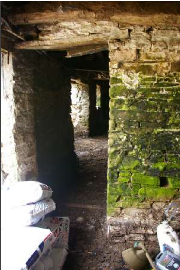
16. LOOKING INTO B1C THROUGH DOOR FROM B1B; VIEWED FROM THE NORTH.
