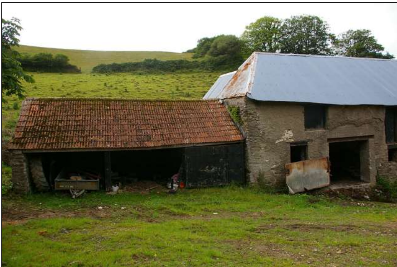
55. IMPLEMENT SHED B2E WITH B2C TO RIGHT; VIEWED FROM THE EAST.
