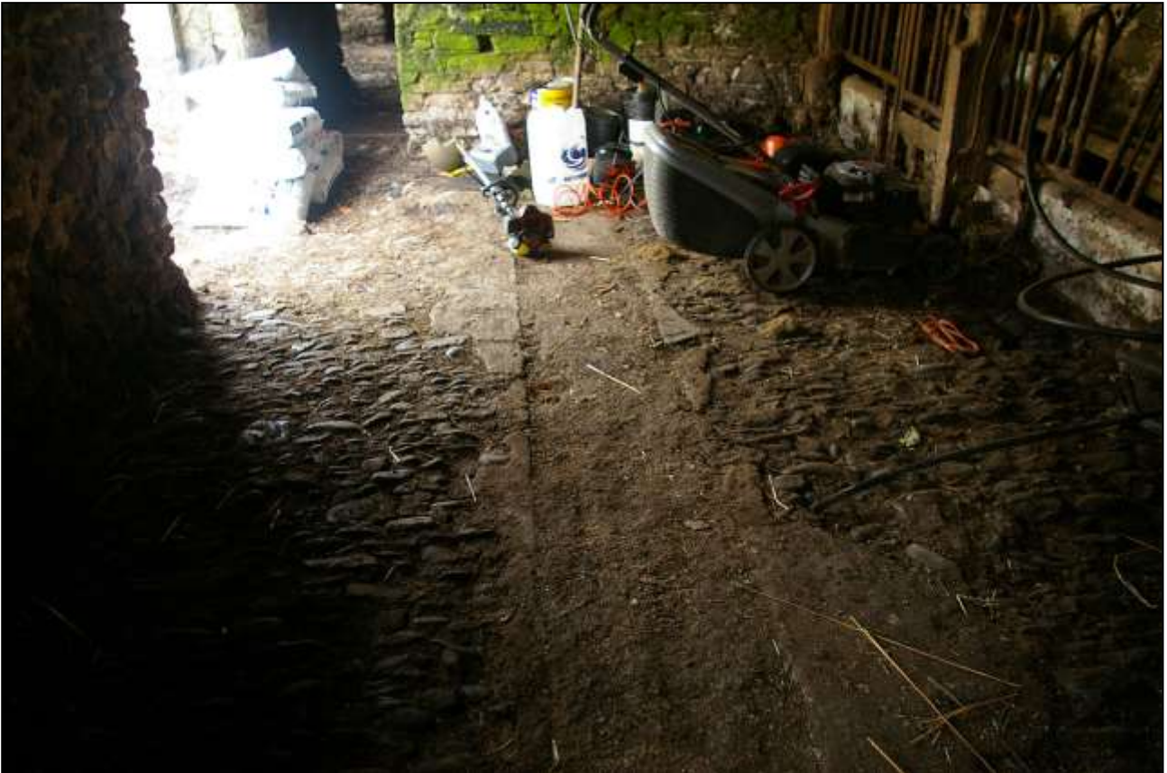
12. COBBLED FLOOR WITH CENTRAL DRAIN IN B1B, MANGER ON RIGHT WITH 20 TH CENTURY STEEL RESTRICTIVE RAILS; VIEWED FROM THE NORTH.
