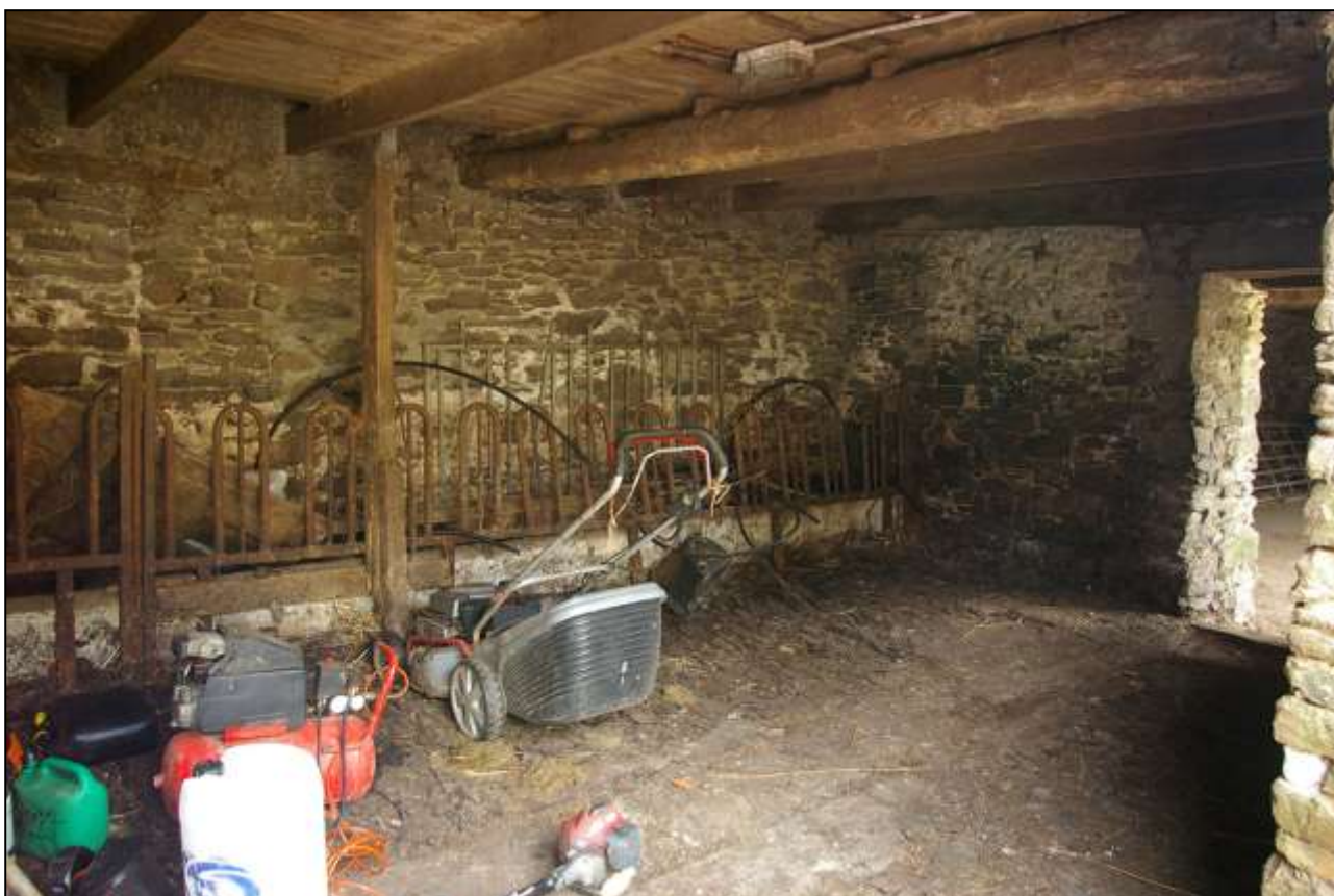
14. THE GROUND FLOOR OF B1B, NOTE BLOCKED DOOR ON LEFT AND 19 TH /20 TH CENTURY MANGER BLOCKING IT; VIEWED FROM THE SOUTH-EAST.
