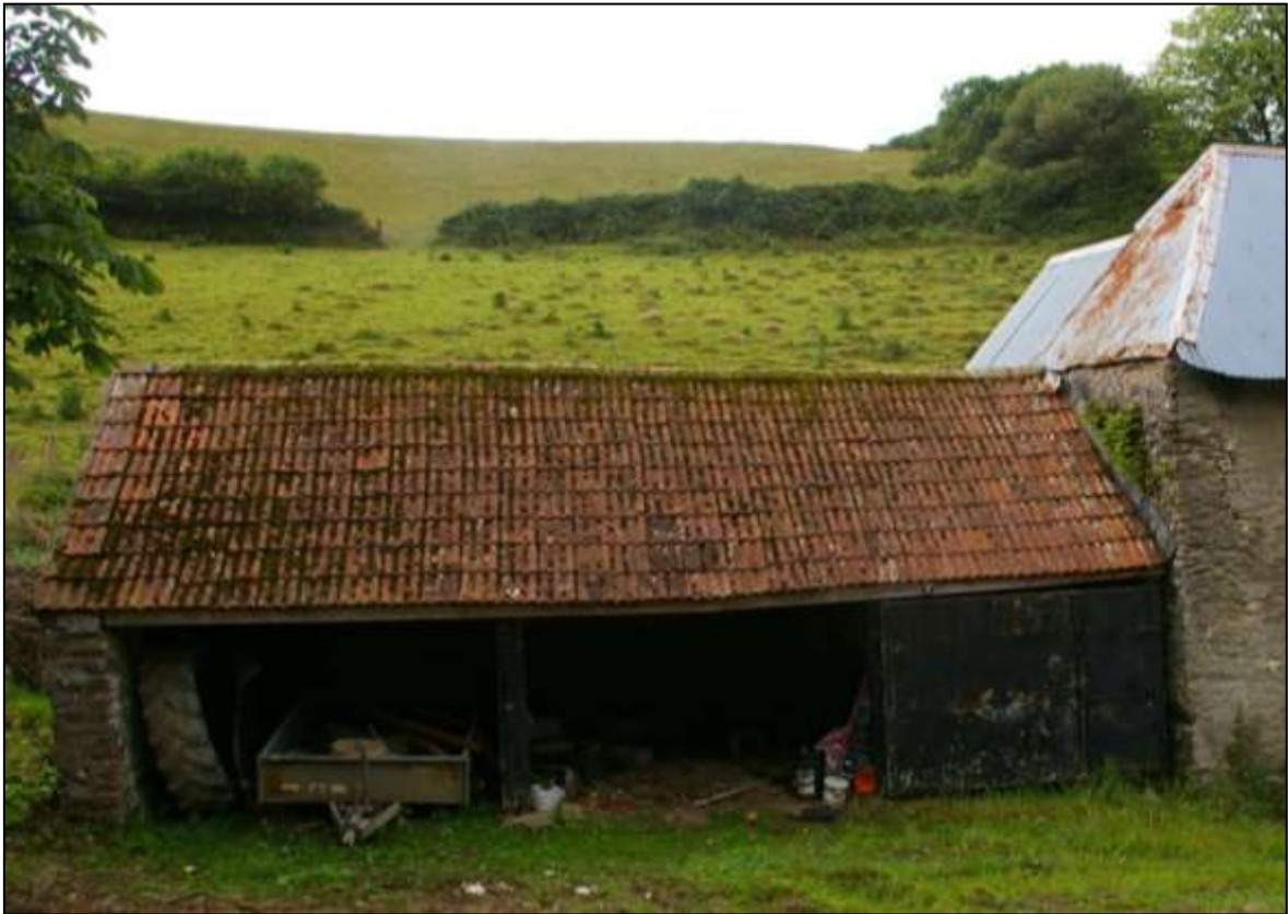
FIGURE 27: EAST FRONT OF IMPLEMENT SHED B2E, WITH B2C TO RIGHT.
