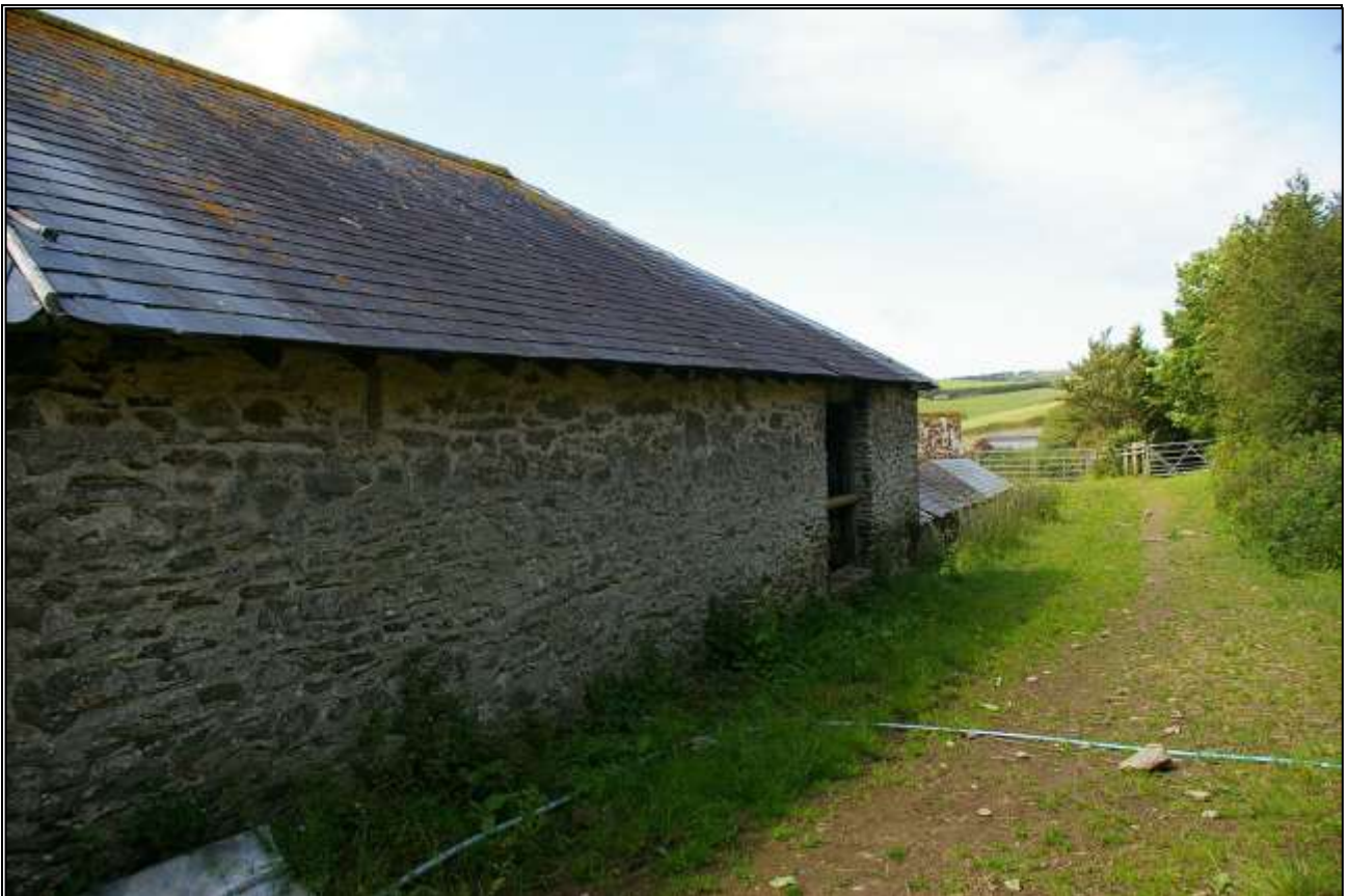
62. THE EAST WALL OF B3a AS REBUILT WHEN THE HORSE ENGINE HOUSE WAS CONSTRUCTED; VIEWED FROM THE SOUTH-EAST.
