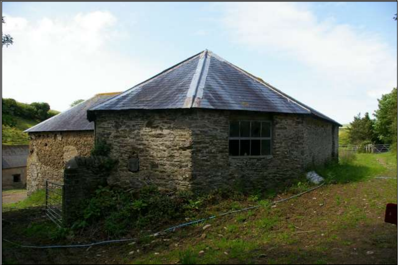
61. B3b. NOTE THE END OF THE AXIAL SUPPORT BEAM IN THE WALL-FACE TO THE LEFT. 20 TH CENTURY CRITTALL-STYLE WINDOWS IN THE OLDER VENTILATION OPENING. VIEWED FROM THE SOUTH-EAST.
