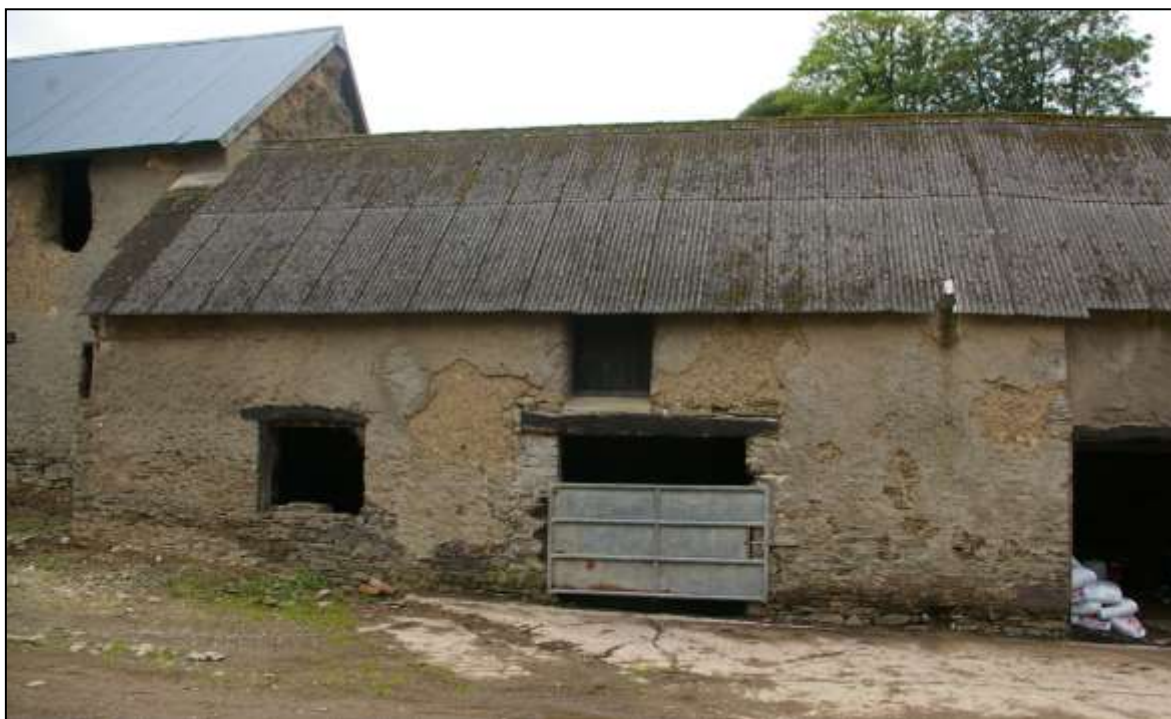
FIGURE 15: EAST ELEVATION OF B1C; VIEWED FROM THE EAST.
