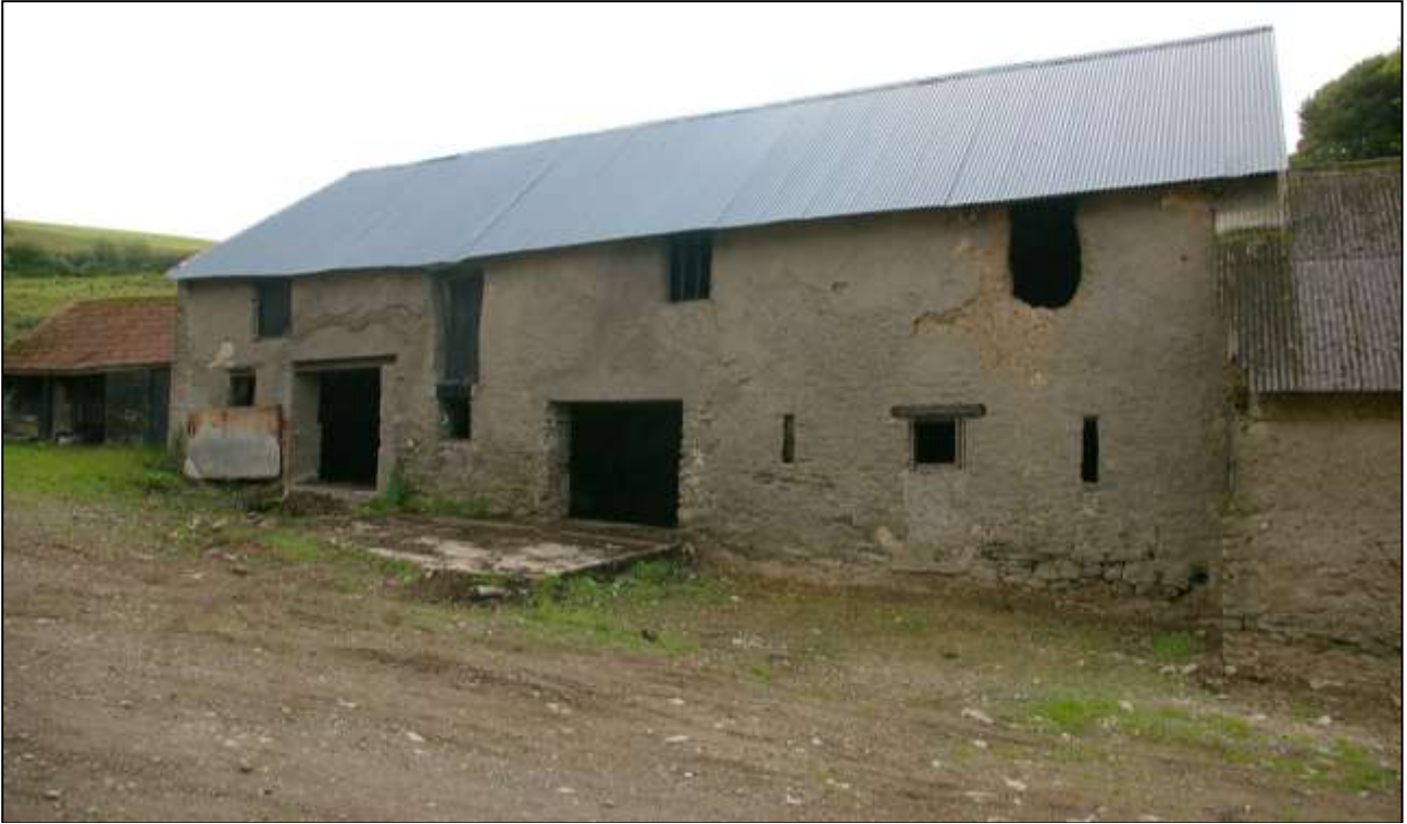
28. THE FRONT EAST ELEVATION OF BUILDING 2; VIEWED FROM THE NORTH-EAST.
