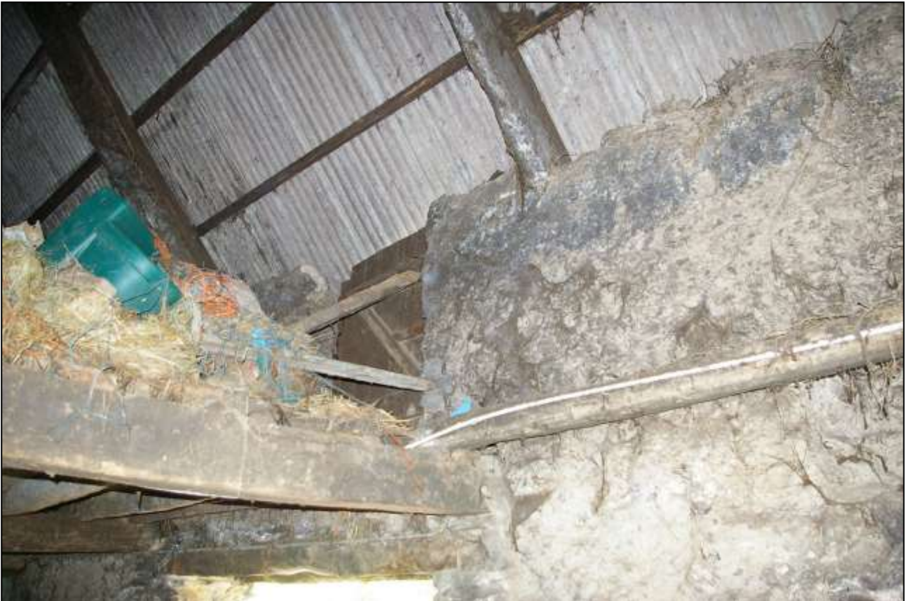
26. THE EAST WALL OF B1c SHOWING LOADING DOOR AND TRACES OF GREY PAINT AND WHITEWASH, WITH PAINTED SOFFITS AND SIDES OF BLADES UP TO FORMER COLLAR LEVEL; VIEWED FROM THE SOUTH-WEST.
