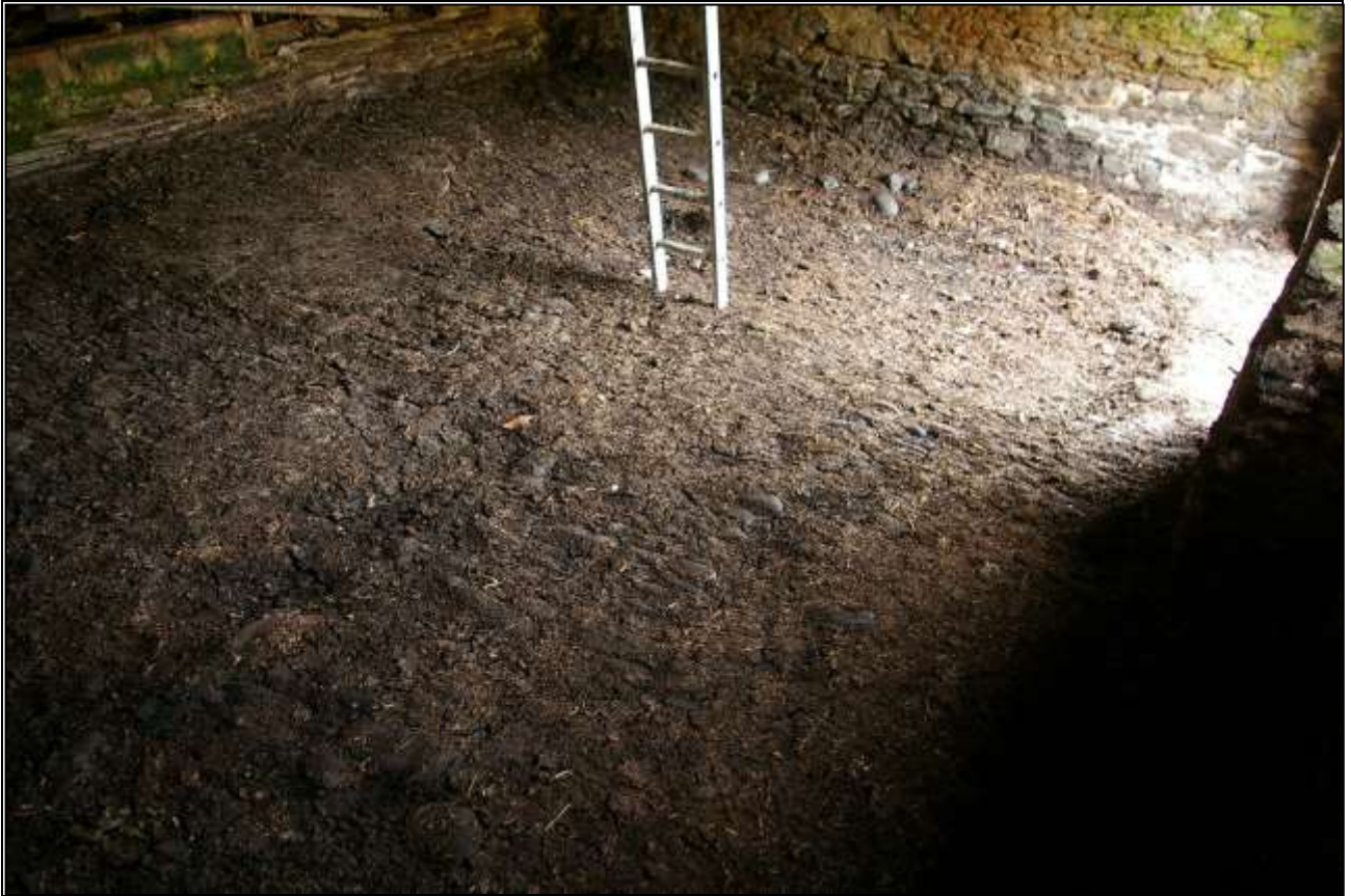
49. DETAIL OF THE COBBLED FLOOR IN B2C; VIEWED FROM THE SOUTH-EAST.
