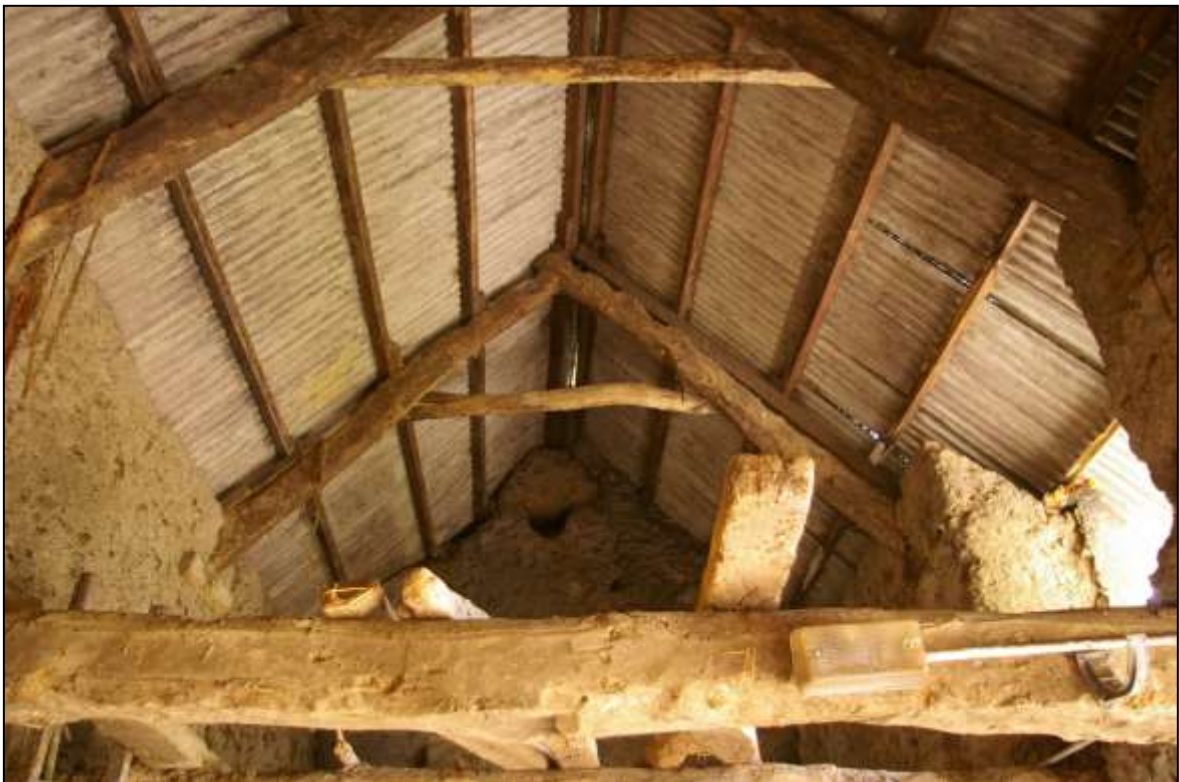
FIGURE 11: THE ROOF STRUCTURE IN B1A; VIEWED FROM THE SOUTH.
