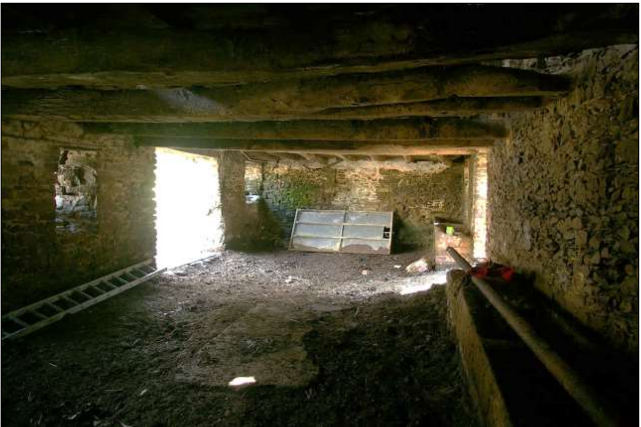
31. GROUND FLOOR OF B2A , WITH REMAINS OF A CONCRETE FLOOR AND DRAIN TO CENTRE LEFT; VIEWED FROM THE NORTH.
