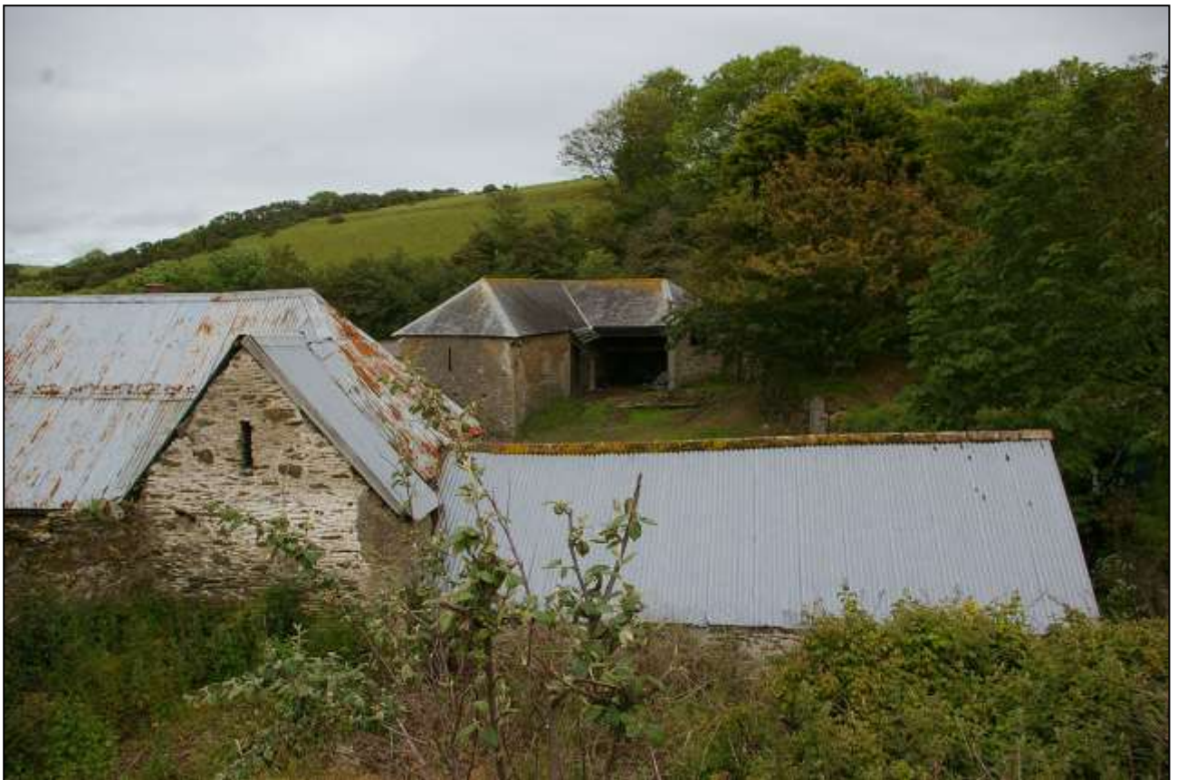
52. VIEW ACROSS BUILDING 2 TO BUILDING 3 IN THE BACKGROUND; VIEWED FROM THE SOUTH-WEST.
