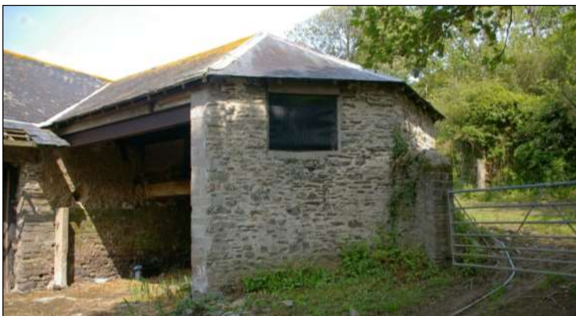
FIGURE 31: HORSE ENGINE HOUSE B3B; VIEWED FROM THE SOUTH-WEST.
