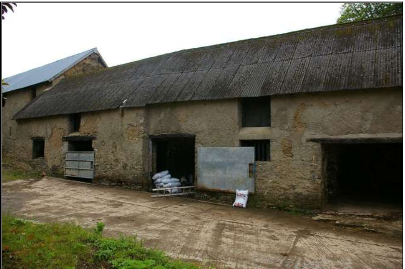
8. EAST FRONT ELEVATIONS OF B1B (CENTRE RIGHT) AND B1C (LEFT); VIEWED FROM THE NORTH-EAST.
