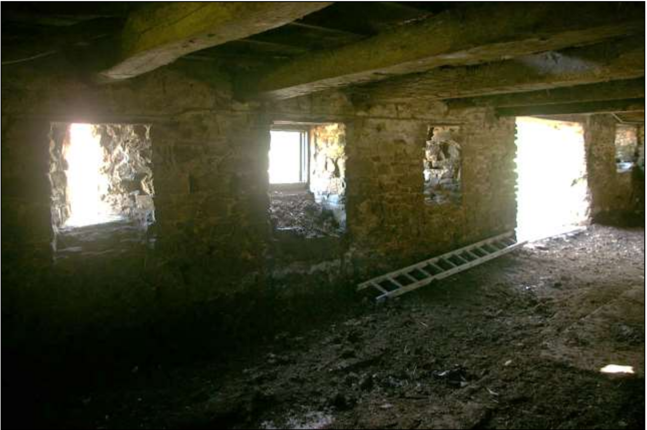
30. SLIT VENTS AND BLOCKED DOOR INSIDE B2A; VIEWED FROM THE NORTH-WEST.
