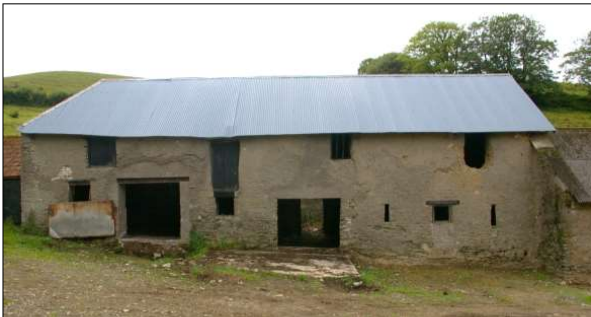
FIGURE 18: EAST FRONT OF BUILDING 2, VIEWED FROM THE EAST.
