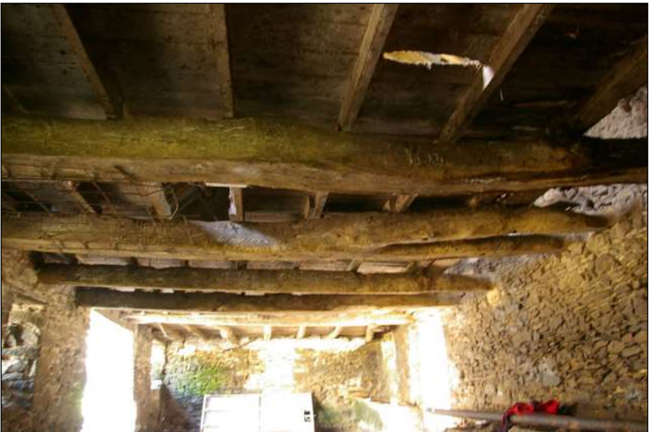
33. HEAVY BEAMS SUPPORTING THE LOFT IN B2A; VIEWED FROM THE NORTH.
