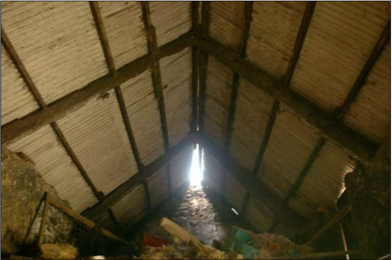
22. ROOF STRUCTURE OVER B1C; VIEWED FROM THE SOUTH.
