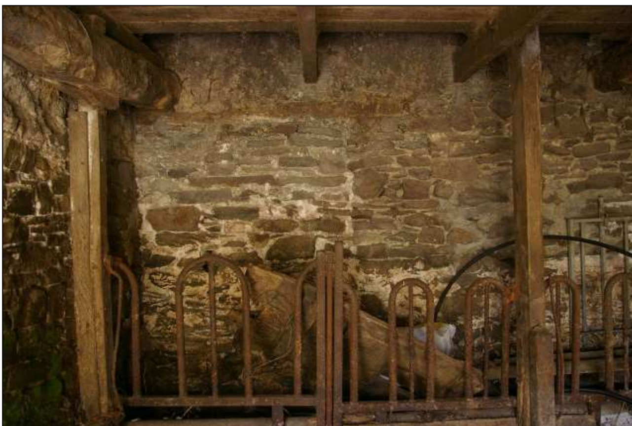
15. BLOCKED PRIMARY DOOR IN THE WEST WALL OF B1B WITH LATER MANGER AND STALL DIVISION POST IN FRONT; VIEWED FROM THE WEST.
