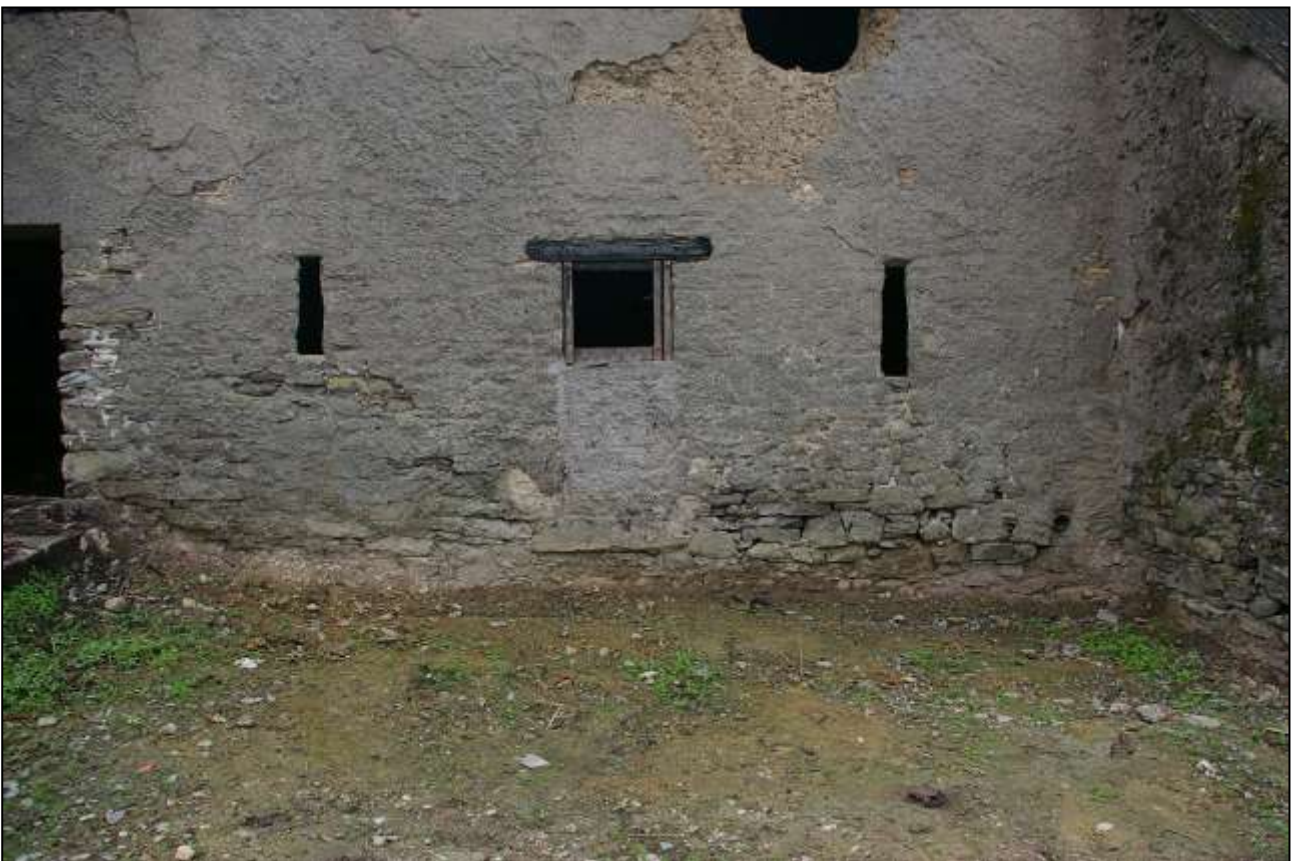
29. BLOCKED DOORWAY AND FLANKING SLIT VENTS IN THE EAST WALL OF B2A, WITH A LARGE HOLE IN THE COB TO TOP RIGHT A VERY WORN PITCHING HATCH; VIEWED FROM THE EAST.
