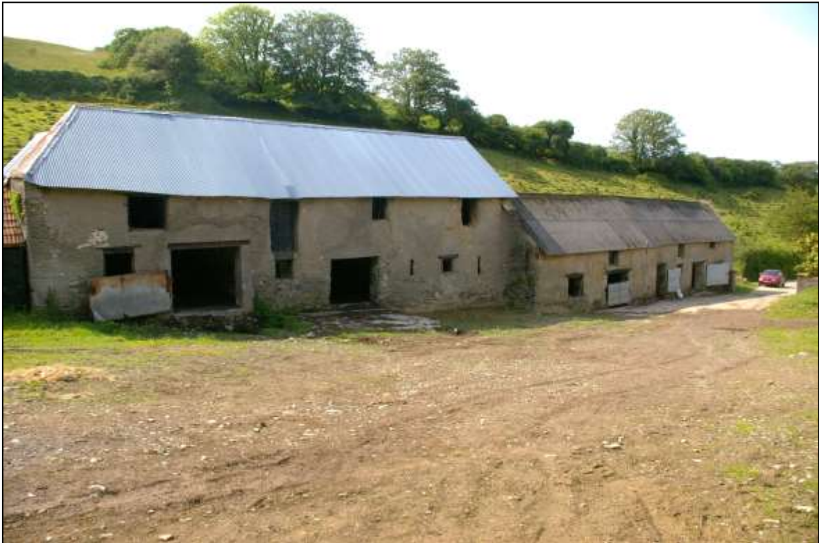
FIGURE 6: B1 (RIGHT) AND B2 (LEFT); VIEWED FROM THE SOUTH-EAST.
