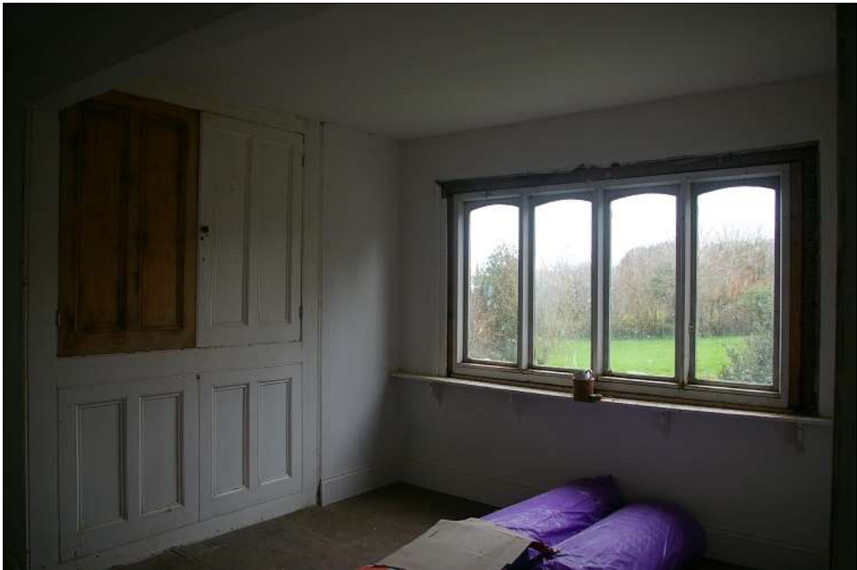
47. DETAIL OF THE PROJECTING STAIR PROJECTION, WITH PAIRS OF LINEN CUPBOARDS AND BRACKETED SHELF UNDER THE WINDOW; FROM THE NORTH-WEST.
