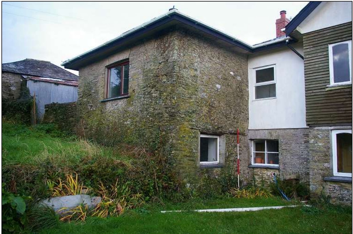
FIGURE 5: THE WEST WING OF TREVEDDA, WITH 2M SCALE; FROM THE EAST-SOUTH-EAST.
