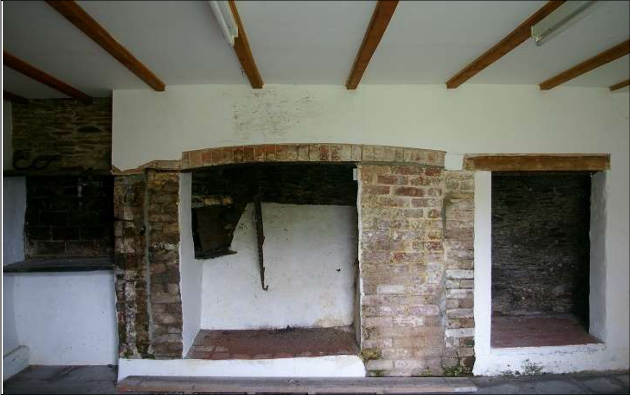
30. THE LATERAL STACK IN R7A; FROM THE EAST.
