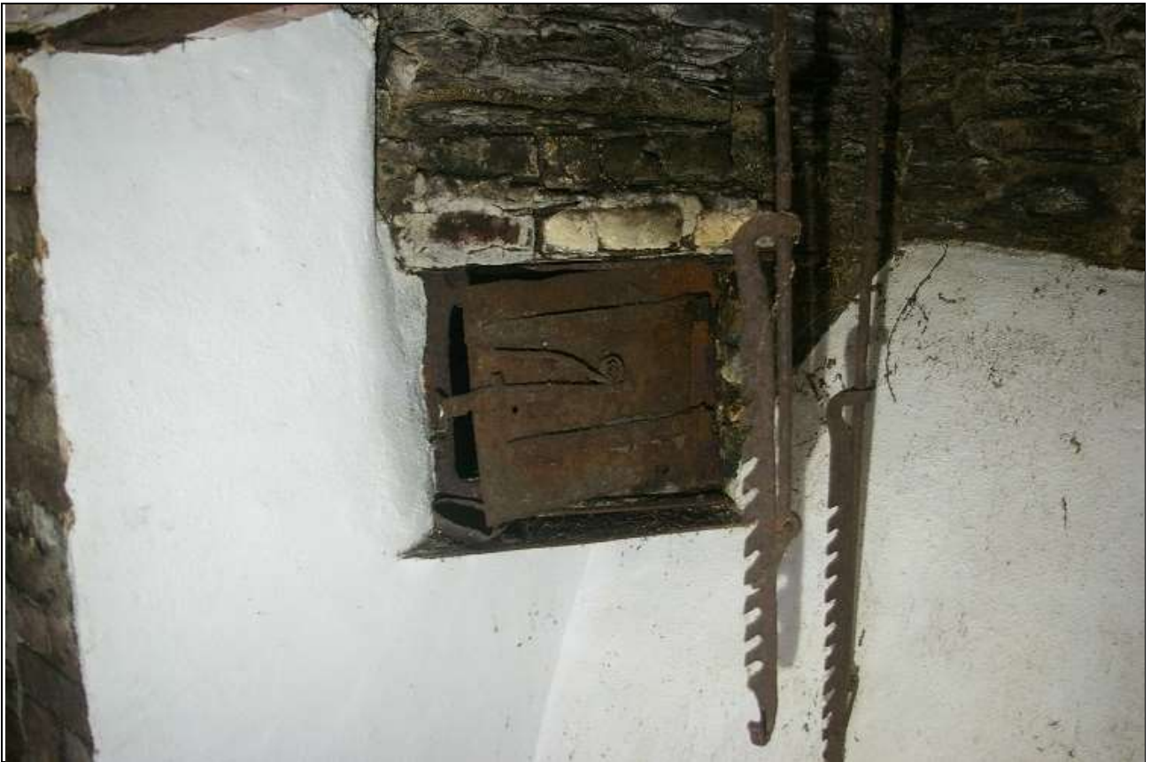
29. THE BREAD OVEN IN THE STACK IN R7A, ALSO POT HANGERS; FROM THE NORTH-EAST.
