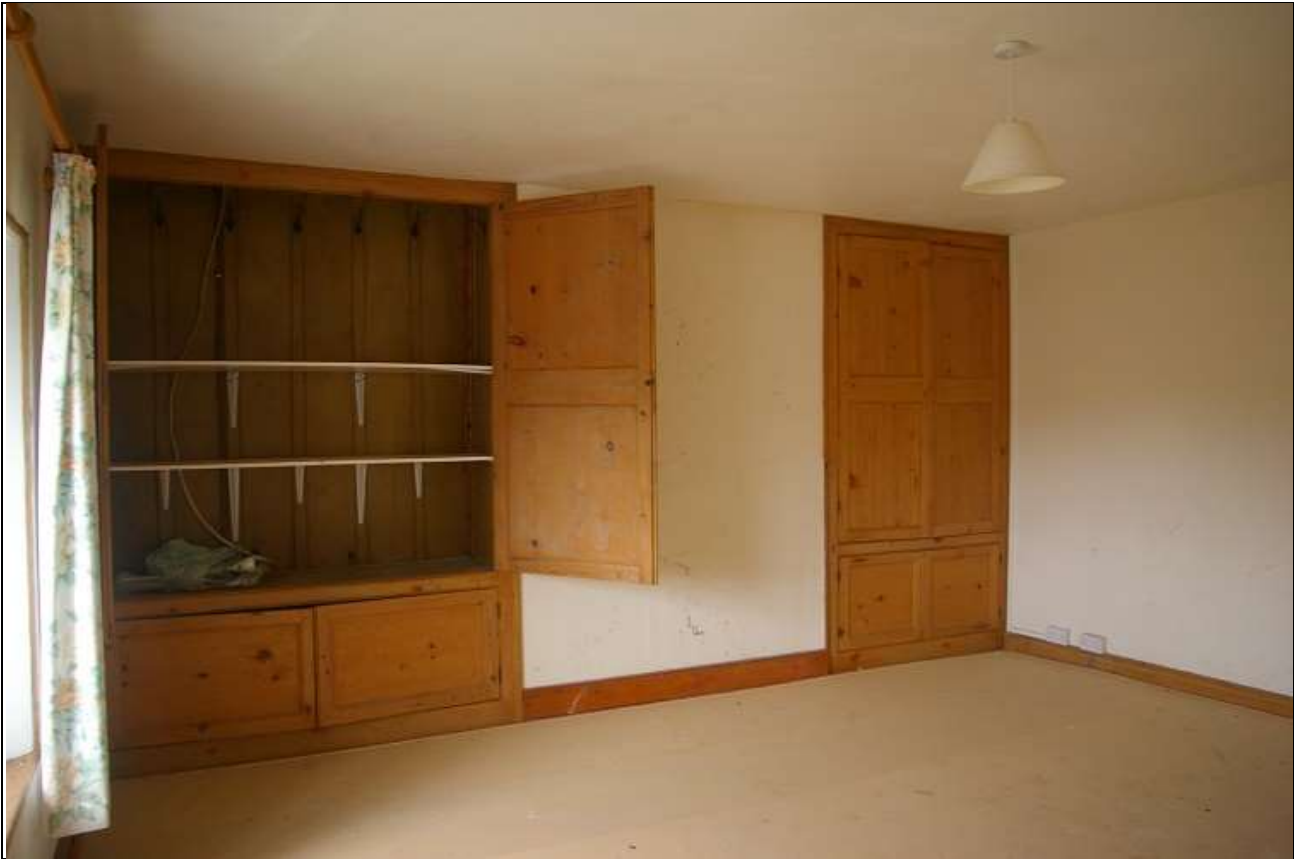
42. THE WIDE DEEP CUPBOARDS IN R12, LINED IN WOOD; FROM THE NORTH-WEST.
