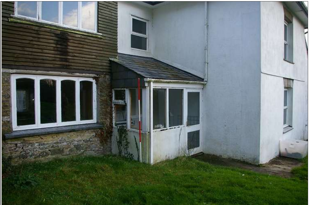
73. THE SUNROOM IN THE ANGLE WITH THE EAST WING, 2M SCALE; FORM THE SOUTH-WEST.
