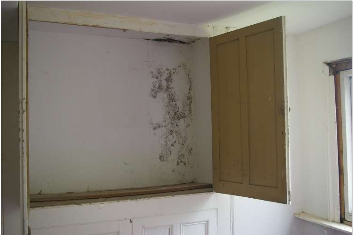
48. INTERIOR OF THE LINEN CUPBOARDS; FROM THE NORTH-WEST.
