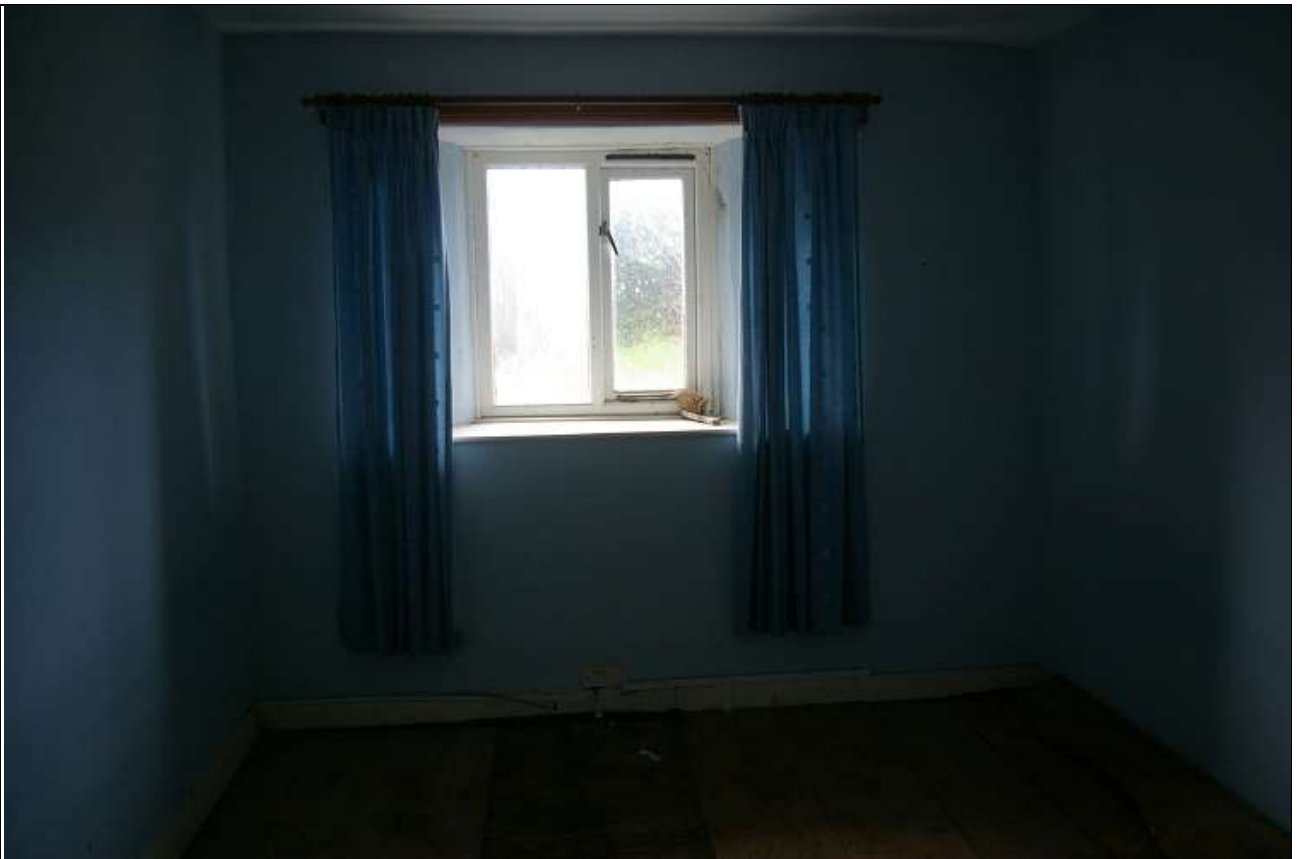
57. R16, A SMALL ROOM FORMED FROM LATH AND PLASTER PARTITIONS, LIT BY A SMALL WINDOW IN THE WEST WALL; FROM THE EAST.
