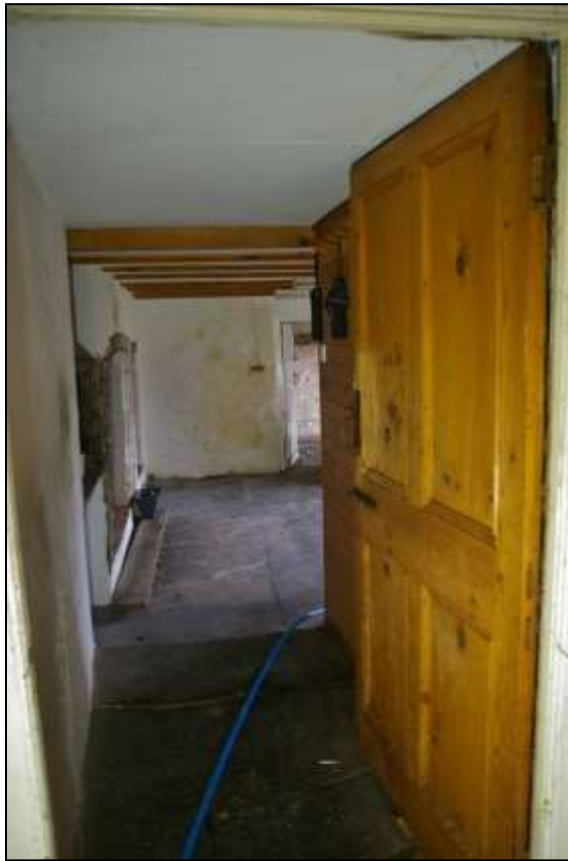
FIGURE 15: VIEW INTO THE REAR SERVICE WING, SHOWING THE LATERAL STACK AND SHORT PASSAGE WITH THICK WALLS AND WORN SLATE FLOOR; FROM THE SOUTH.
