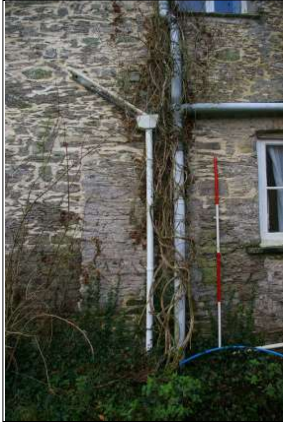
76. THE BLOCKED REAR CROSS PASSAGE DOOR IN THE NORTH WALL OF THE MAIN RANGE, WITH GOOD SLAB QUOINS AND CURVING OAK LINTEL, 2M SCALE; FROM THE NORTH.
