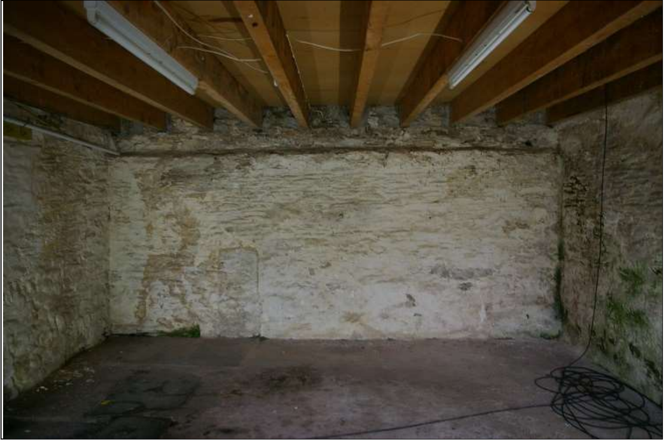
32. THE WEST WALL OF R8, WITH LEDGE FOR FORMER LOFT, MUCH LOWER THEN CURRENT FLOOR; FROM THE EAST.
