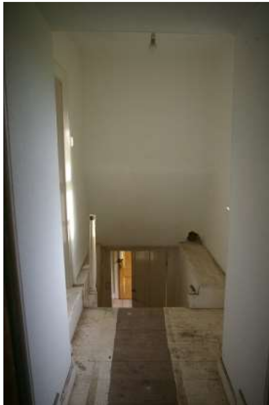
59. LOBBY INTO R9B THE WEST STAIRS; FROM THE WEST.
