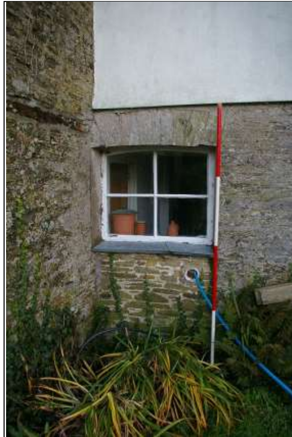
72. BLOCKED DOOR IN THE SOUTH WALL OF THE CENTRAL MAIN RANGE, IN AN 18 TH /19 TH WALL, WITH 2M SCALE, LEADING INTO THE WEST LOBBY AND KITCHEN R2A BEYOND; FROM THE SOUTH-SOUTH-EAST.
