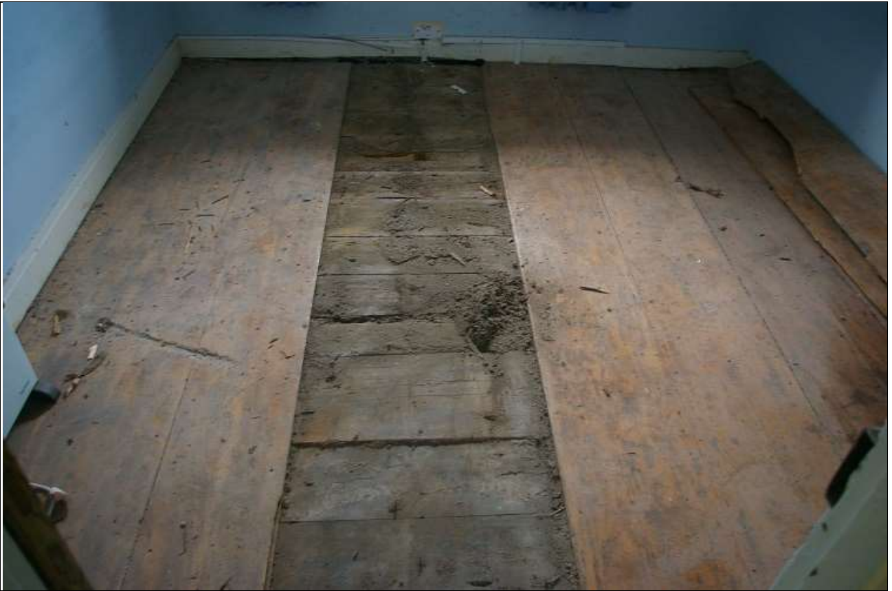
56. THE FLOOR IN R16, REUSED 17 TH CENTURY OR EVEN LATER 16 TH CENTURY BOARDS, RE-LAID OVER AN EARLIER FLOOR OF A MIX OF EVEN WIDTH AND WIDE BOARDS; FROM THE EAST.
