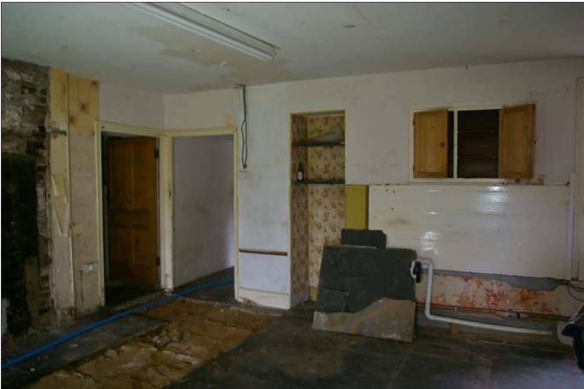
4. THE WEST END OF THE NORTH WALL, WITH A SERIES OF OPENINGS FOR CUPBOARDS SET INTO A POTENTIAL AREA OF BLOCKING, WITH DOORS TO SERVICE AND REAR SERVICE WING; FROM THE SOUTH-EAST.
