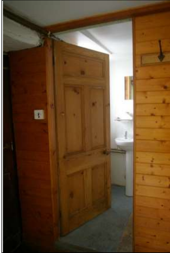
28. SMALL BOARDED PARTITIONS FORM A BATHROOM IN THE CORNER OF R7A, A SMALL ROOM, R7B; FROM THE NORTH-WEST.
