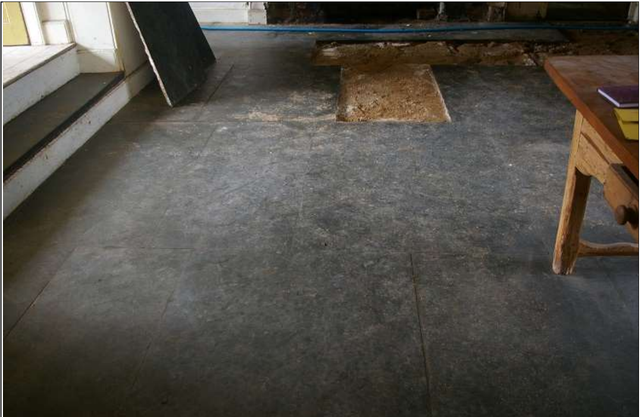
8. THE FINE SLATE FLAGSTONE FLOOR IN R2A; FROM THE EAST.
