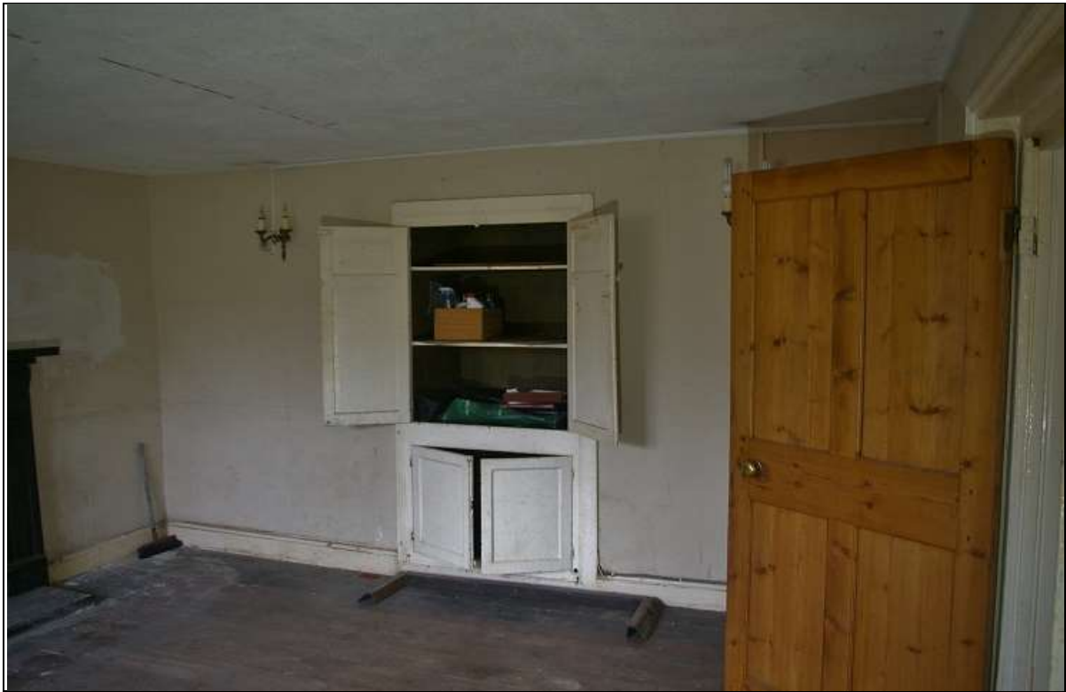
FIGURE 13: THE PARLOUR, WITH BLOCKED DOOR TO SOUTH, NOW SET WITH A PANELLED CUPBOARD; FROM THE NORTH-WEST.
