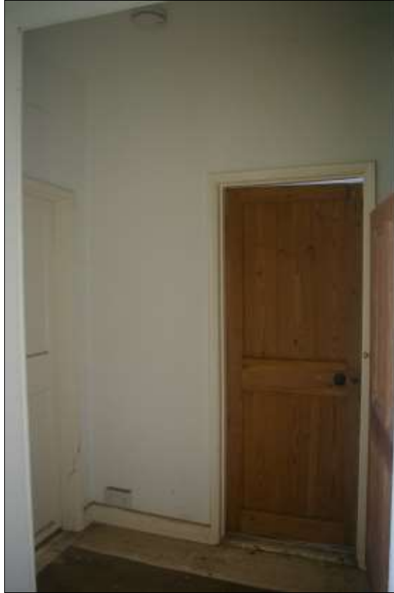
58. THE LOBBY R14; FROM THE EAST, SHOWING DOORS TO R15, R16 AND SMALL CUPBOARD FORMED AGAINST BLOCKED DOOR TO R18, TO THE NORTH.
