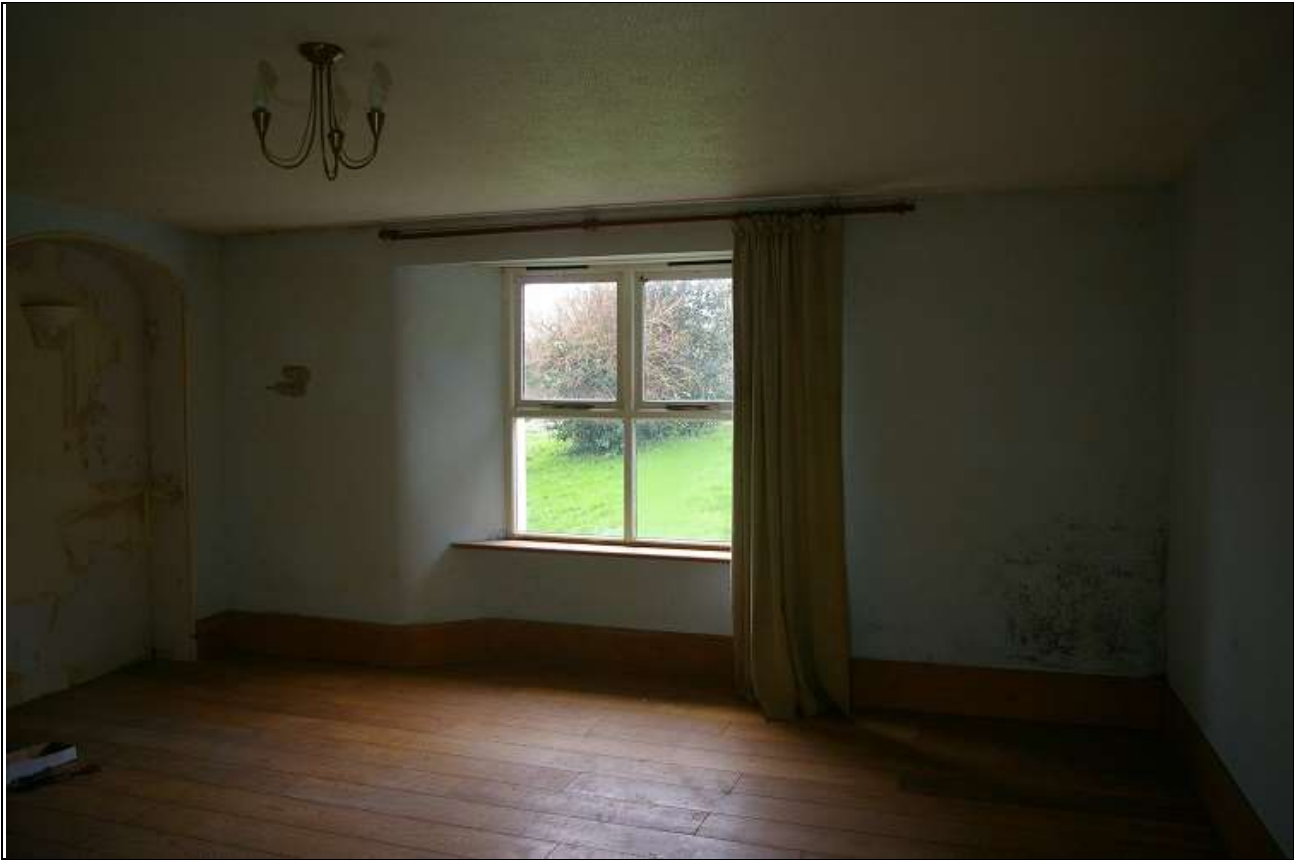
14. THE DRAWING ROOM WITH MODERN REPLACEMENT WINDOW; FROM THE NORTH-WEST.
