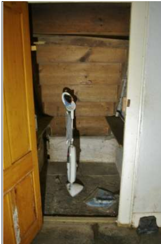
2. UNDER STAIR CUPBOARD; FROM THE EAST.
