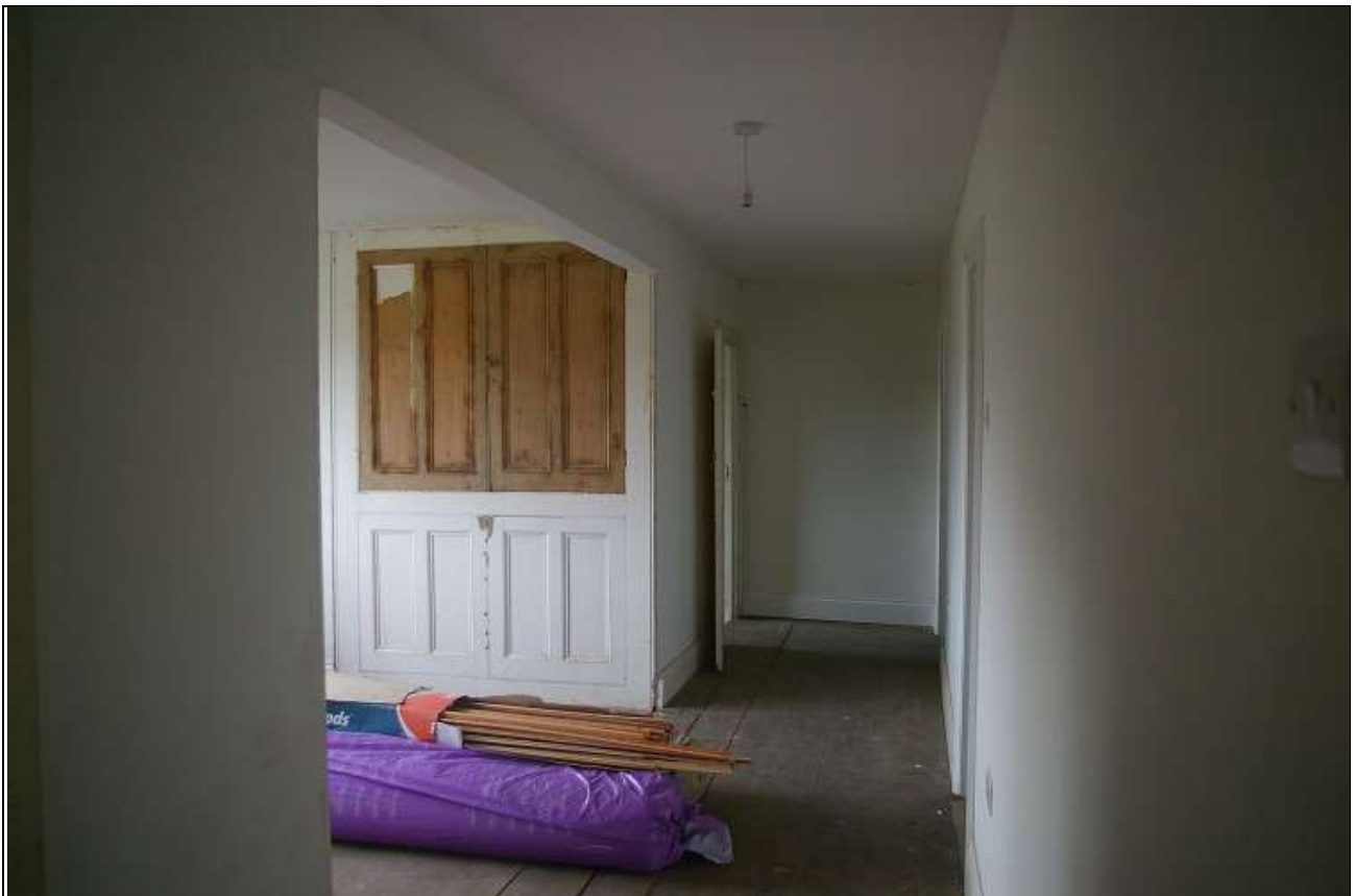
45. R10, THE LANDING WHICH LINKS THE EAST AND WEST WINGS AND REAR WING, CORRIDOR FORMED FROM LATH AND PLASTER PARTITIONS; FROM THE EAST.
