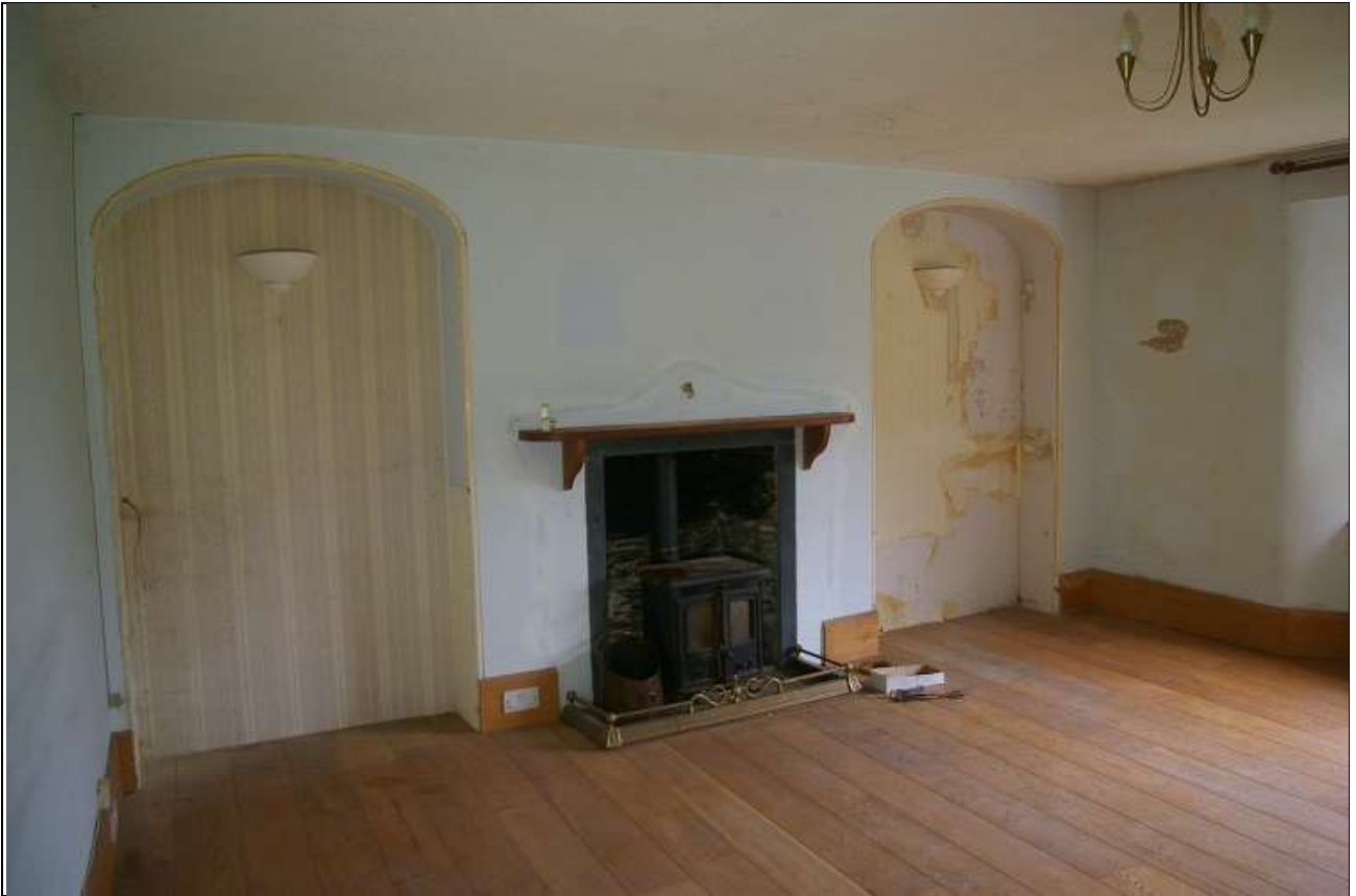
12. ROOM 3, THE DRAWING ROOM, WITH BASKET ARCH ALCOVES, THE FIREPLACE MUCH ALTERED; FROM THE WEST-NORTH-WEST.
