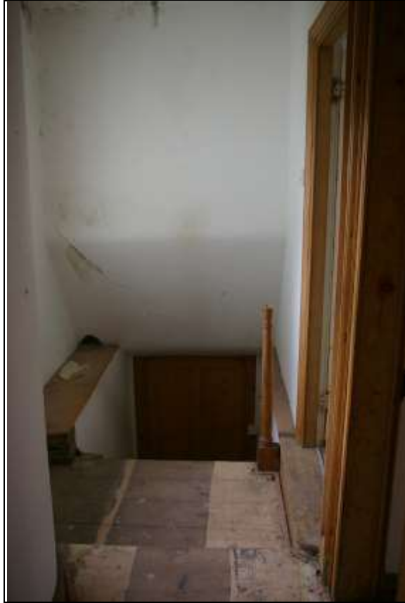
36. THE EASTERN STAIR LOBBY, R9A; FROM THE EAST.
