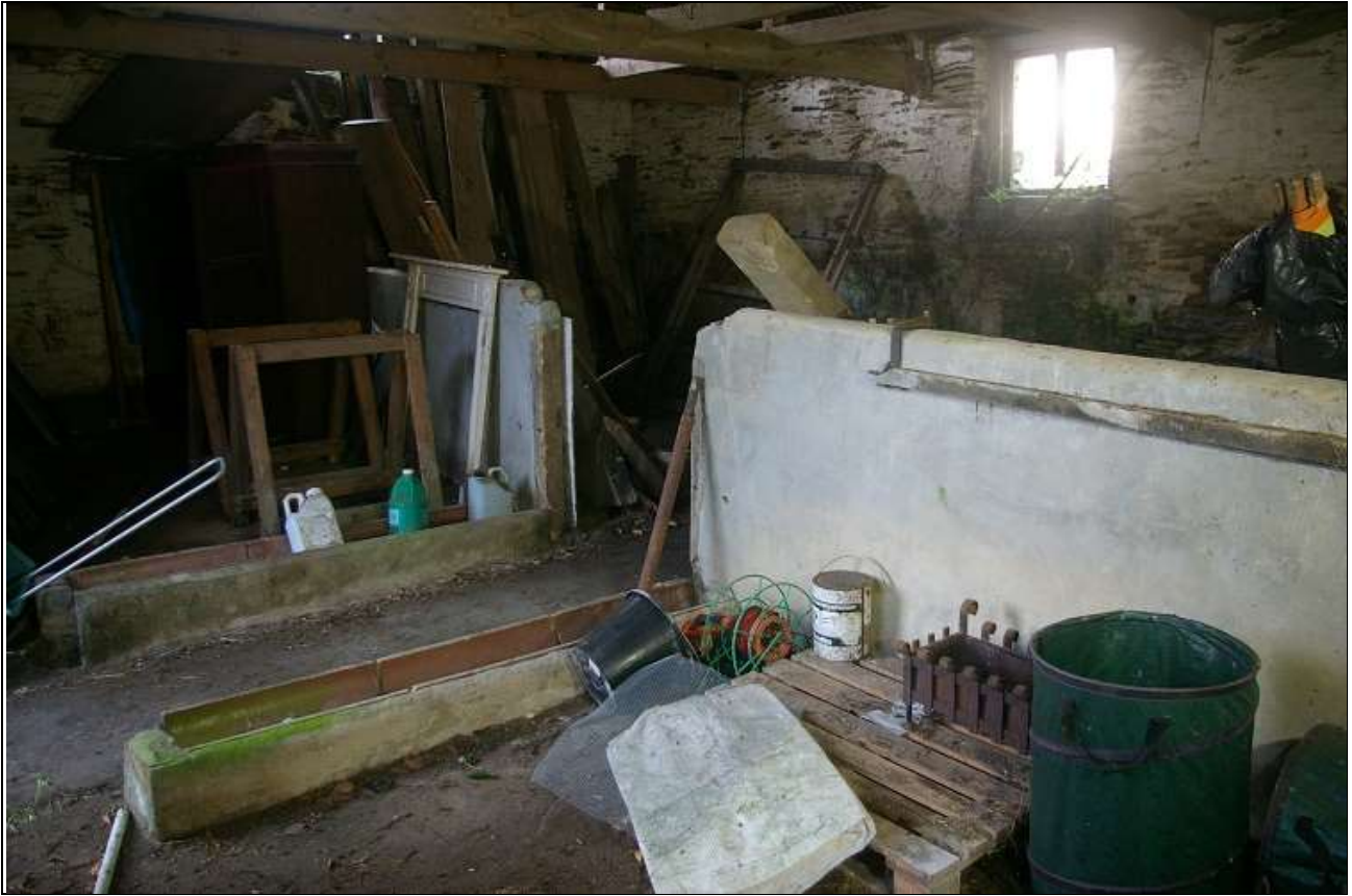
92. THE INTERIOR OF THE STABLES, DIVIDED INTO CONCRETE PENS, NOTE THE STORAGE OF A FINE MANTLED FIRE SURROUND, POSSIBLY FROM R12, WHICH SHOWS A SCAR OF ONE HAVING BEEN REMOVED; FROM THE NORTH-WEST.
