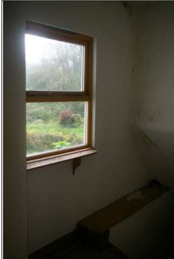
37. WINDOW WITH BRACKETED SHELF IN R9A; FROM THE EAST-NORTH-EAST.
