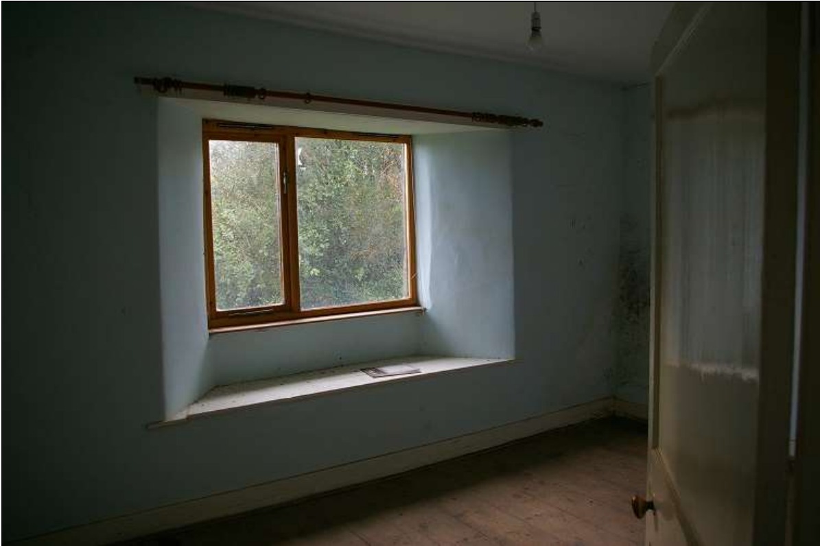
52. R15, WITH LARGE WINDOW IN SOUTH WALL, WITH PLANK WINDOW SEAT AND GOO TWO PANEL DOOR FORM THE LOBBY, R14; FROM THE NORTH-EAST.
