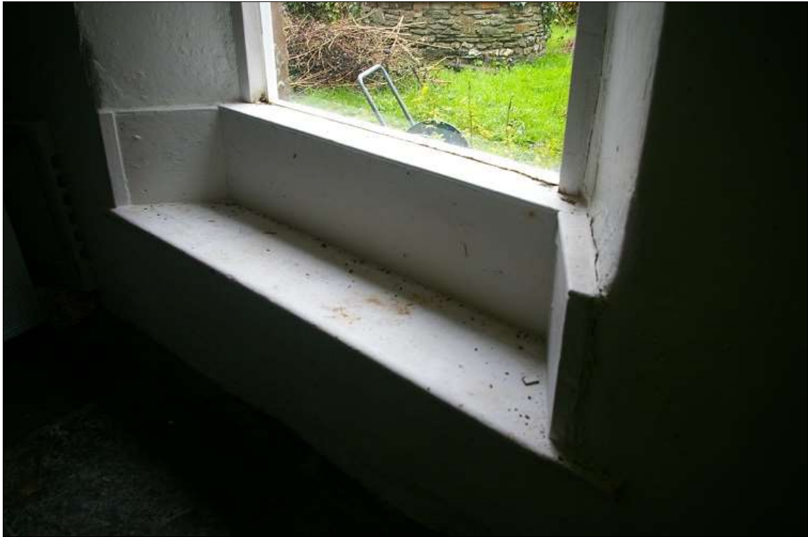
27. THE PLANK BEADED WINDOW SEAT IN R7A; FROM THE SOUTH-WEST.
