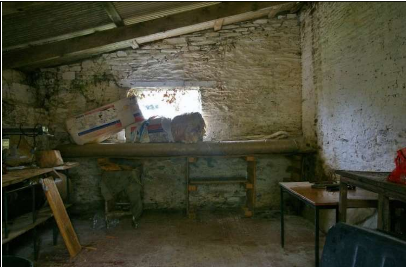
85. THE INTERIOR OF OB2; FROM THE NORTH.
