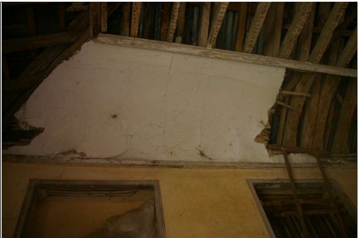
10. THE CAVETTO EAVES TO THE VAULTED CEILING; FROM THE EAST-SOUTH-EAST.
