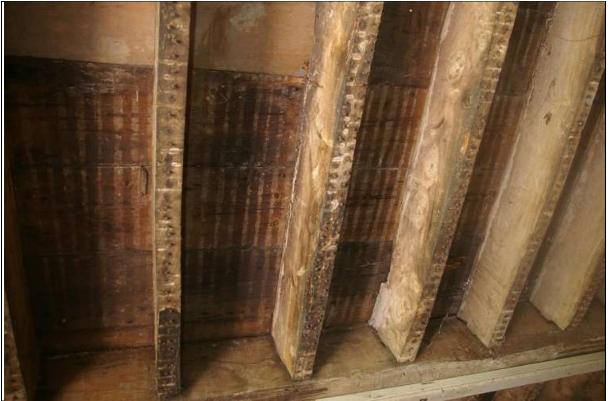
25. THE JOISTS AND REUSED WIDE PLANKS OF THE FLOOR OF THE LOFT IN ELEMENT B; FROM THE SOUTH-EAST.
