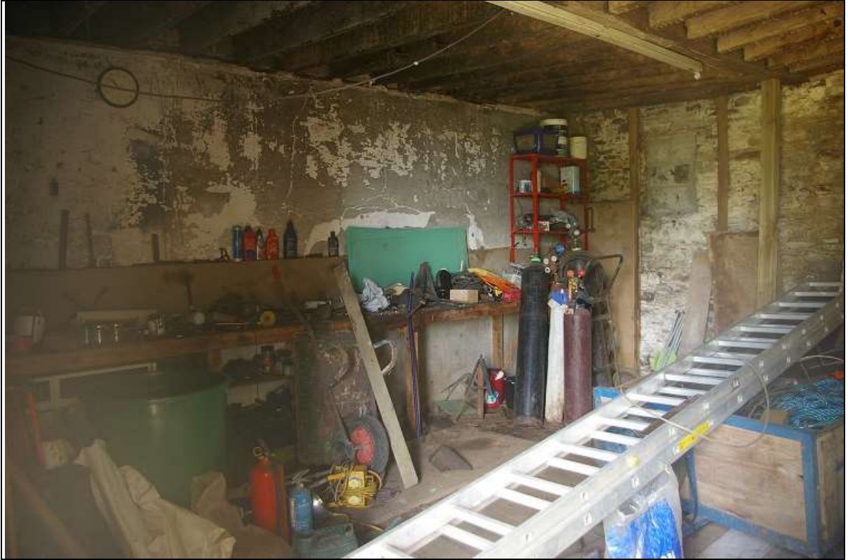
23. THE PLASTERED PARTITION WALL IN ELEMENT B, ROOM 2; FROM THE SOUTH-EAST.
