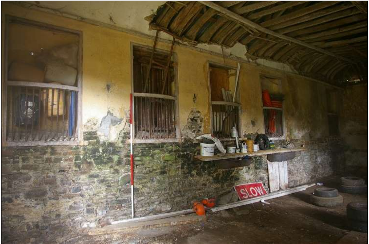
FIGURE 10: THE TROUGHS AND FEED BOXES, WITH HAYRICKS DEVELOPED IN ELEMENT A OF THE BUILDING TO THE WEST IN THE 19 TH CENTURY (2M SCALE).
