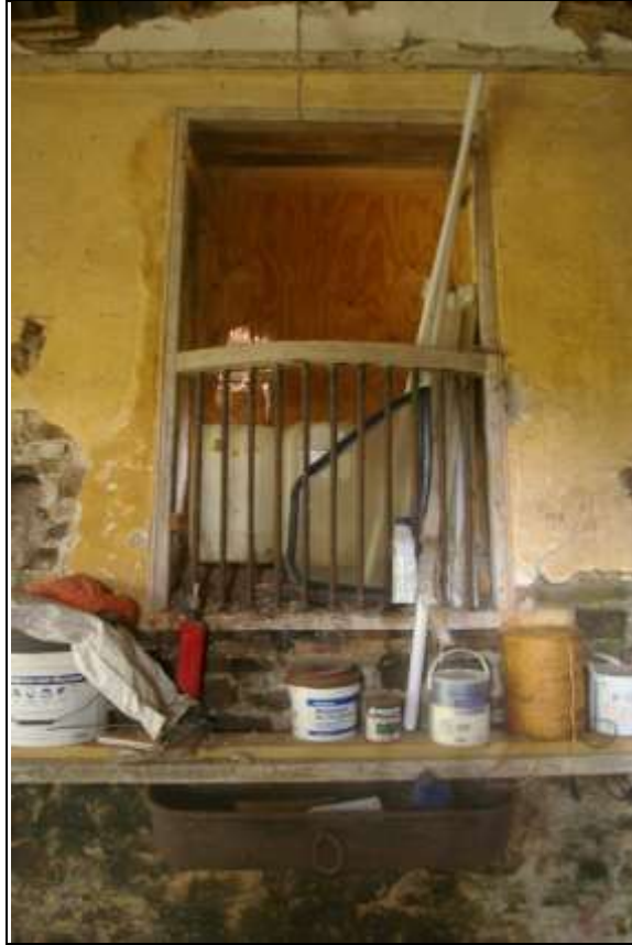
11. ONE OF THE HAY-BOXES, WITHIN ITS FRAMED ALCOVE, WITH A CAST IRON FEEDER TROUGH BENEATH; FROM THE EAST.
