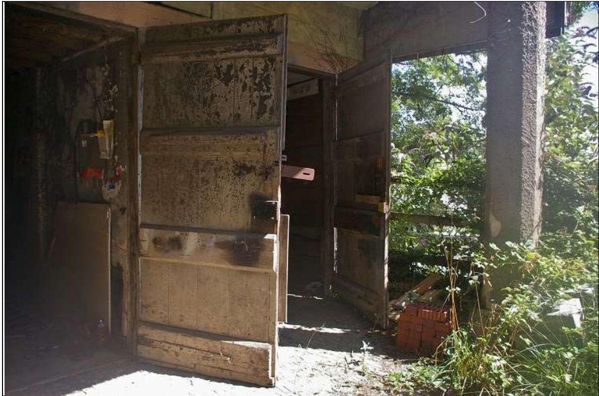
20. THE DOORS RESET AND REUSED IN ELEMENT B; FROM THE WEST-SOUTH-WEST.
