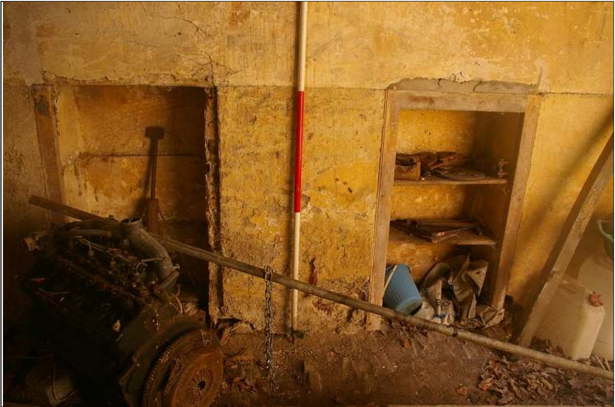
9. THE TWO FRAMED CUPBOARDS IN THE EAST WALL OF THE STABLES, WITH 2M SCALE; FROM THE WEST.
