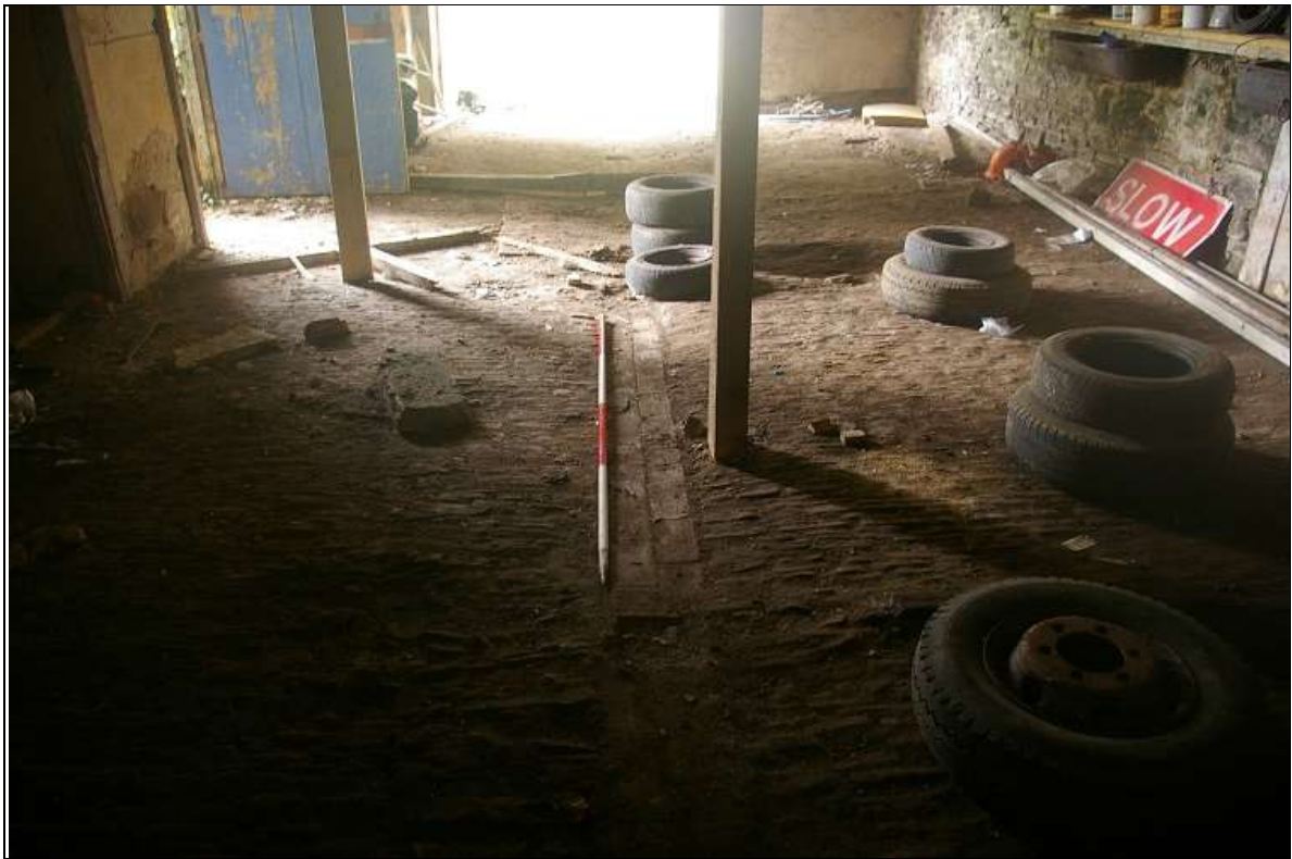
14. THE COBBLED FLOOR OF ELEMENT A, WITH 2M SCALE; FROM THE NORTH.
