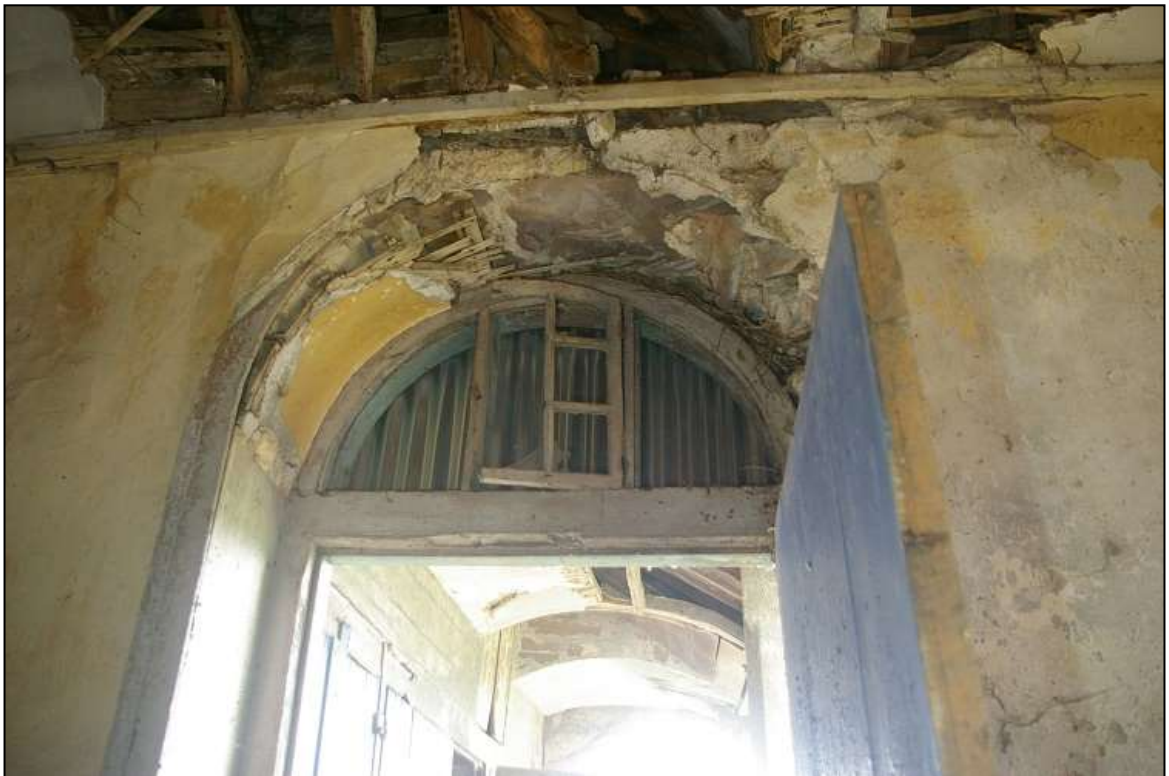
18. THE ROUND HEADED DOORWAY, WITH FANLIGHT, INCLUDING CASEMENT WINDOW; FROM THE WEST.
