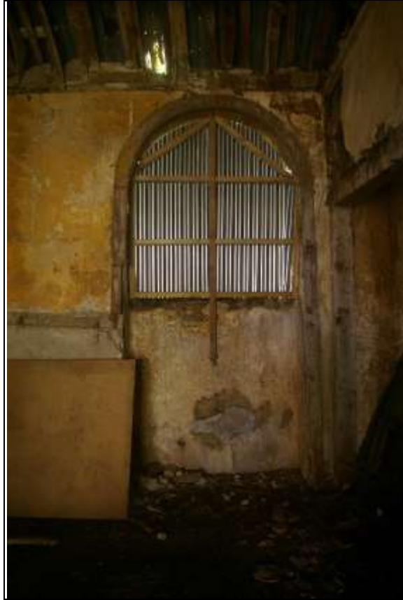
13. THE ROUND-HEADED ALCOVE IN THE NORTH WALL; FROM THE SOUTH.
