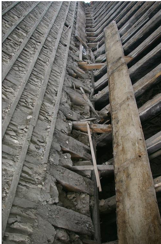
19. THE EXPOSED PLANKS OF THE VALLEY GUTTER; FROM THE EAST.
