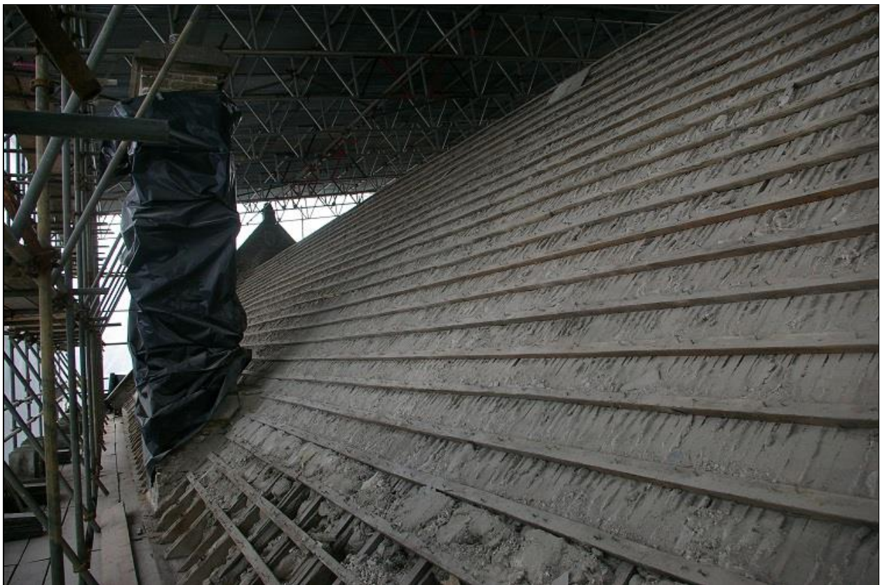
14. THE NORTH FACE OF THE NORTH AISLE ROOF; FORM THE WEST-NORTH-WEST.
