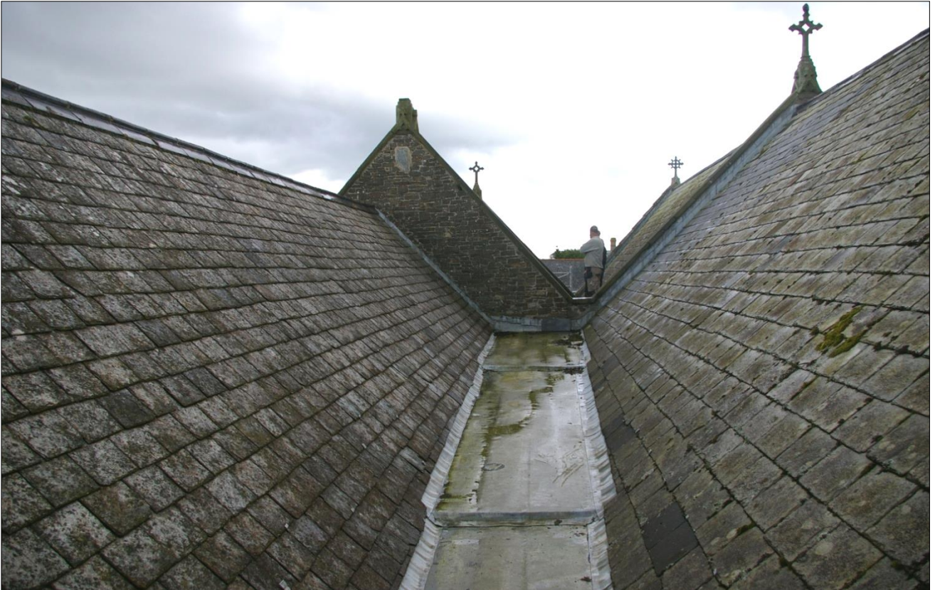
9. THE WIDE END OF THE VALLEY GUTTER WHERE THE NORTH AISLE AND NAVE MEET THE EASTERN PART OF THE CHURCH; VIEWED FROM THE WEST.
