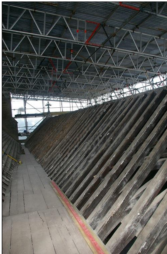
FIGURE 5: THE NORTH AISLE ROOF STRIPPED OF SLATE; FROM THE EAST-NORTH-EAST.
