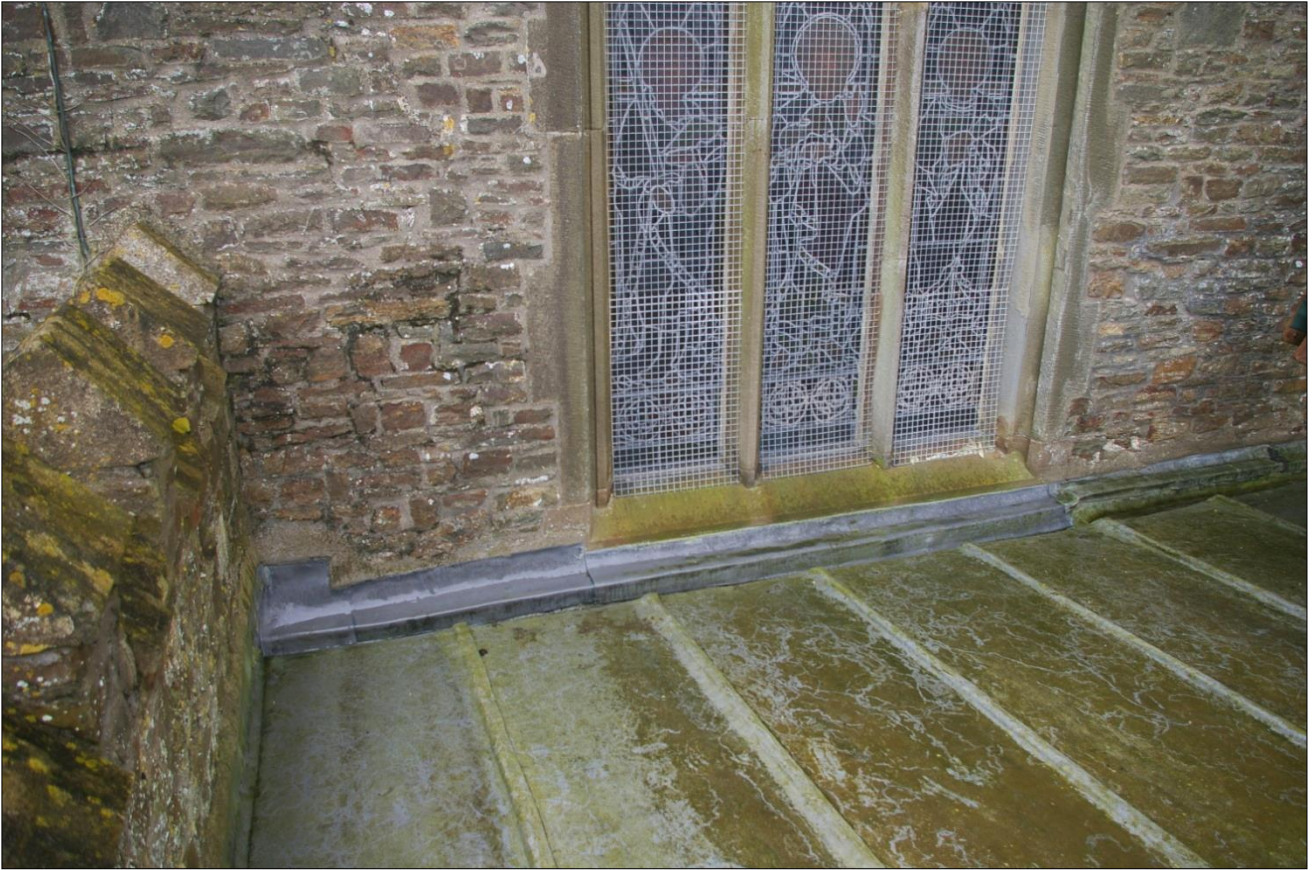
3. THE LEAD BOX DRAIN AND SHALLOW MONOPITCH OF THE ROOF UNDER THE WEST WINDOW OF THE NORTH AISLE; VIEWED FROM THE WEST-NORTH-WEST.
