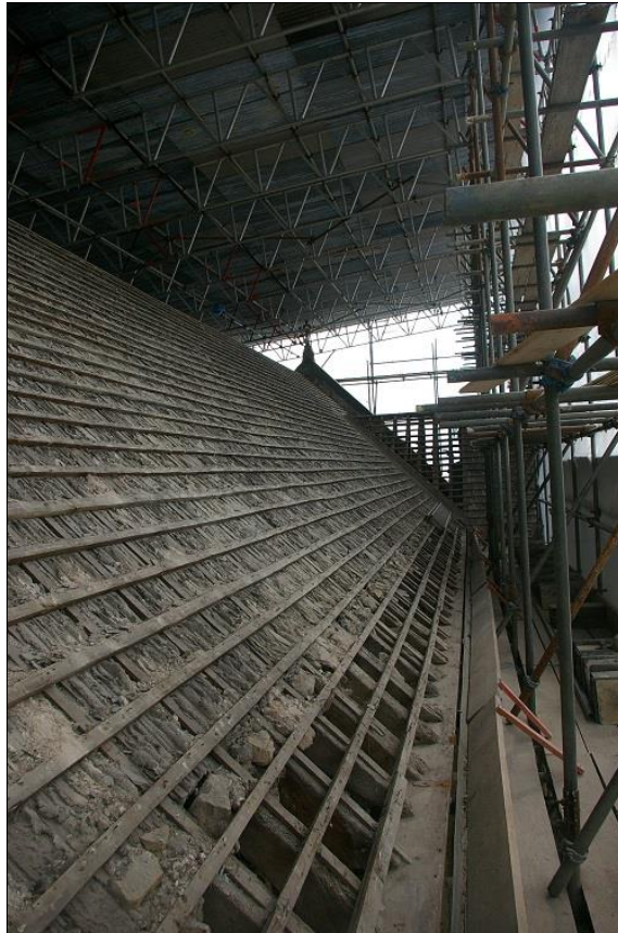
13. THE NORTH FACE OF THE NORTH AISLE ROOF; FROM THE EAST-NORTH-EAST.
