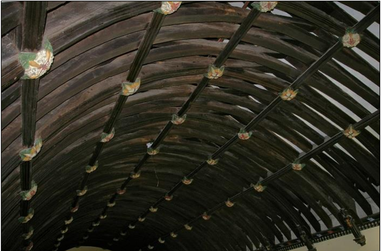
FIGURE 3: THE INTERIOR OF THE NAVE ROOF; FROM THE NORTH-WEST.
