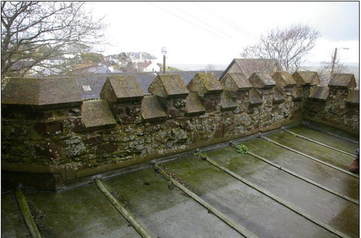
FIGURE 2: THE ROOF AND CRENELATIONS OF THE VESTRY; FROM THE SOUTH-EAST.
