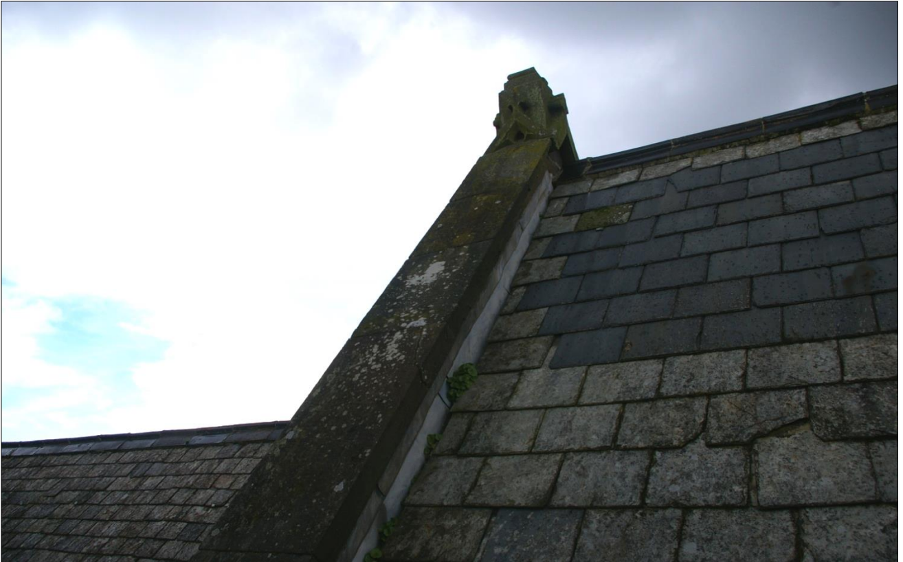
11. THE RAISED GABLE BETWEEN THE NORTH AISLE TO THE LEFT AND THE HIGHER PROFILE OF THE ROOF OF THE LAY CHAPEL TO THE RIGHT, SHOWING HOW OFFSET THE ROOF OF THE NORTH AISLE IS IN COMPARISON TO THE REST; VIEWED FROM THE SOUTH-EAST.
