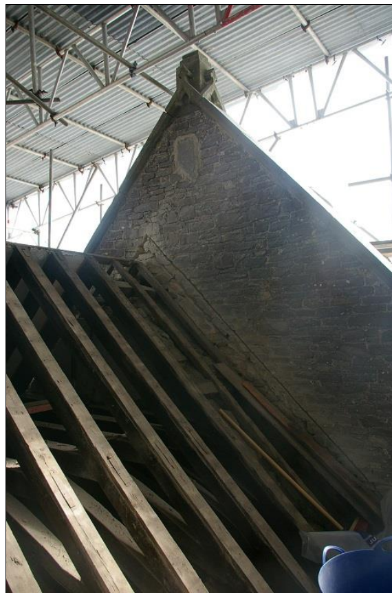
16. THE ROOFLINE SCAR AND SOCKET HOLE ON THE NORTH AISLE, EAST END; FROM THE SOUTH-WEST.
